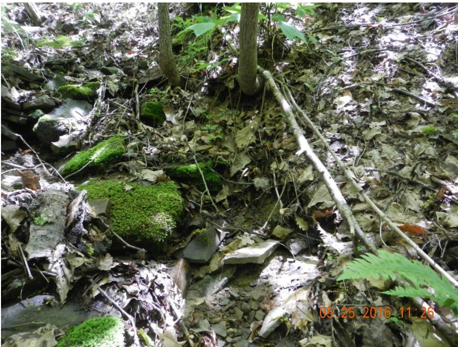
Waterbody SPOA410 scouring facing east
