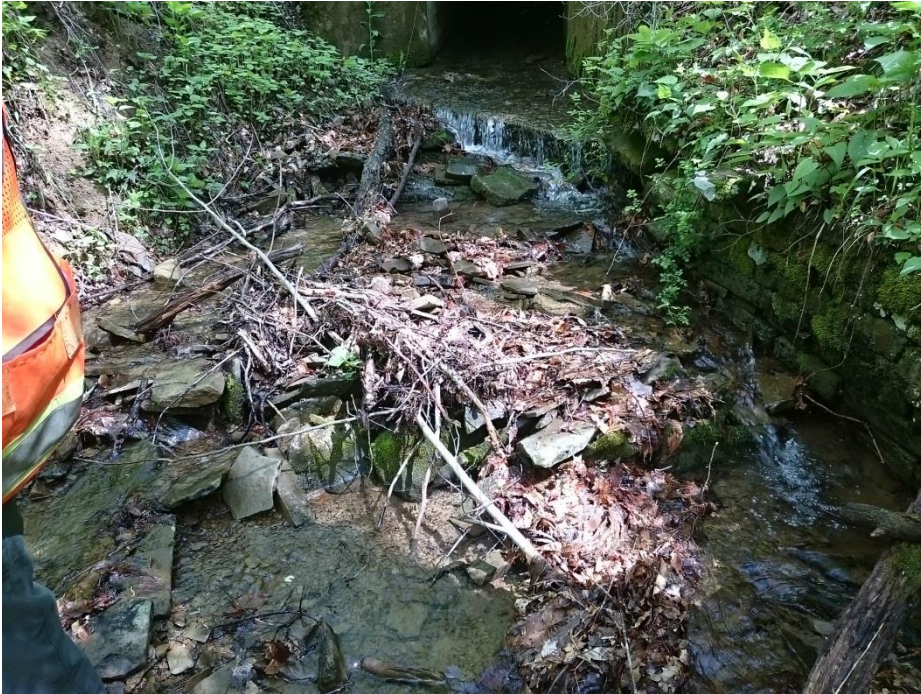
Waterbody SPOA404 facing north upstream
