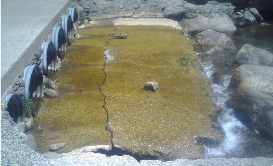
Waterbody spoe048 facing north across
