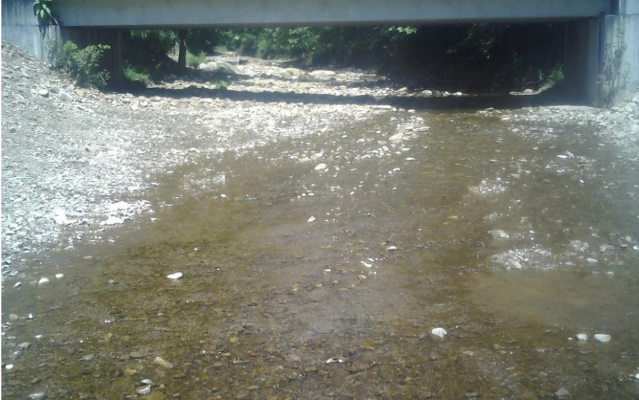
Waterbody spoe048 facing west upstream
