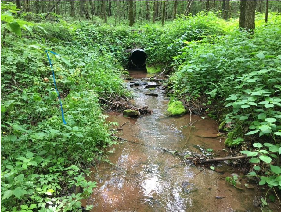
Waterbody SPOA427 facing southwest upstream
