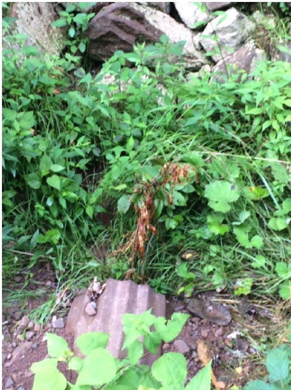
Waterbody SPOE031 facing west upstream
