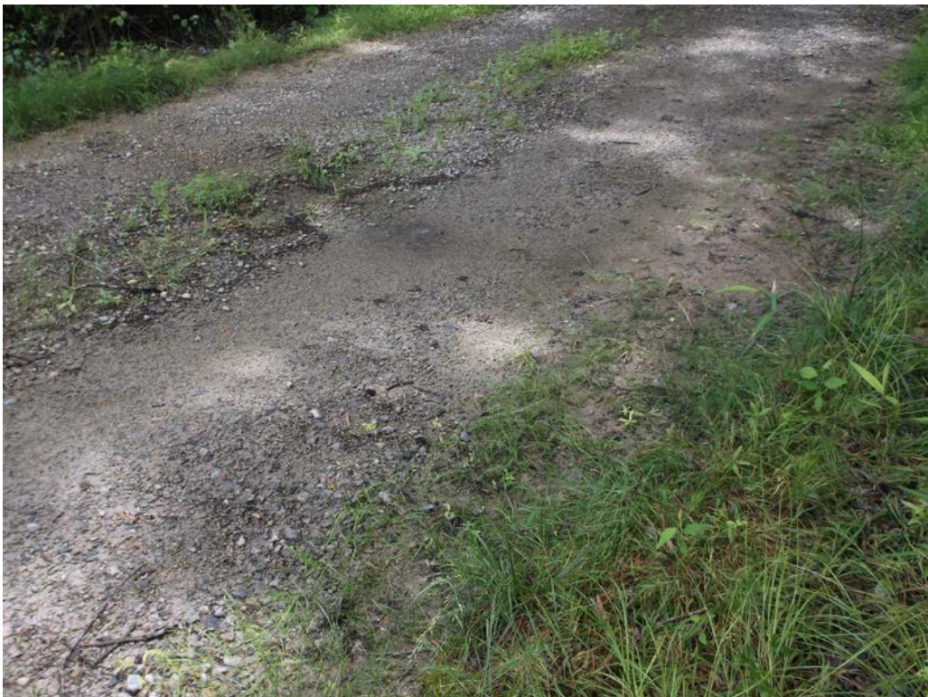
Upland data point wnrp017_u facing northeast.
