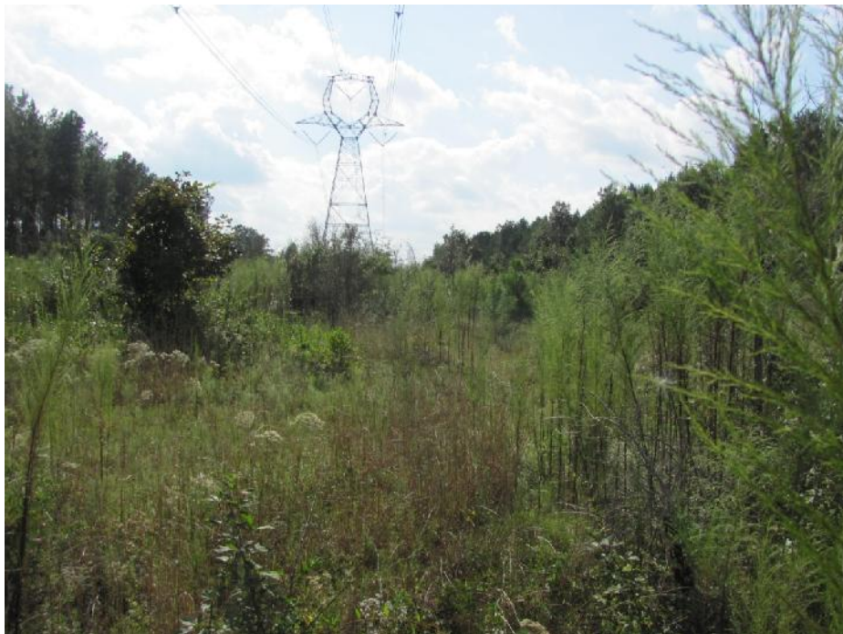
Upland data point wcmh004_u facing south
