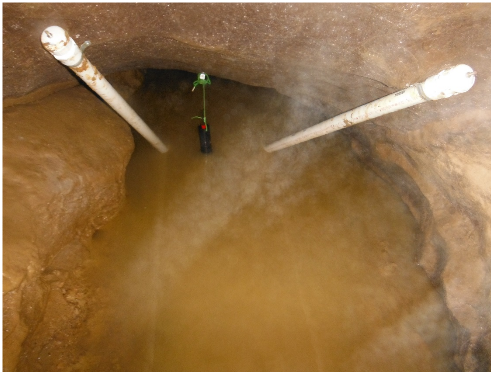
Figure 2. Installed Data Loggers
