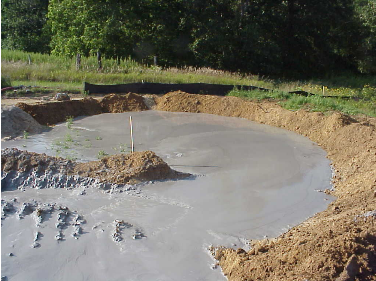
Figure 4. Inadvertent Drilling Fluid Return
