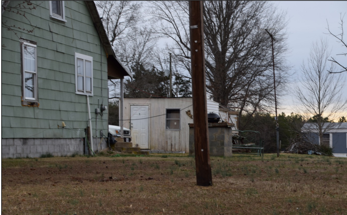
Figure 16. 014-5090, wood shed, facing southeast.
