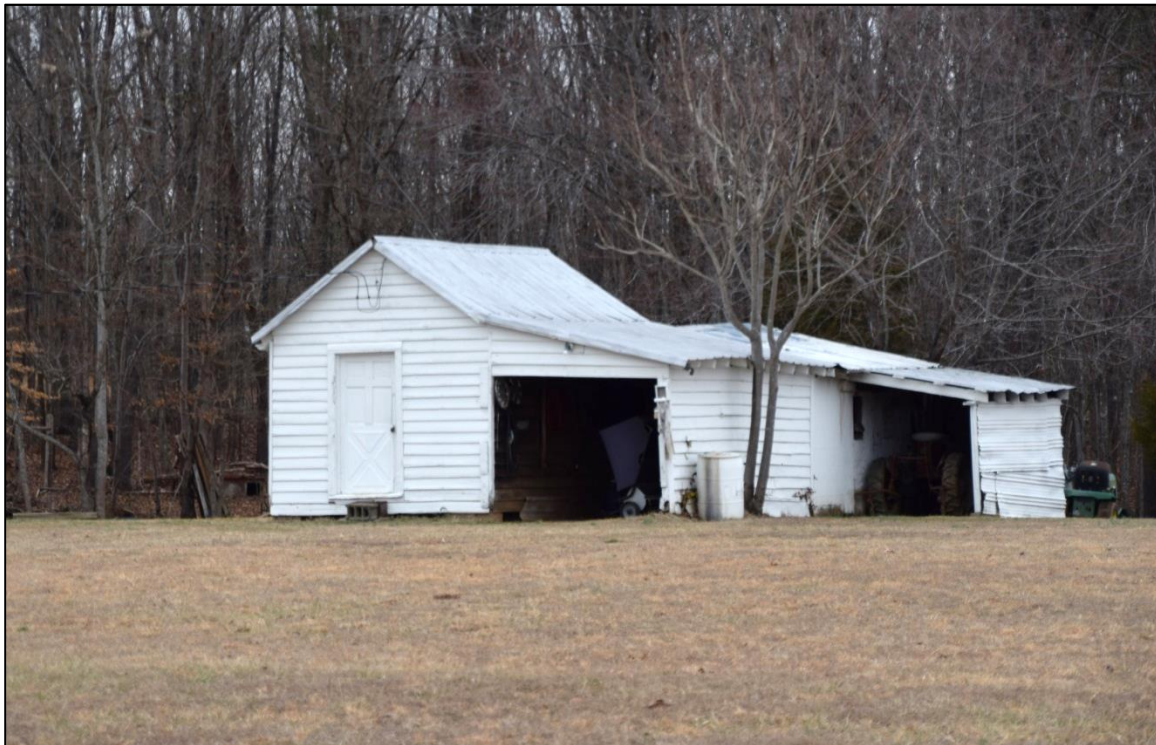
Figure 11. 014-5089, shed facing northwest.
