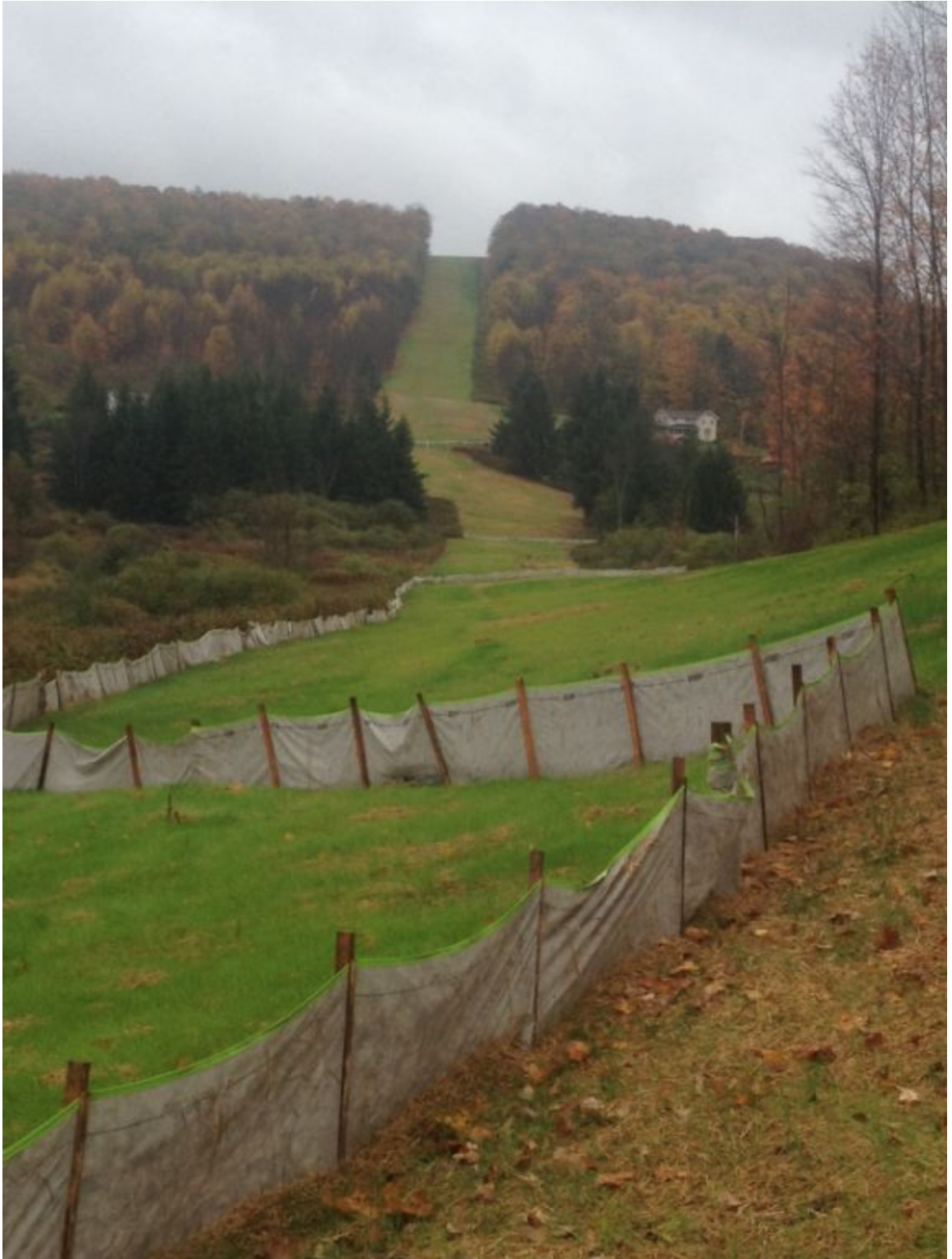
Figure 23 - TL 610, Restored Right of Way
