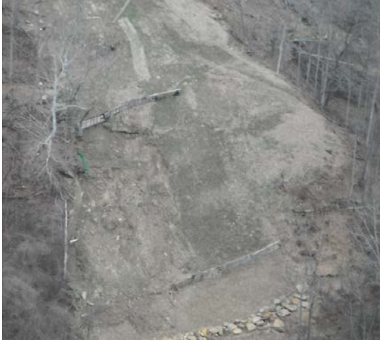
Soil movement following event – Aerial view
