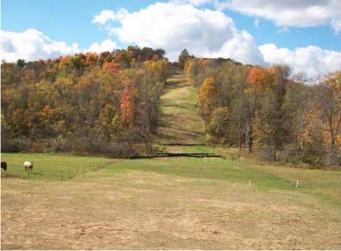
Figure 9 - TL 492 Ext 4, Restored Right of Way
