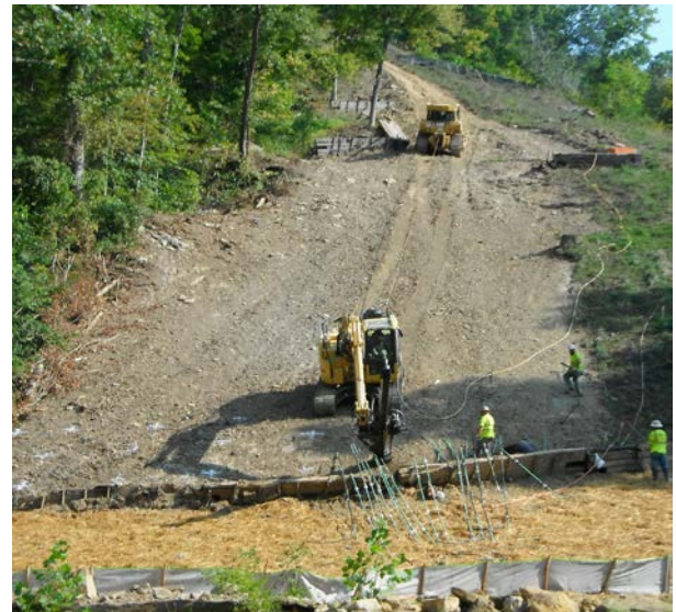
Restoration operations – Installation of soil nails
