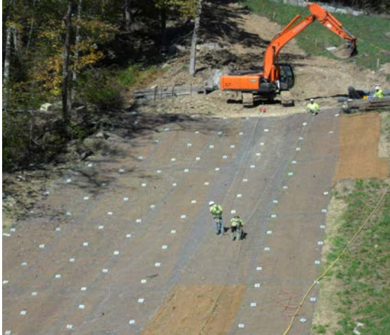
Restoration operations – Installation of soil nails with TECO mesh
