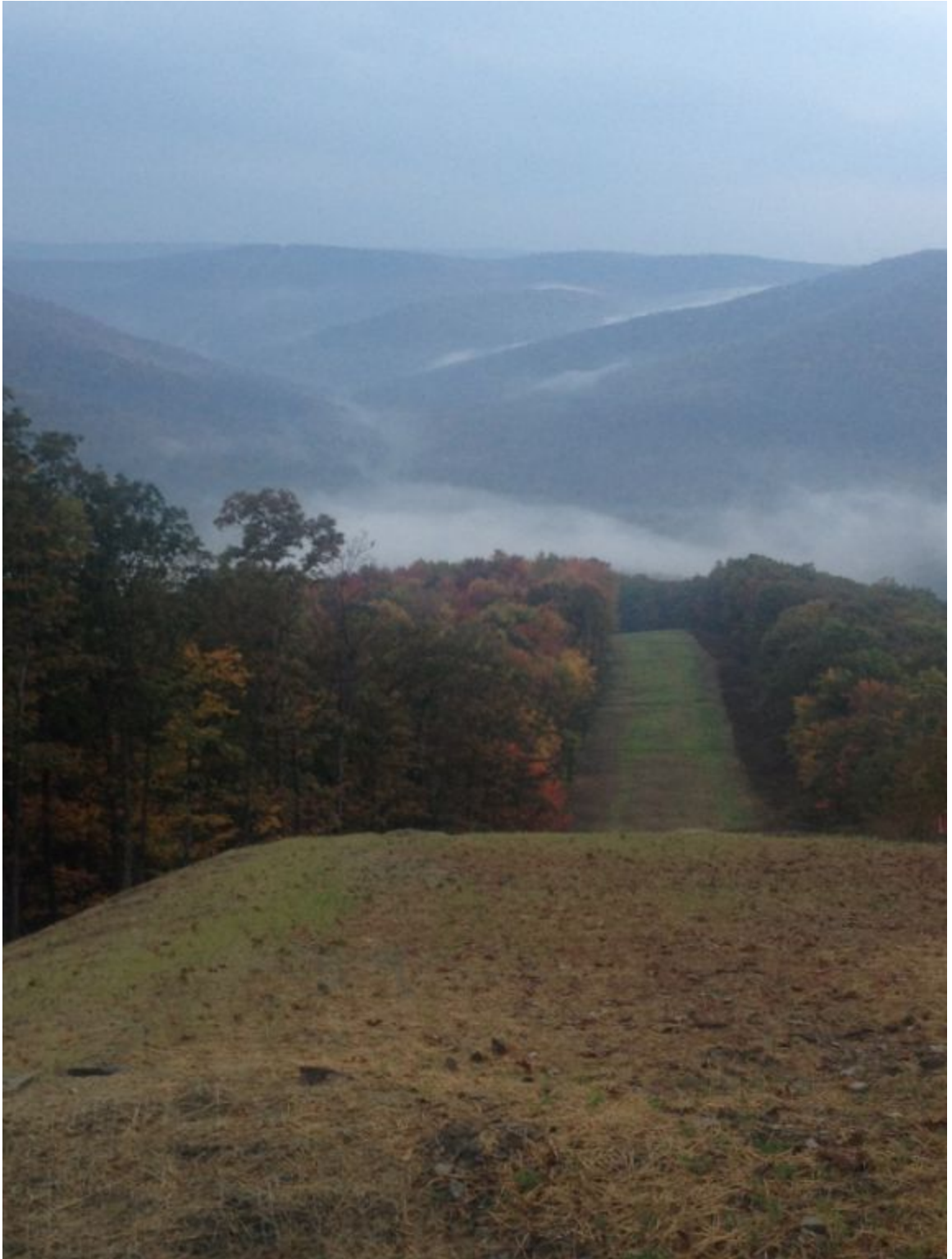
Figure 21 - TL 610 Ext 1, Restored Right of Way
