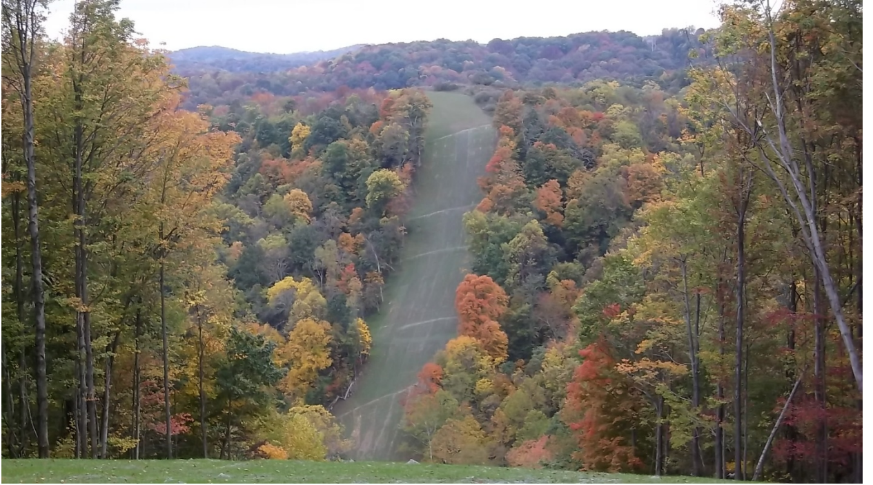
Figure 13 - TL 590, Restored Right of Way
