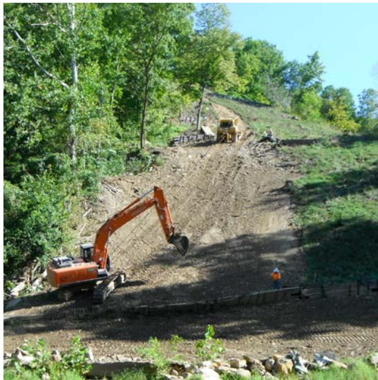
Restoration operations – final grading
