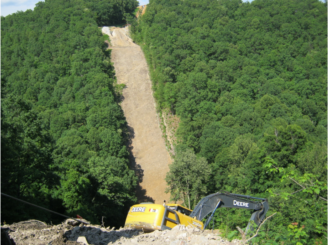
Figure 6 - TL 585, Final Grade Established
