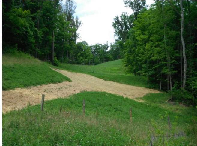
Fish Creek Slip Repair
