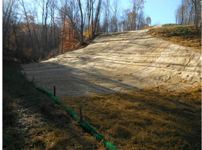
Burch Ridge Slip Repair
