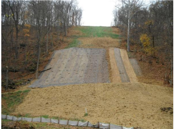
Grave Creek Slip Repair
