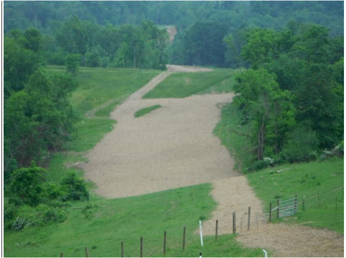
Access Road Slip Repair
