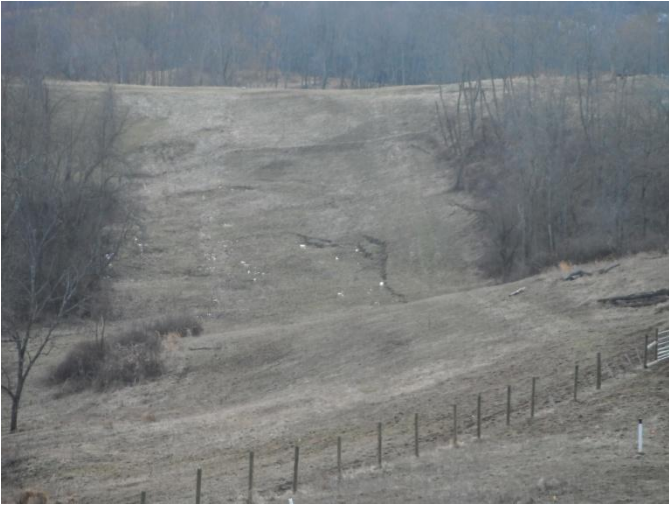
Access Road Slip
