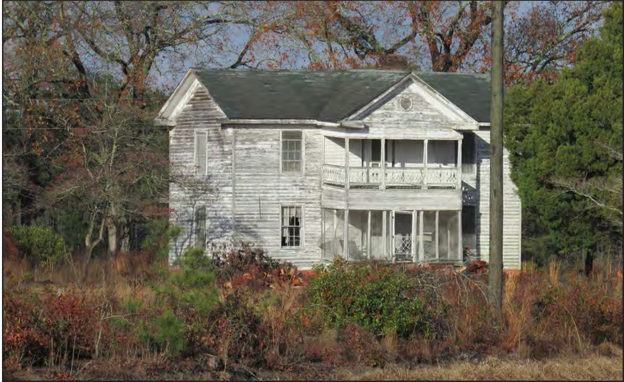
Photo 165. RB0678, house, facing northwest.
