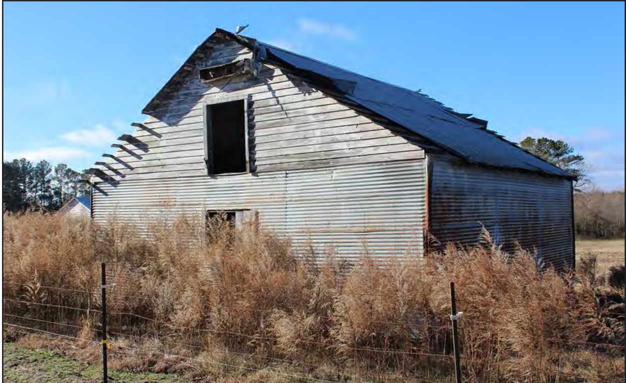
Photo 38. HX0229, facing southwest.
