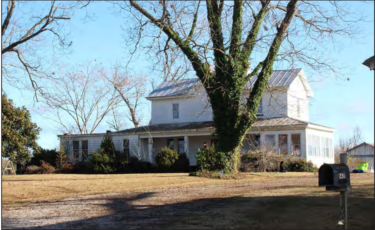
Photo 27. HX0227, main house, facing northeast.
