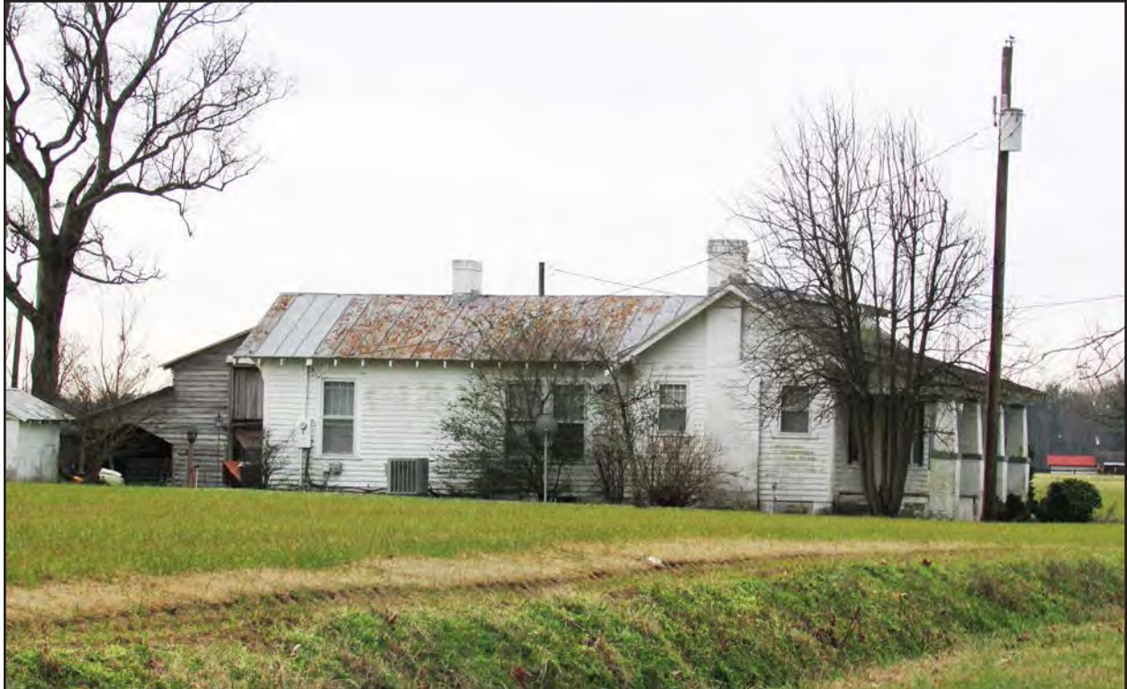
Photo 162. NS1517, dwelling, facing southwest.
