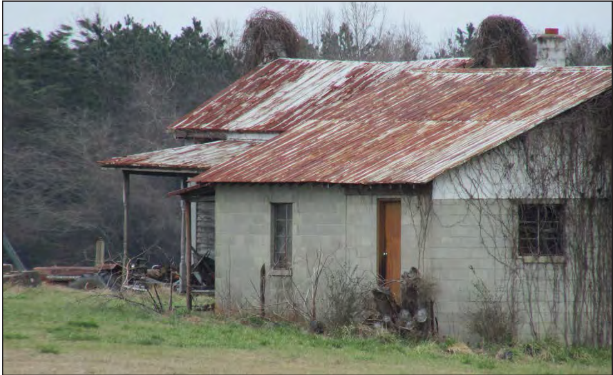
Photo 149. NS1504, facing northeast.
