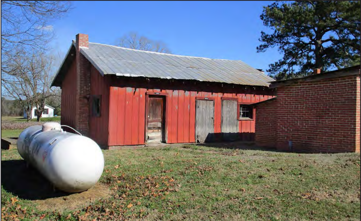
Photo 22. HX0021, wash room/laundry, facing northeast.
