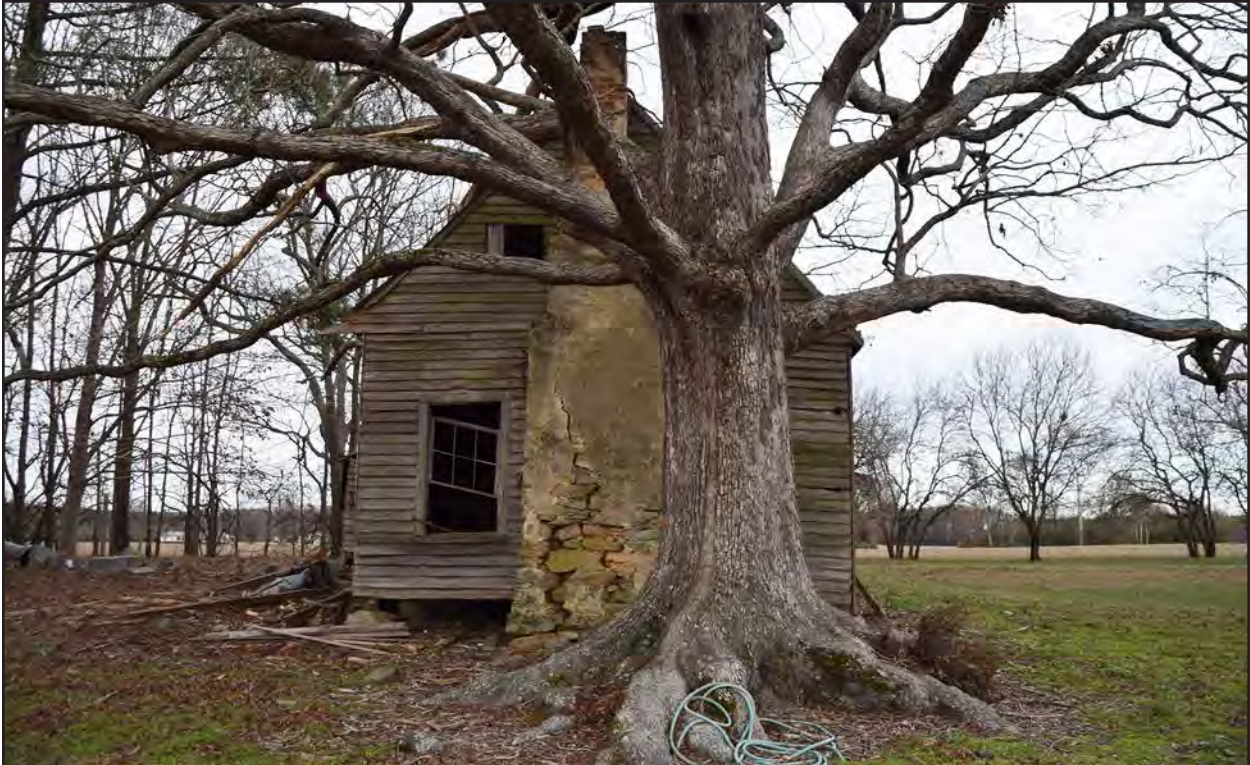
Photo 132. NS0650, cabin, facing east.
