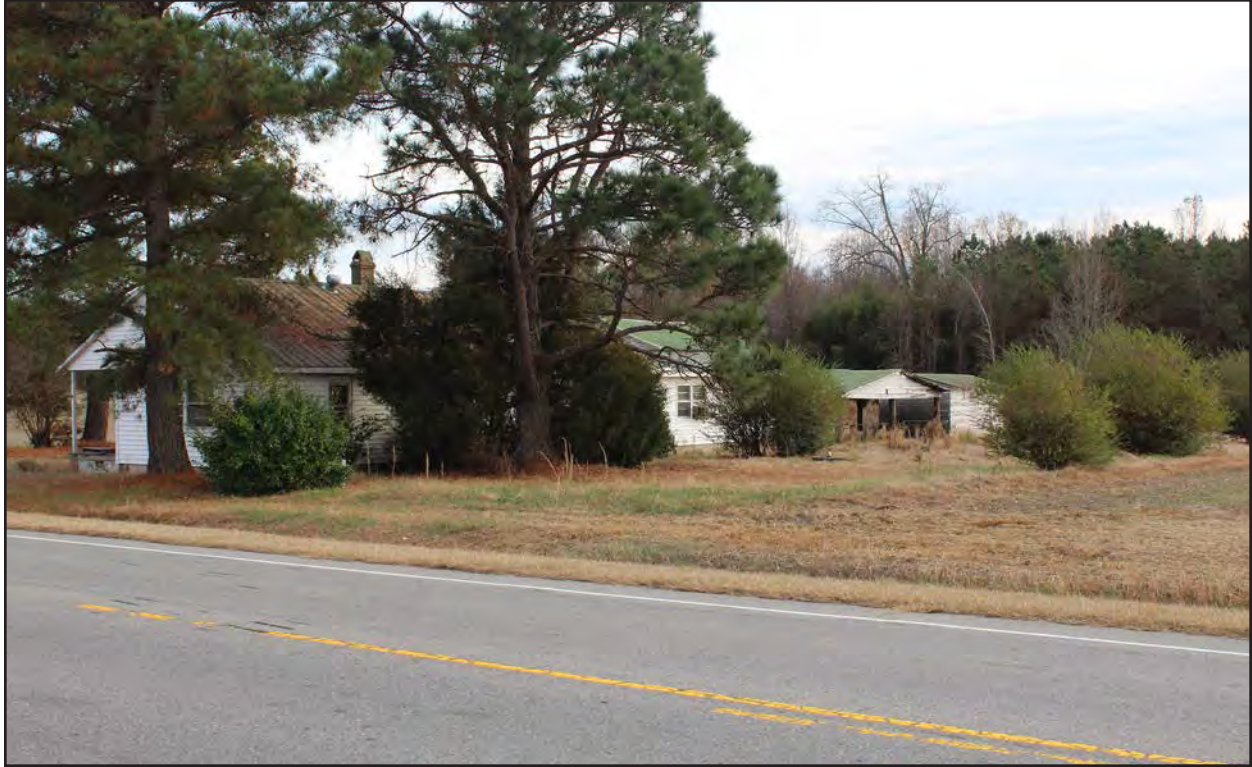
Photo 79. JT1864, house with rear wings, facing southeast.
