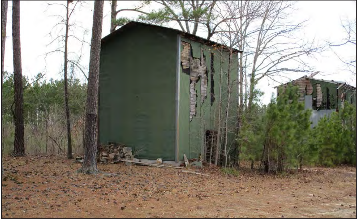
Photo 153. NS1508, ca. 1950–1960s storage structure, facing northwest.
