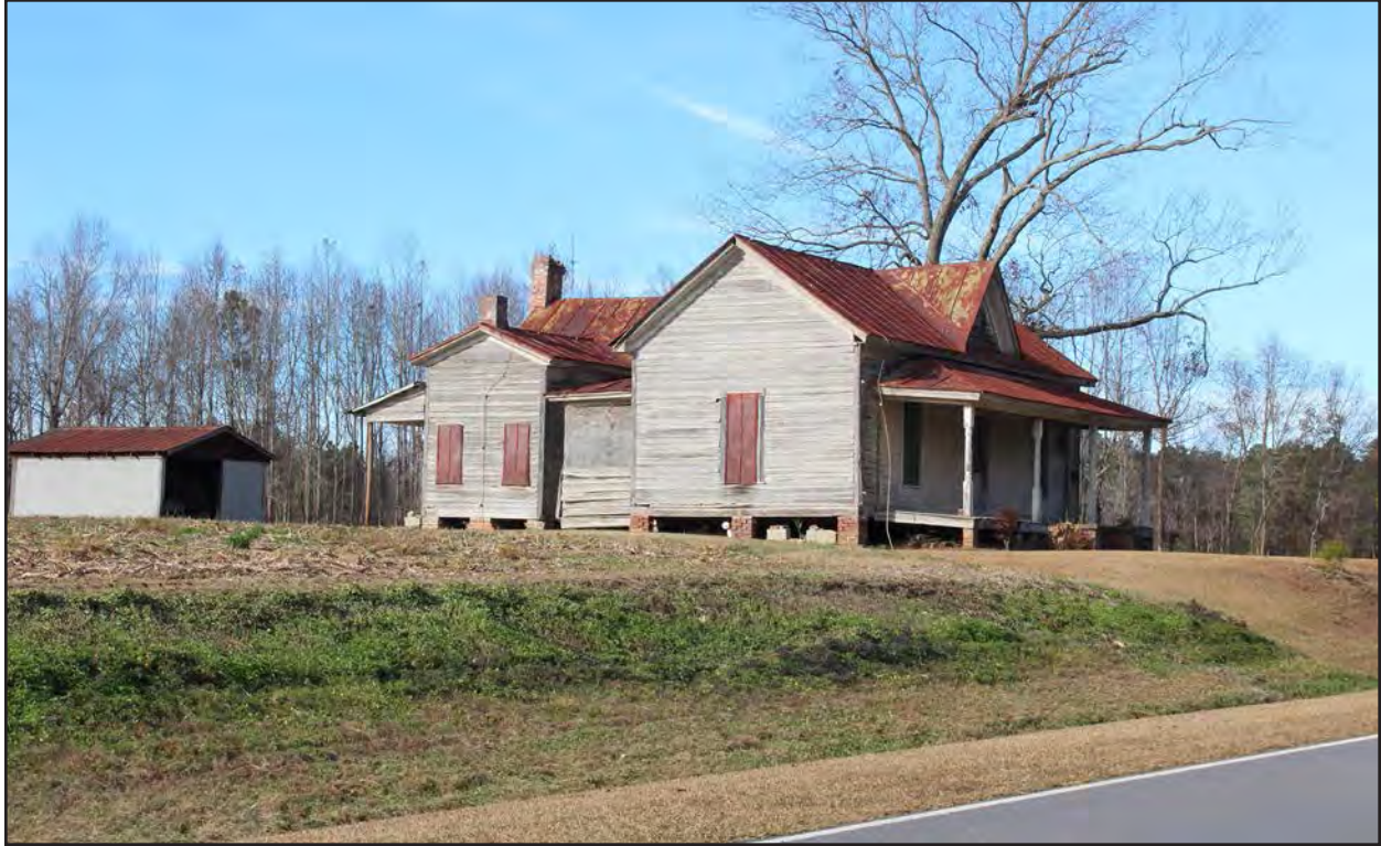
Photo 181. WL2012, facing north-northwest.
