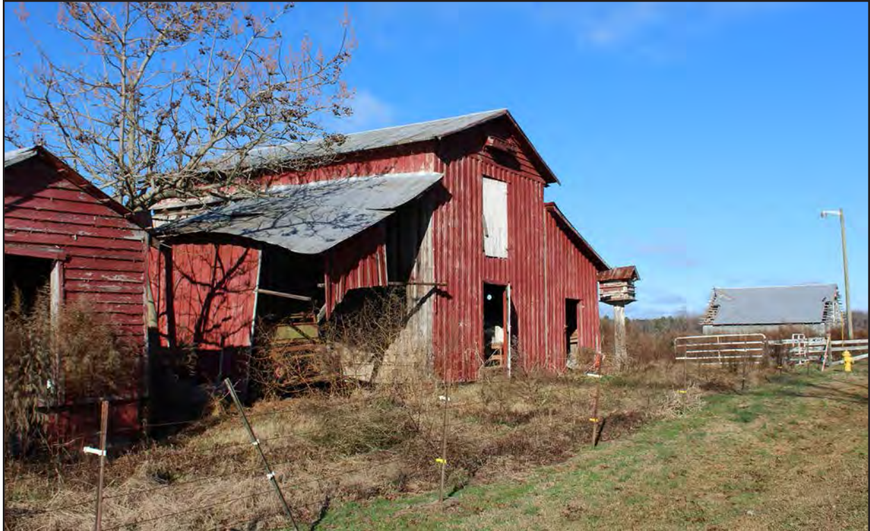
Photo 36. HX0229, facing north-northwest.
