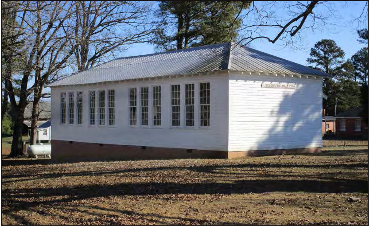
Photo 41. HX1556 (Allen Grove Rosenwald School), facing east.
