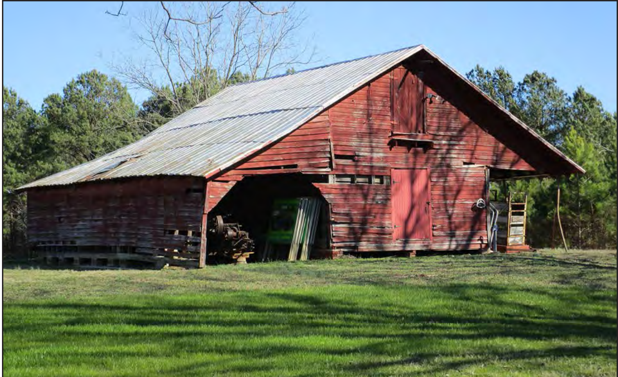
Photo 14. HX0021, corn and equipment barn, facing east-northeast.
