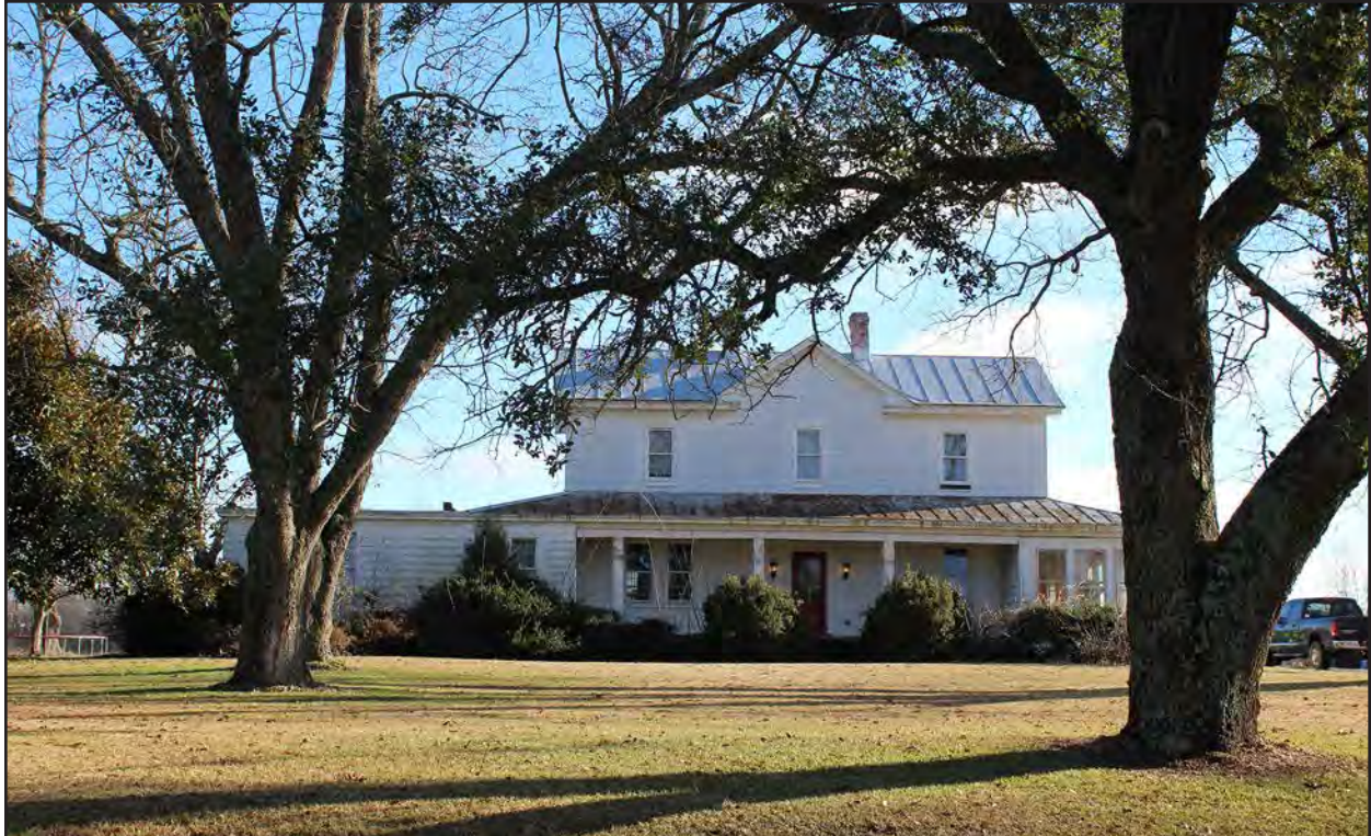
Photo 26. HX0227, main house, facing east.
