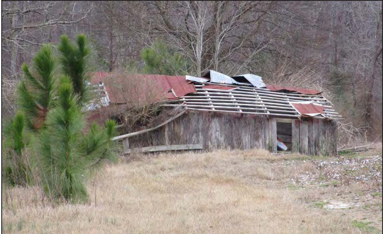
Photo 52. HX1581, storage structure, facing south.
