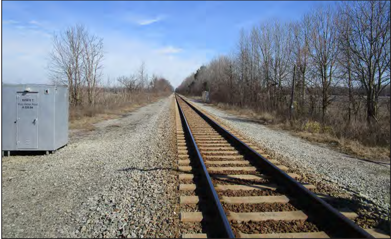
Photo 1. CD1450 (Fayetteville Cutoff), facing west.
