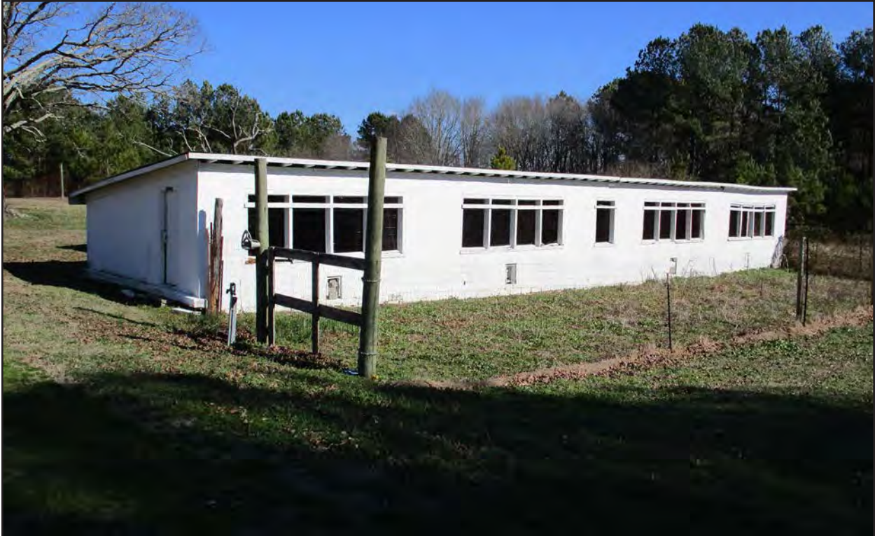
Photo 16. HX0021, chicken house, facing east.
