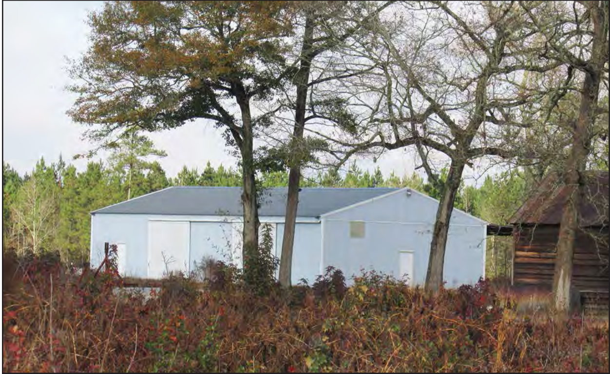
Photo 169. RB0678, agricultural/storage outbuilding, facing north.
