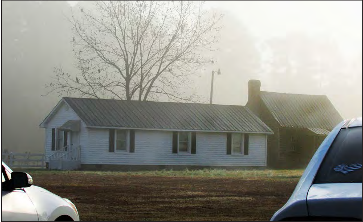
Photo 93. JT1920, accessory structure 2, facing southeast.
