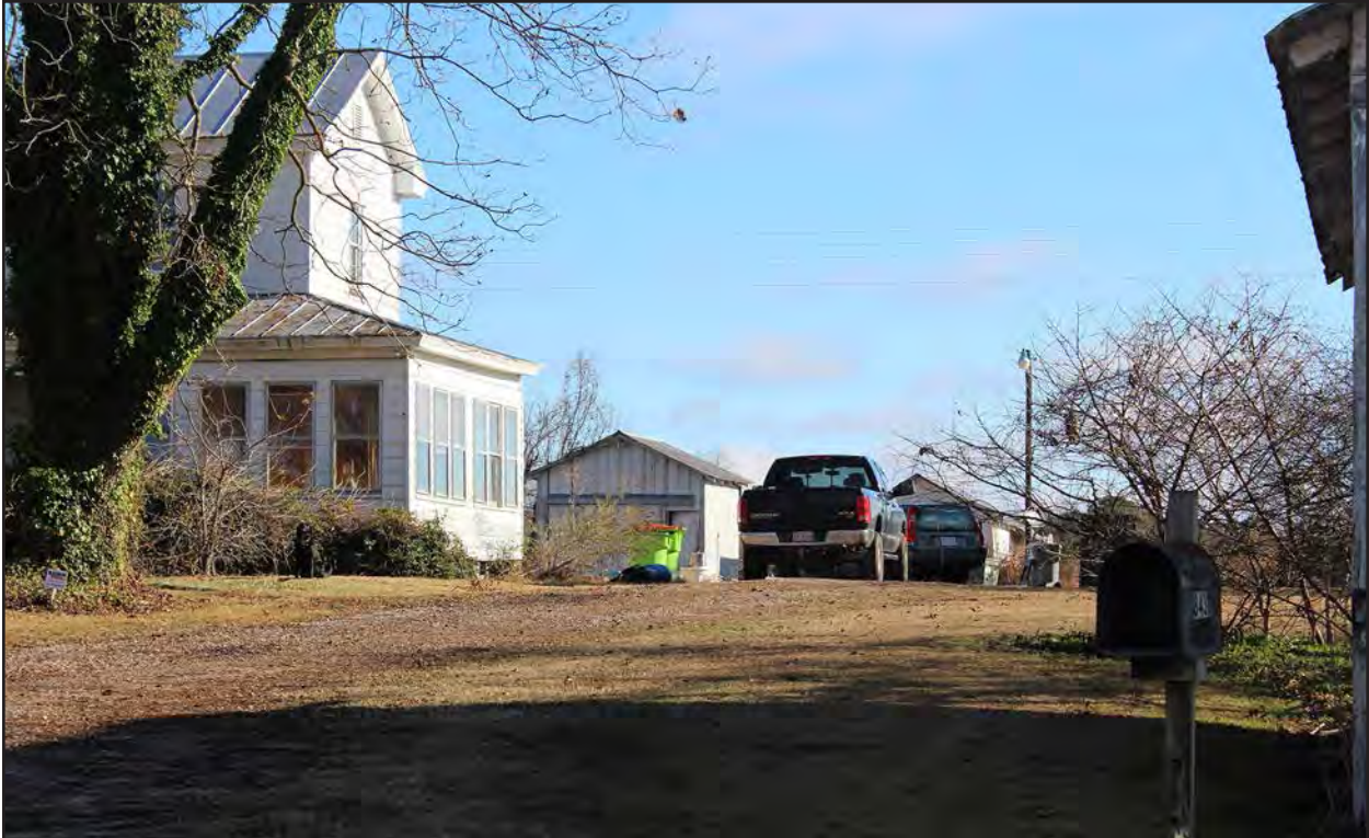
Photo 30. HX0227, rear accessory structure, facing east.
