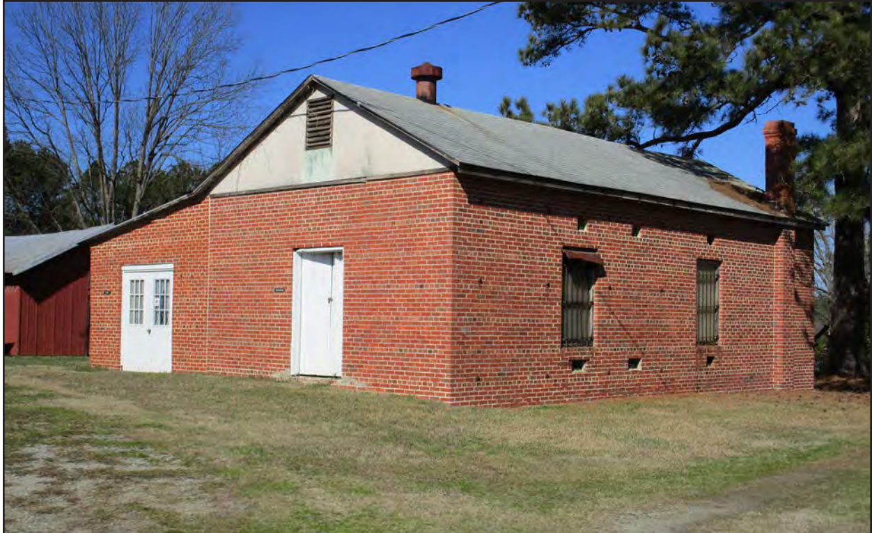
Photo 18. HX0021, smokehouse, facing north.
