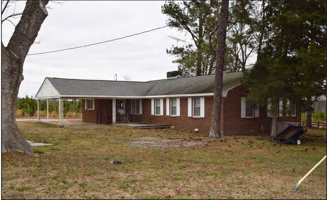
Photo 45. HX1581, facing northeast.
