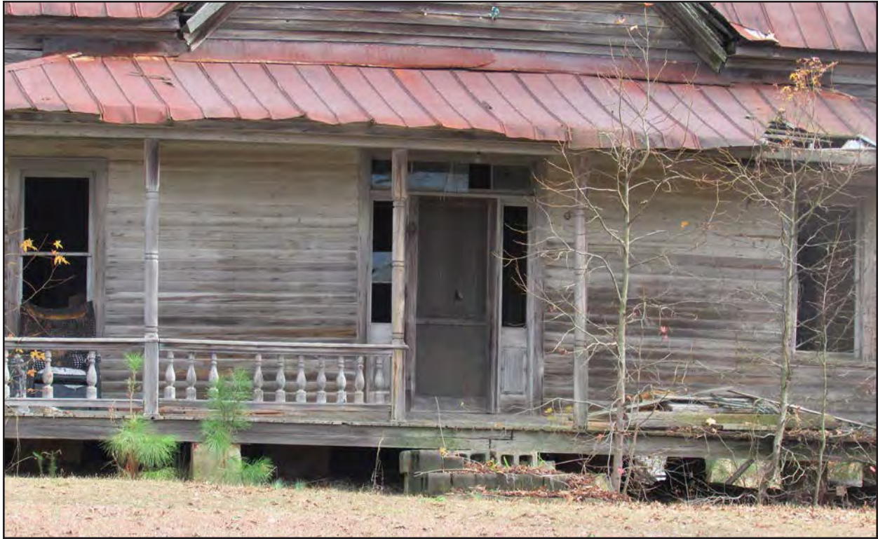
Photo 115. JT1937, main entrance facing east.
