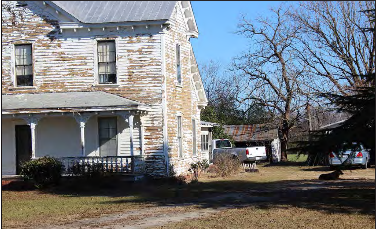
Photo 66. JT0957, gabled accessory structure 2, facing east-northeast.
