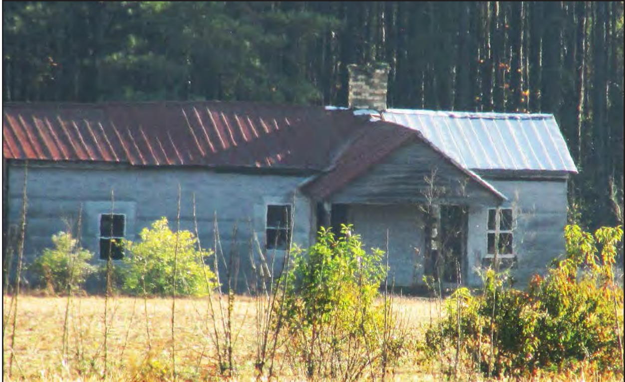
Photo 172. RB0680, house, porch detail.
