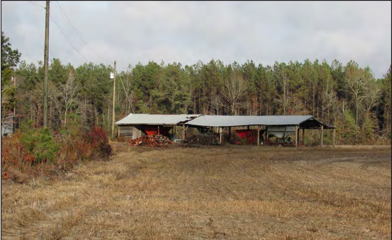
Photo 168. RB0678, pole shelters, facing northeast.
