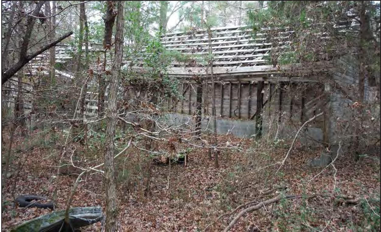
Photo 58. HX1597, barn, facing north.
