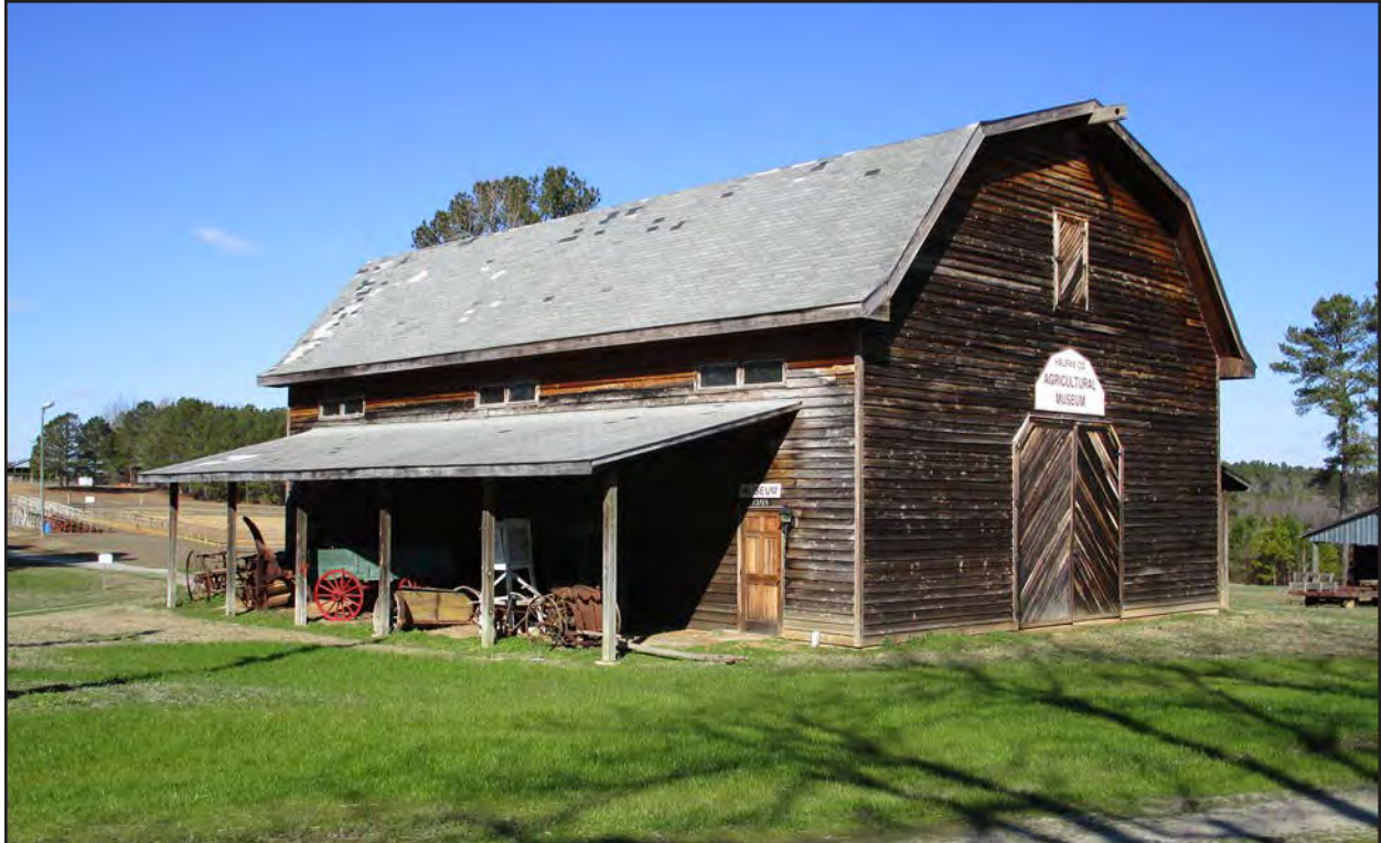
Photo 10. HX0021, barn, facing north.
