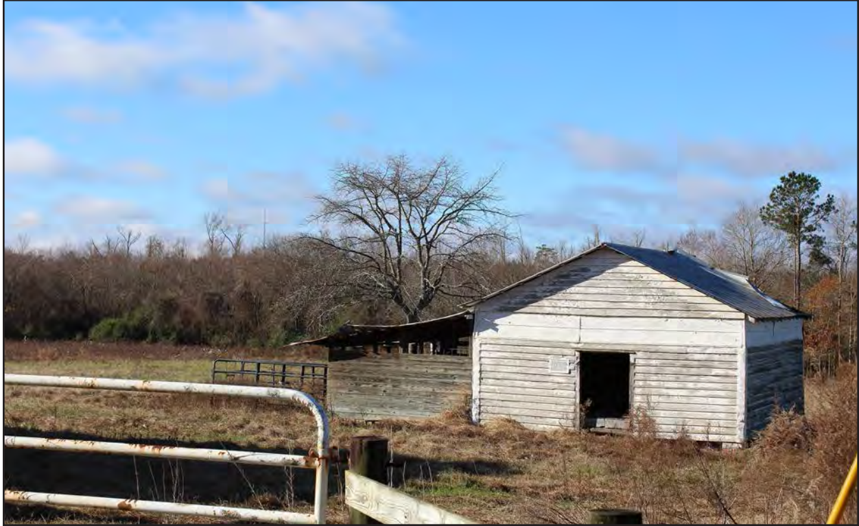
Photo 37. HX0229, facing southwest.
