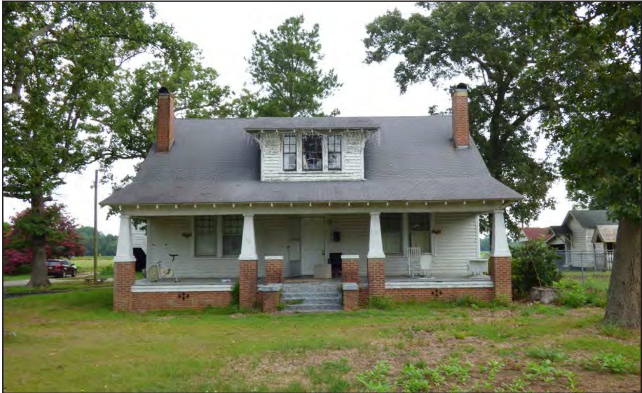
Photo 137. NS1493, dwelling, facing north.
