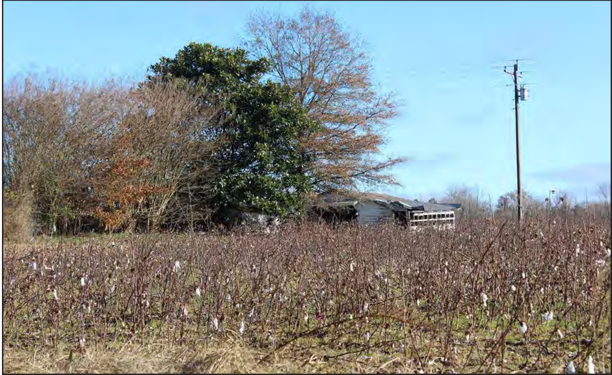
Photo 31. HX0227, rear accessory structure, facing northeast.
