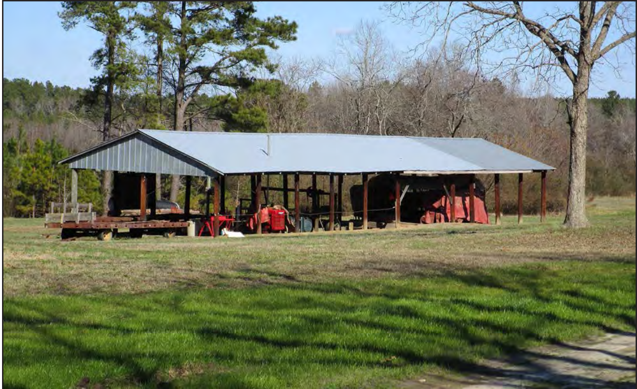
Photo 12. HX0021, equipment shed, facing north-northeast.
