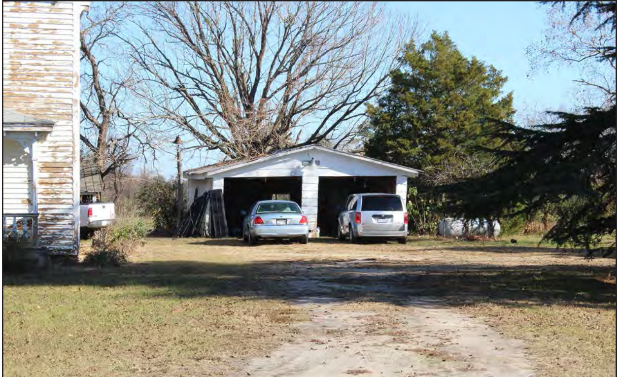
Photo 64. JT0957, garage, facing east.
