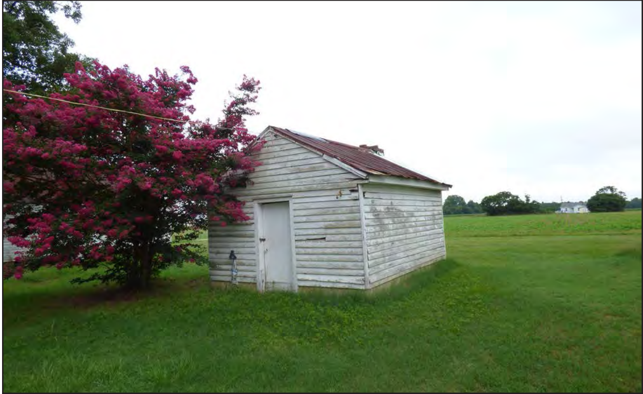
Photo 141. NS1493, agricultural outbuilding, facing northwest.
