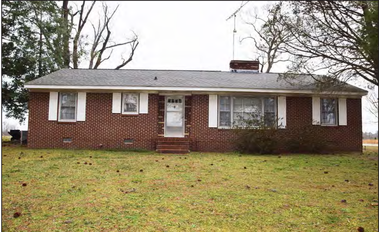
Photo 44. HX1581, facing north-northwest.
