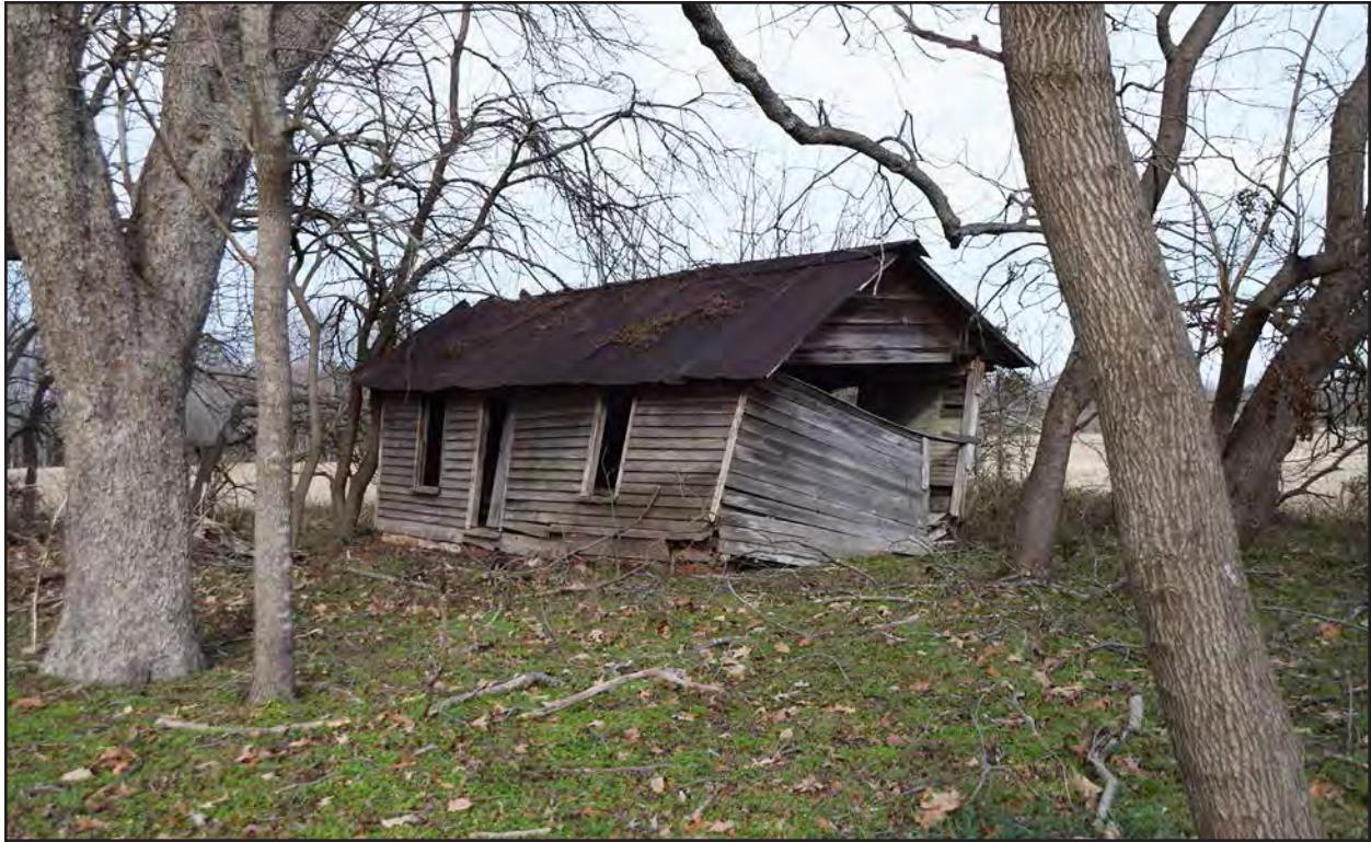
Photo 133. NS0650, summer kitchen, facing northeast
