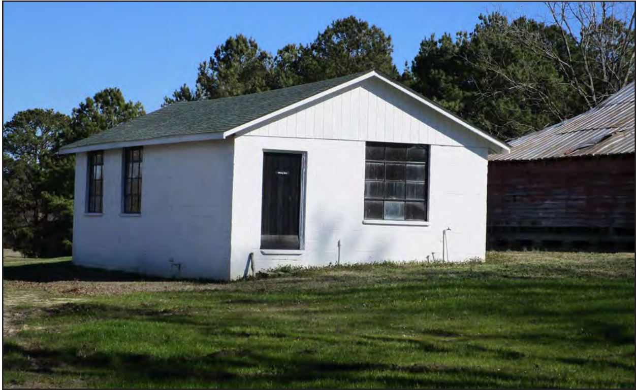
Photo 13. HX0021, milking barn, facing northeast.
