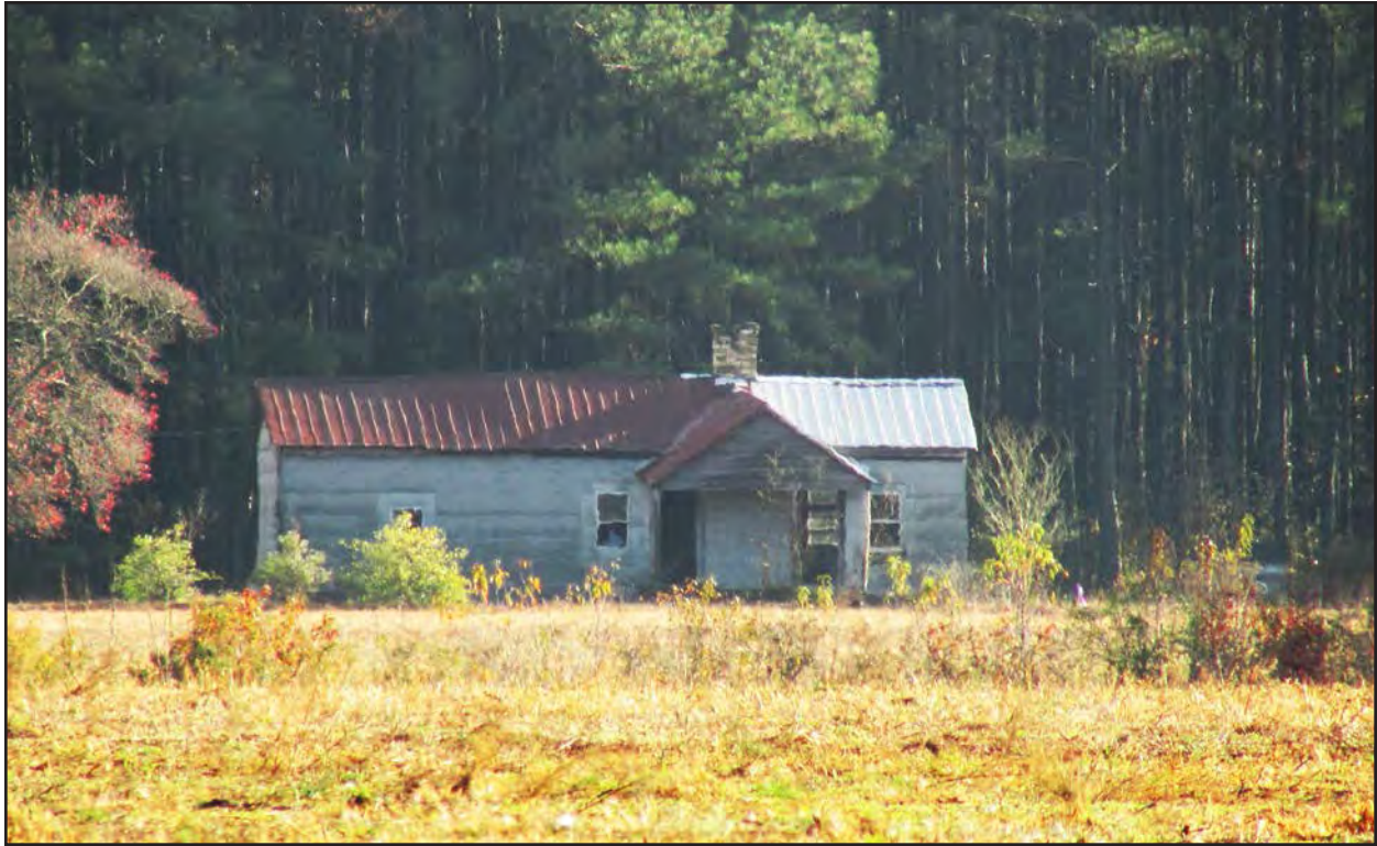
Photo 171. RB0680, house, facing southeast.
