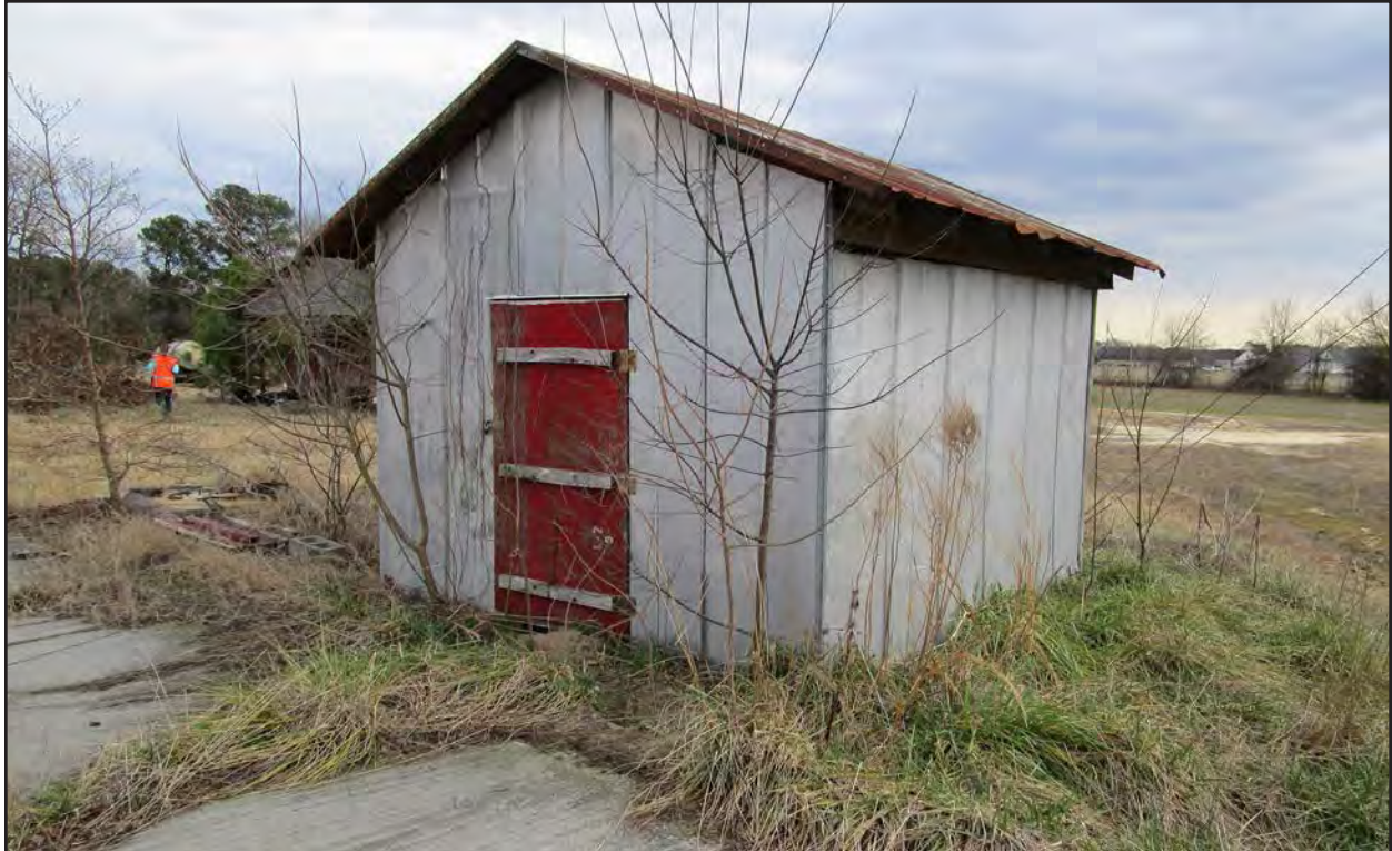
Photo 158. NS1508, ca. 1960 structure, facing southwest.
