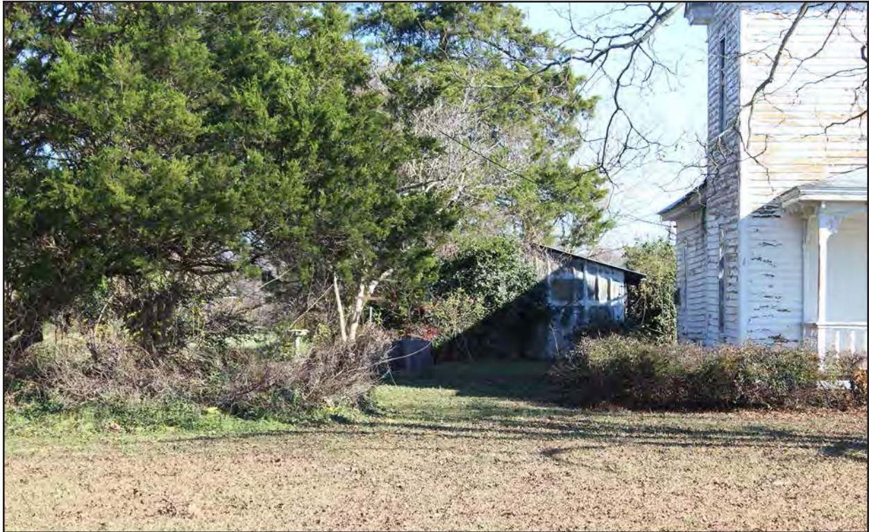
Photo 65. JT0957, gabled accessory structure 1, facing east.
