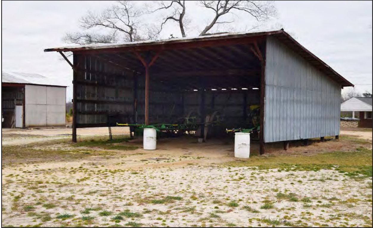
Photo 49. HX1581, equipment shelter, facing northeast.
