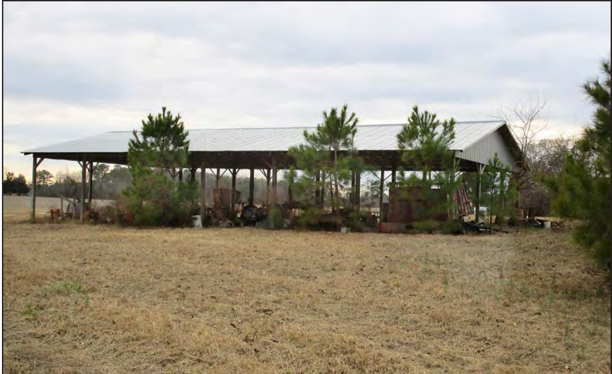
Photo 160. NS1508, pole shed, facing southwest.
