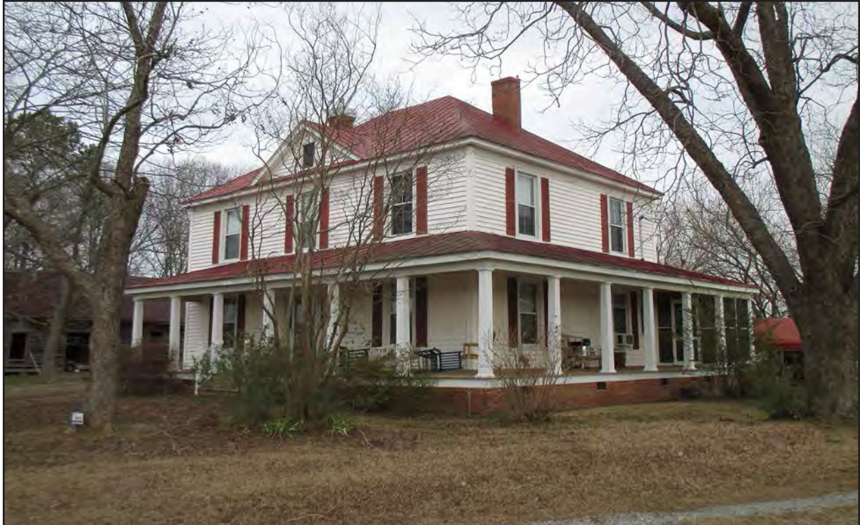
Photo 124. NS0650, house, facing northeast.
