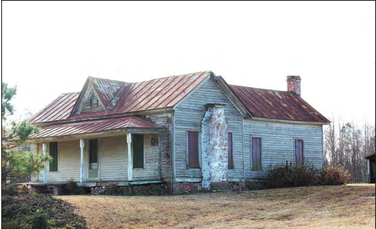
Photo 180. WL2012, facing southwest.
