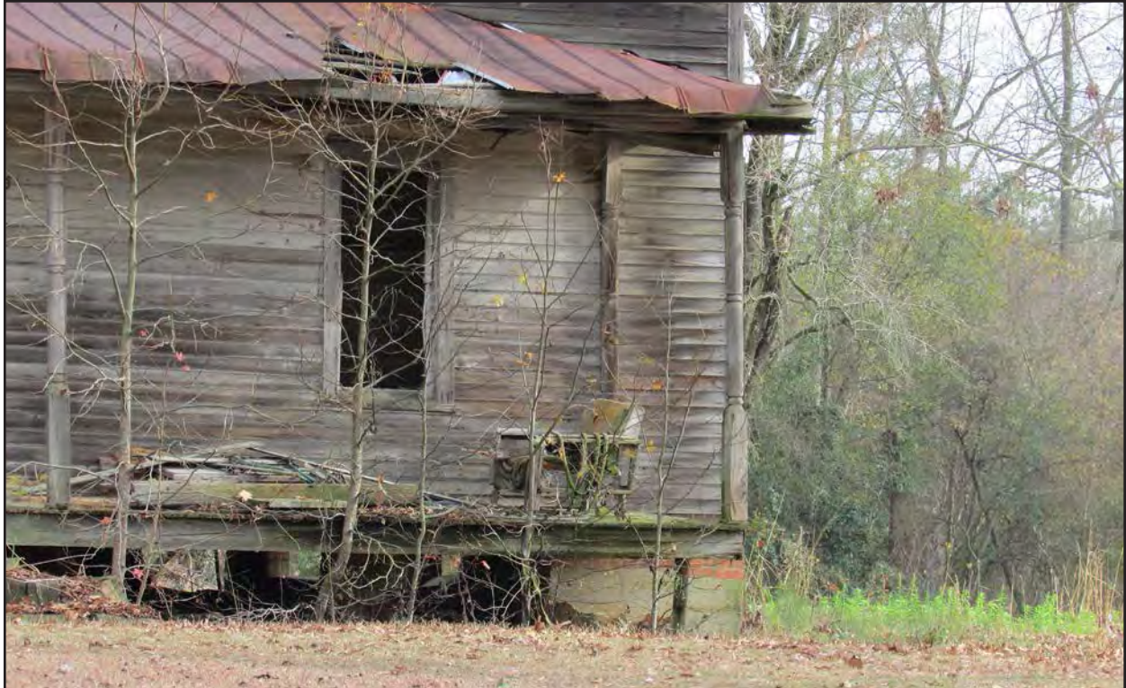
Photo 112. JT1937, foundation, facing southeast.
