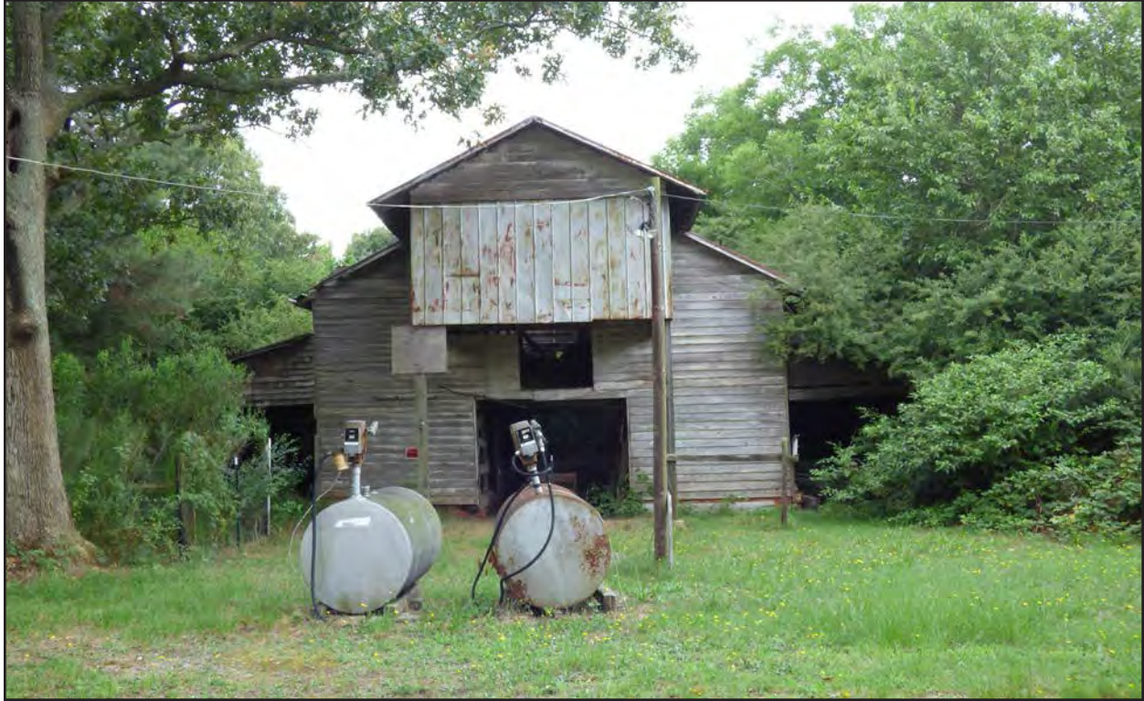
Photo 139. NS1493, hay barn, facing west.
