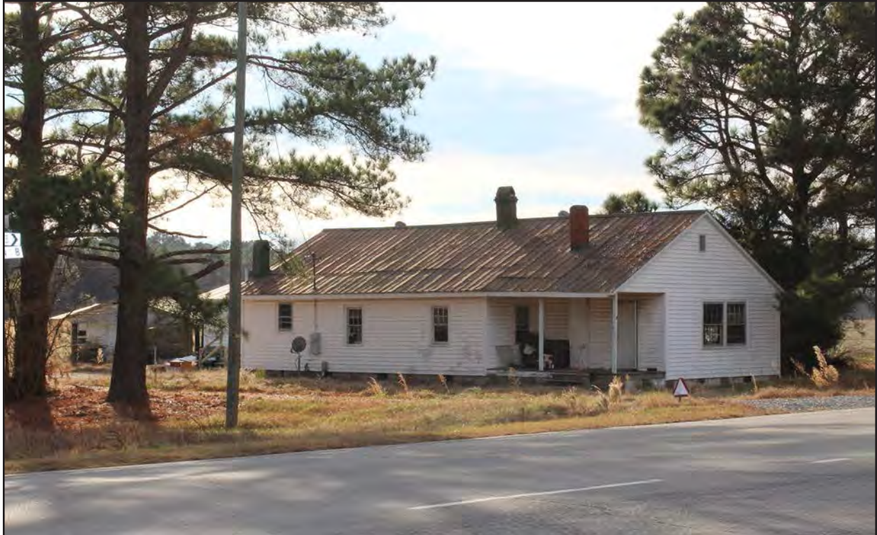
Photo 78. JT1864, house, facing southwest.
