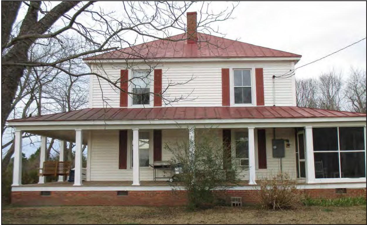
Photo 125. NS0650, house, facing north.
