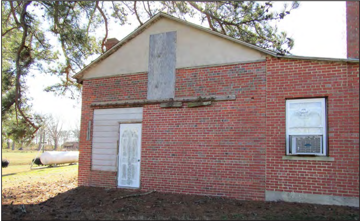
Photo 19. HX0021, barn door on smokehouse, facing south.
