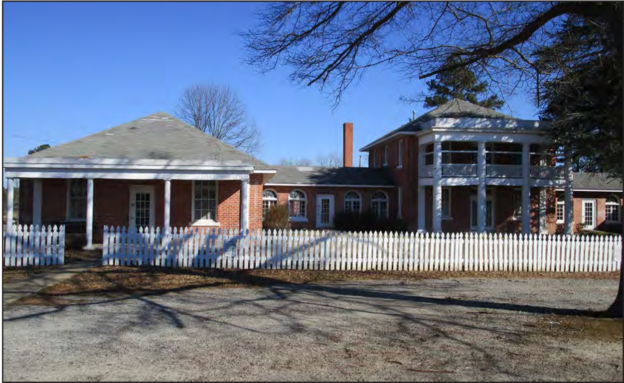
Photo 7. HX0021, facing northeast.
