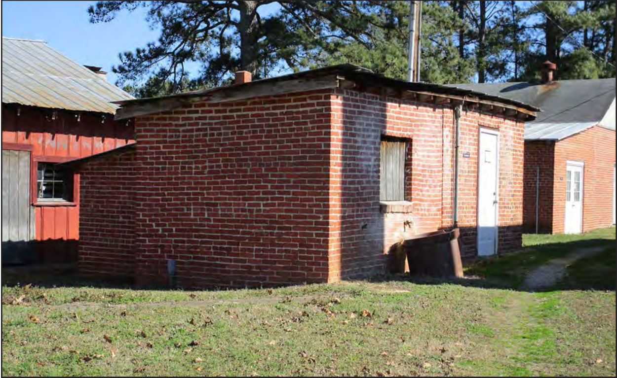
Photo 21. HX0021, pumphouse, facing east.
