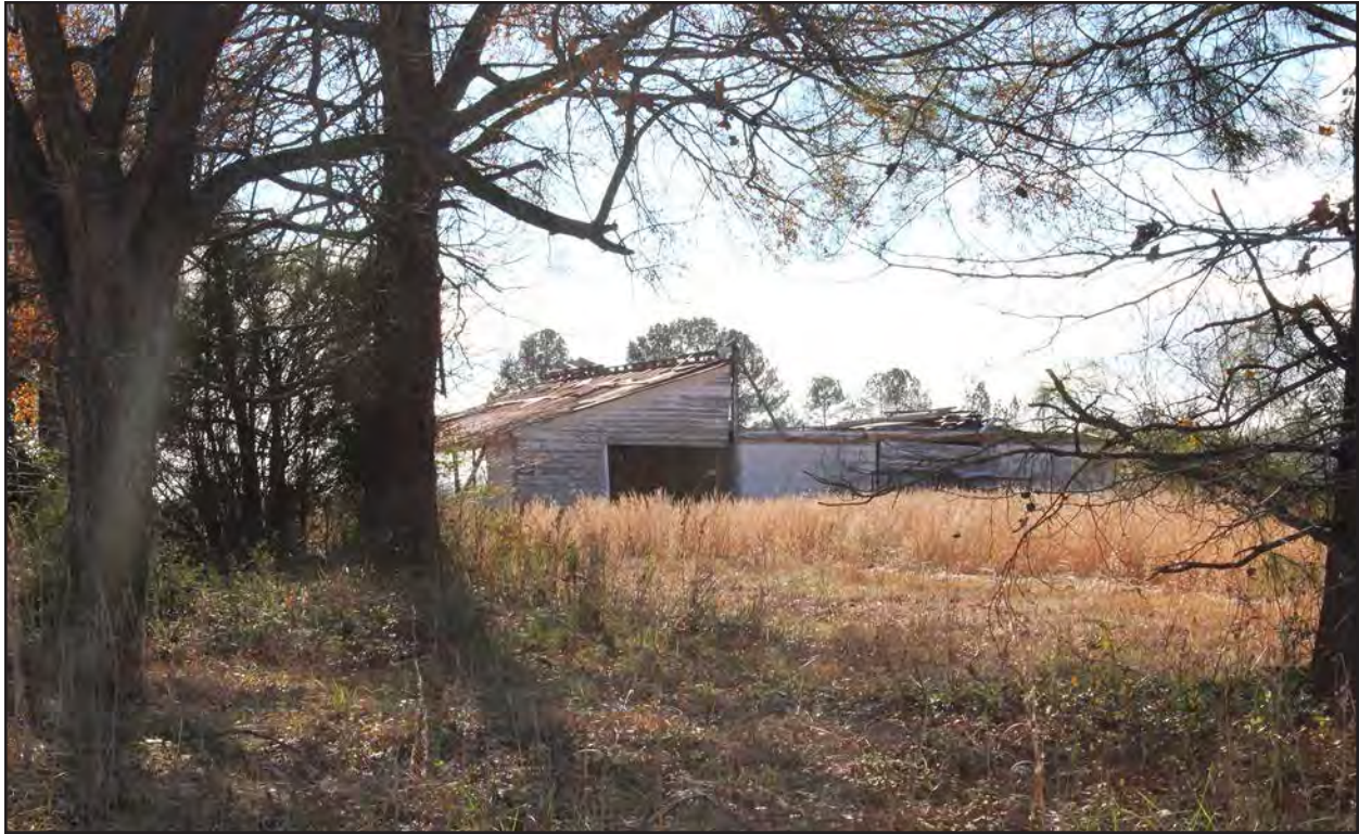
Photo 89. JT1919, accessory structure, facing south-southeast.
