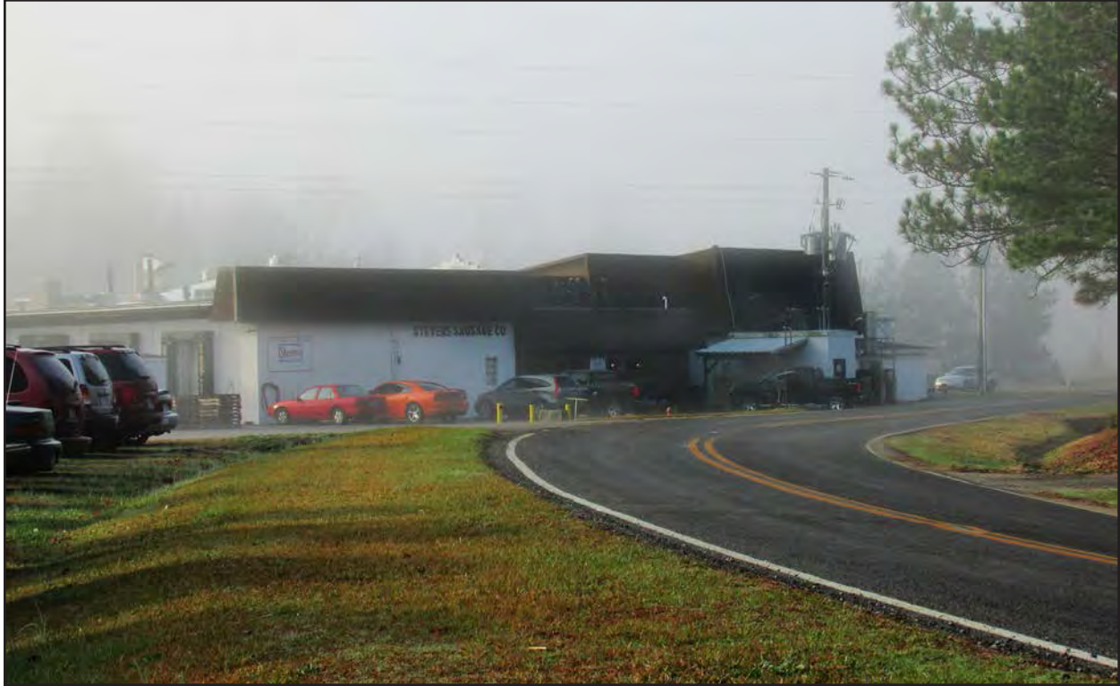
Photo 95. JT1921 (Stevens Sausage Company plant), facing south.
