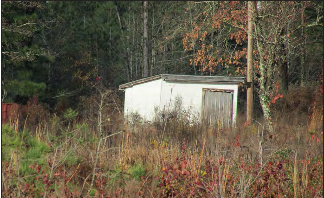
Photo 170. RB0678, well house, facing north.
