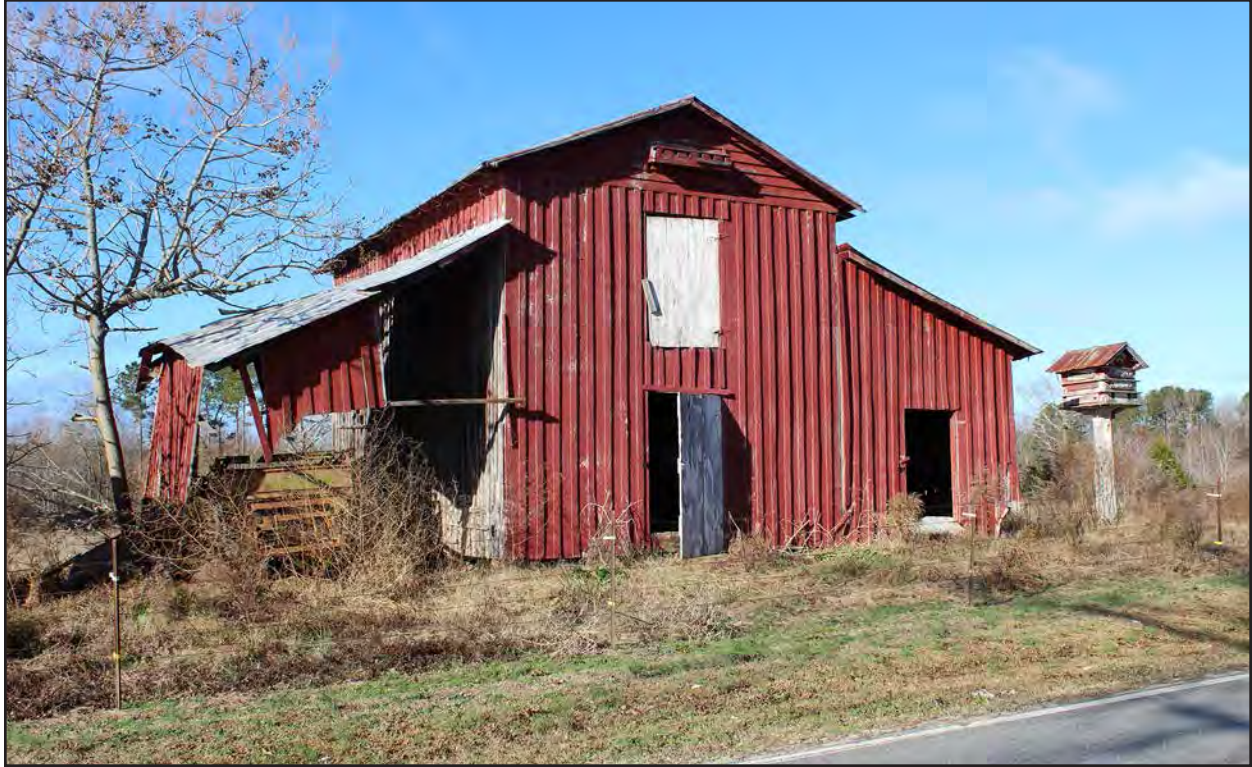
Photo 33. HX0228, birdhouse, and HX0229, pack house, facing northwest.
