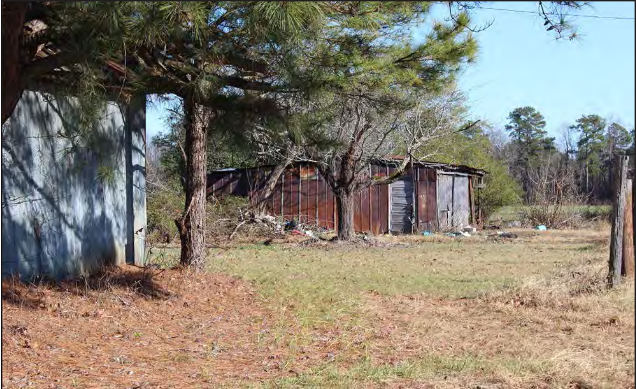
Photo 70. JT0957, gabled accessory structure 3, facing east.
