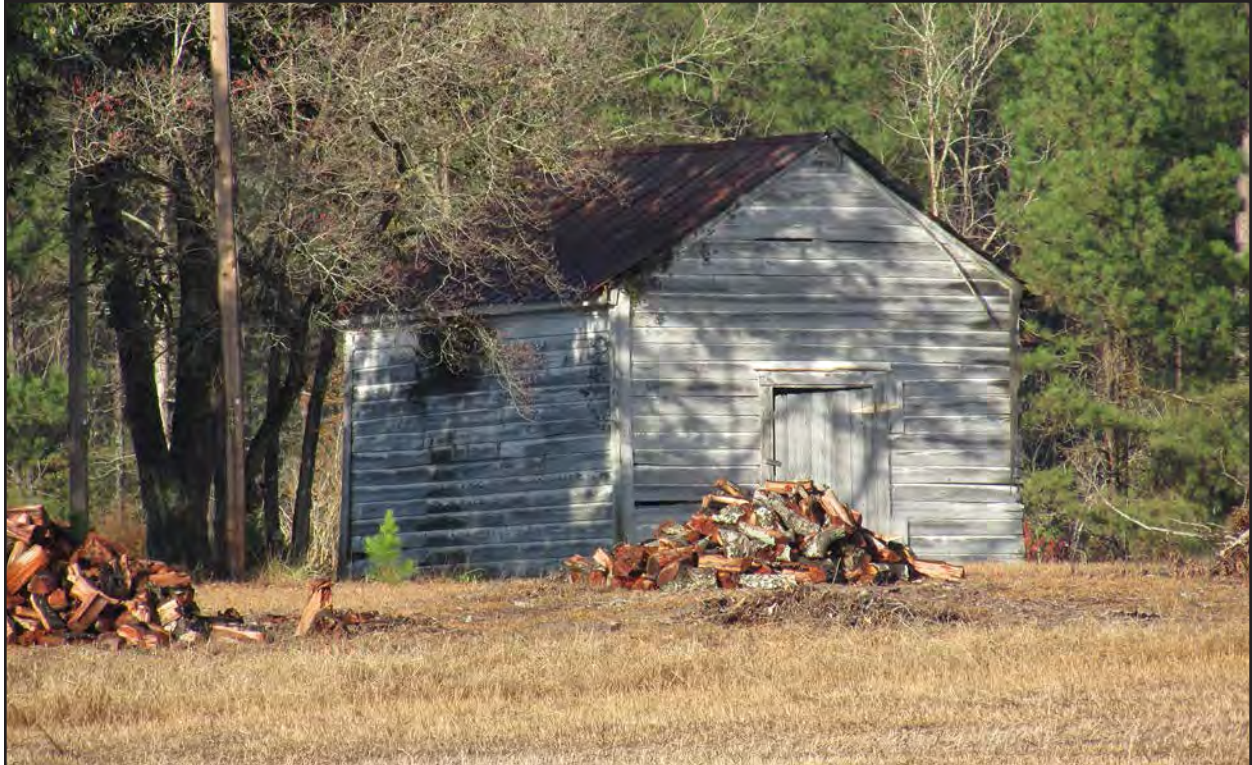
Photo 166. RB0678, shed, facing north.
