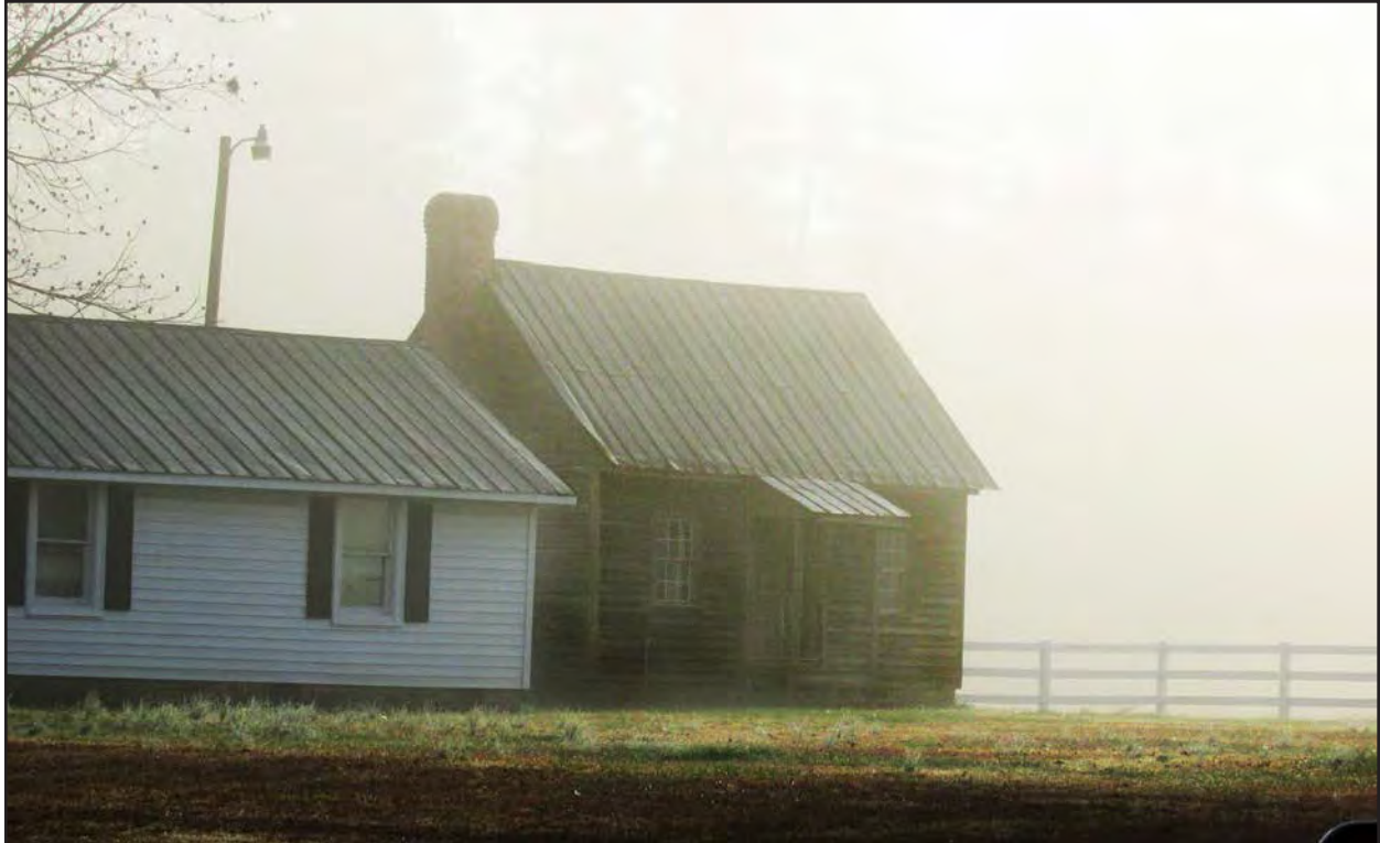
Photo 92. JT1920, log cabin, facing southeast.
