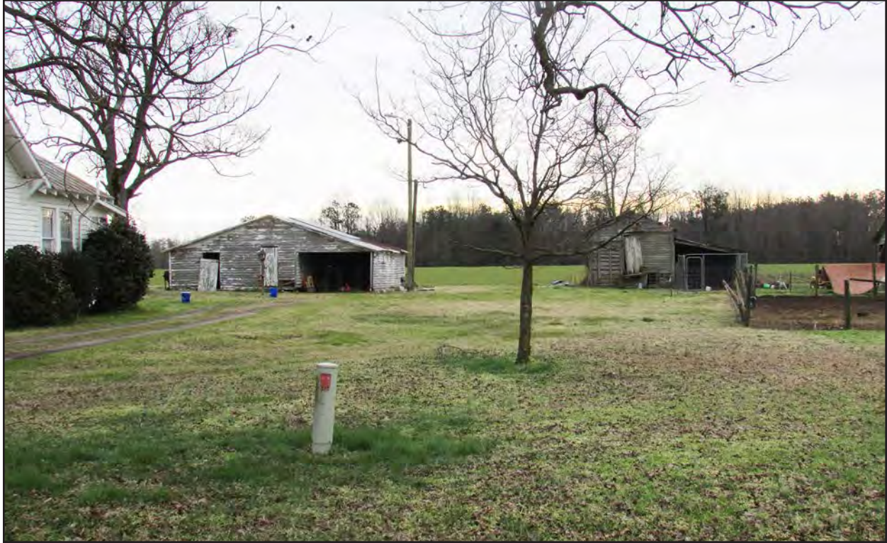
Photo 163. NS1517, outbuildings, facing southeast.
