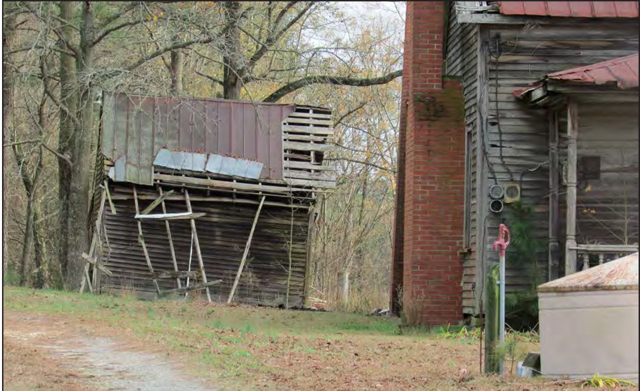
Photo 116. JT1937, accessory structure facing east.
