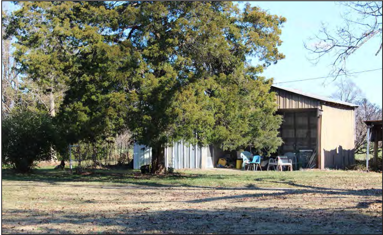
Photo 67. JT0957, storage structure, facing east-northeast.
