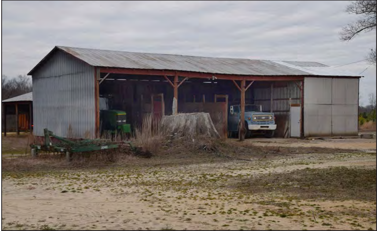
Photo 47. HX1581, garage, facing northeast.
