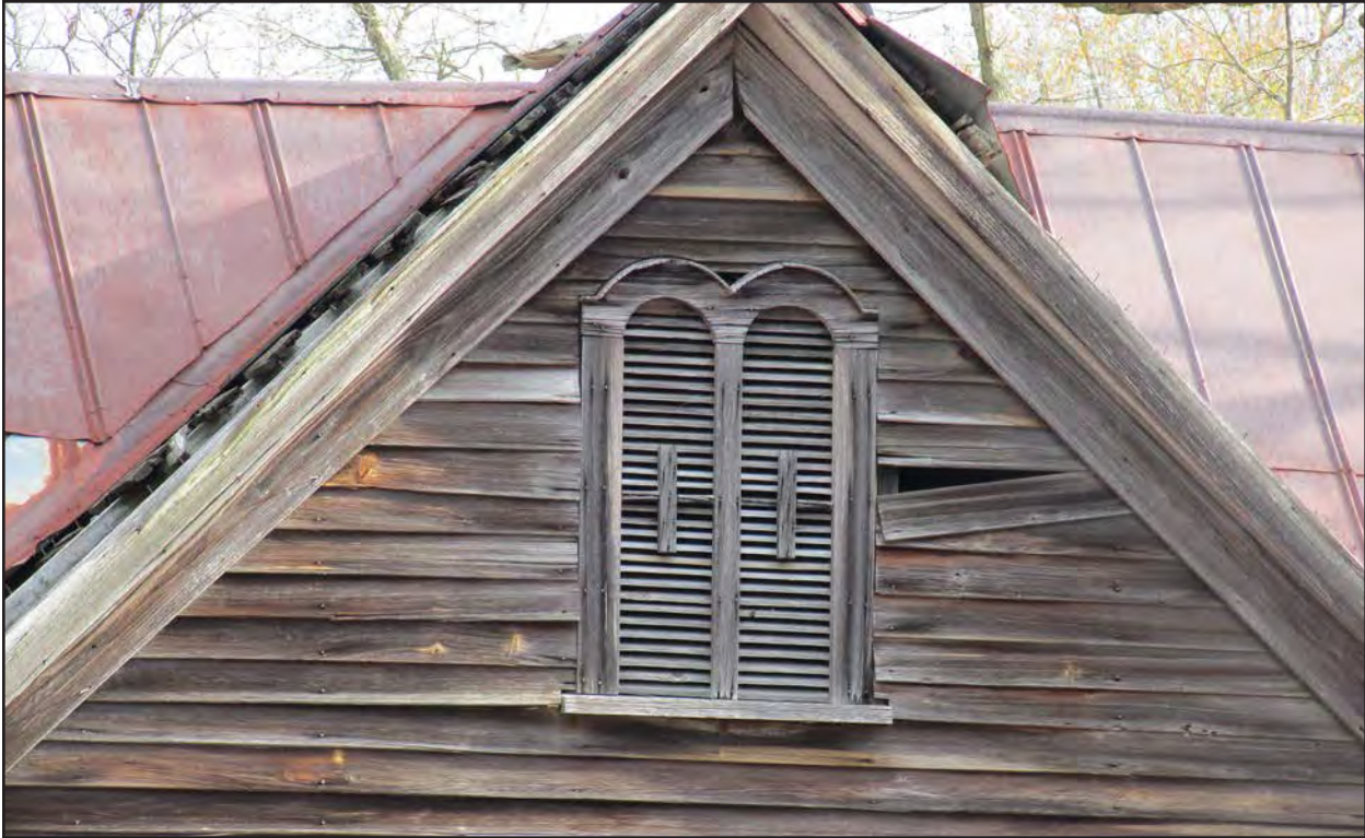
Photo 114. JT1937, vent details, facing east.
