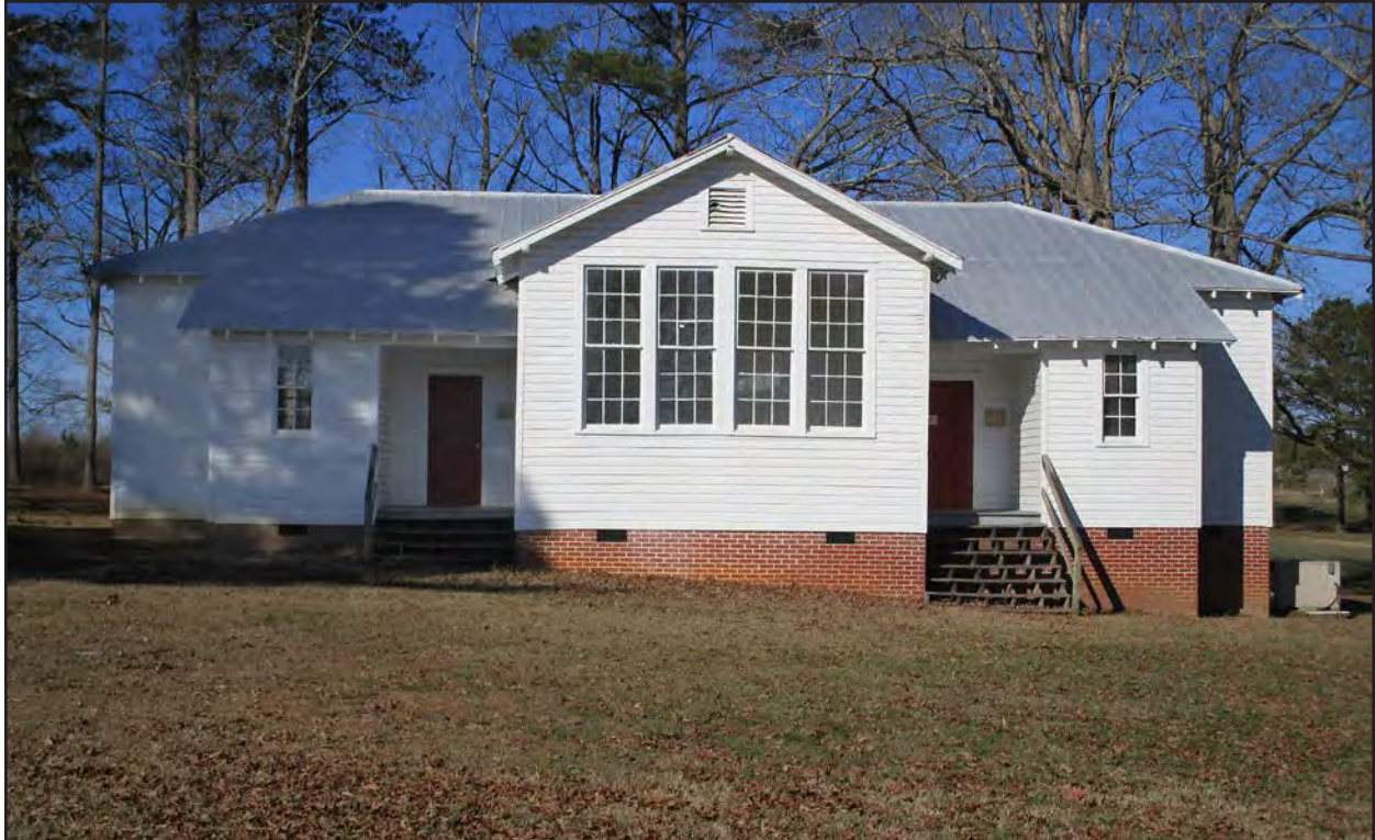
Photo 42. HX1566 (Allen Grove Rosenwald School), facing northwest.
