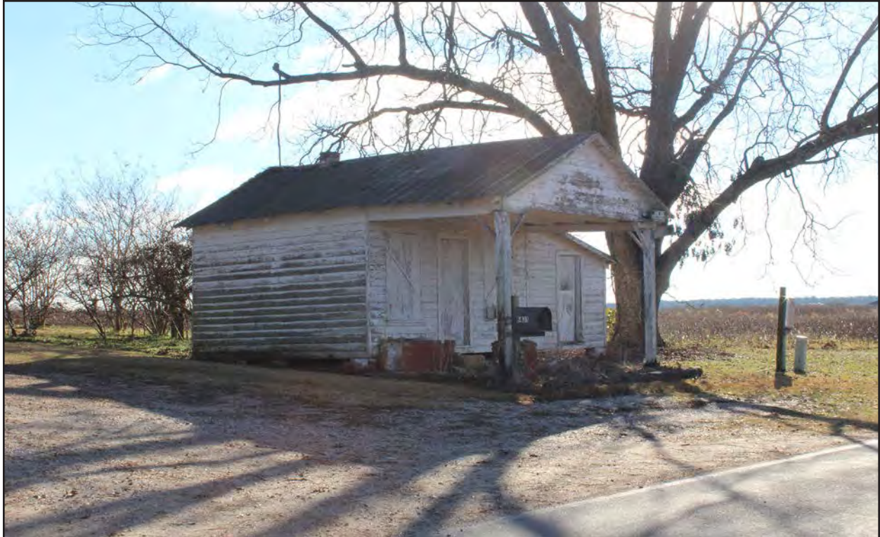
Photo 32. HX0227, rear accessory structure, facing southeast.
