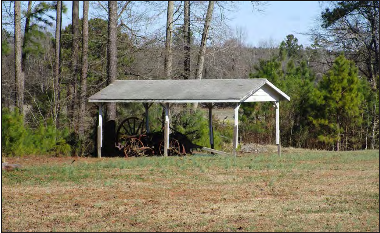
Photo 11. HX0021, shed, facing north-northeast.
