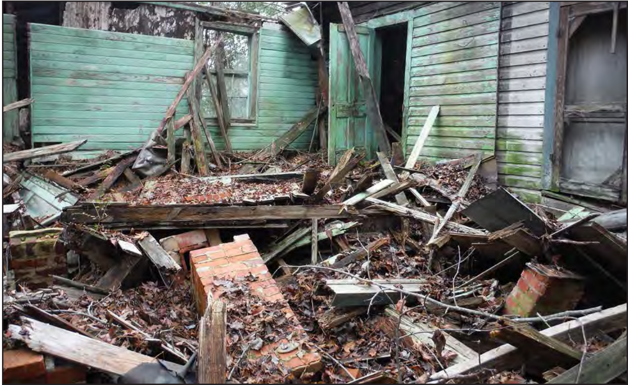
Photo 57. HX1597, dwelling, collapsed addition, facing south.
