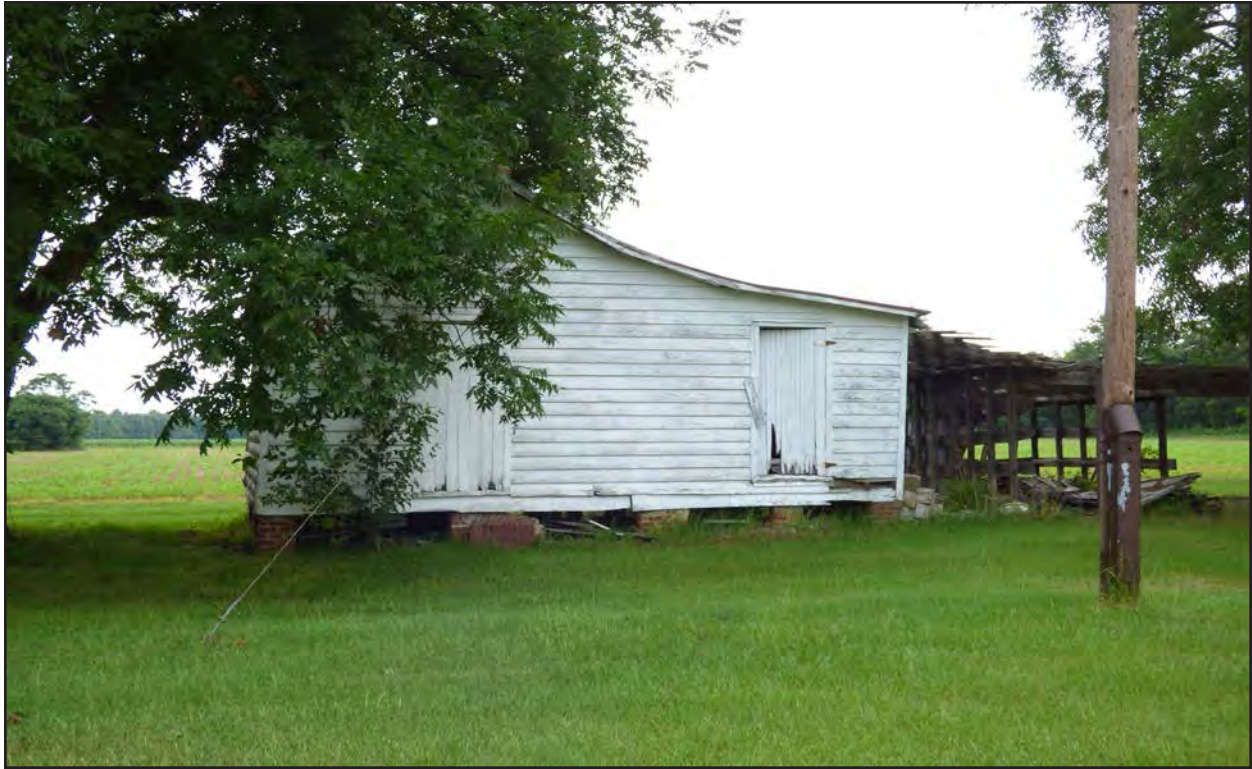
Photo 143. NS1493, agricultural outbuildings, facing north.
