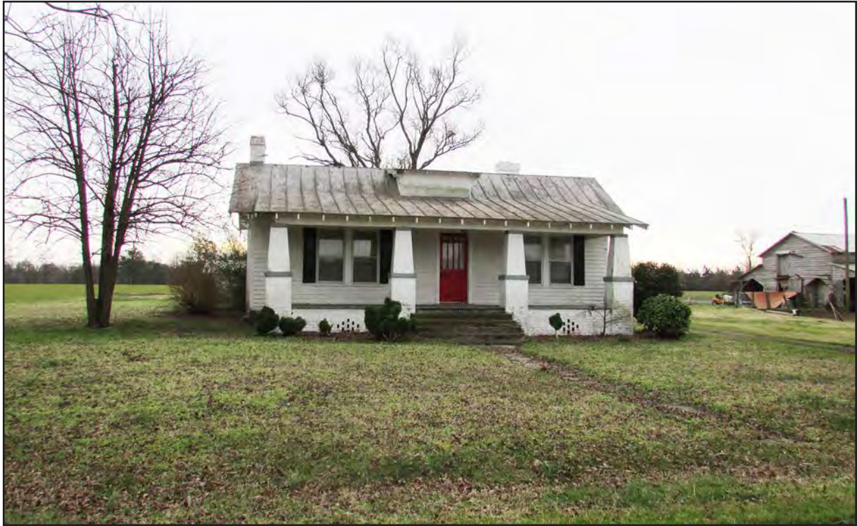
Photo 161. NS1517, dwelling, facing south-southeast.
