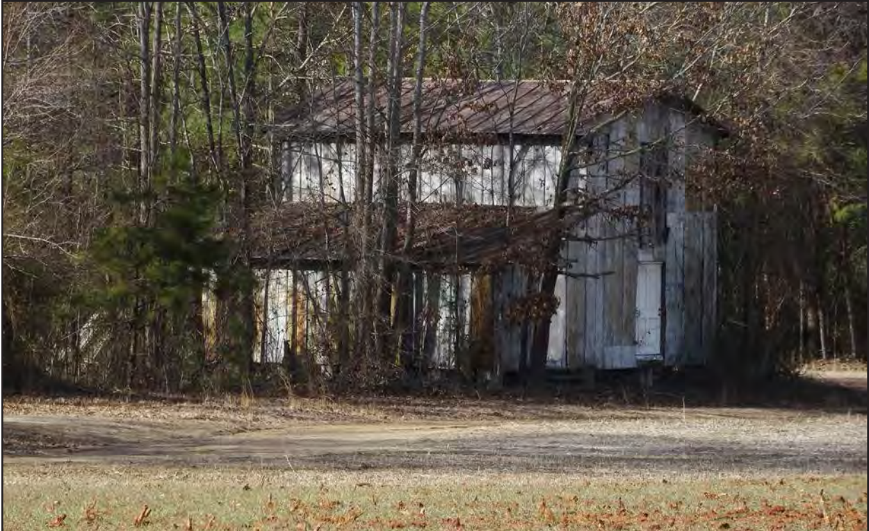
Photo 178. WL2002, barn, facing north-northwest.
