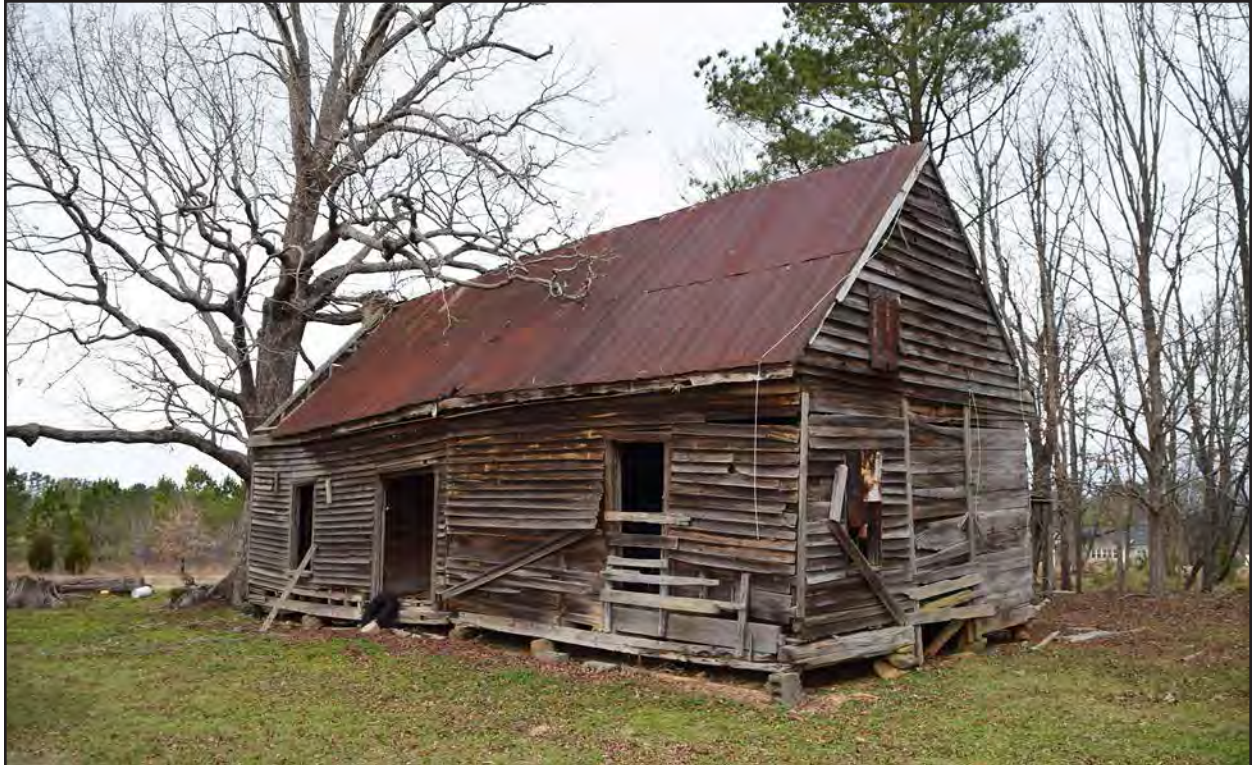
Photo 130. NS0650, cabin, facing northwest.
