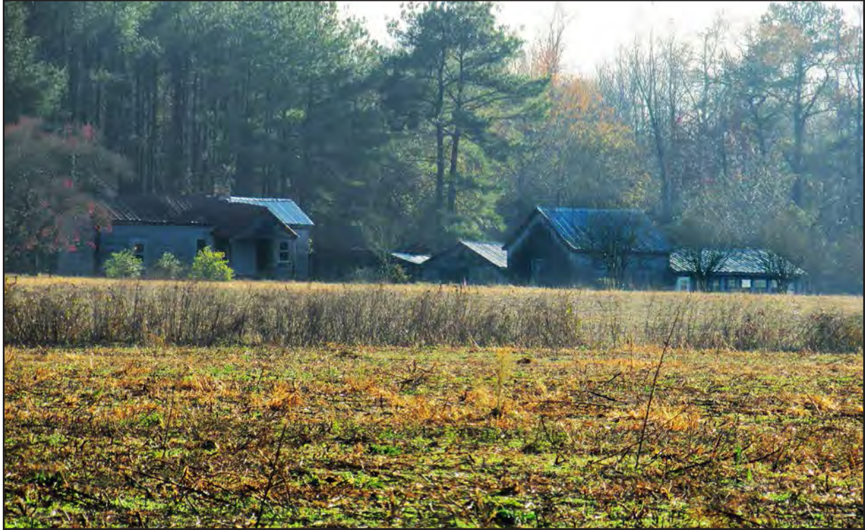
Photo 173. RB0680, agricultural outbuildings, facing south.
