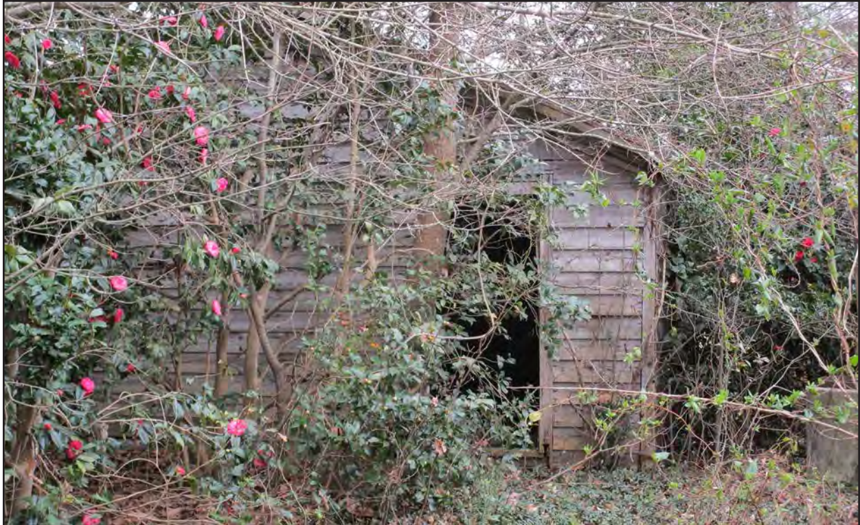
Photo 110. JT1935 accessory structure 2, facing south.
