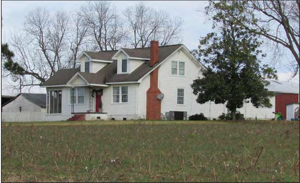
Photo 53. HX1583, facing northeast.
