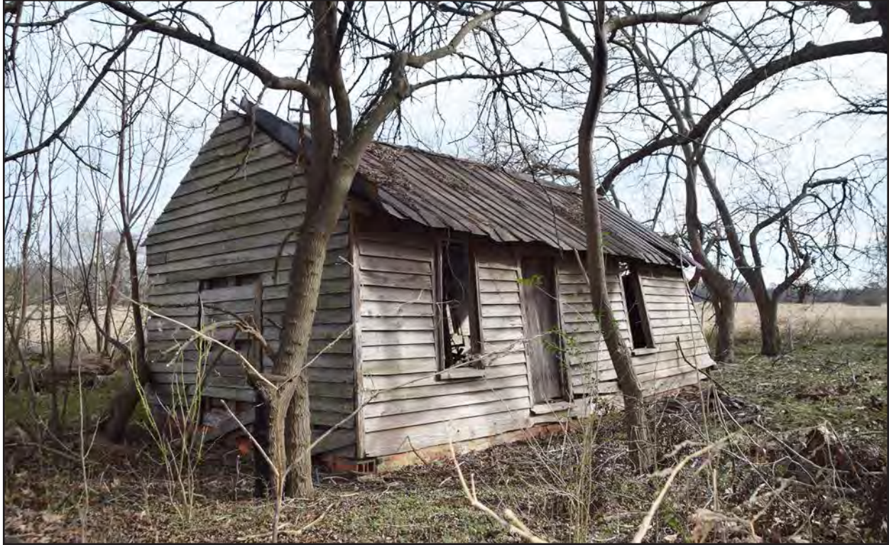
Photo 135. NS0650 summer kitchen, facing northeast.
