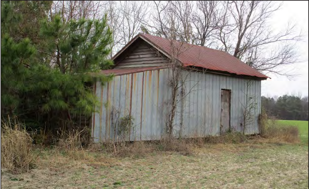
Photo 106. JT1935 accessory structure 1, facing southeast.
