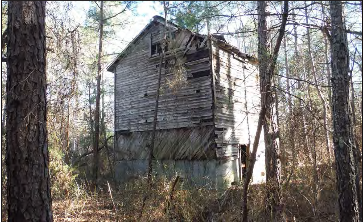
Photo 60. HX1597, tobacco barn 2, facing northeast.
