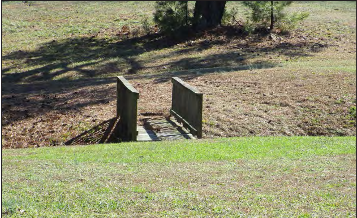
Photo 25. HX0021, wooden bridge, facing south-southeast.
