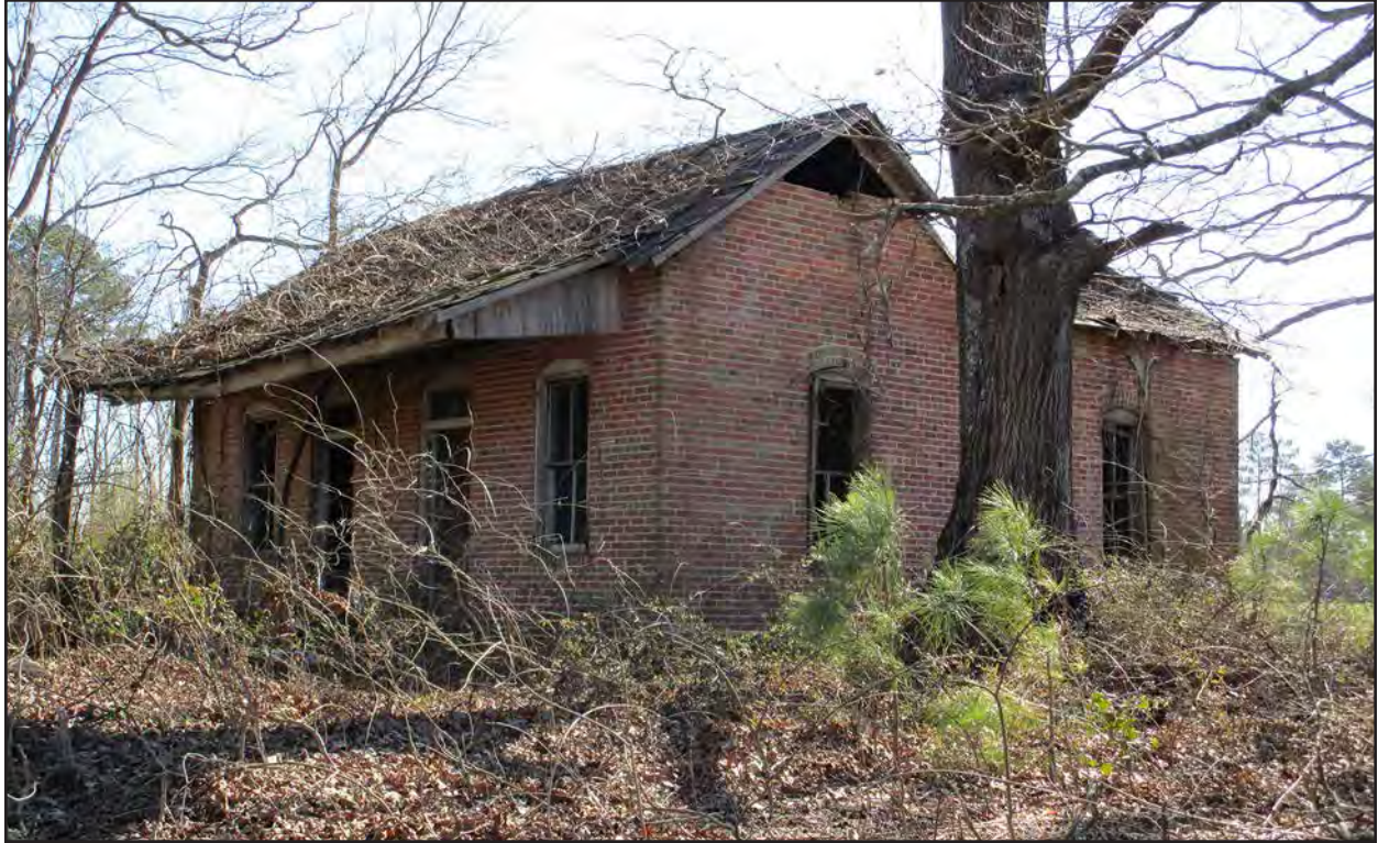
Photo 39. HX0354, facing south.
