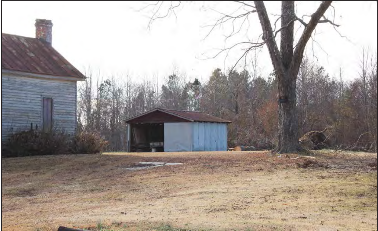
Photo 182. WL2012, outbuilding, facing southwest.
