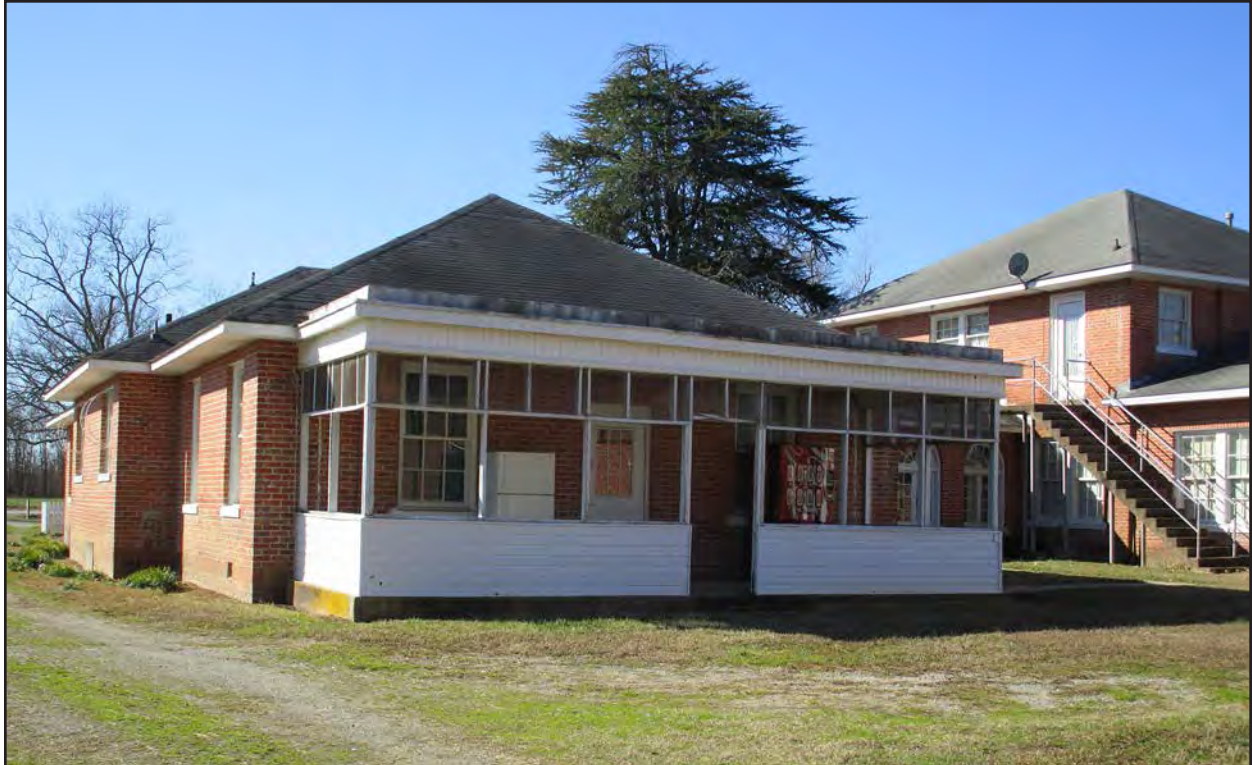
Photo 8. HX0021, facing southwest.
