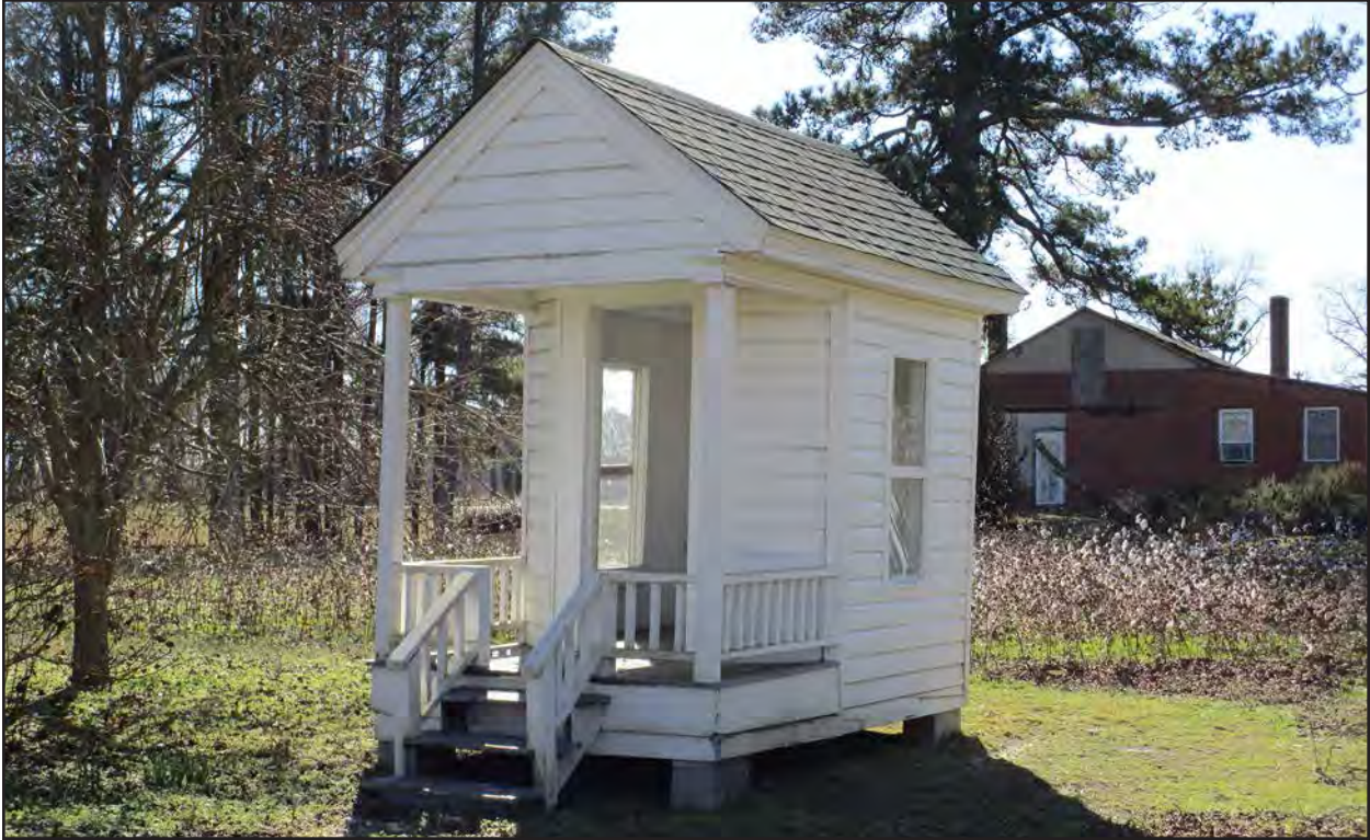
Photo 15. HX0021, accessory building, facing south-southwest.
