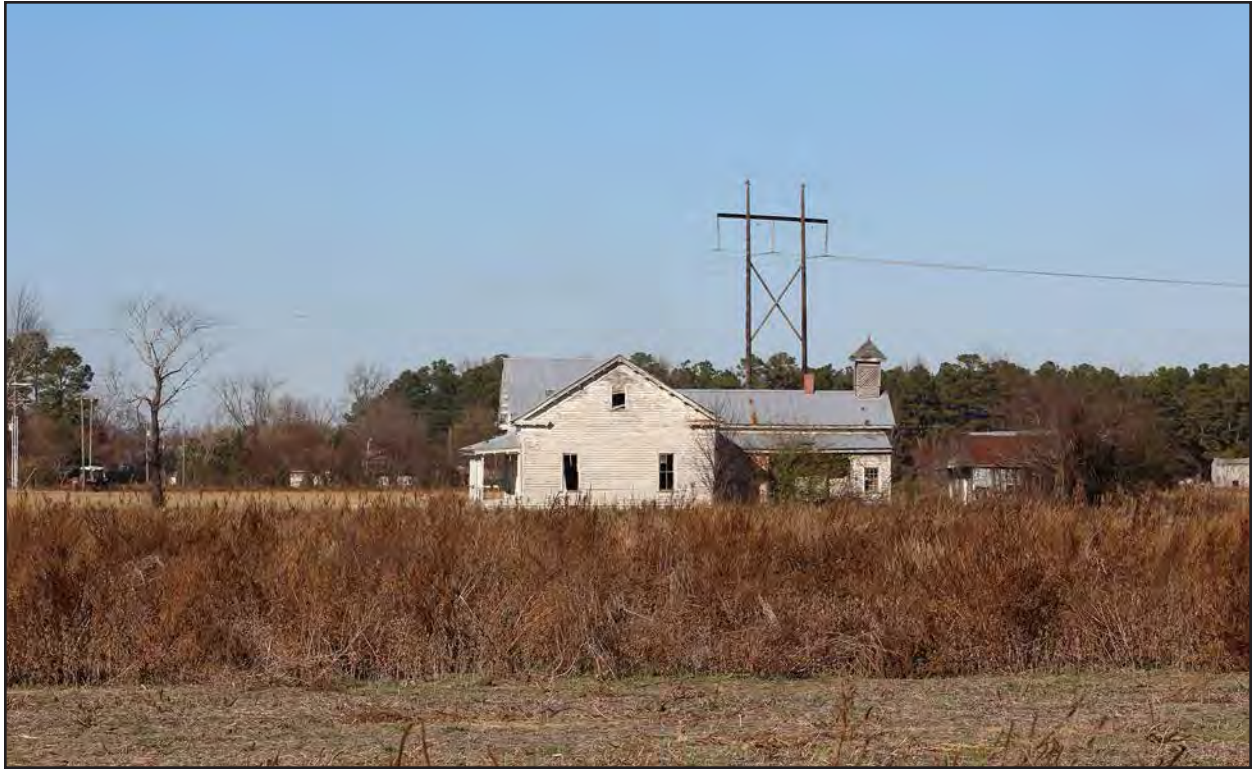
Photo 121. JT1969, facing north.
