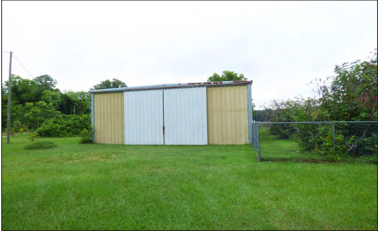
Photo 147. NS1493, metal workshop building, facing south.
