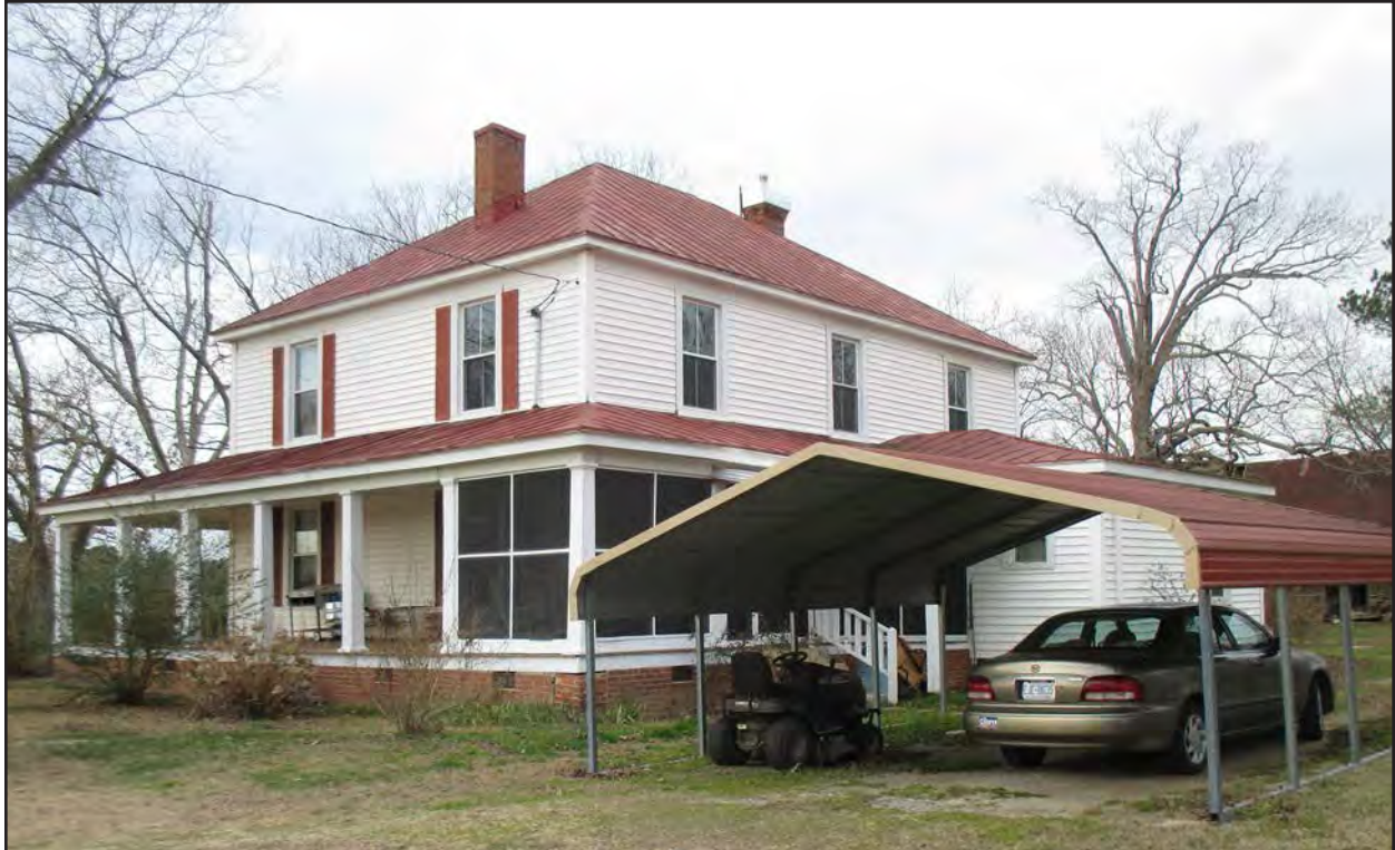
Photo 136. NS0650, carport, facing northwest.
