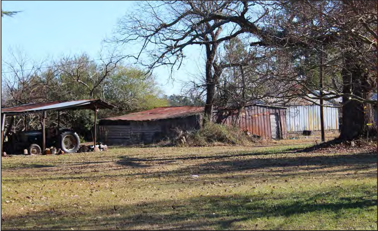
Photo 69. JT0957, gabled accessory structure 3, facing southeast.
