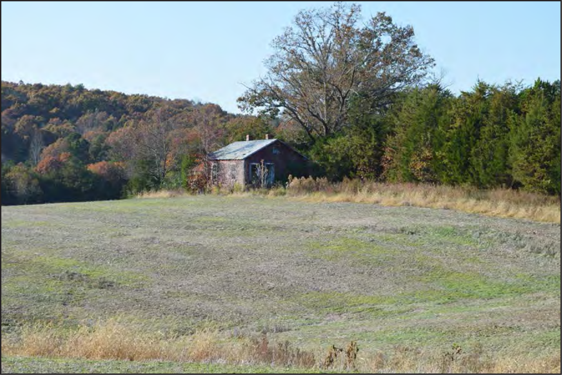
Figure 232. 014-5086, house with surroundings, facing northwest.
