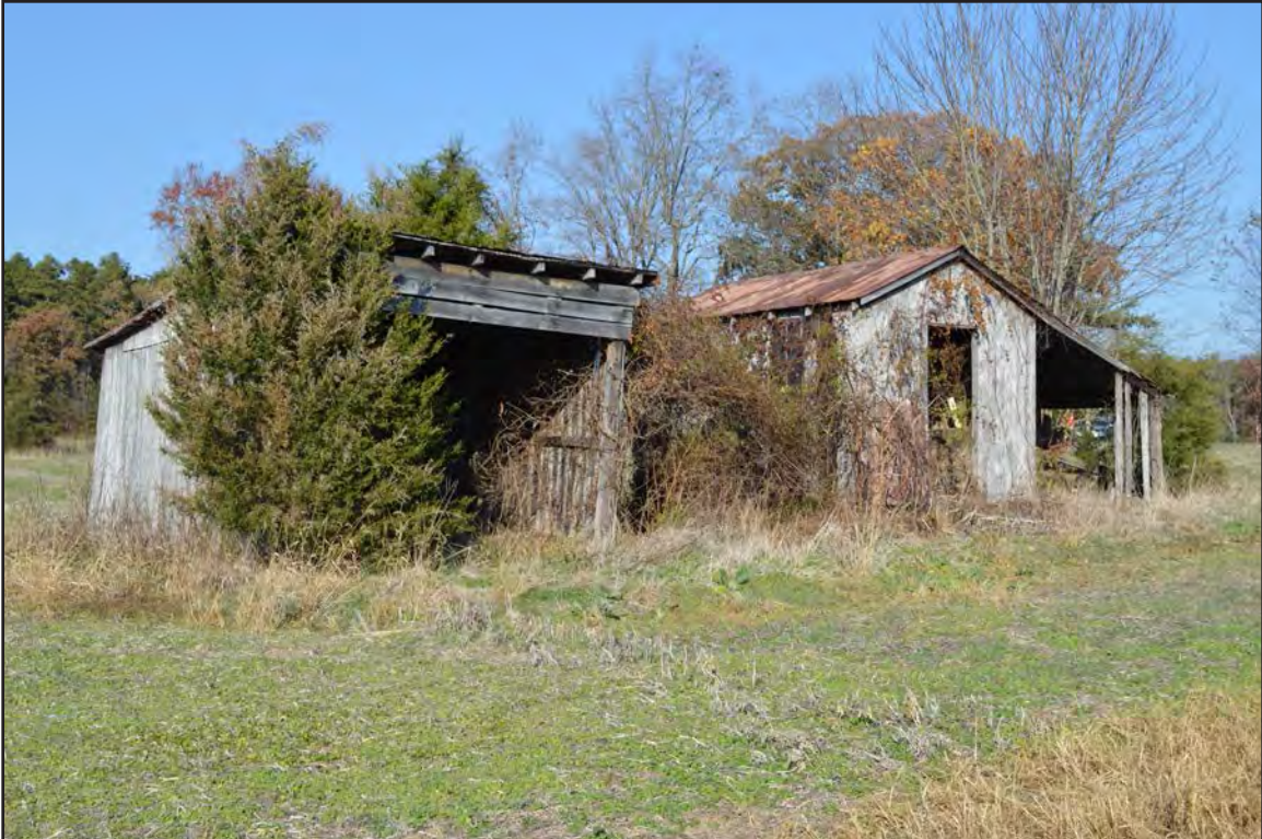
Figure 230. 014-5085, ca. 1920s sheds, facing northeast.
