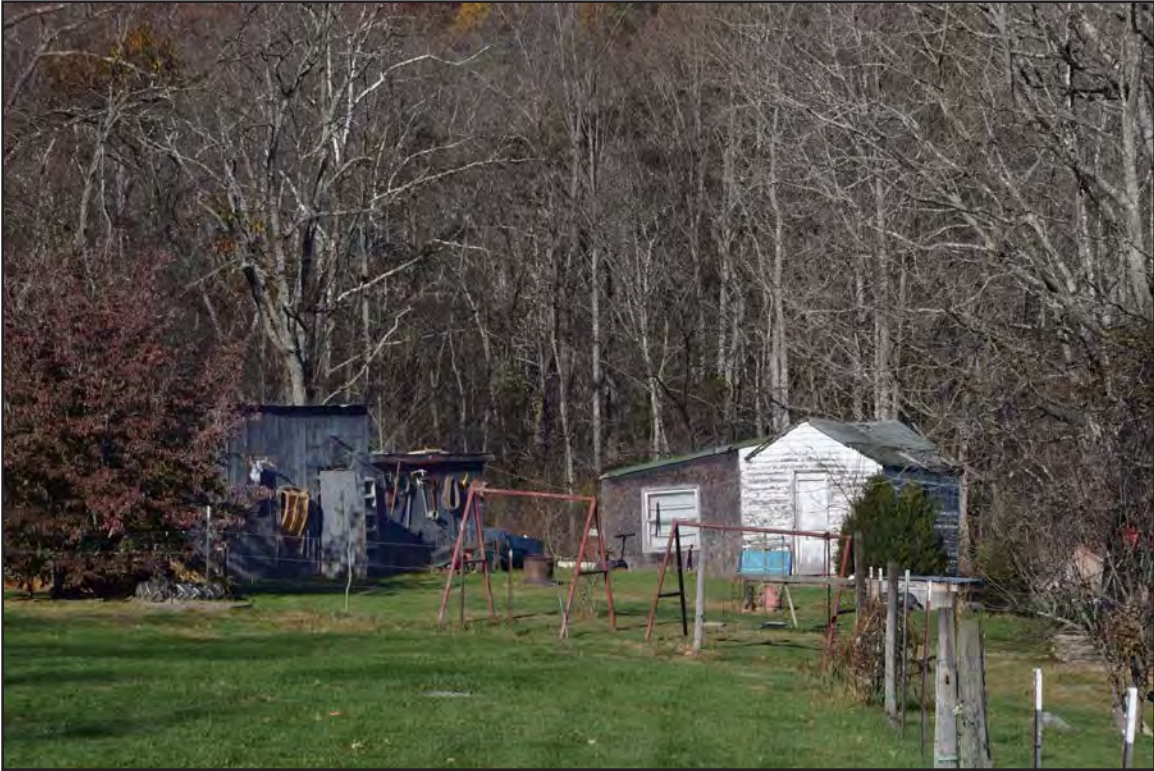
Figure 83. 007-5712 Shed 2 and Shed 3, facing west.
