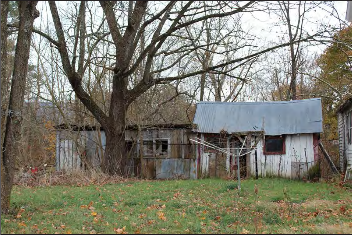
Figure 158. 007-5731, shed, facing south.
