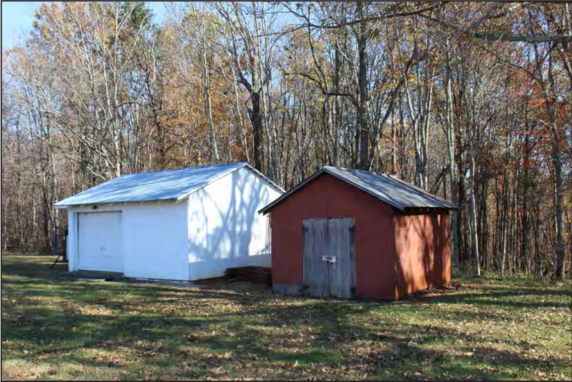
Figure 253. 062-5229, Shed 1 and Shed 2, facing northeast.
