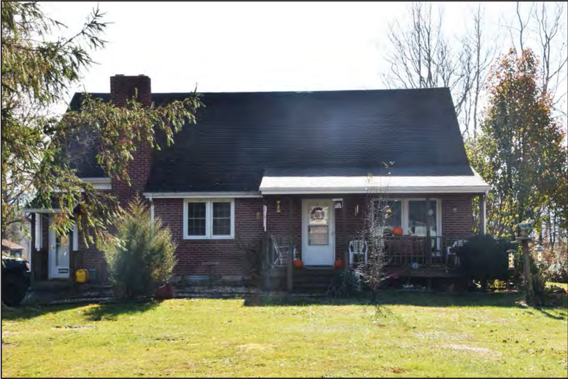
Figure 139. 007-5726, house, facing southwest.
