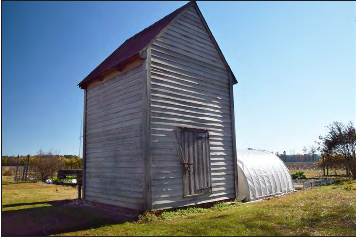
Figure 269. 133-0101, smokehouse, facing south.
