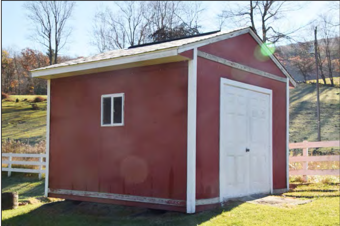
Figure 64. 007-5709, Outbuilding 3, facing southwest.
