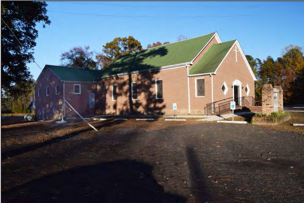
Figure 238. 026-5257, church, facing northeast.
