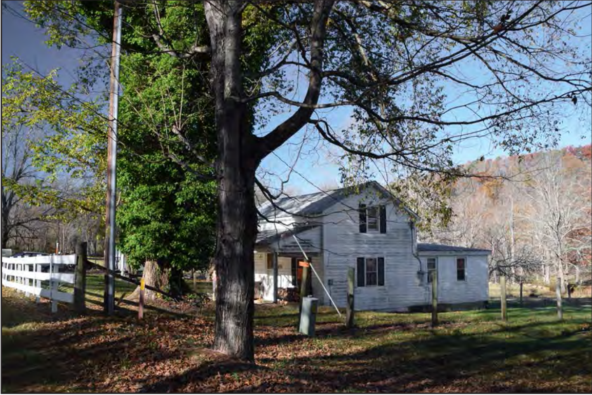
Figure 95. 007-5715, garage, facing west.
