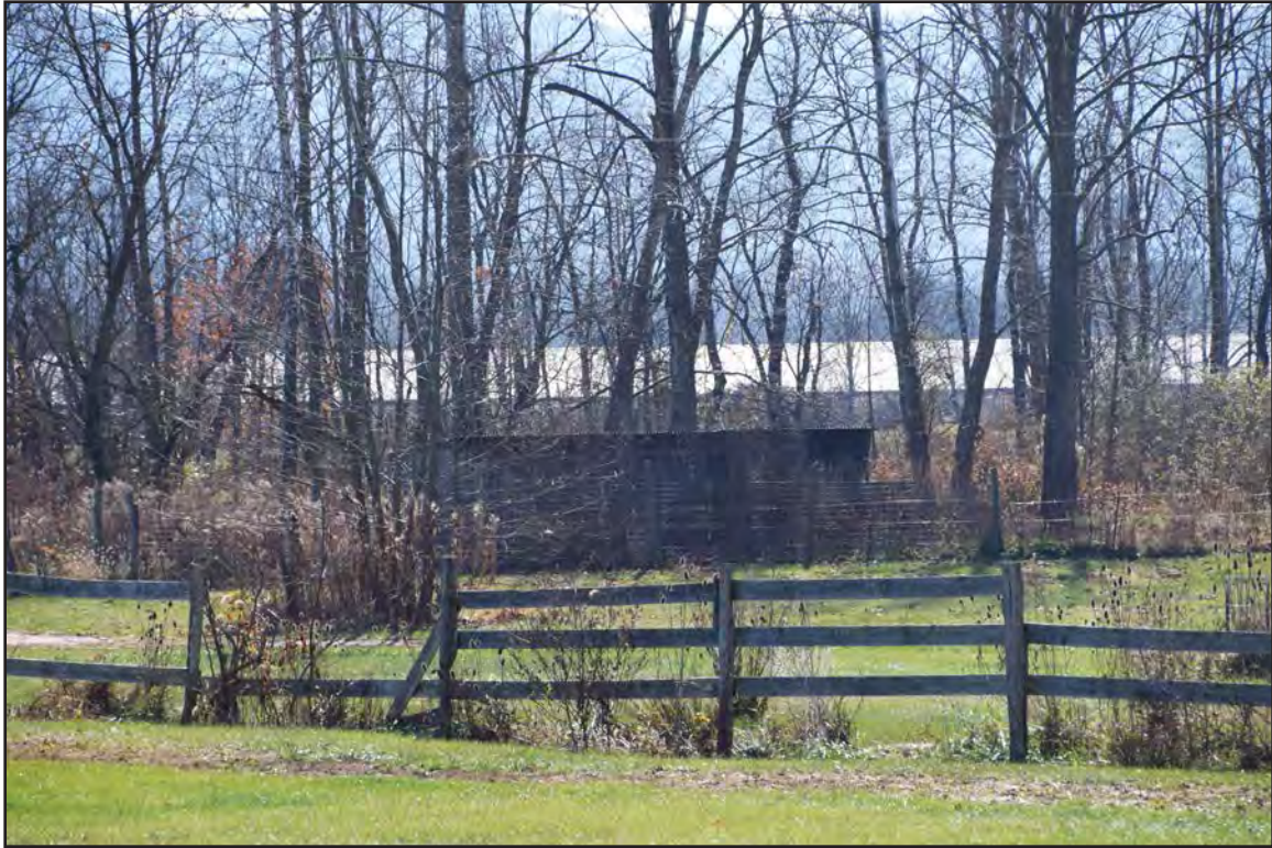
Figure 13. 007-0467, chicken house, facing southwest.
