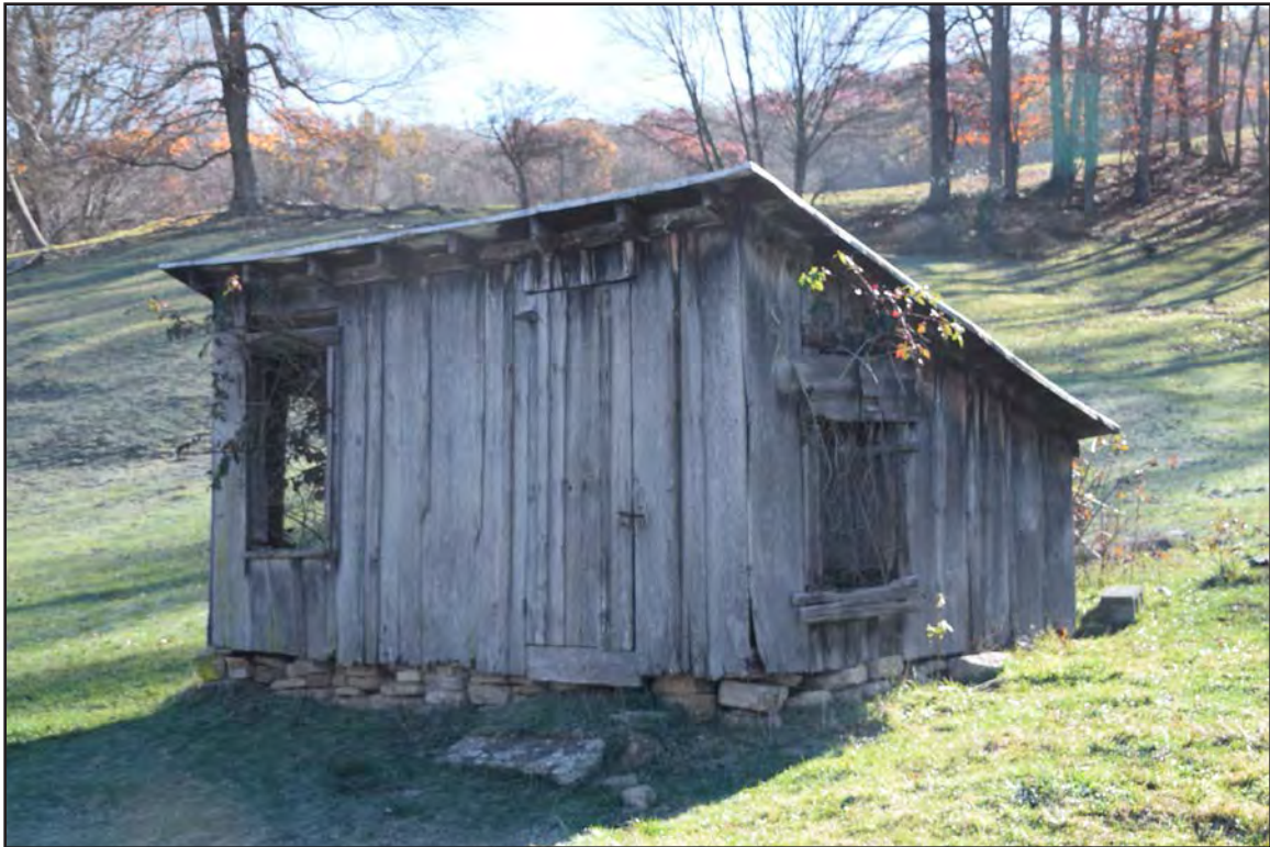
Figure 63. 007-5709, Outbuilding 2, facing southeast.
