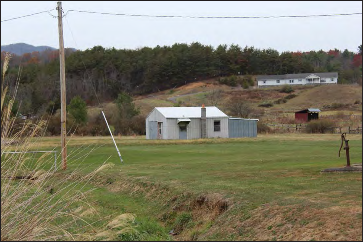
Figure 177. 007-5736, outbuilding, facing northeast.
