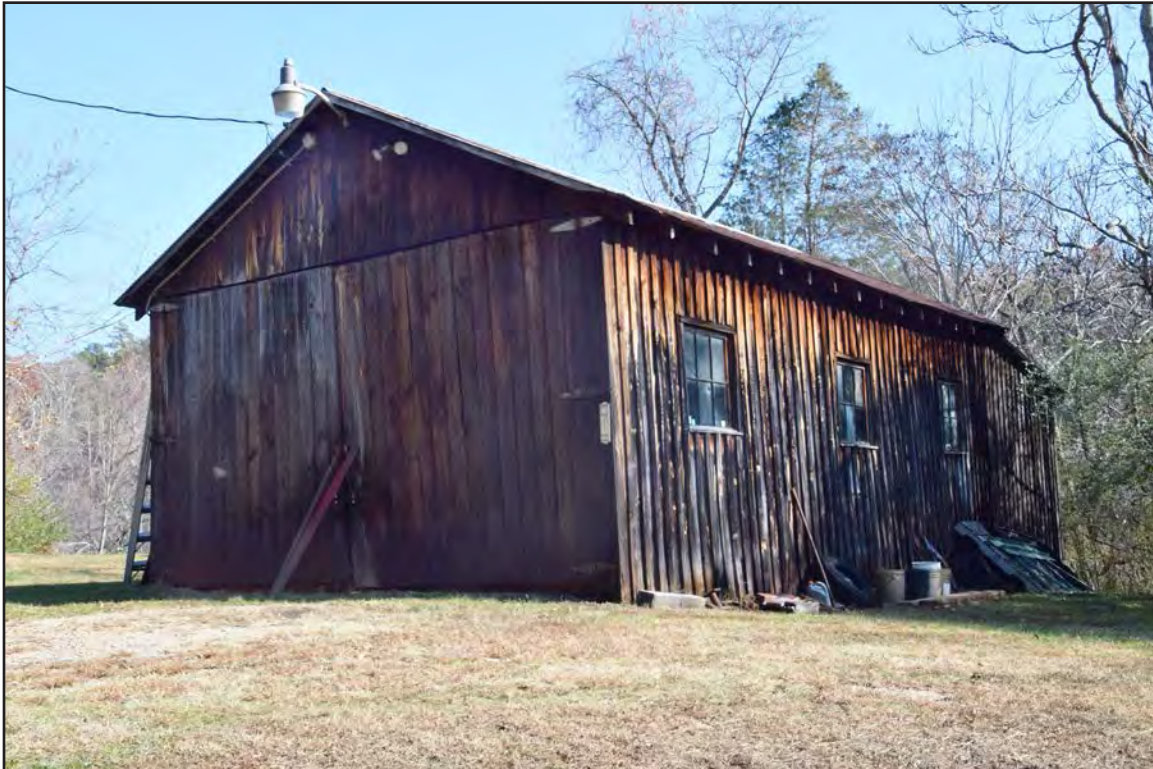
Figure 248. 062-5223, garage, facing southeast.
