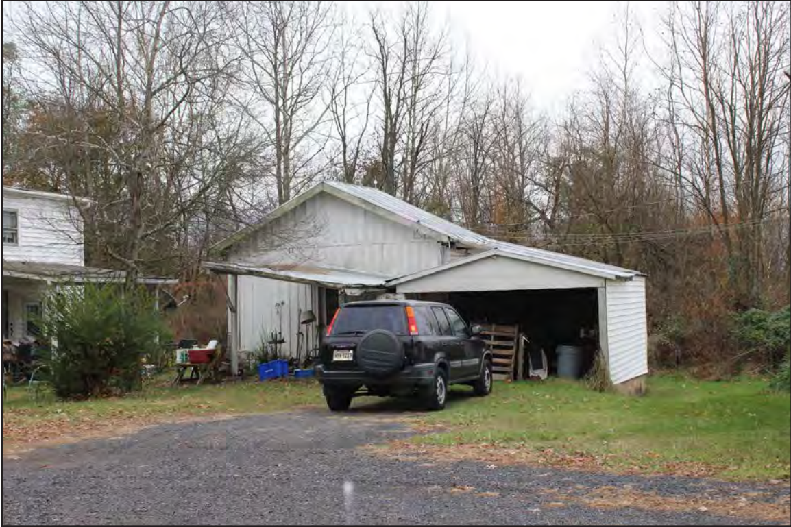
Figure 21. 007-0476, garage and shed, facing southeast.
