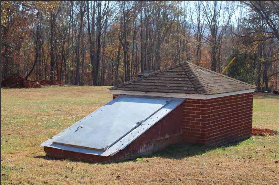
Figure 254. 062-5229, well house, facing southeast.
