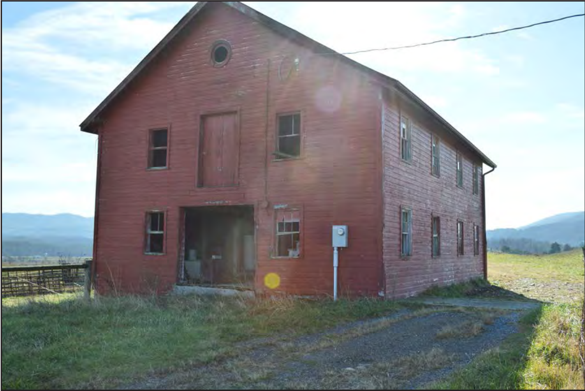
Figure 7. 007-0463, Barn 1, facing south.
