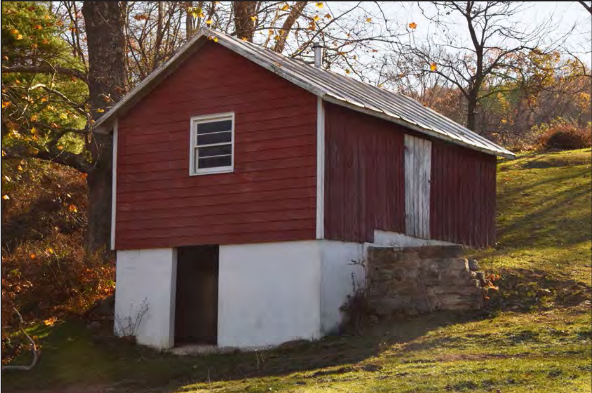
Figure 62. 007-5709, Outbuilding 1, facing southeast.
