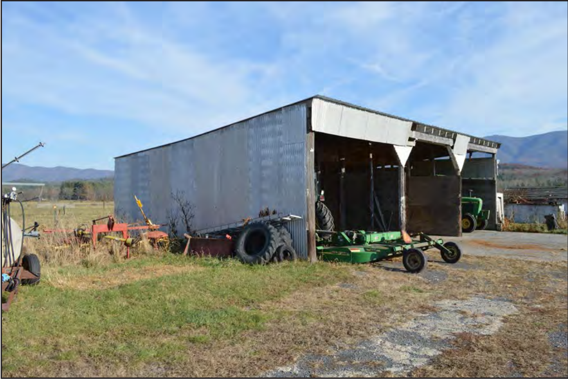
Figure 90. 007-5714, shed, facing east.
