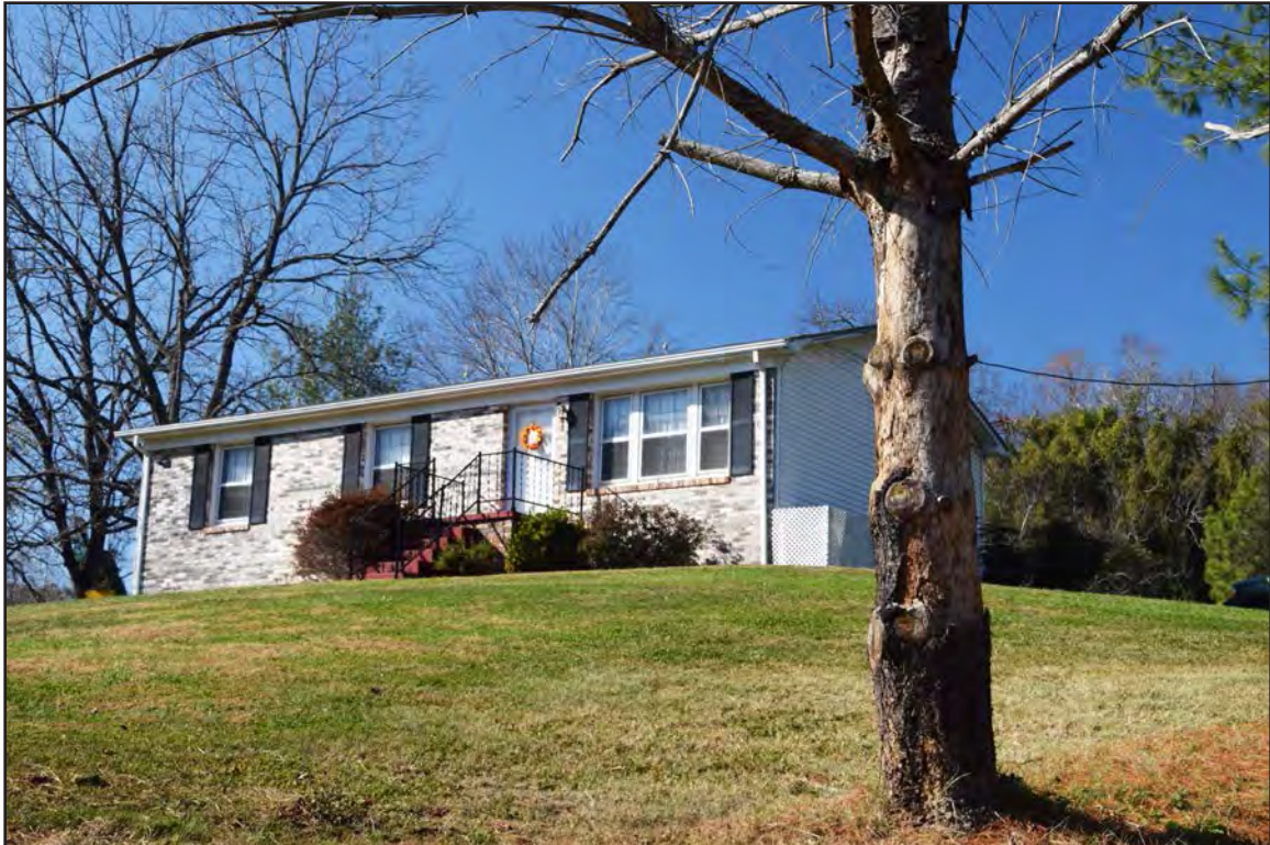
Figure 246. 062-5223, house, facing west.
