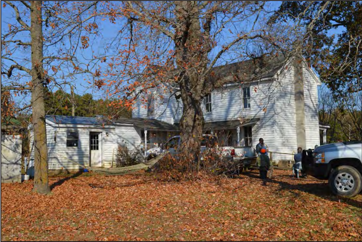
Figure 225. 014-5085, house, facing northeast.
