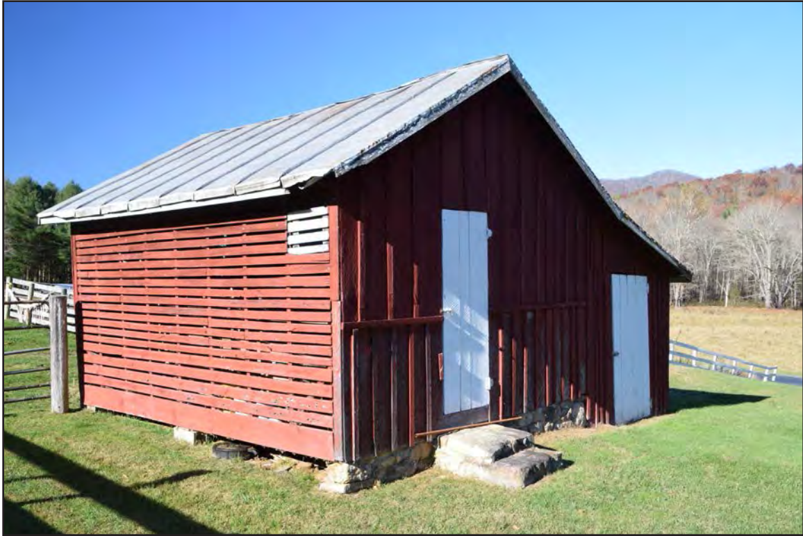
Figure 65. 007-5709, Outbuilding 4, facing southwest.
