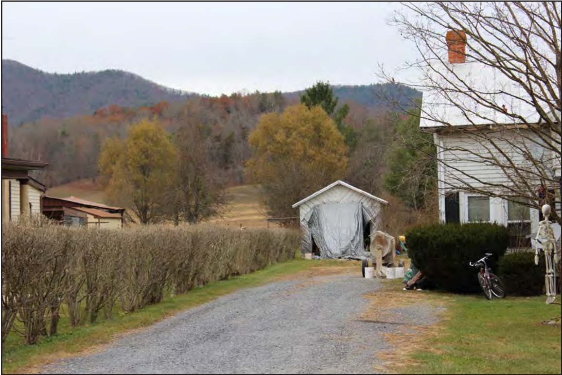
Figure 163. 007-5733, garage, facing north.
