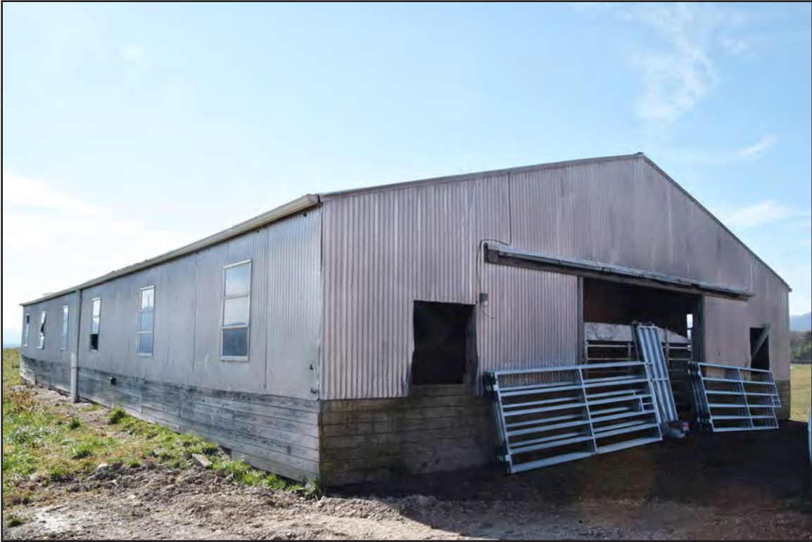
Figure 9. 007-0463, Barn 3, facing southeast.
