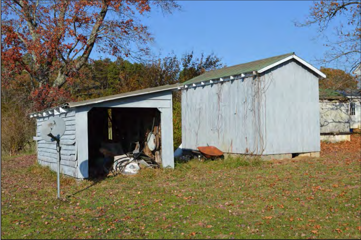
Figure 227. 014-5085, ca. 1930 outbuildings, facing northeast.
