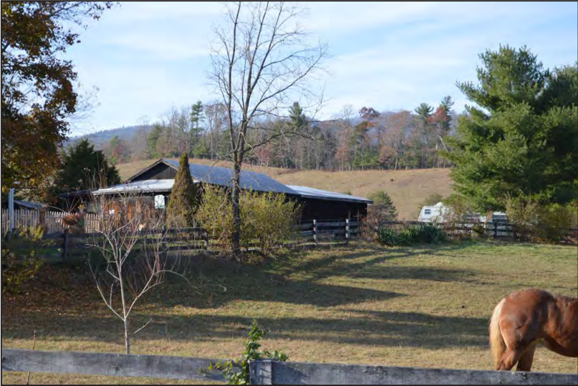
Figure 51. 007-5706, outbuilding, facing west.
