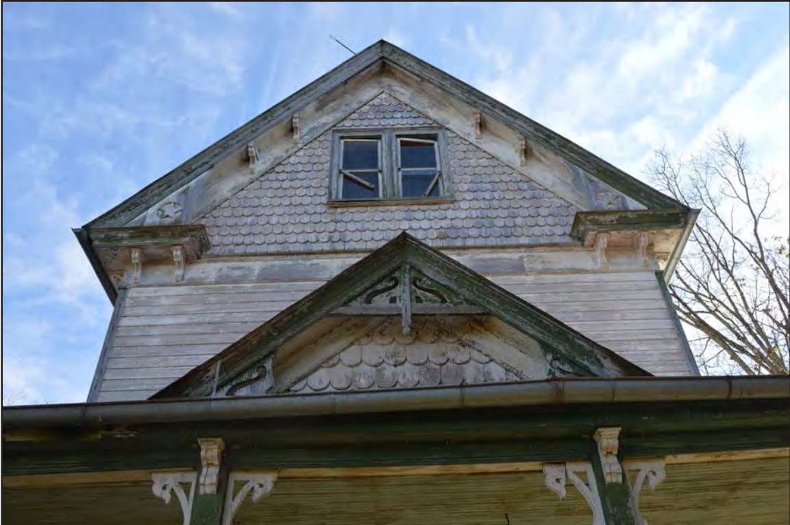
Figure 26. 007-0487, gable details on house, facing southeast.
