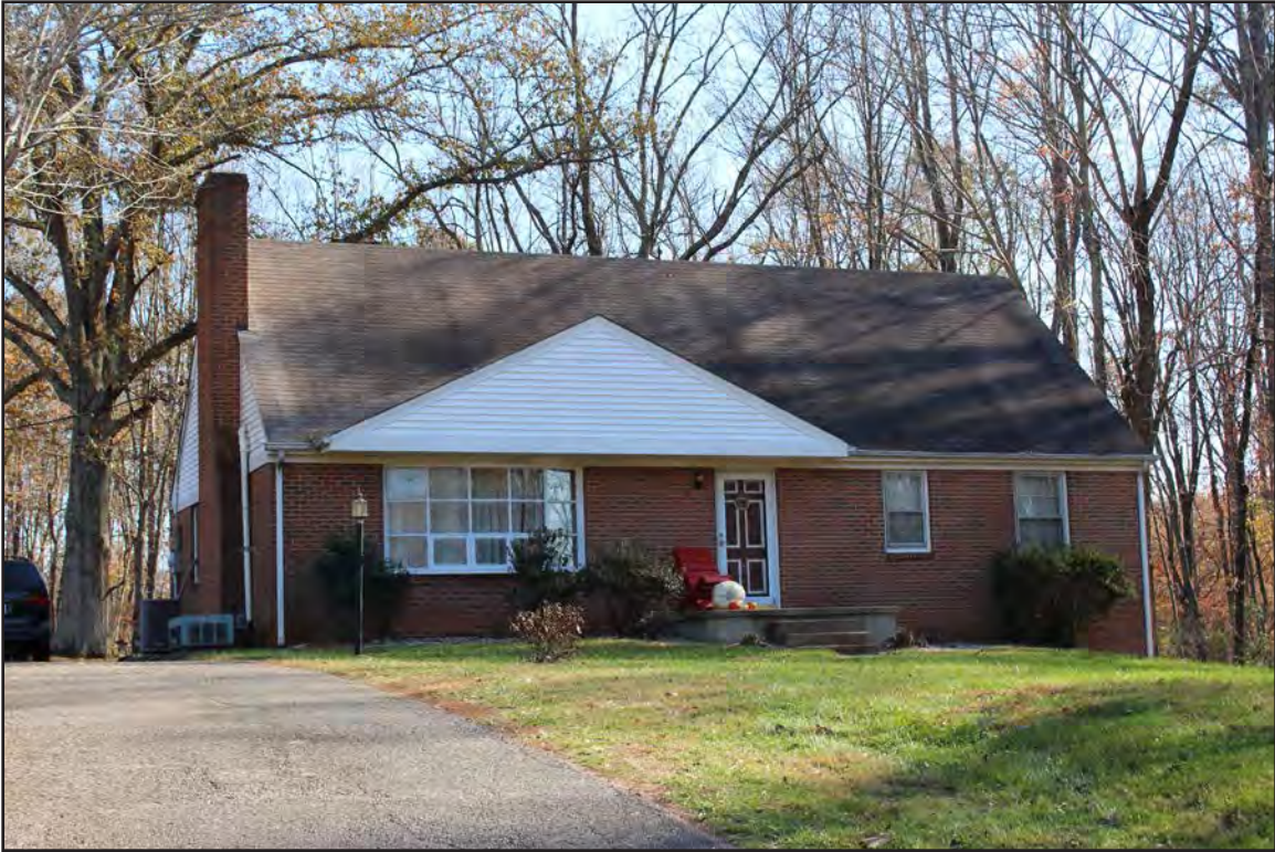
Figure 255. 062-5229, parsonage, facing east-southeast.
