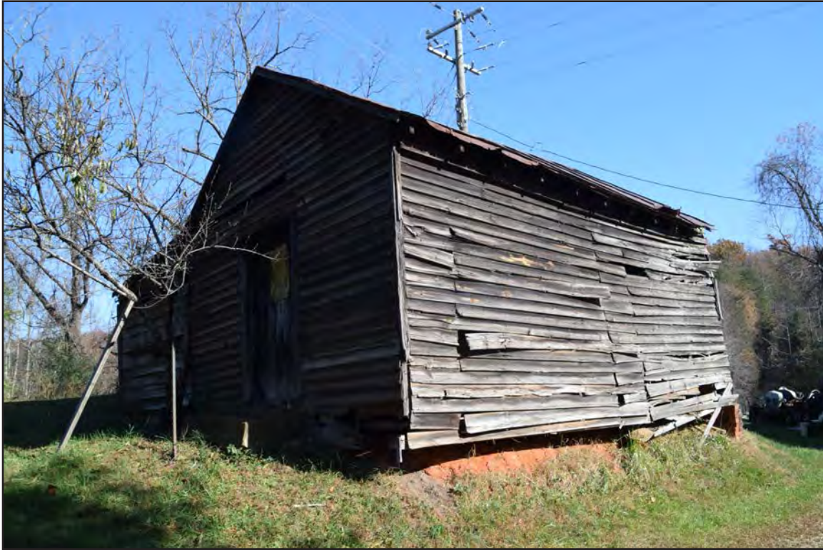
Figure 247. 062-5223, outbuilding, facing southeast.
