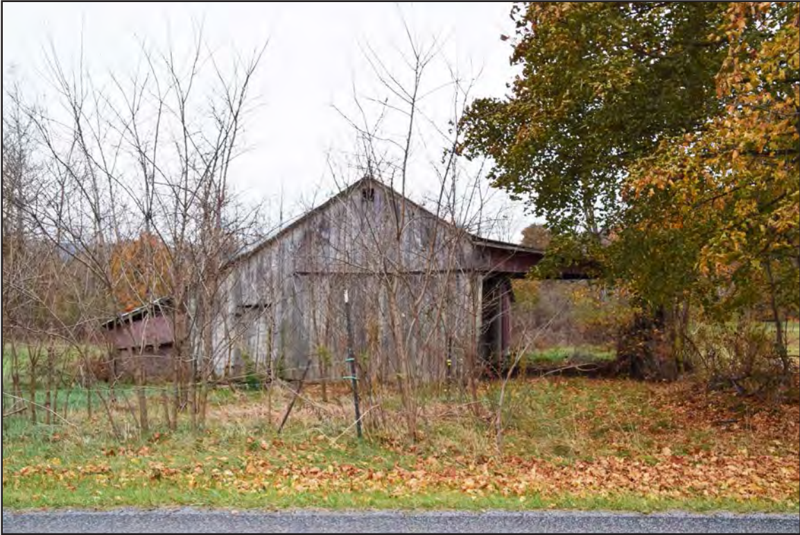
Figure 123. 007-5722, Barn 1, facing south.
