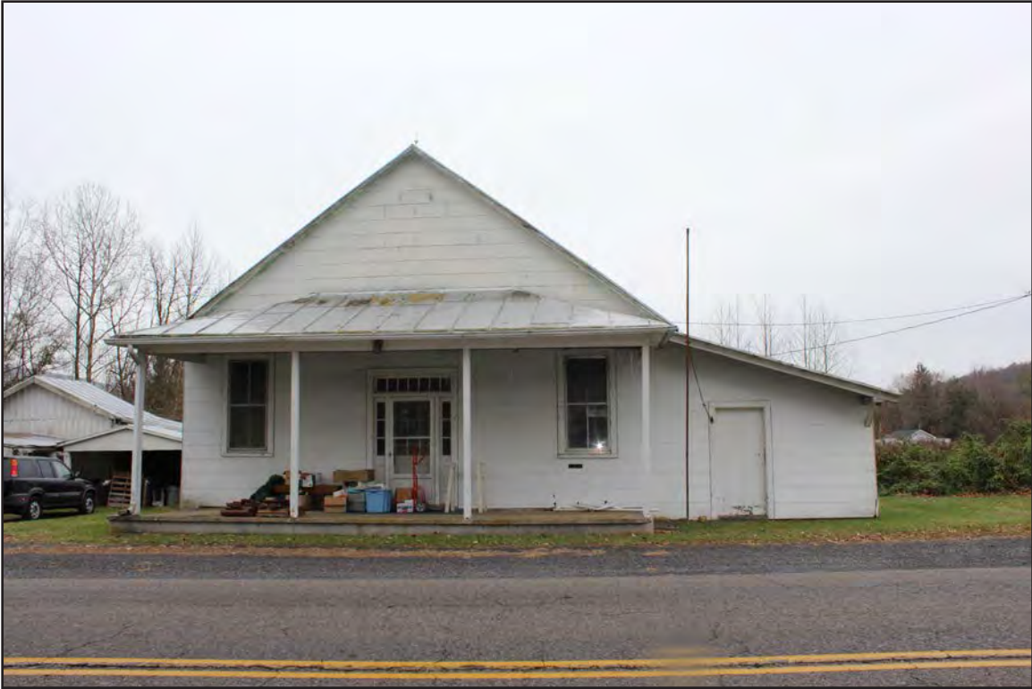
Figure 15. 007-0476, store, facing south.
