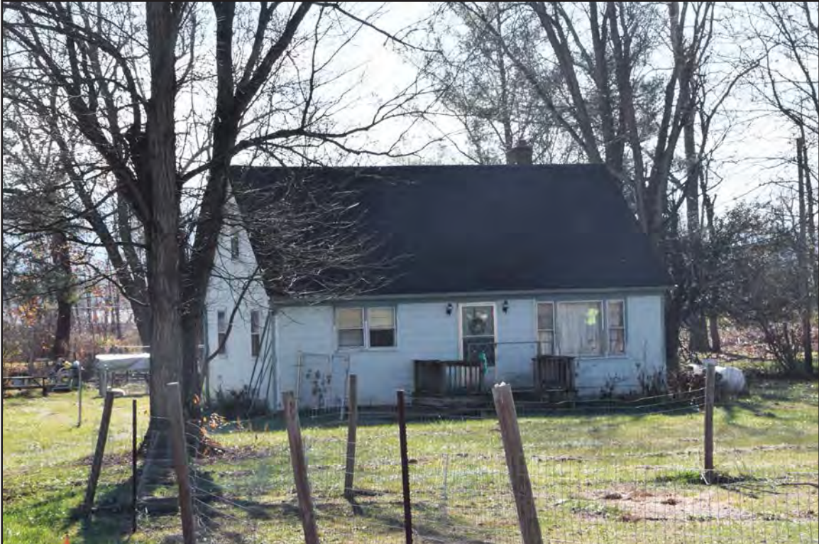
Figure 142. 007-5727, house, facing southwest.
