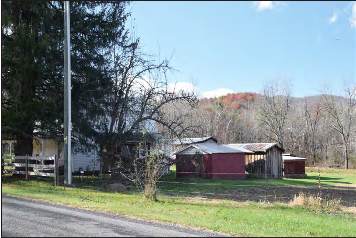
Figure 77. 007-5711, Outbuildings 4-6, facing west.
