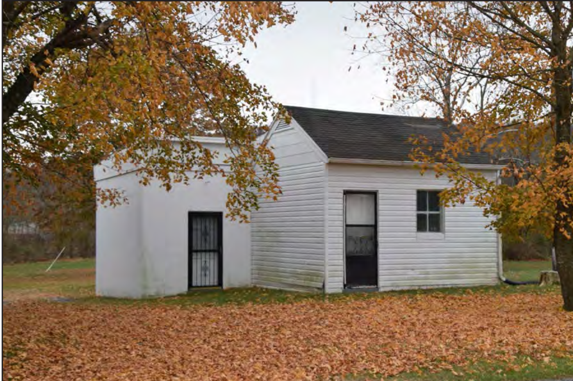
Figure 120. 007-5721, building, facing southeast.
