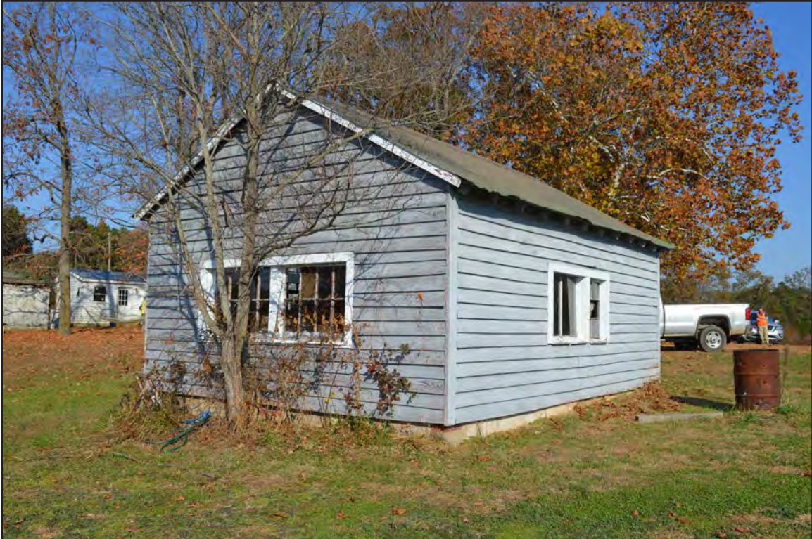
Figure 228. 014-5085, ca. 1930 outbuilding, facing northeast.
