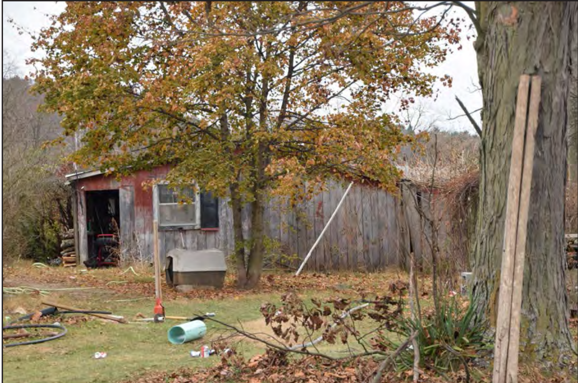
Figure 132. 007-5724, shed, facing northeast.
