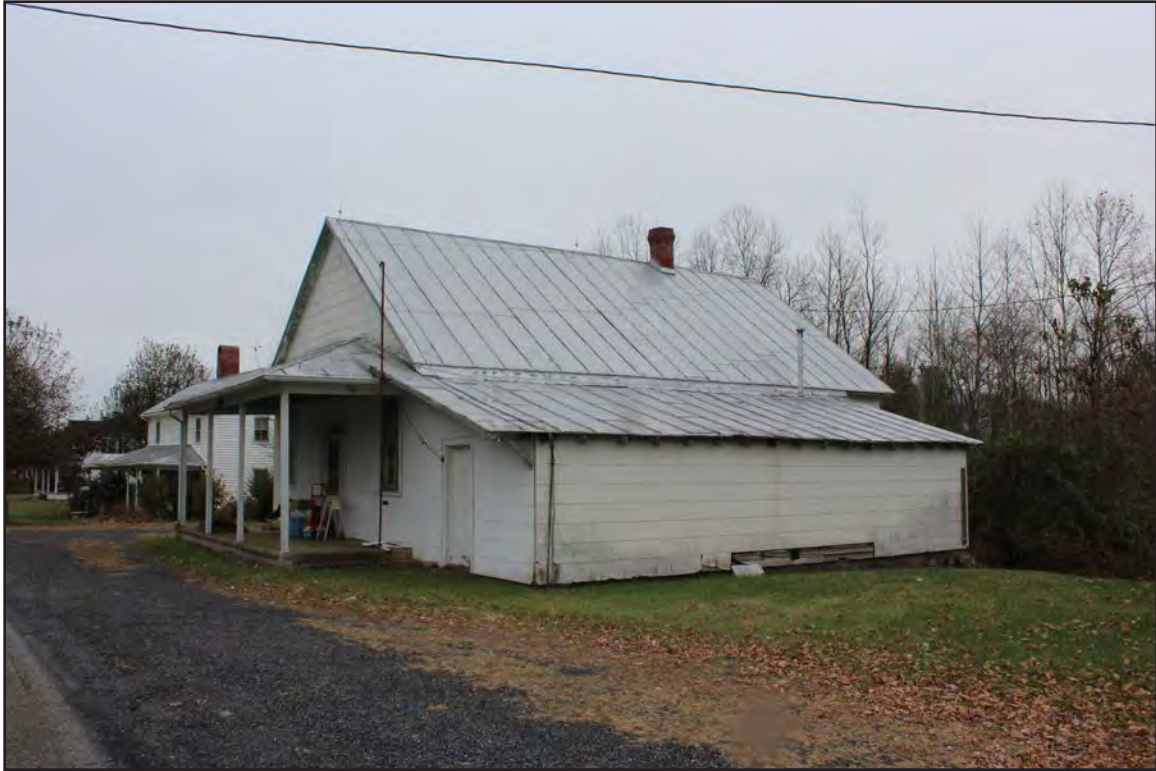
Figure 17. 007-0476, store, facing southeast.
