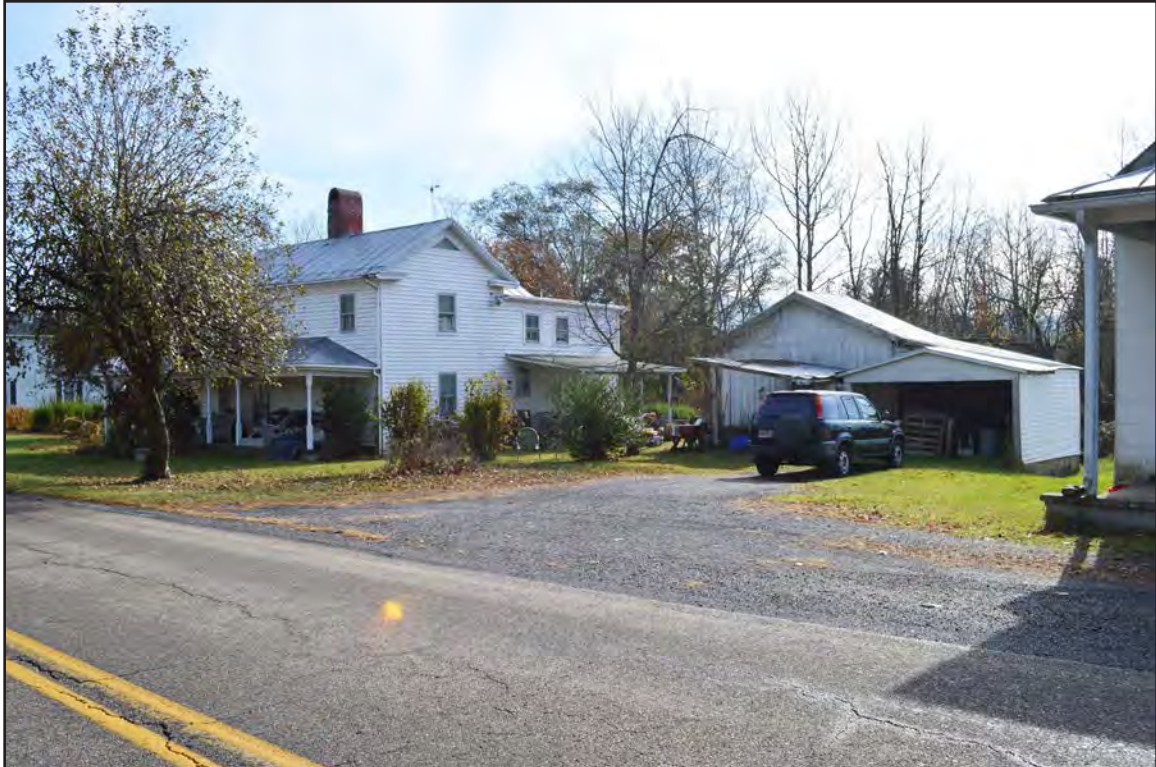
Figure 18. 007-0476, dwelling house, facing southwest.
