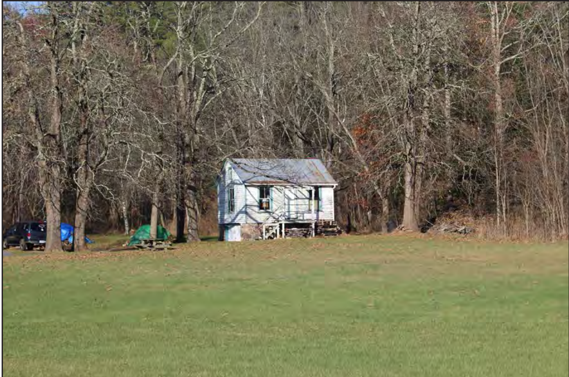
Figure 4. 007-0447. Outbuilding 1, facing southeast.
