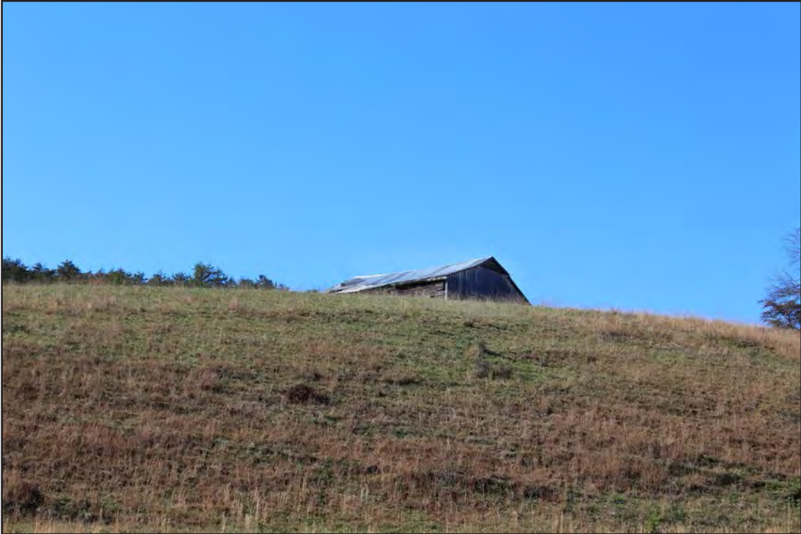
Figure 214. 008-5065, barn, facing west.
