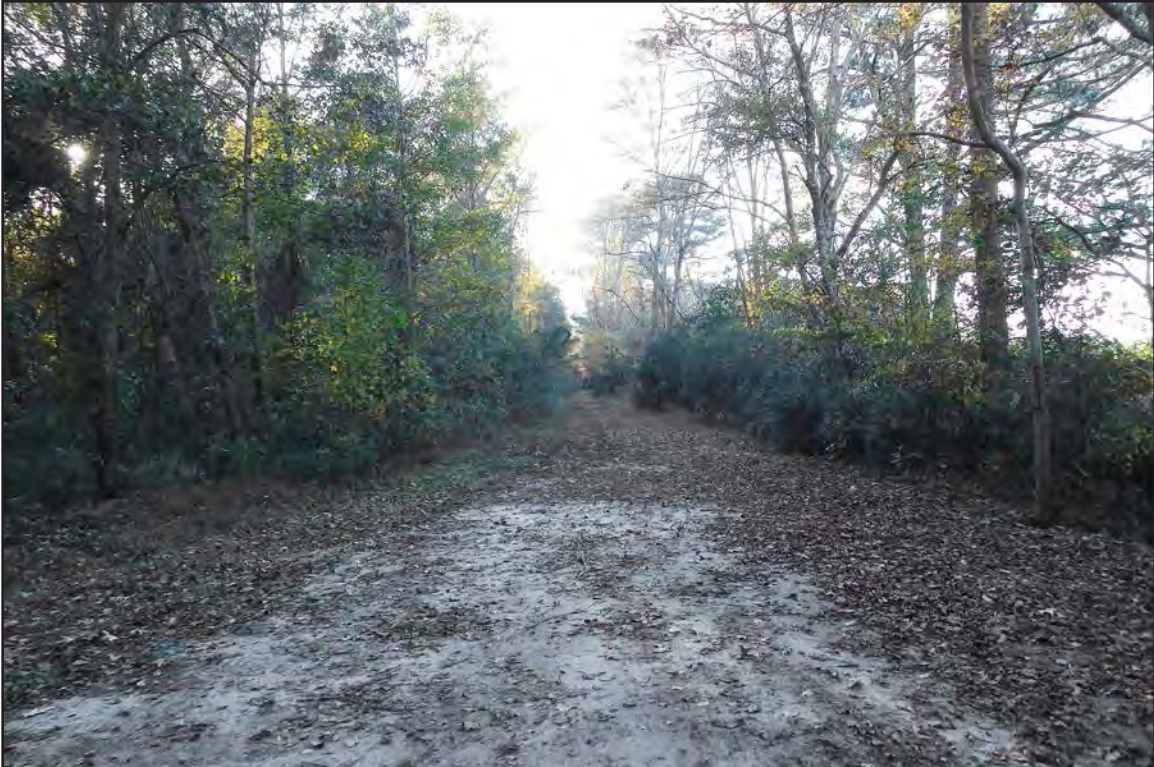
Figure 262. 131-5325, proposed access road 27-002-AR1, facing west.
