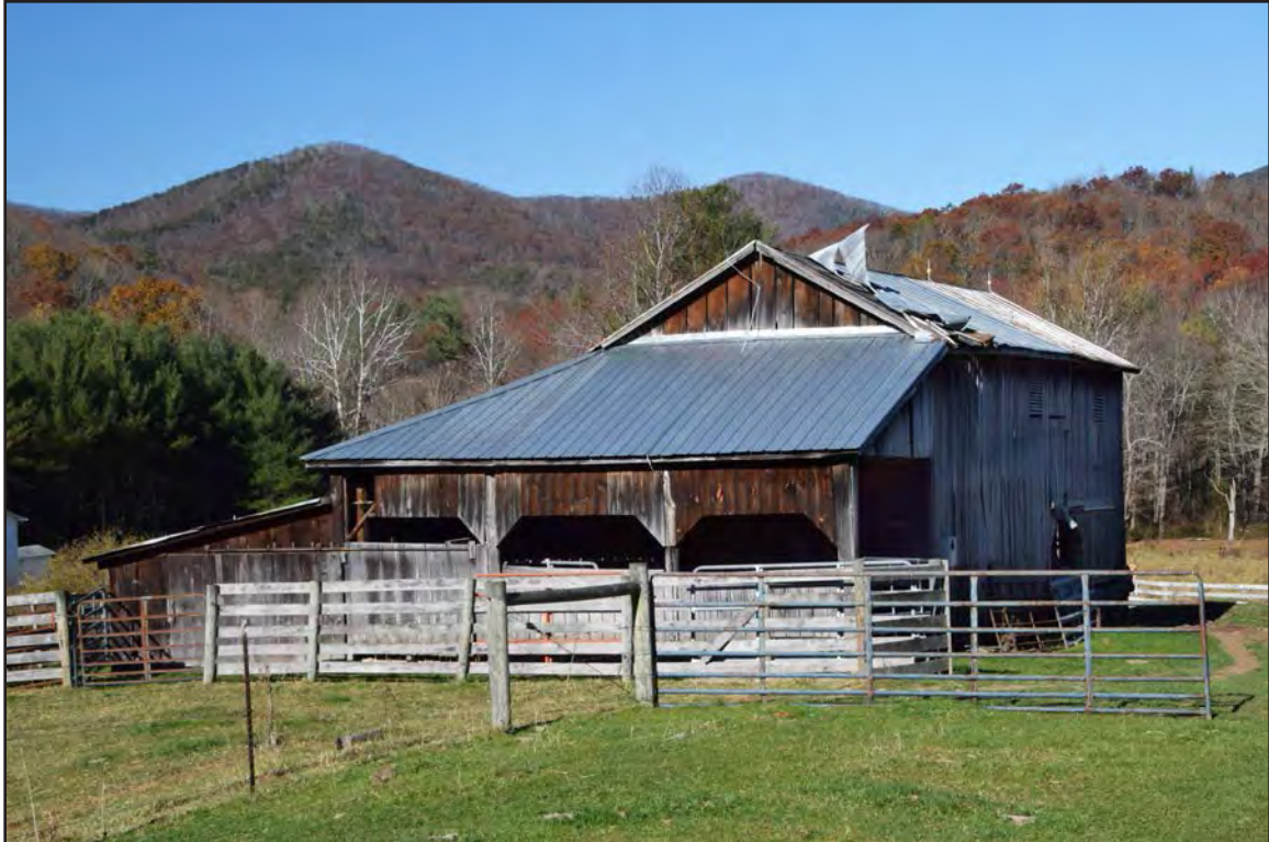
Figure 66. 007-5709, corn crib and barn, facing east.
