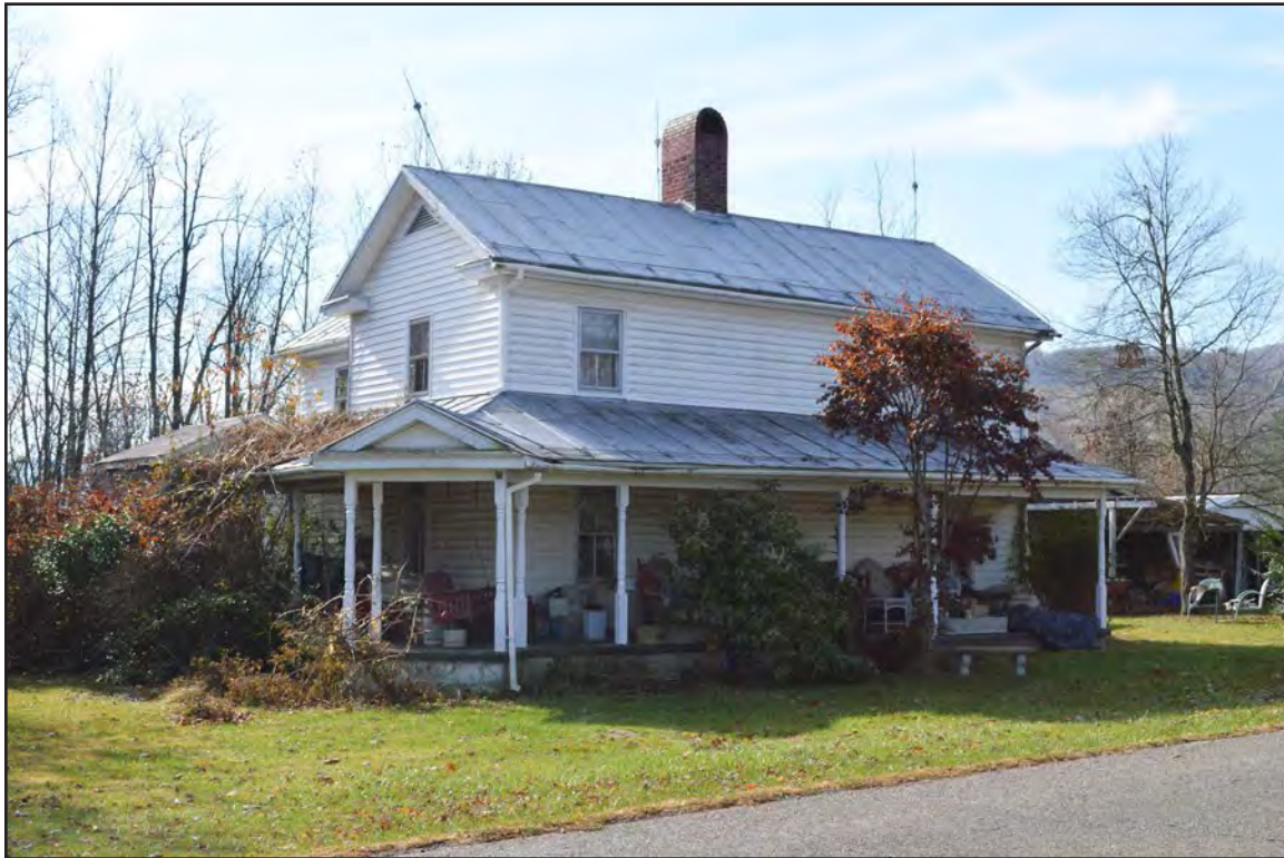
Figure 19. 007-0476, dwelling house, facing southwest.
