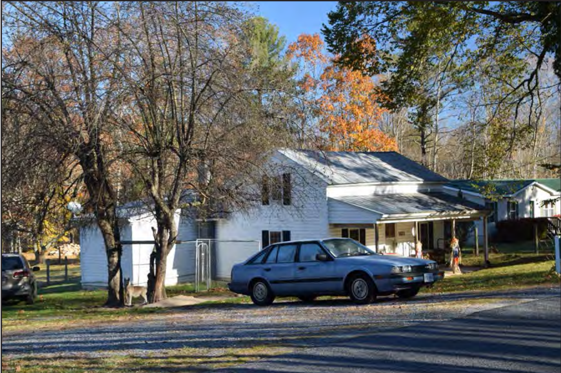
Figure 94. 007-5715, house, facing northeast.
