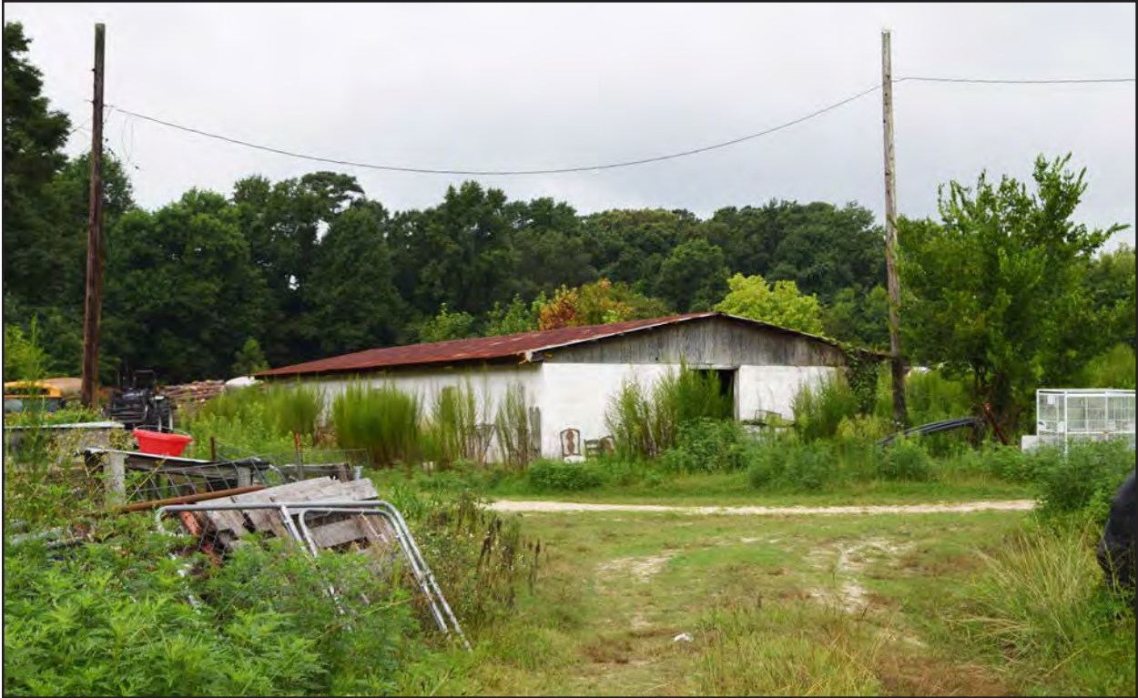
Figure 242. 133-0215 historic barn 1, facing southeast.
