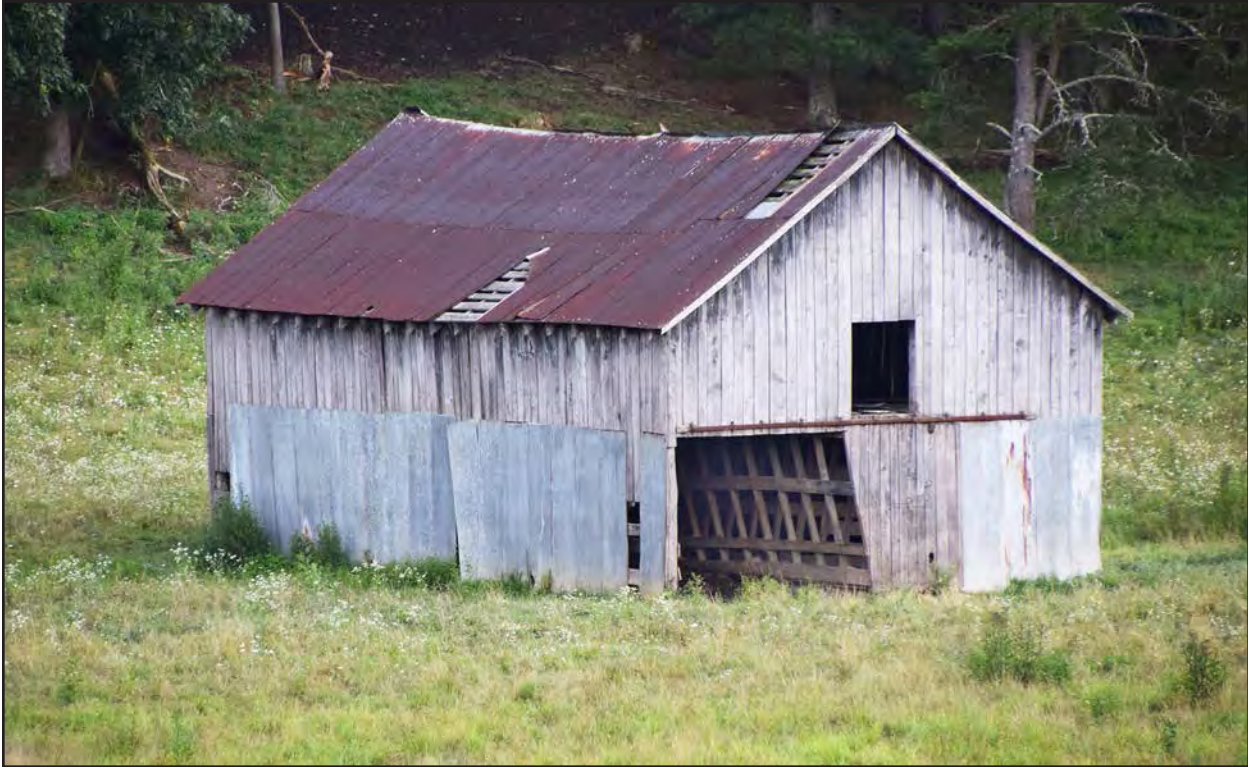
Figure 36. 007-0480, barn 1, facing south.
