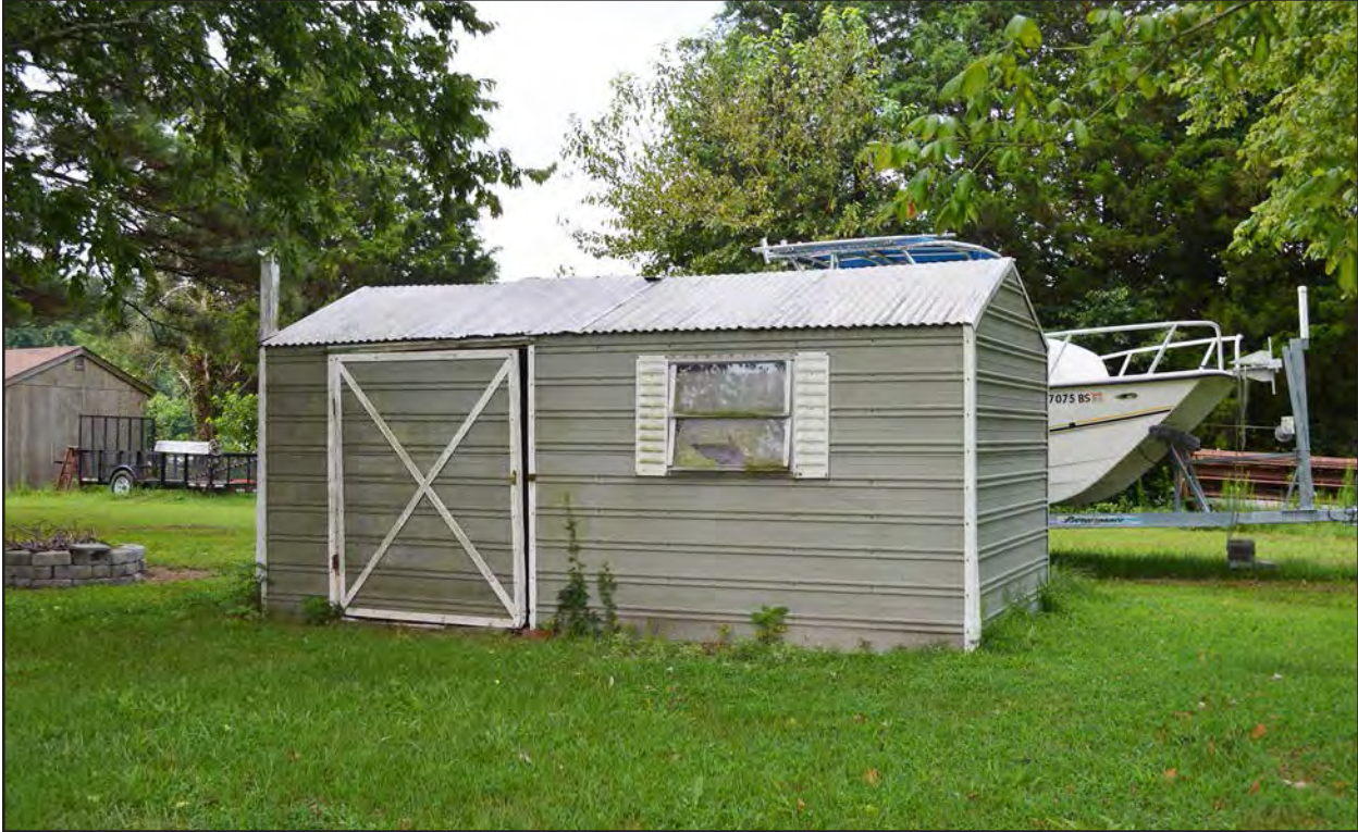
Figure 270. 133-5566, shed 1, facing southwest.
