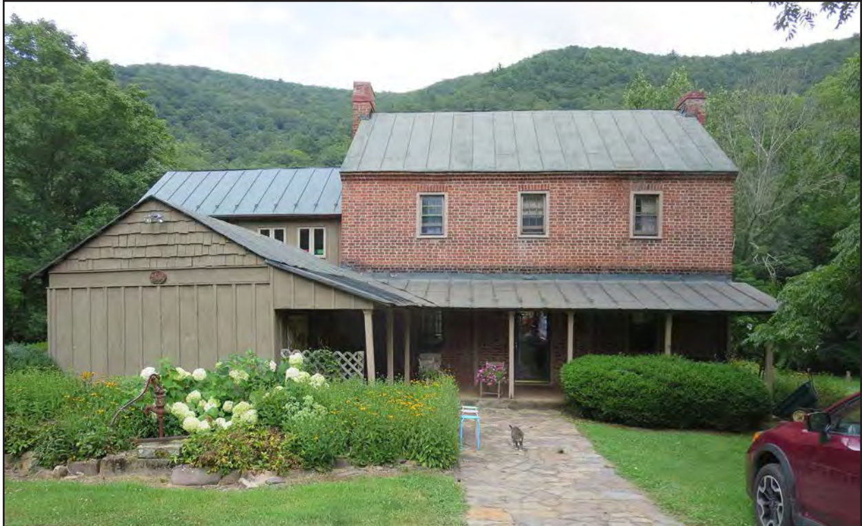
Figure 166. 045-0007, view of west elevation, facing east.
