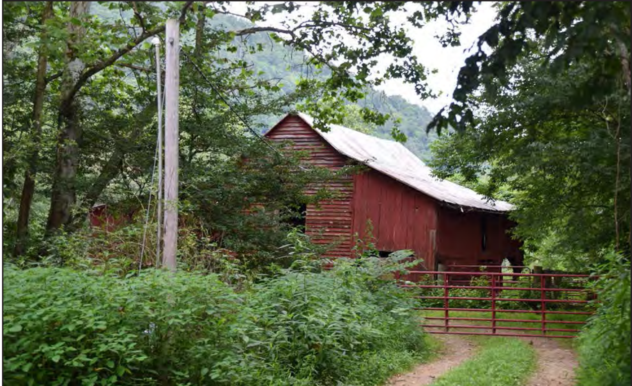
Figure 168. 045-0007, barn, facing south.
