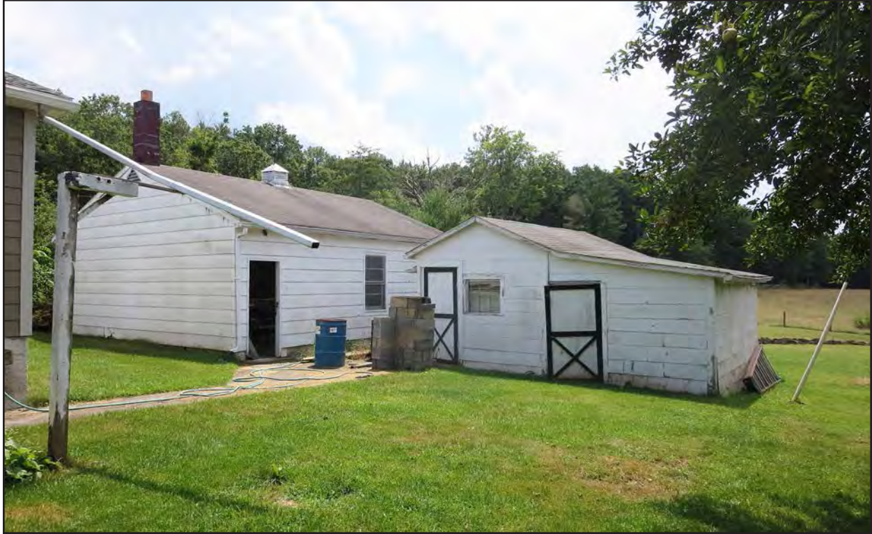
Figure 139. 008-5056, garage and accessory building, facing south.
