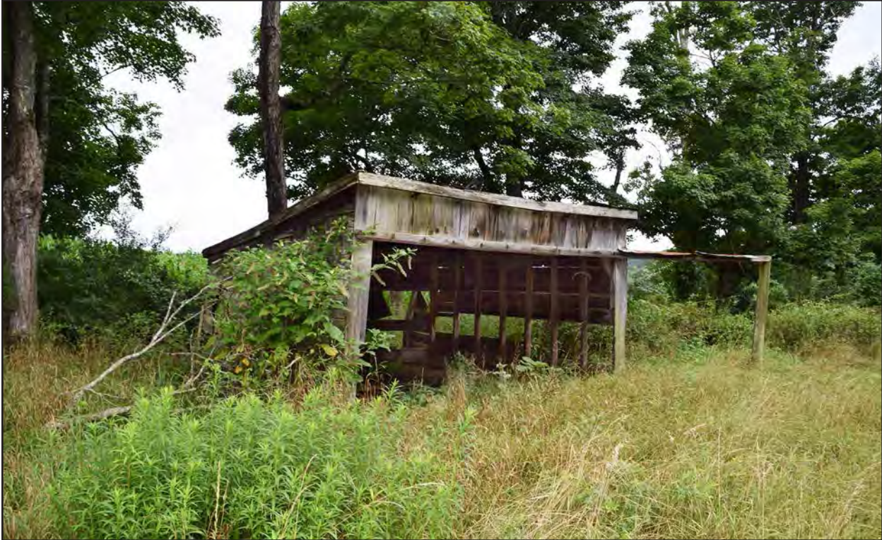
Figure 29. 007-0457, shed 2, facing southwest.
