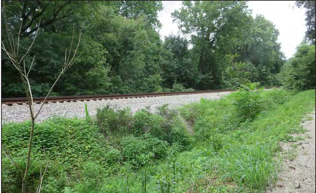
Figure 226. 062-5180, from Midway Mills Lane, facing south-southeast.
