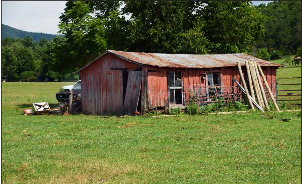
Figure 88. 007-5691, shed 2, facing northeast.
