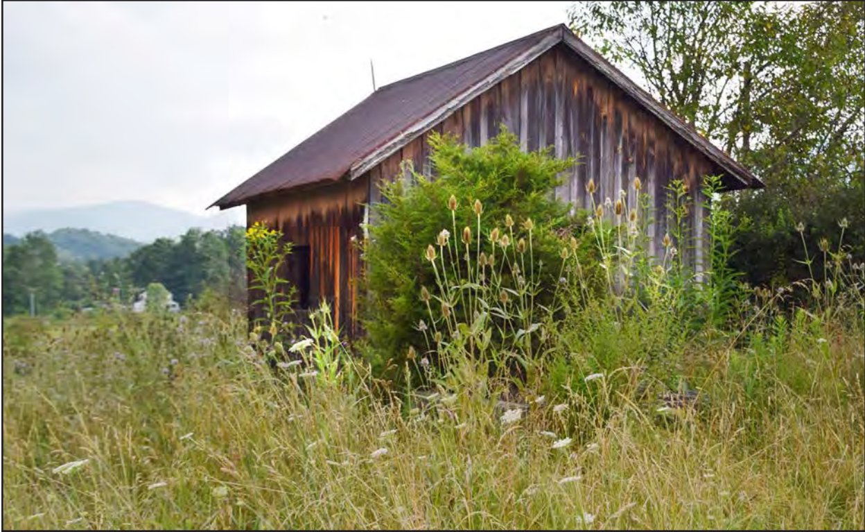
Figure 35. 007-0480, shed 1, facing east.
