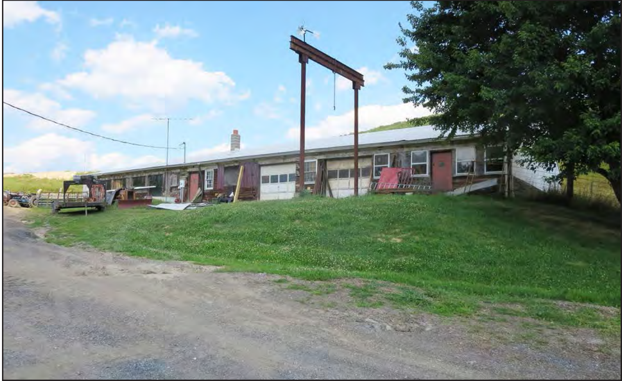
Figure 159. 008-5063, turkey house, facing east.
