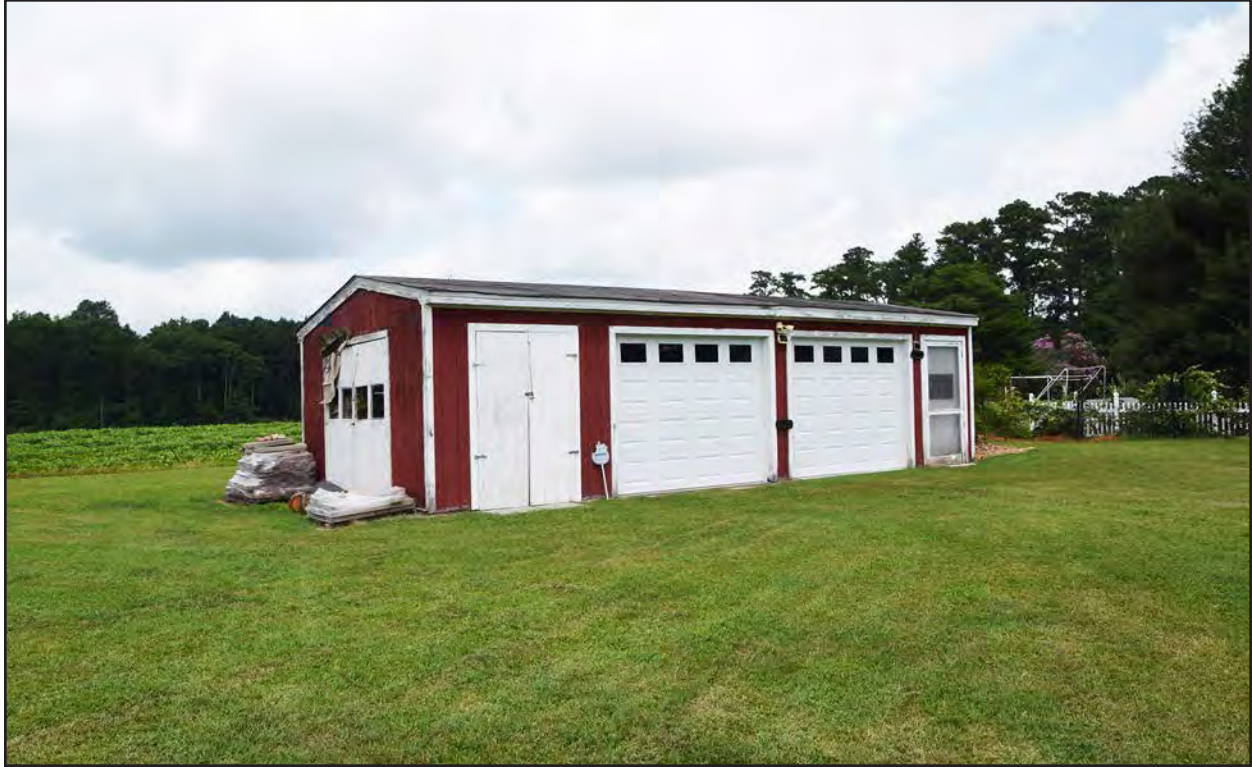
Figure 293. 133-5575, shed, facing northeast.
