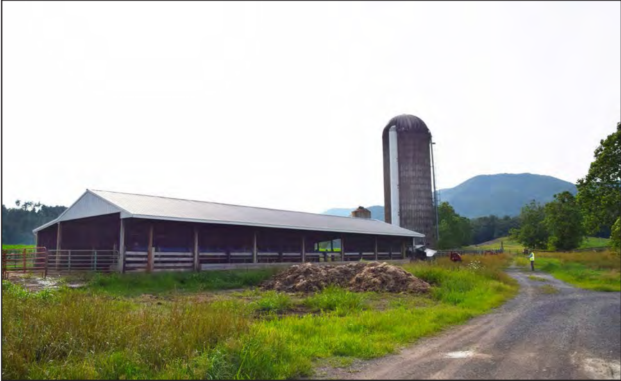
Figure 15. 007-0103, barn, facing north-northwest.
