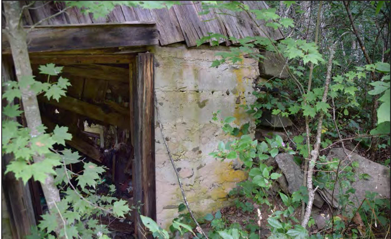
Figure 196. 045-5079, root cellar, facing northeast.
