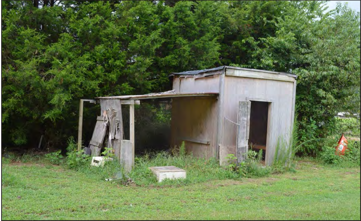
Figure 271. 133-5566, shed 2, facing west.
