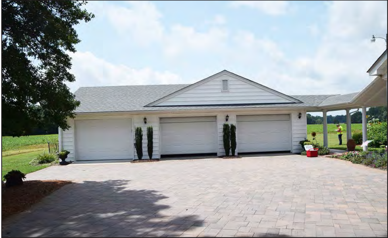
Figure 291. 133-5575, garage, facing west.
