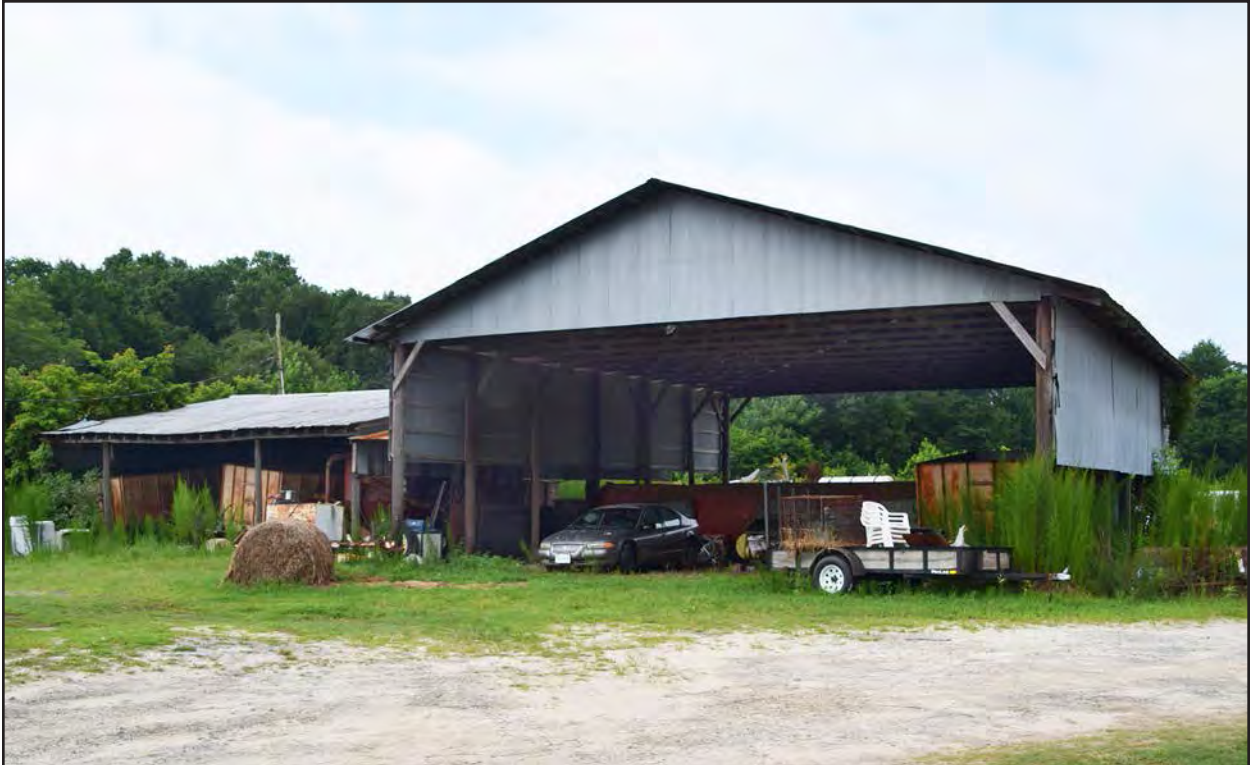
Figure 244. 133-0215 historic barn 2, facing southwest.
