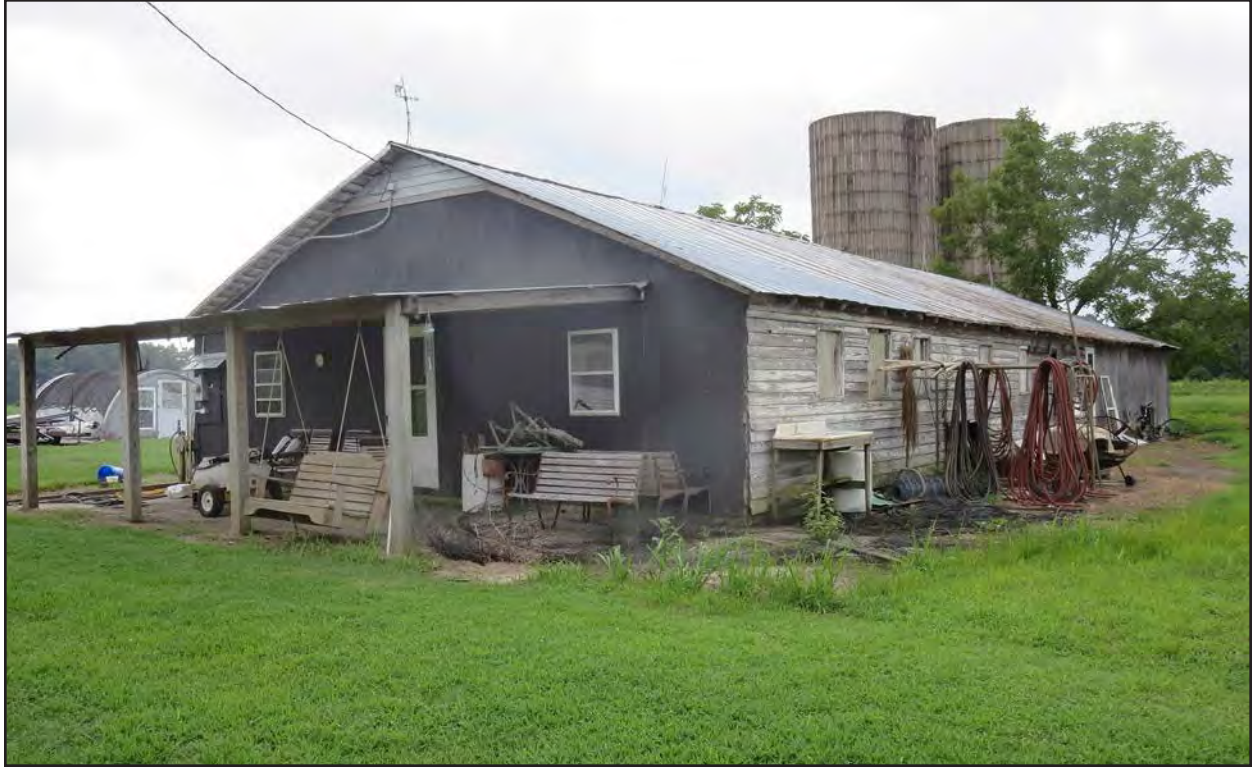
Figure 275. 133-5571, agricultural outbuilding 1 addition showing original rear section, facing southwest.
