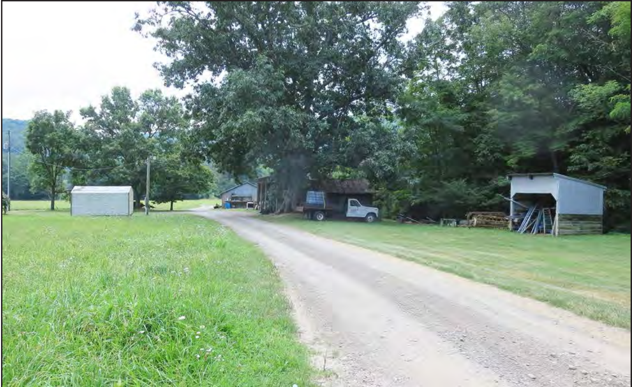
Figure 54. 007-5682, historic and modern outbuildings, facing south.
