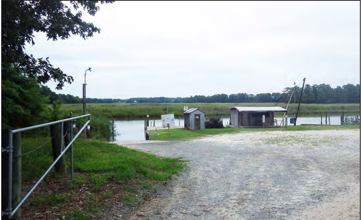
Figure 246. 133-5039, marina, facing northeast.
