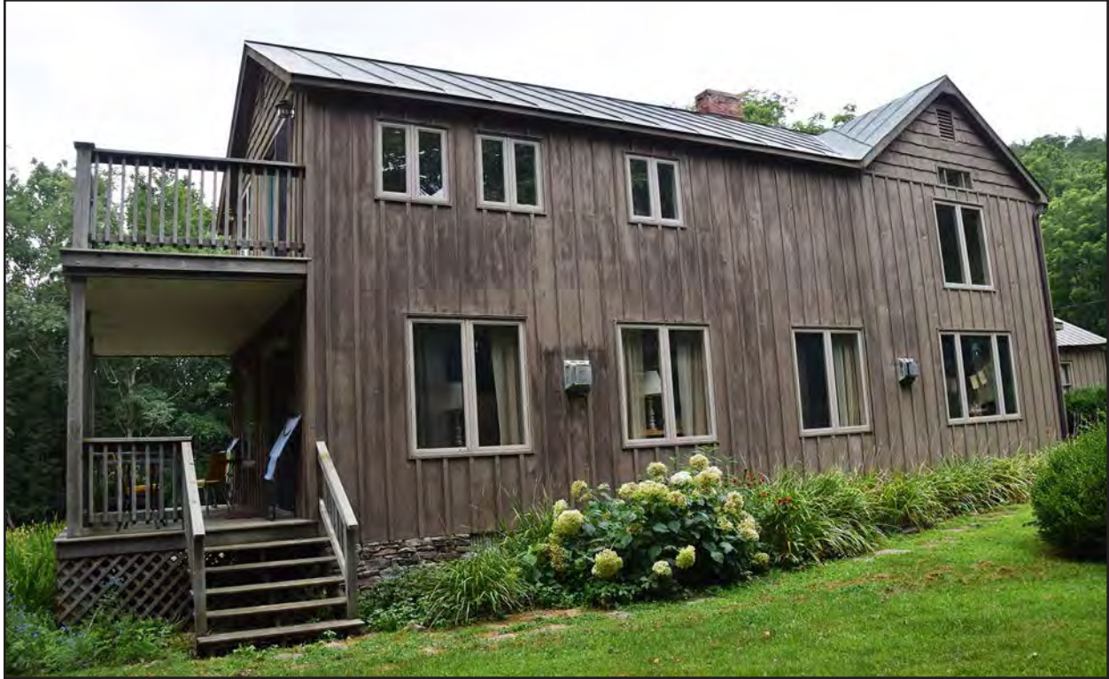
Figure 167. 045-0007, view of additions, facing south.
