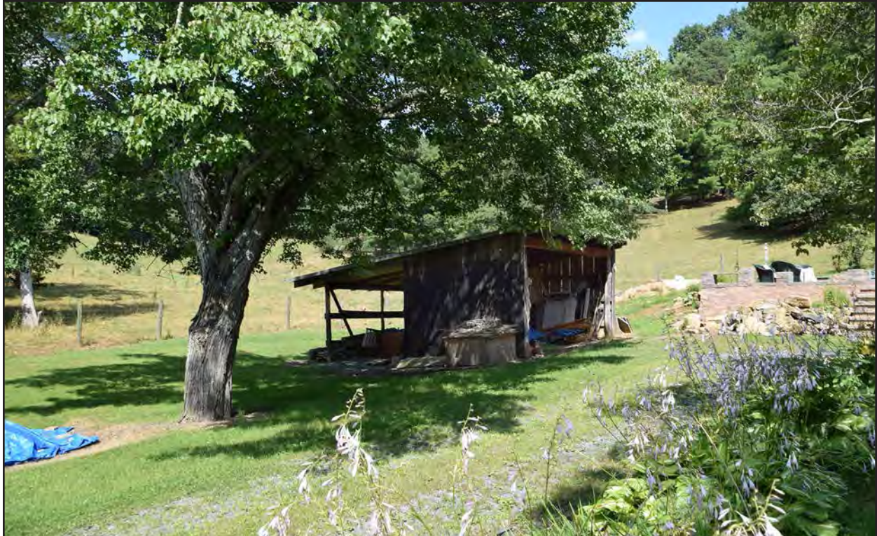
Figure 156. 008-5062, one bay shed, facing east.
