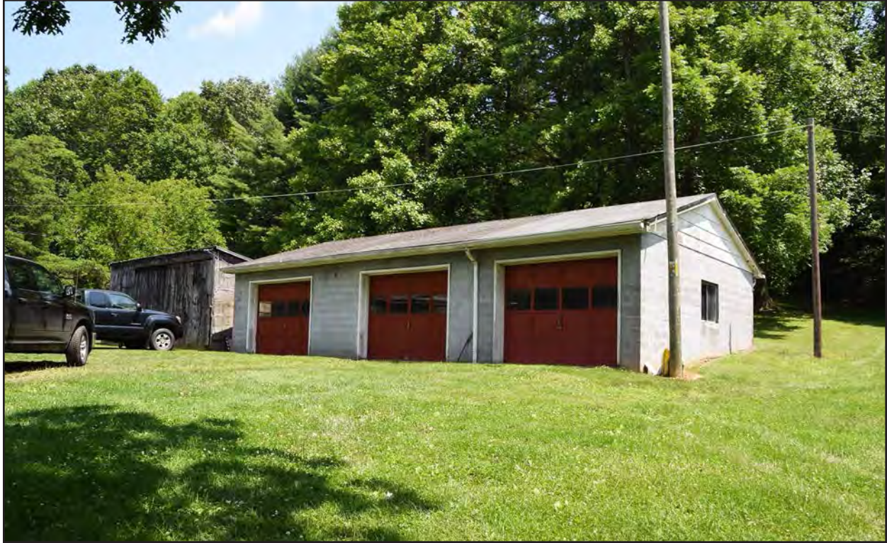
Figure 59. 007-5683, garage and shed, facing southwest.
