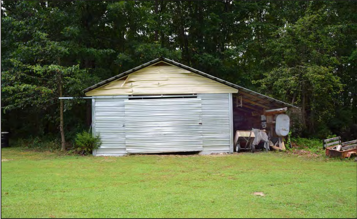
Figure 45. 007-5596, shed, view south.
