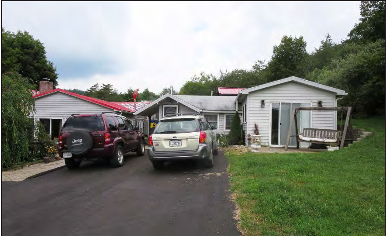
Figure 101. 007-5693, accessory building, facing northwest.
