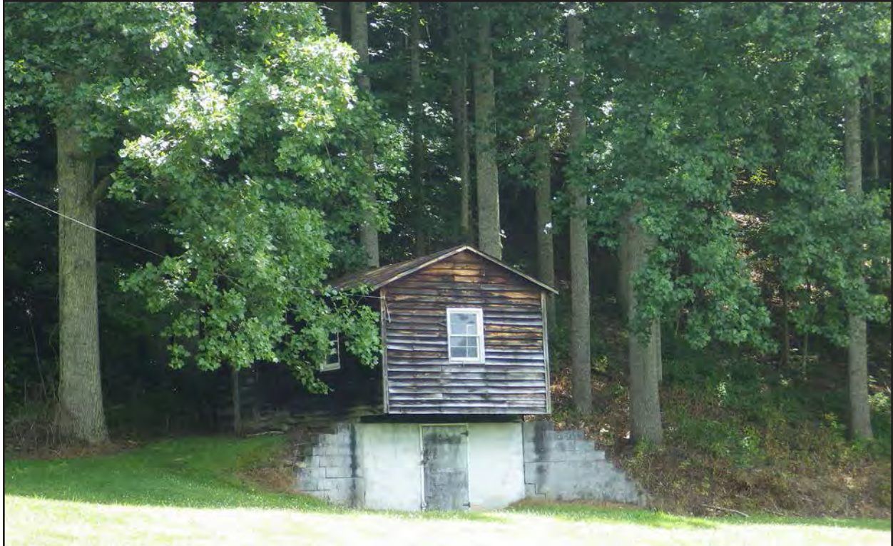
Figure 58. 007-5683, root cellar, facing south.
