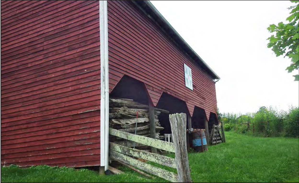
Figure 175. 045-0055, barn 1, facing north-northwest.
