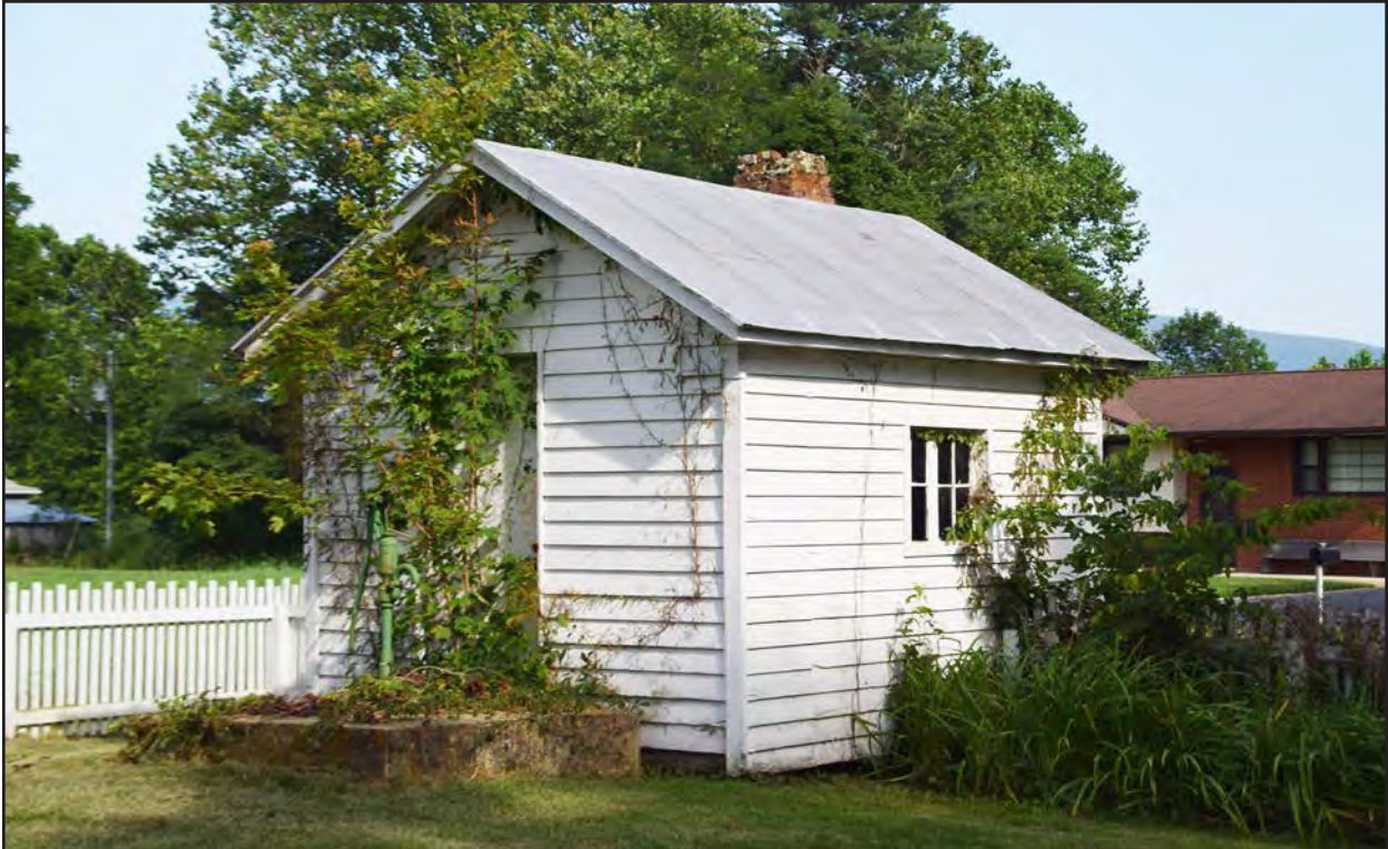
Figure 6. 007-0103, summer kitchen, facing south.
