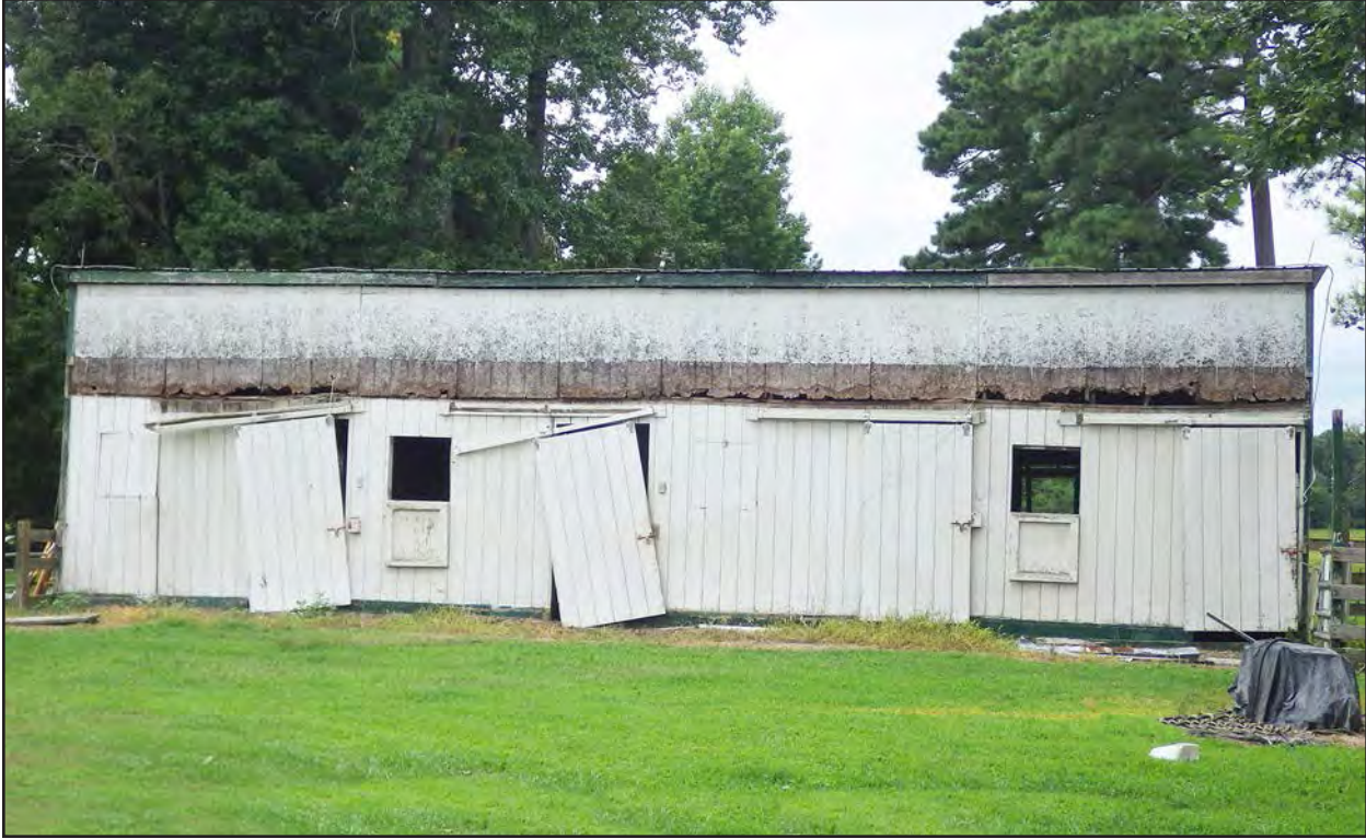
Figure 296. 133-5578, barn 1 facing west.
