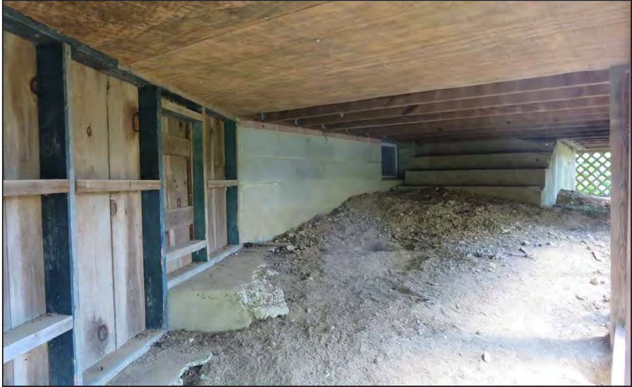
Figure 155. 008-5062, beneath front porch, facing south.
