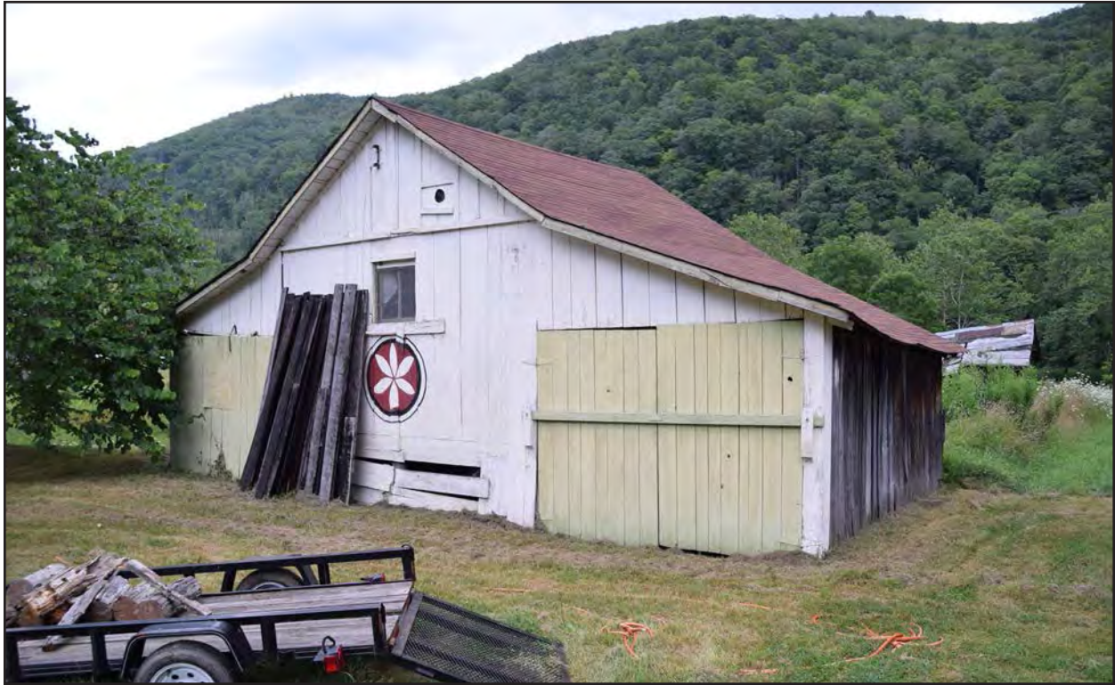
Figure 209. 045-5082, barn, facing west.
