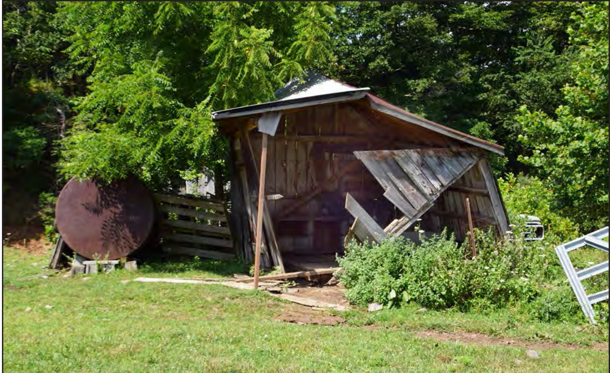
Figure 90. 007-5691, shed 4, facing southwest.
