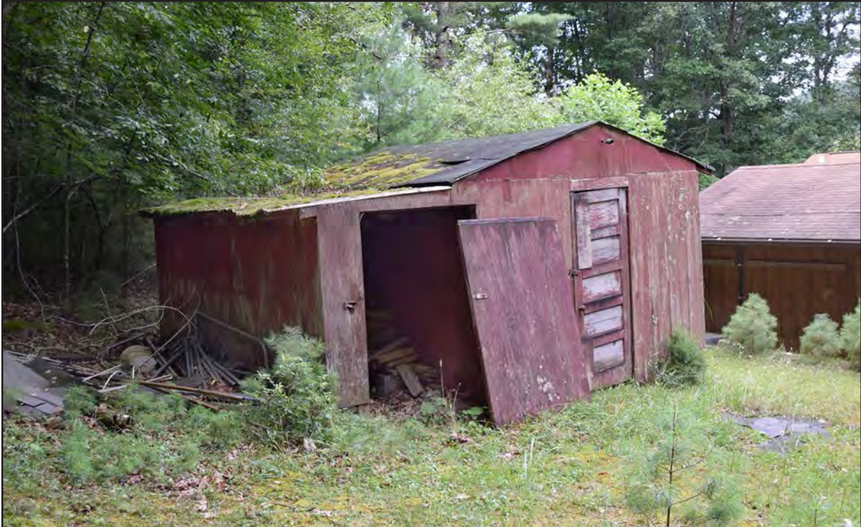
Figure 148. 008-5060 shed, facing west.
