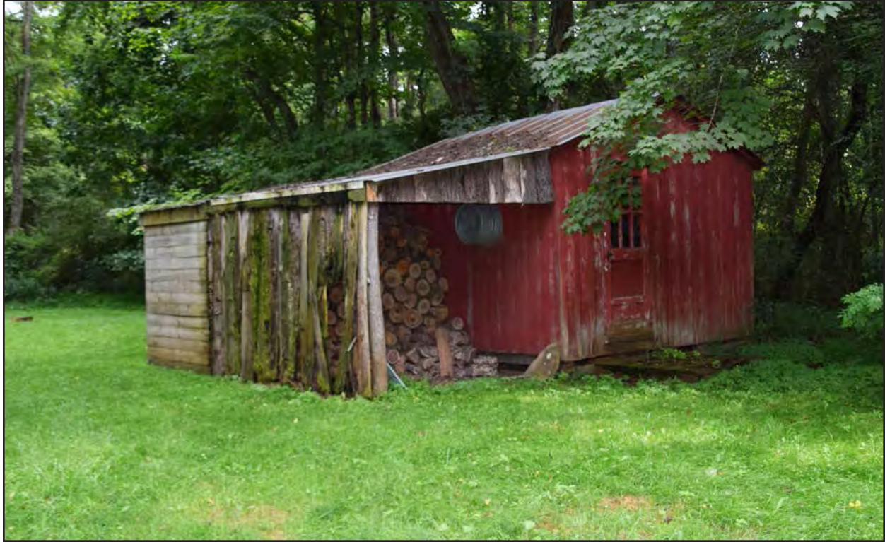
Figure 23. 007-0455, shed, facing southwest.
