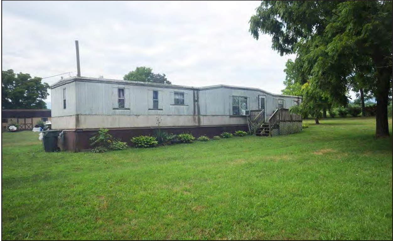
Figure 119. 007-5698, modular home, facing southwest.
