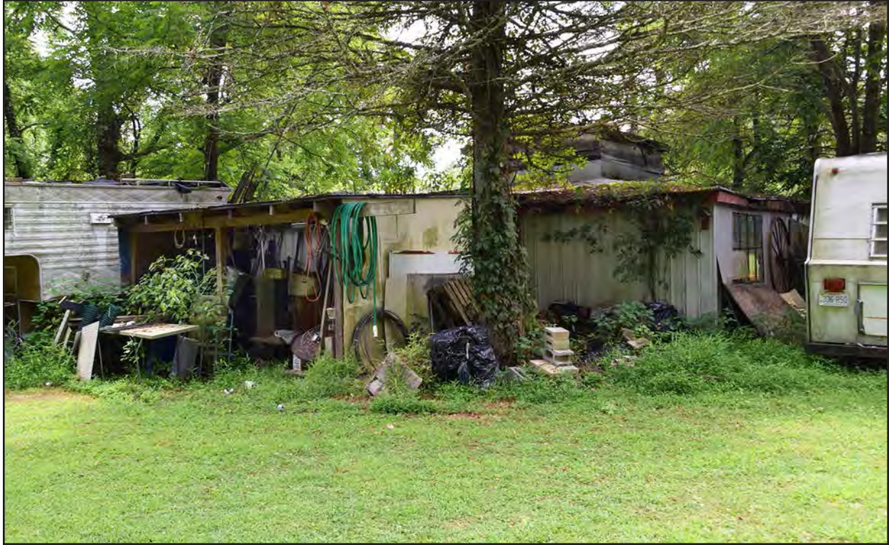
Figure 71. 007-5686, outbuilding, facing south.
