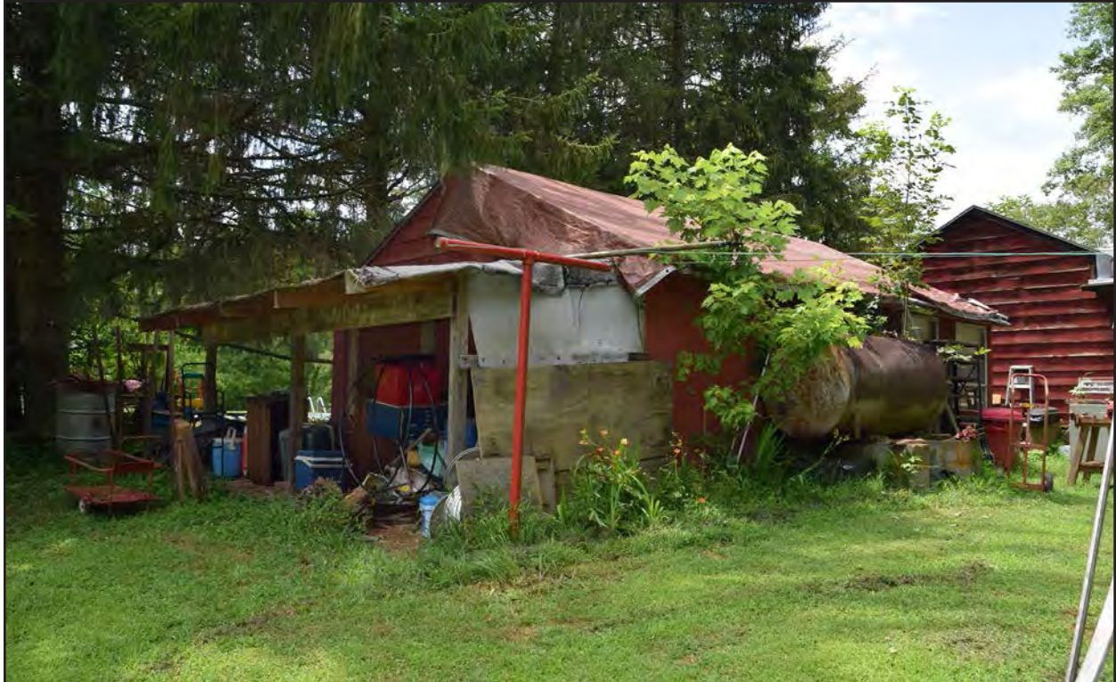
Figure 70. 007-5686, shed, facing west.
