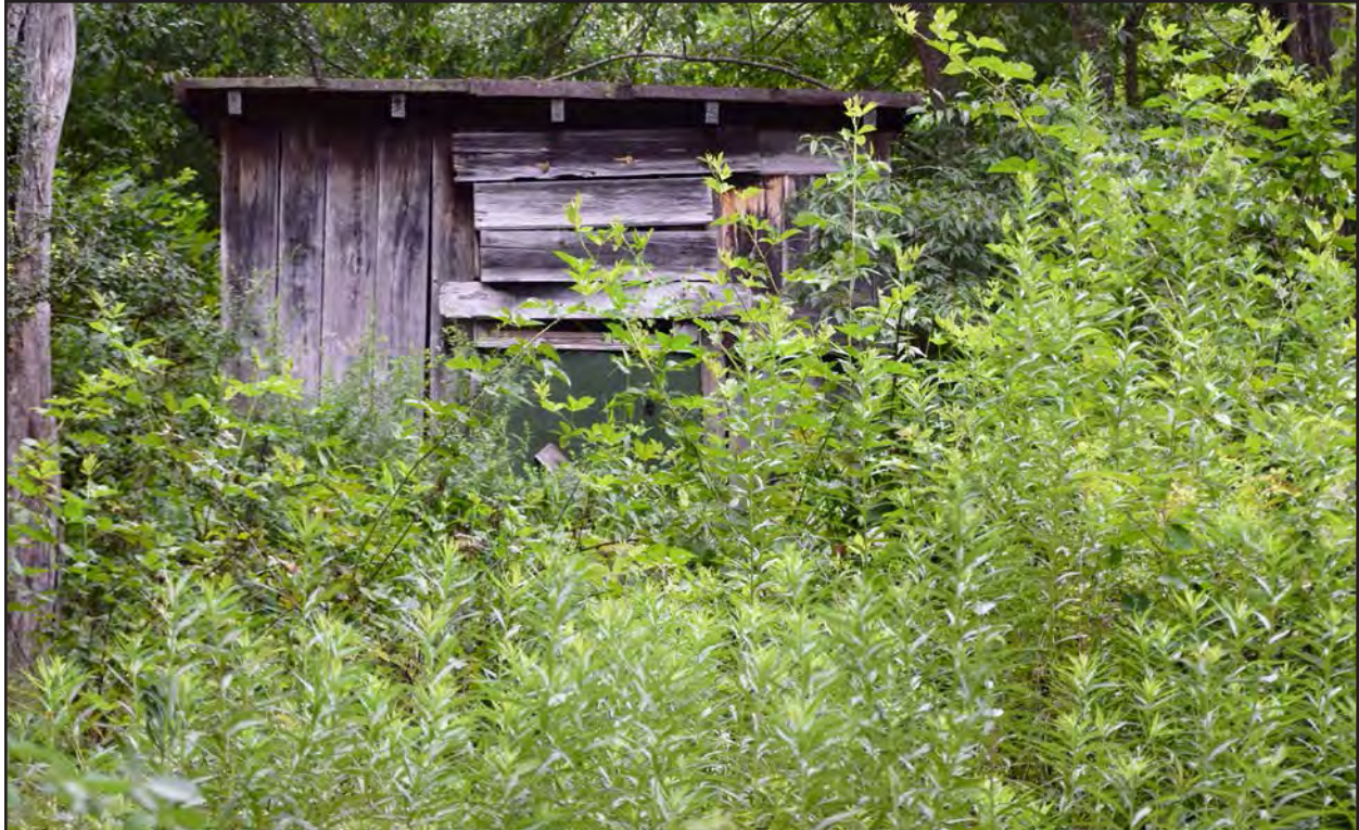
Figure 28. 007-0457, shed 1, facing east. 28
