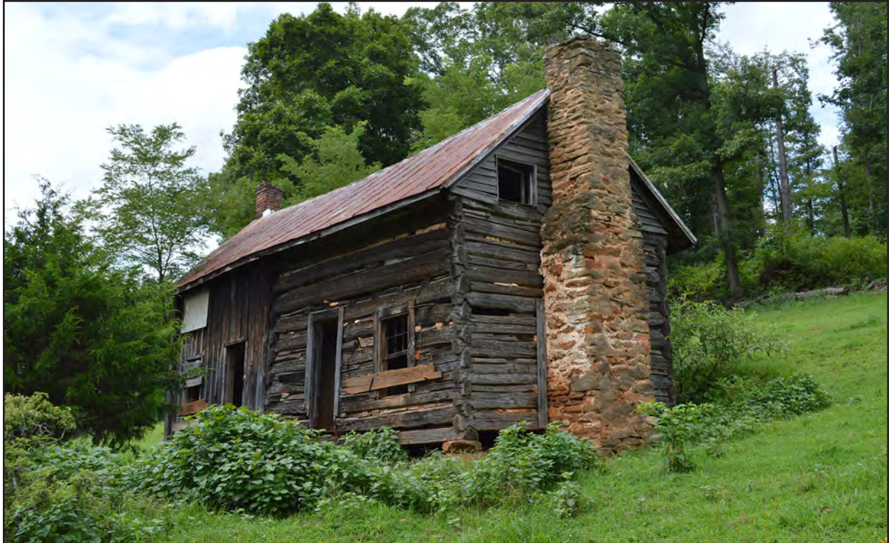
Figure 228. 062-5221, log cabin, facing northwest.
