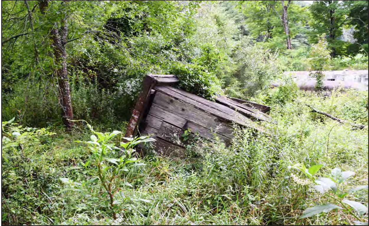
Figure 27. Outhouse, 007-0457, facing south.
