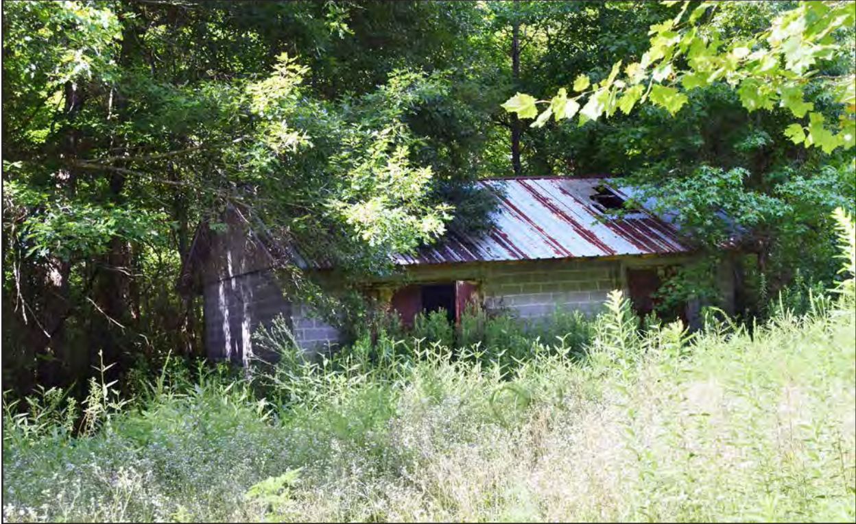
Figure 278. 133-5572, storage structure, facing northeast.
