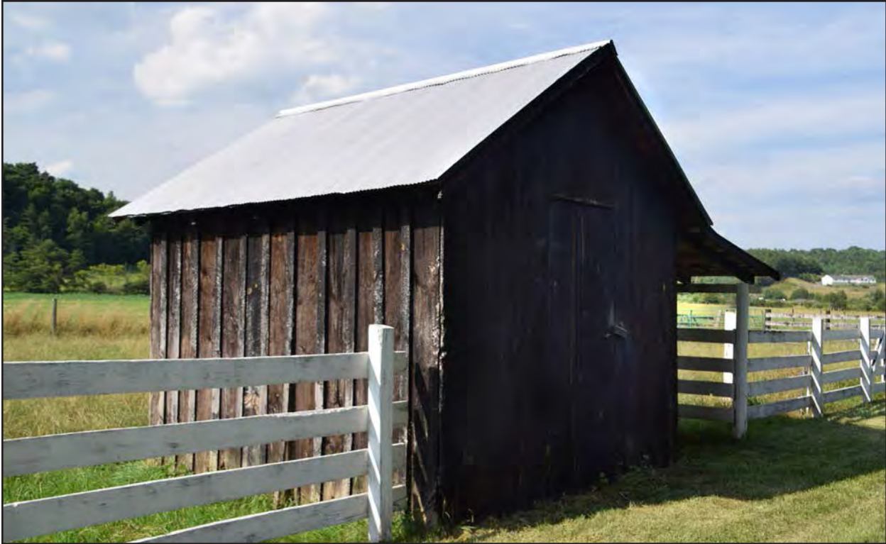
Figure 8. 007-0103, shed, facing northeast.
