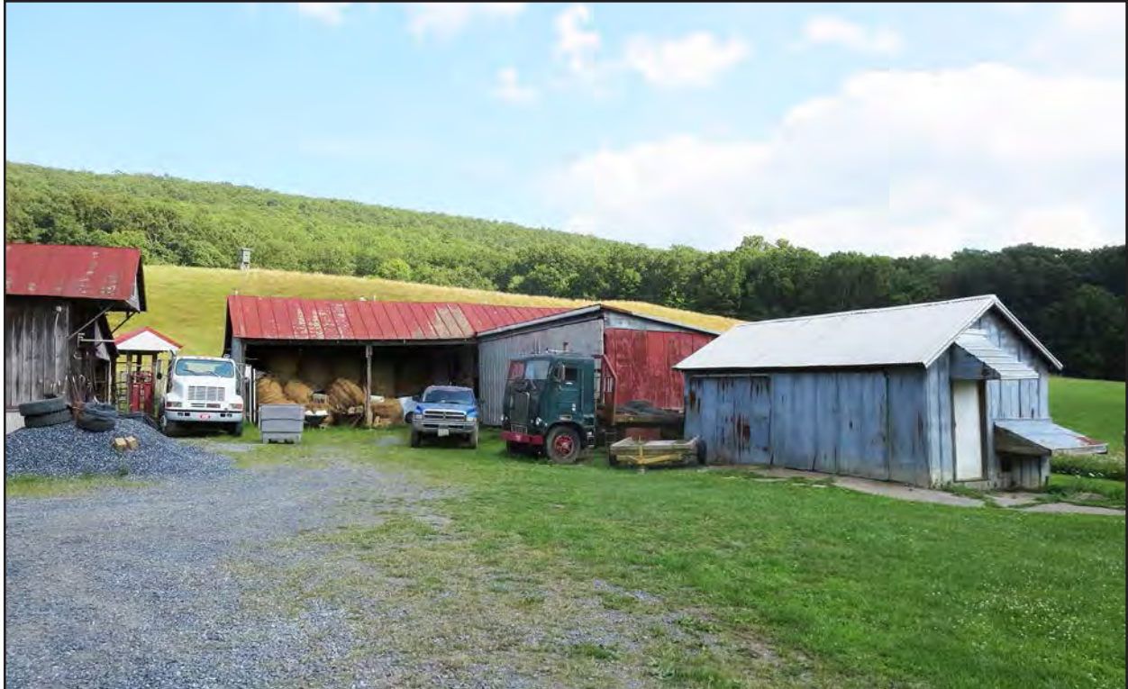
Figure 158. 008-5063, oldest outbuildings, facing southeast.
