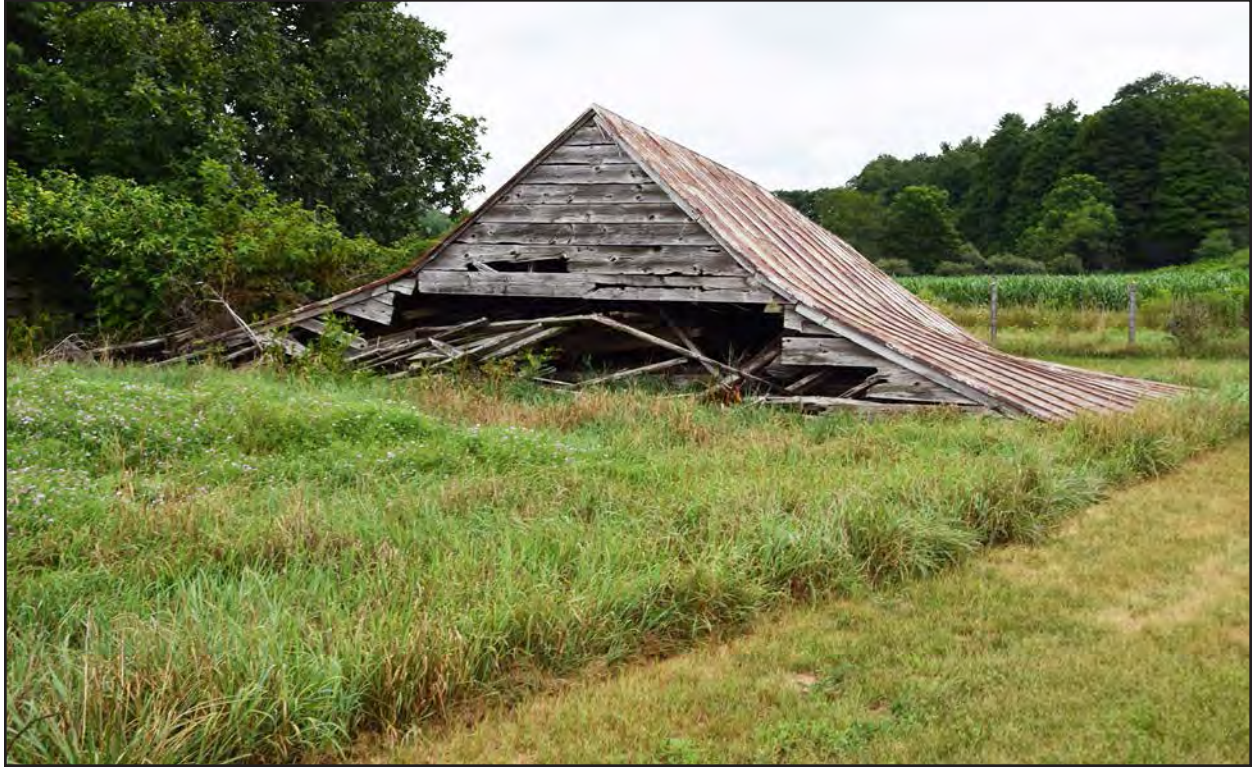
Figure 31. 007-0457, barn 2, facing south.
