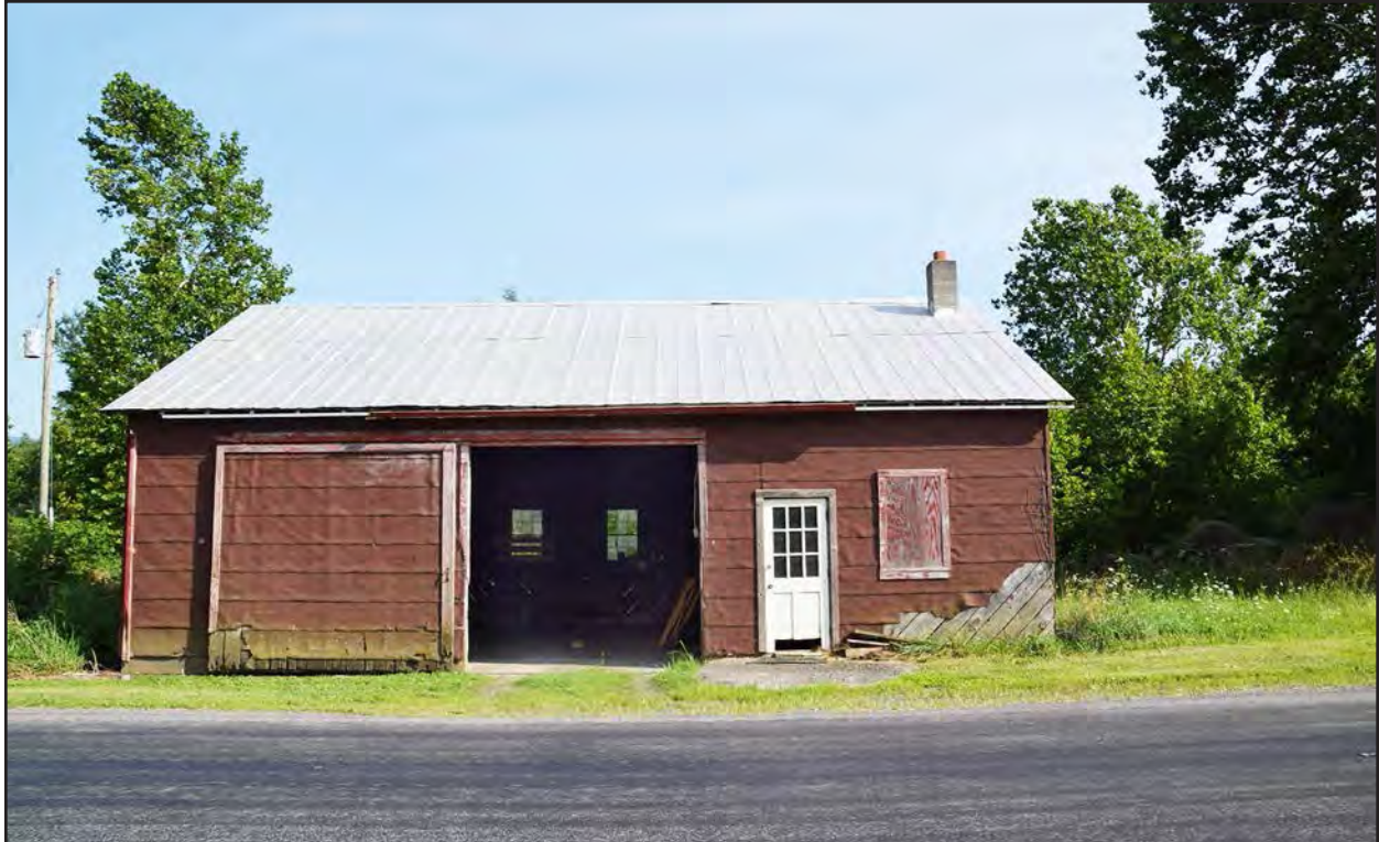
Figure 10. 007-0103, workshop, facing south.
