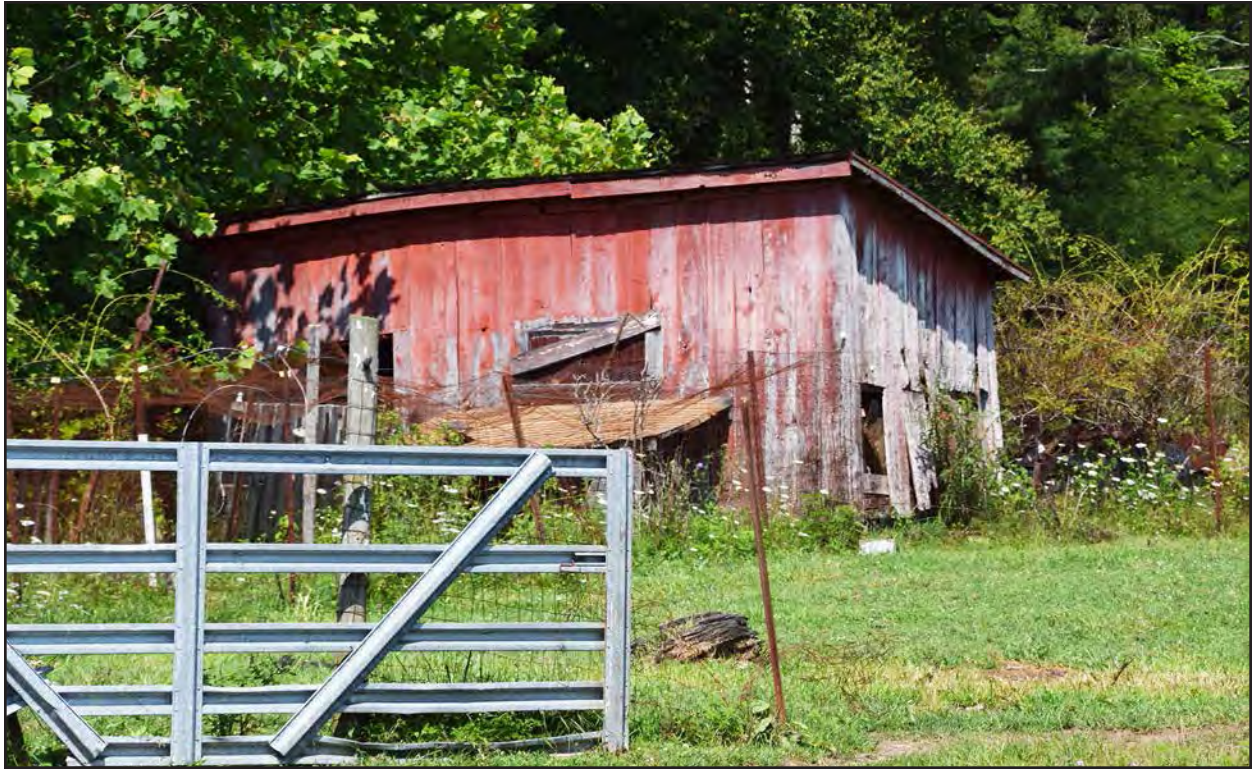
Figure 89. 007-5691, shed 3, facing northwest.
