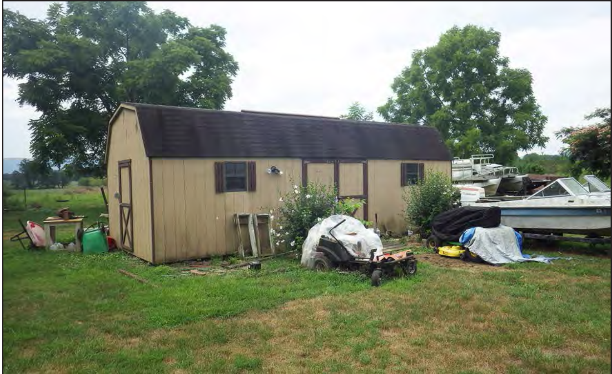
Figure 120. 007-5698, shed 1, facing southwest.
