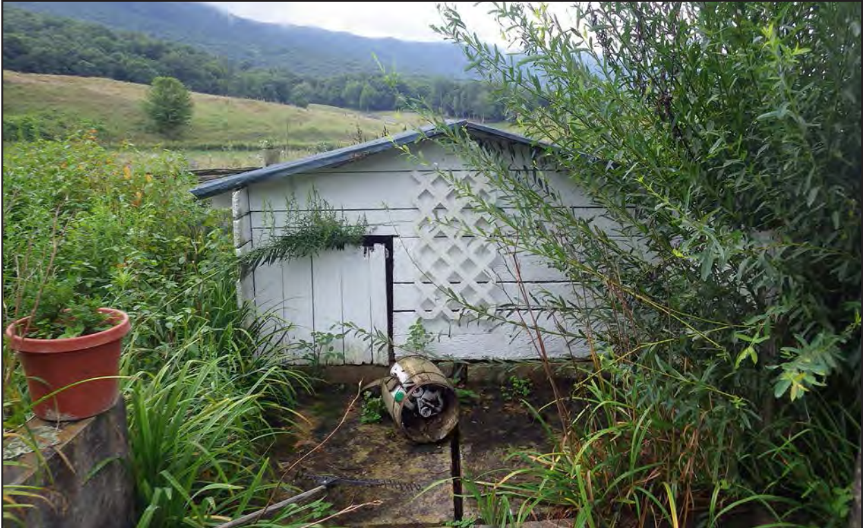
Figure 182. 045-0055, shed 2, facing south.
