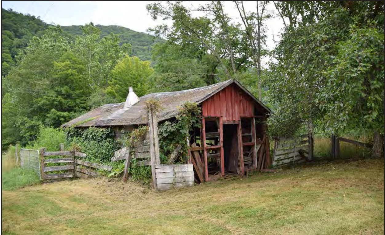
Figure 210. 045-5082, animal shelter, facing east.
