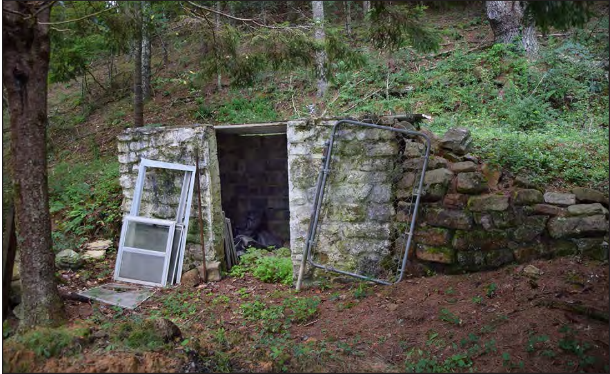
Figure 145. 008-5059, root cellar, facing south.
