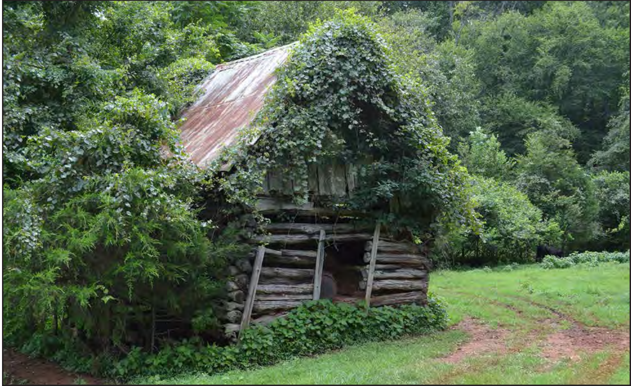
Figure 229. 062-5221, log barn 1, facing south.
