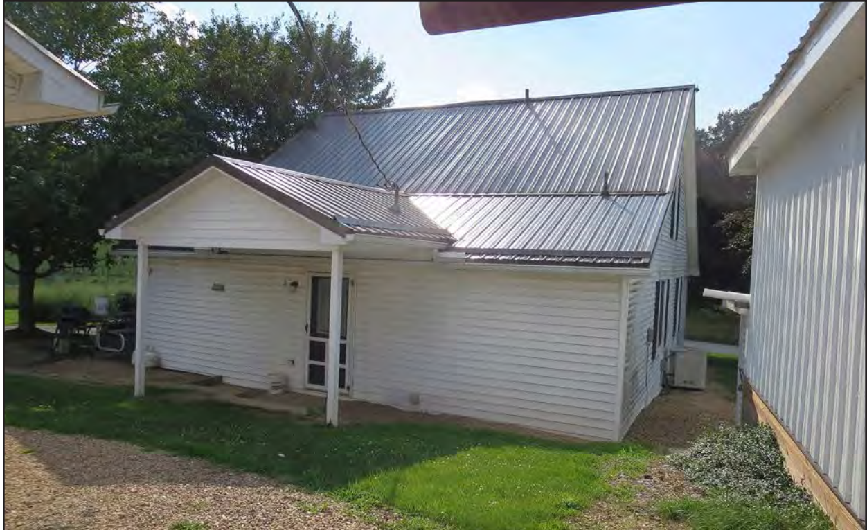
Figure 160. 008-5063, rear of house, facing west.
