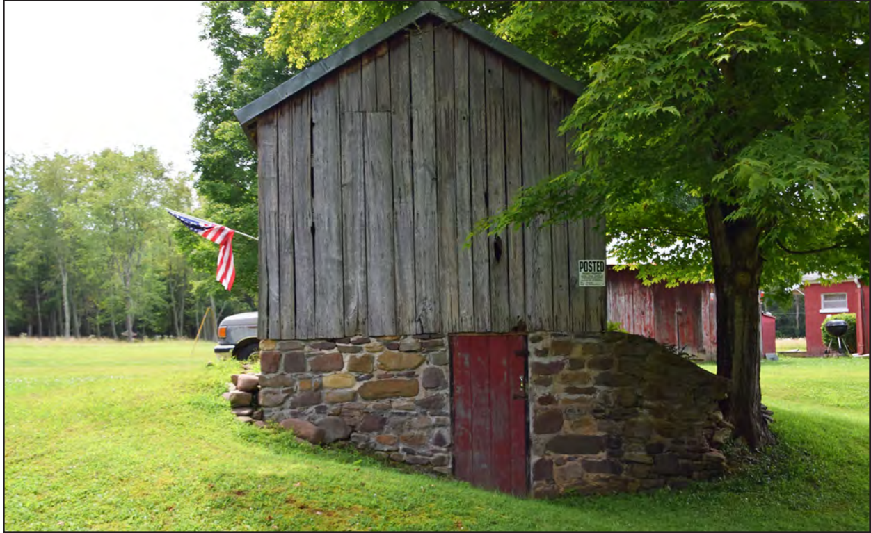
Figure 77. 007-5688, root cellar, facing south.
