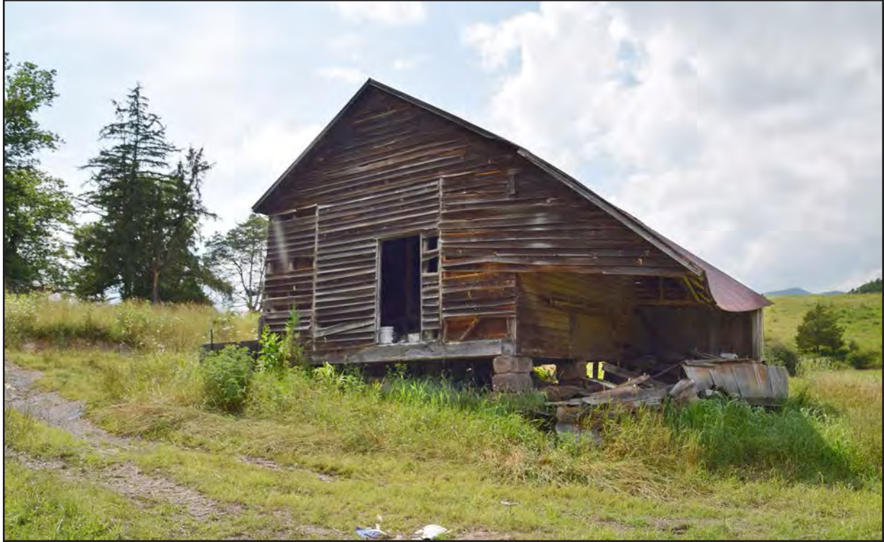
Figure 37. 007-0480, shed 2, facing northwest.
