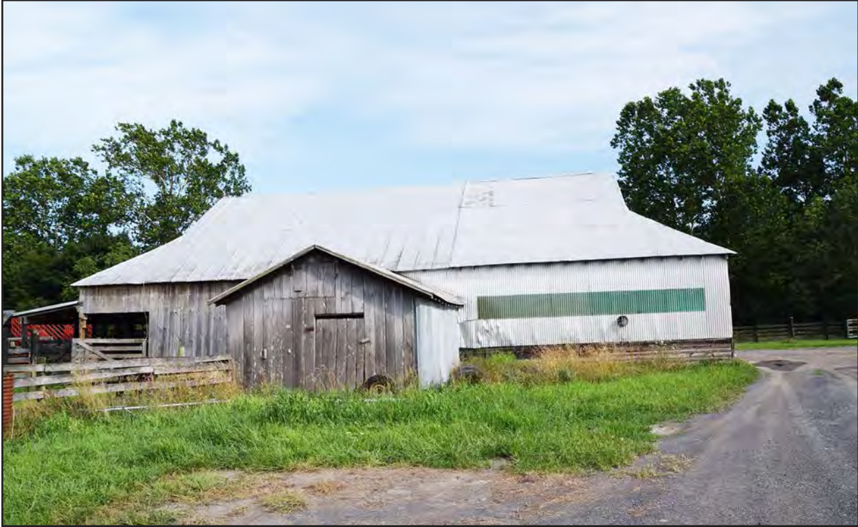
Figure 13. 007-0103, barn, facing south.
