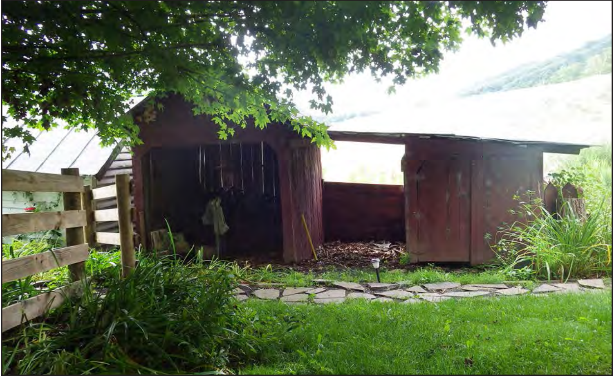
Figure 181. 045-0055, shed 2, facing southwest.
