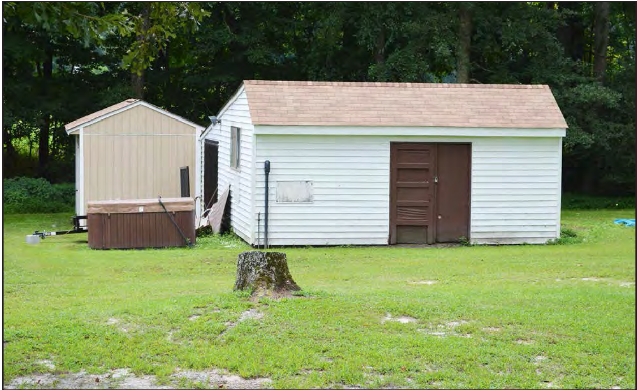
Figure 285. 133-5574, storage shed, facing south.
