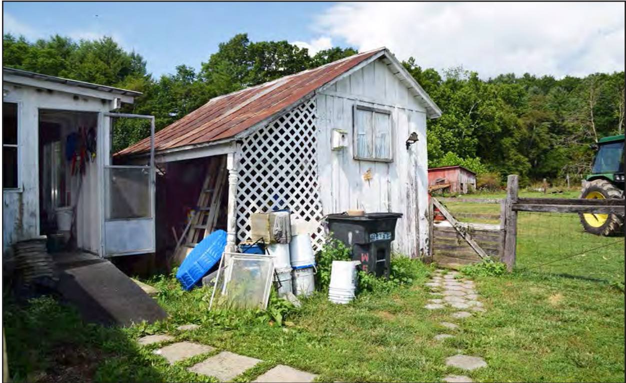
Figure 87. 007-5691, shed 1, facing northwest.
