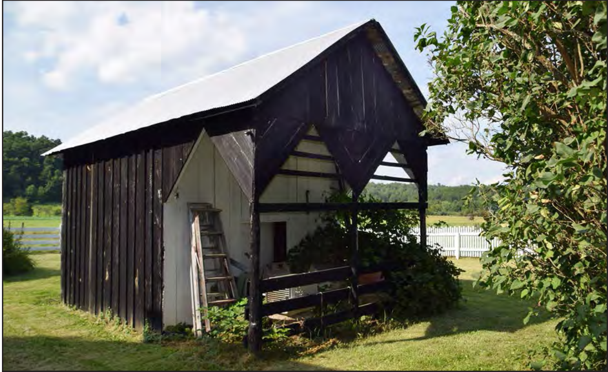
Figure 9. 007-0103, shed, facing northeast.
