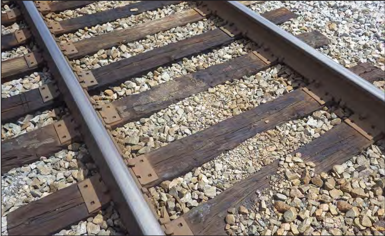
Figure 248. 091-5098, view of track.
