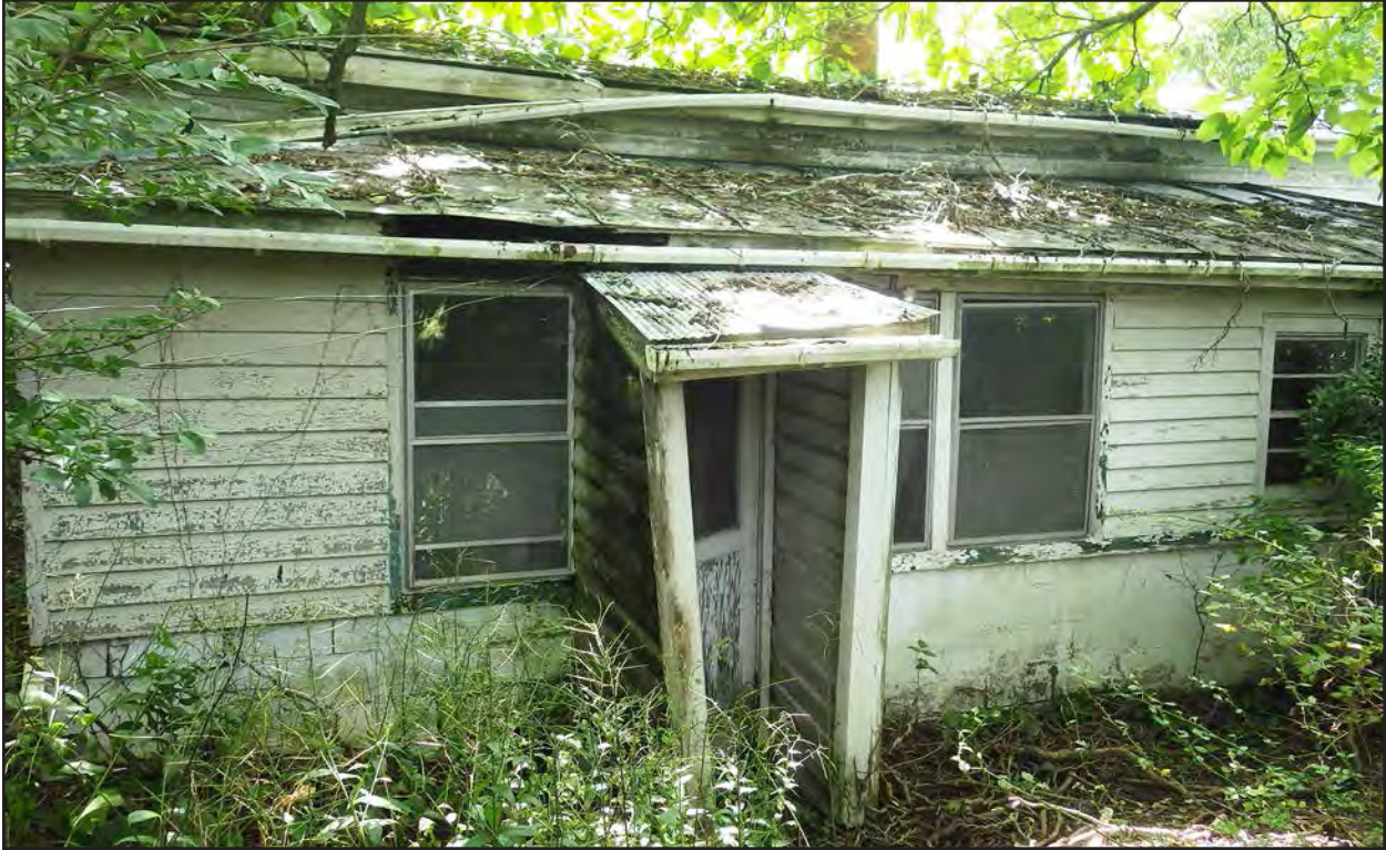
Figure 97. 007-5692, rear shed addition, facing south.
