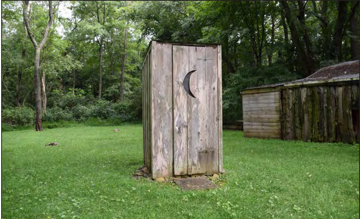
Figure 22. 007-0455, outhouse, facing west.
