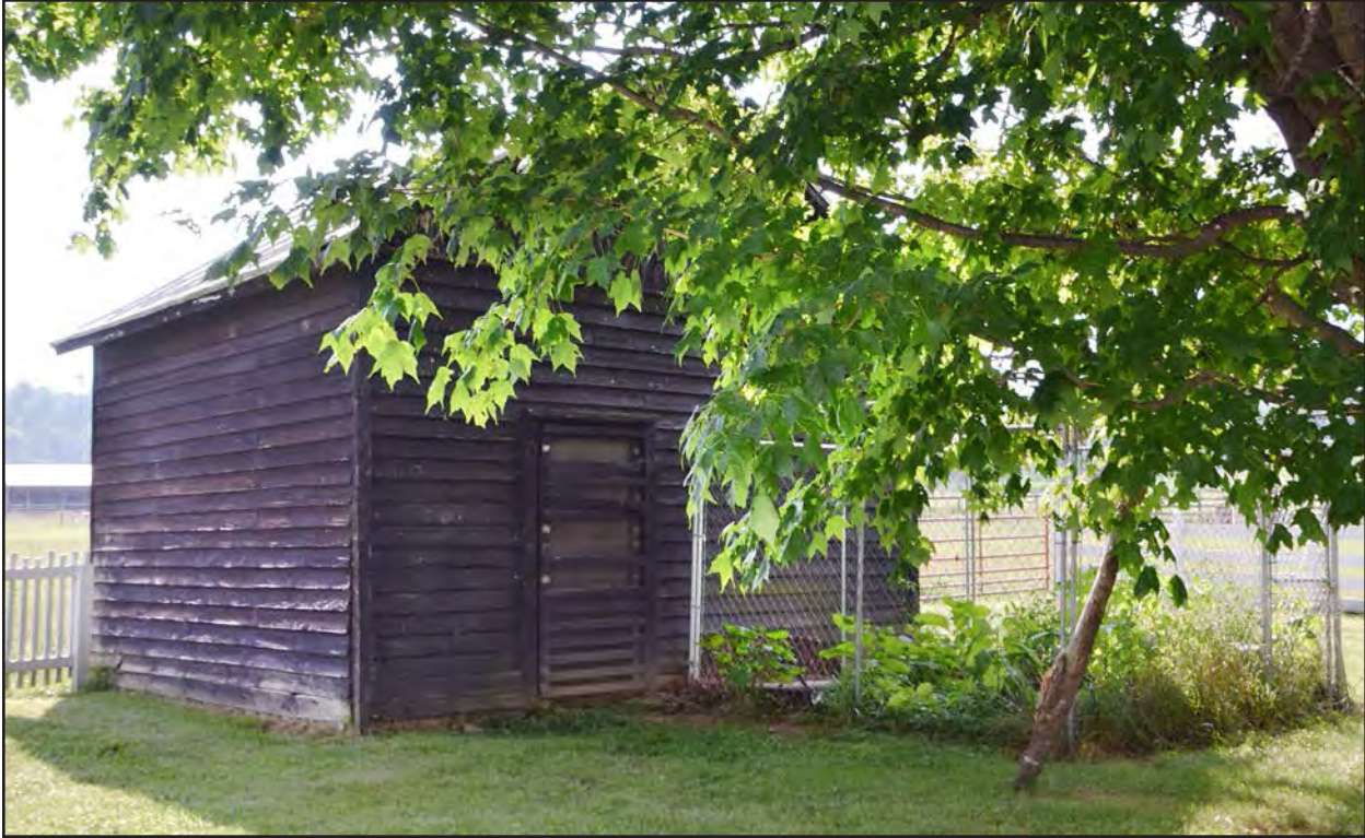
Figure 7. 007-0103, shed, facing northwest.
