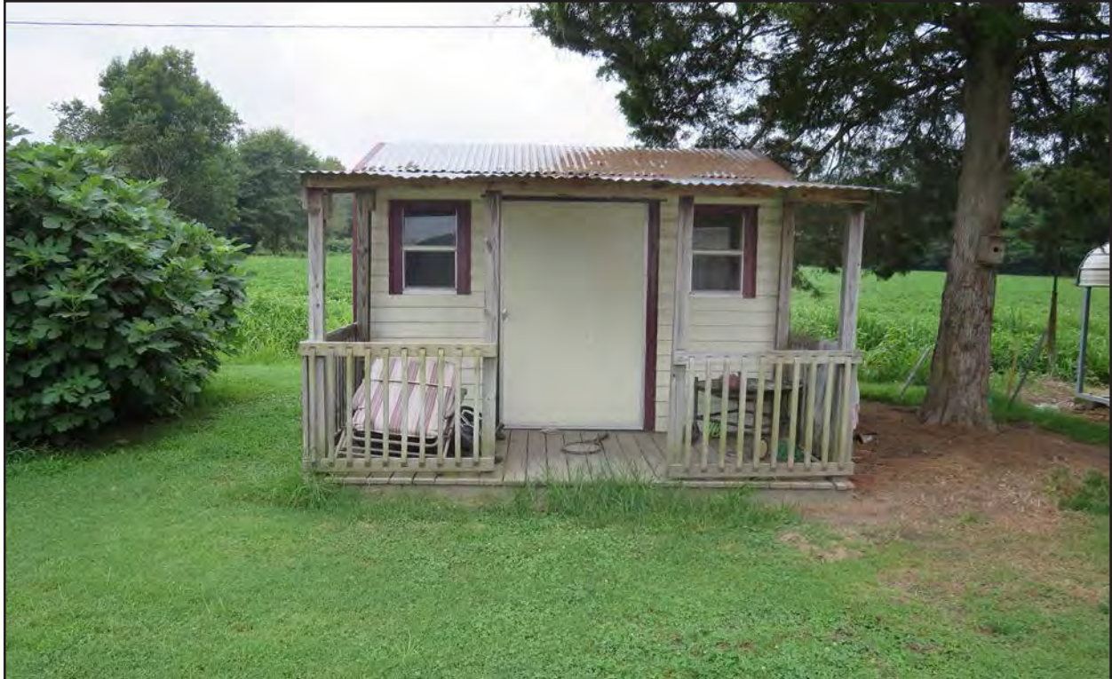
Figure 274. 133-5571, shed 1, facing west.
