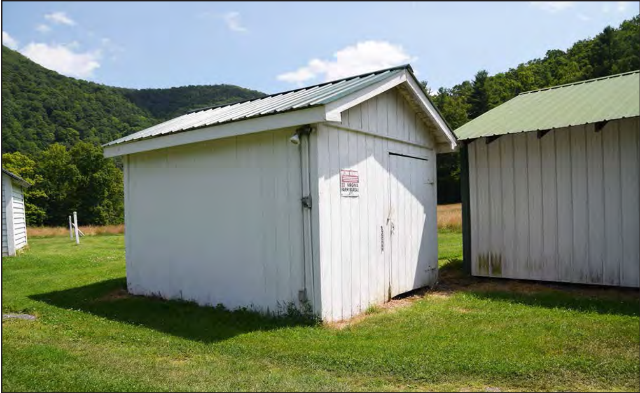
Figure 204. 045-5081, shed 2, facing south.
