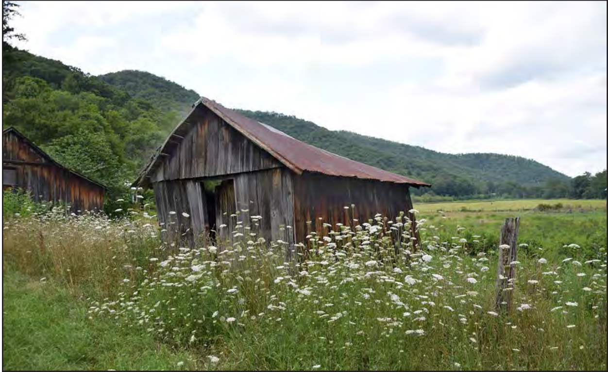
Figure 211. 045-5082, shed facing north.
