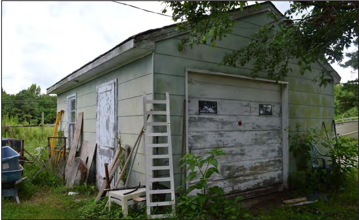
Figure 255. 133-5444, garage, facing southeast.
