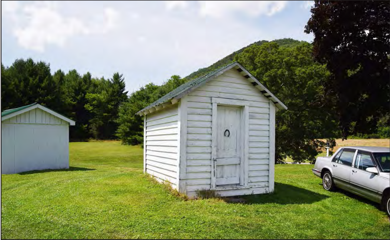
Figure 203. 045-5081, shed 1, facing northwest.
