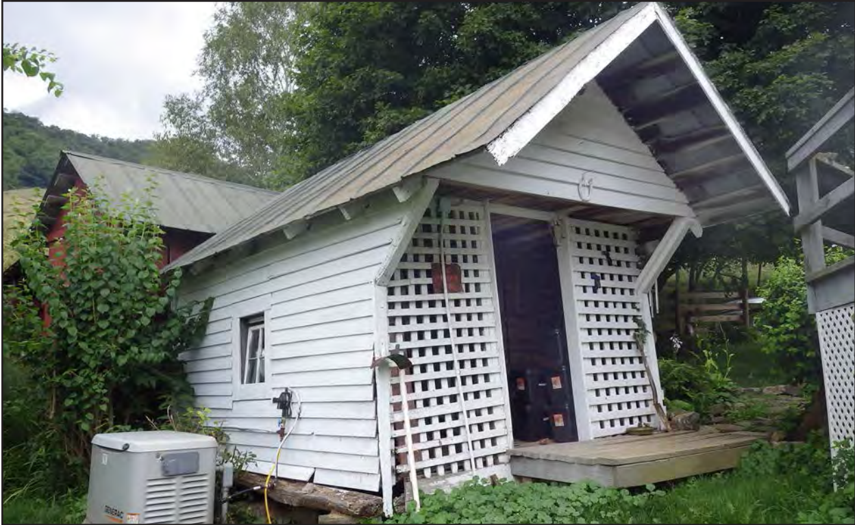
Figure 180. 045-0055, shed 1, facing north.
