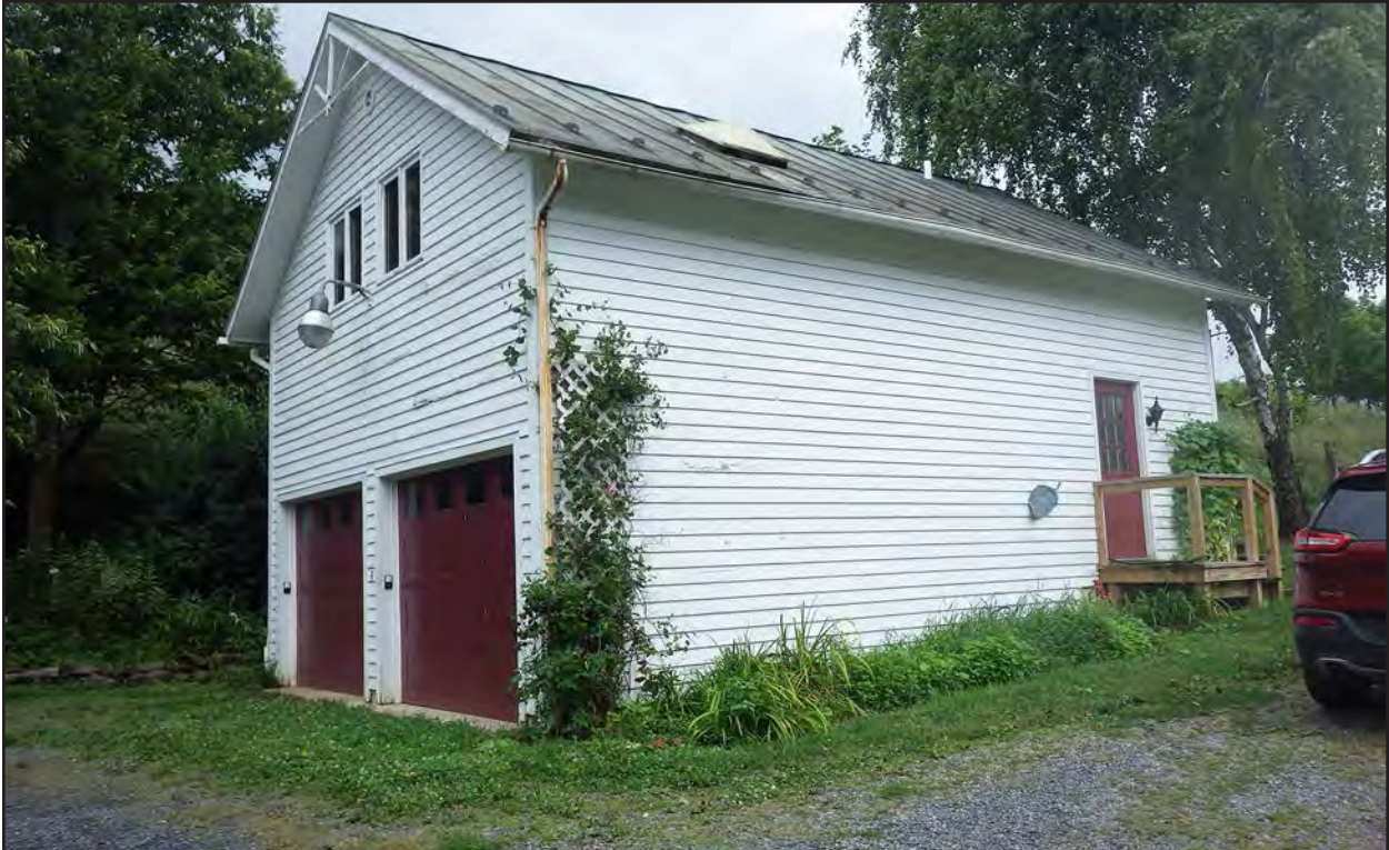
Figure 178. 045-0055, garage, facing north.
