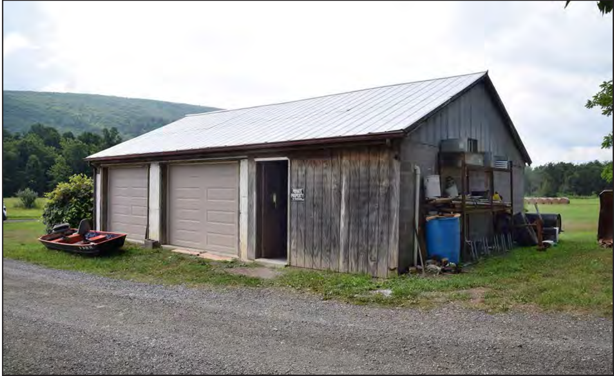
Figure 51. 007-5682, storage building, facing south.
