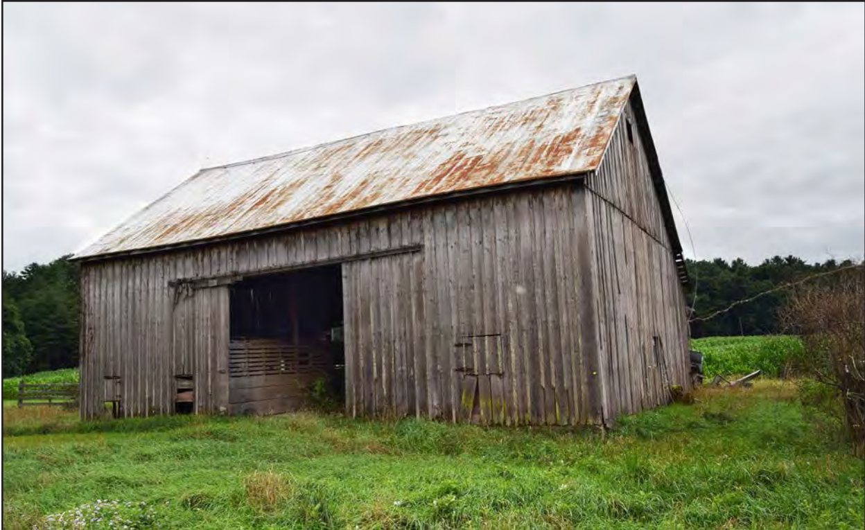
Figure 30. 007-0457, barn 1, facing southeast.
