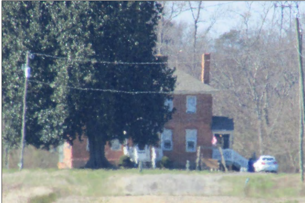
Photo 3: House at 203 Upton Lane (133-0025), North Elevation.
