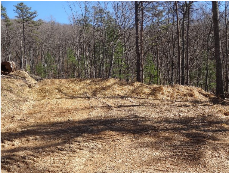
Tank trap at start of Temporary Road
