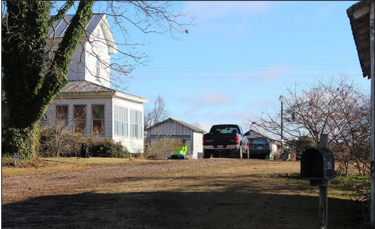
Photo 30. HX0227, rear accessory structure, facing east.
