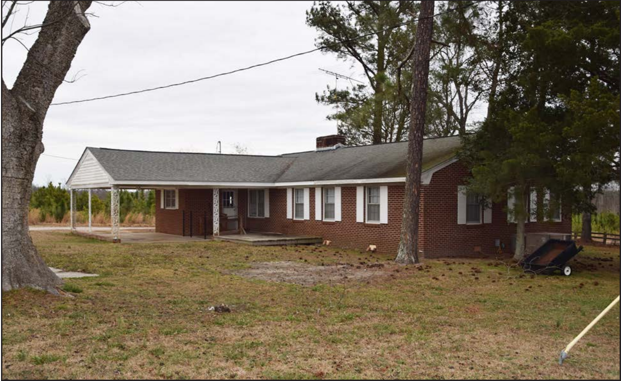
Photo 45. HX1581, facing northeast.
