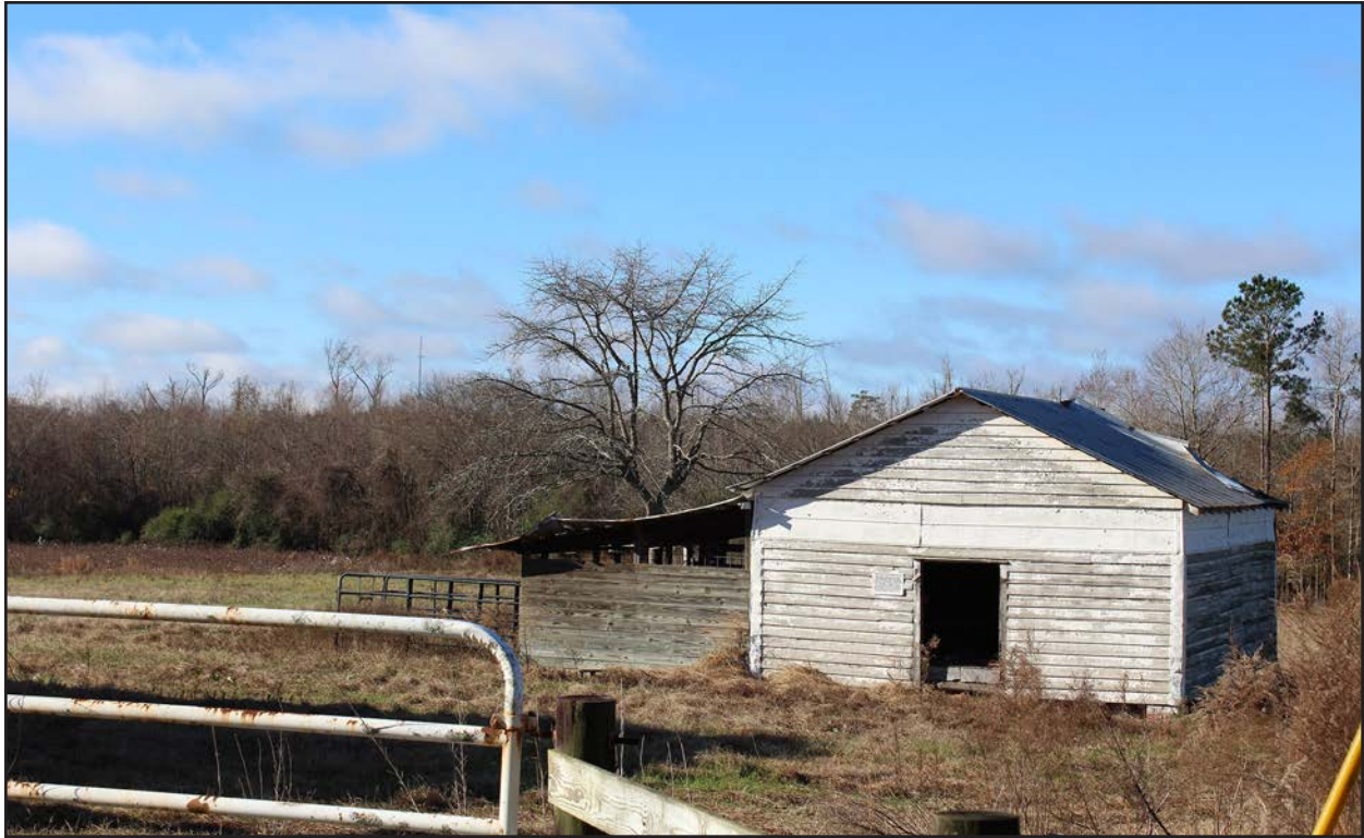
Photo 37. HX0229, facing southwest.
