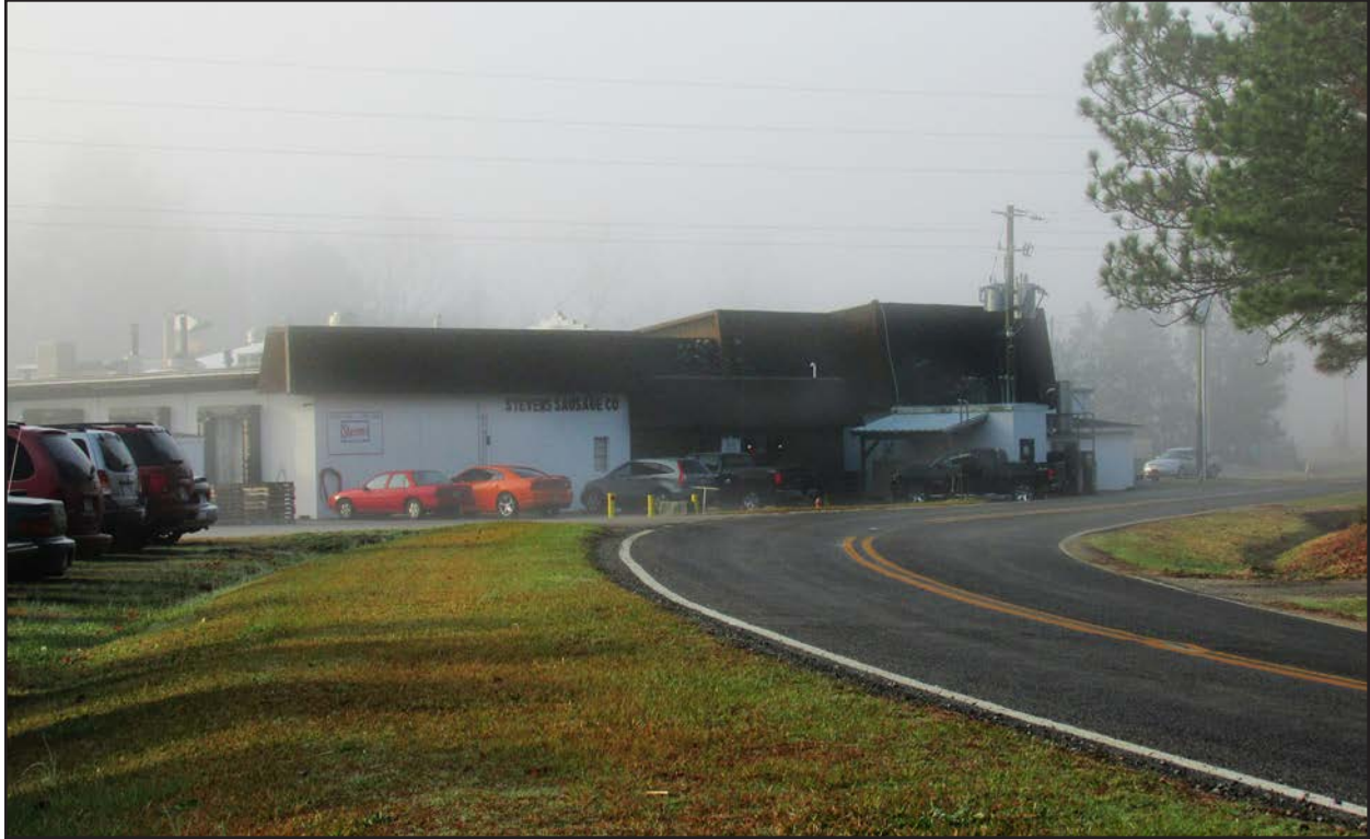
Photo 95. JT1921 (Stevens Sausage Company plant), facing south.
