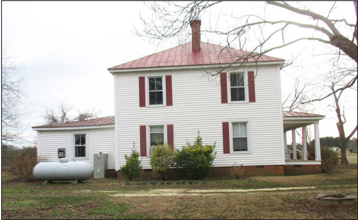
Photo 127. NS0650, house, facing south.
