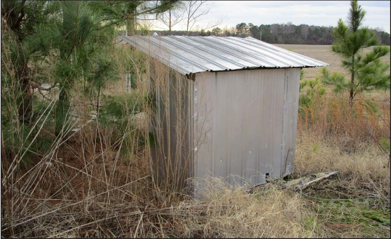
Photo 157. NS1508, small shed, facing southeast.
