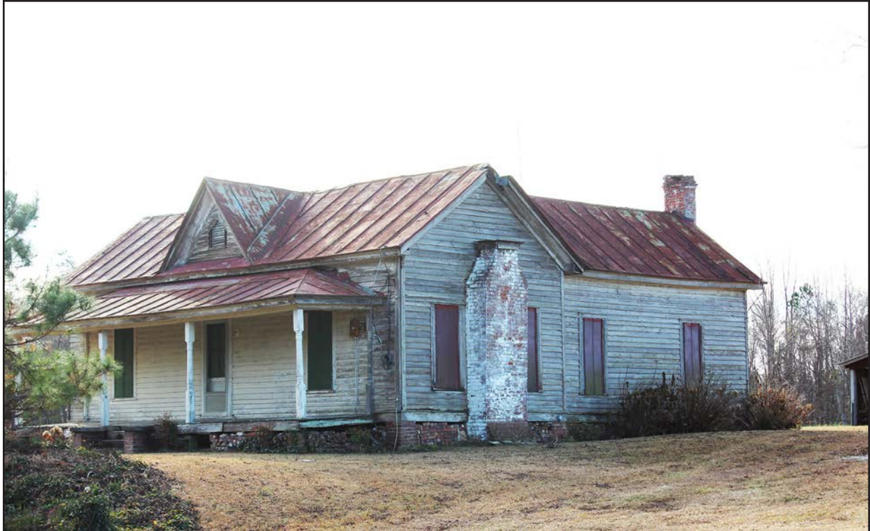
Photo 180. WL2012, facing southwest.
