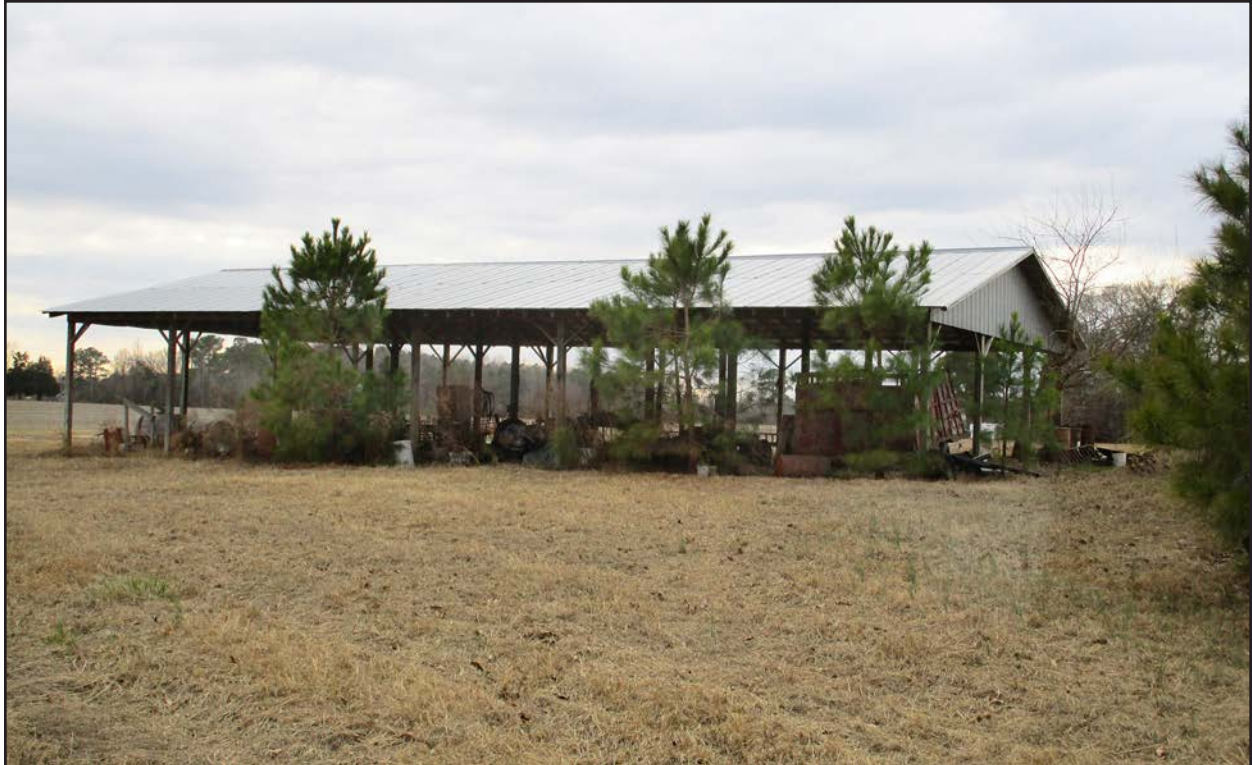
Photo 160. NS1508, pole shed, facing southwest.
