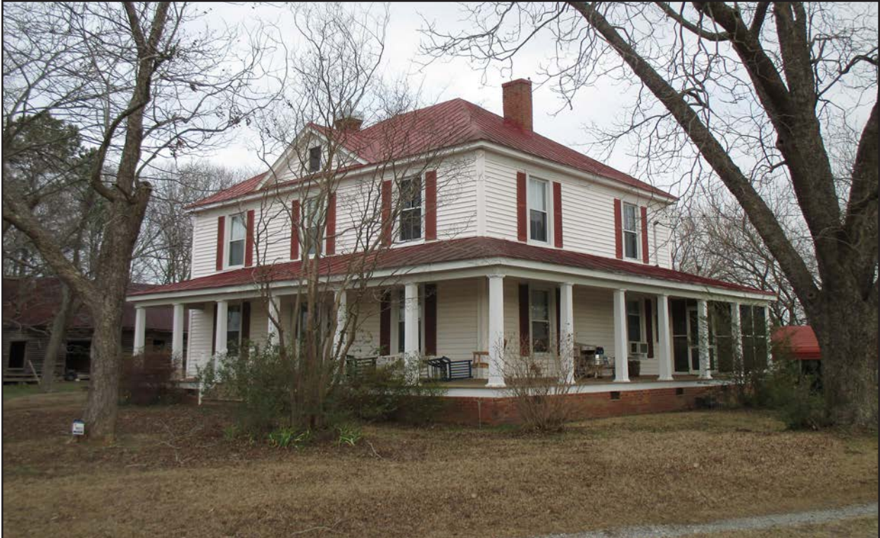
Photo 124. NS0650, house, facing northeast.
