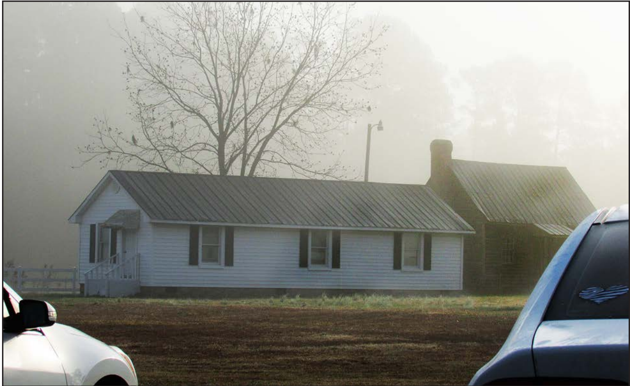
Photo 93. JT1920, accessory structure 2, facing southeast.
