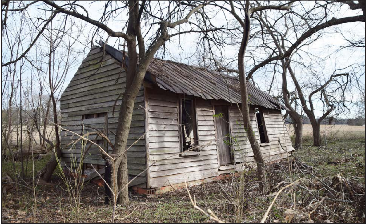
Photo 135. NS0650 summer kitchen, facing northeast.
