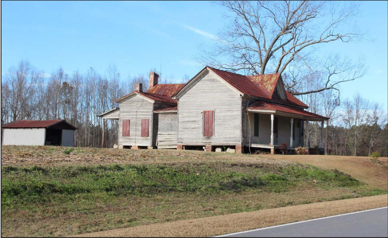
Photo 181. WL2012, facing north-northwest.
