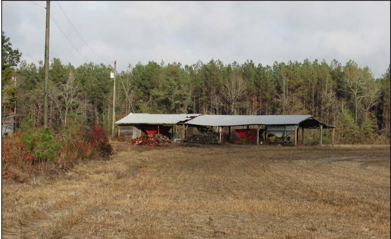
Photo 168. RB0678, pole shelters, facing northeast.
