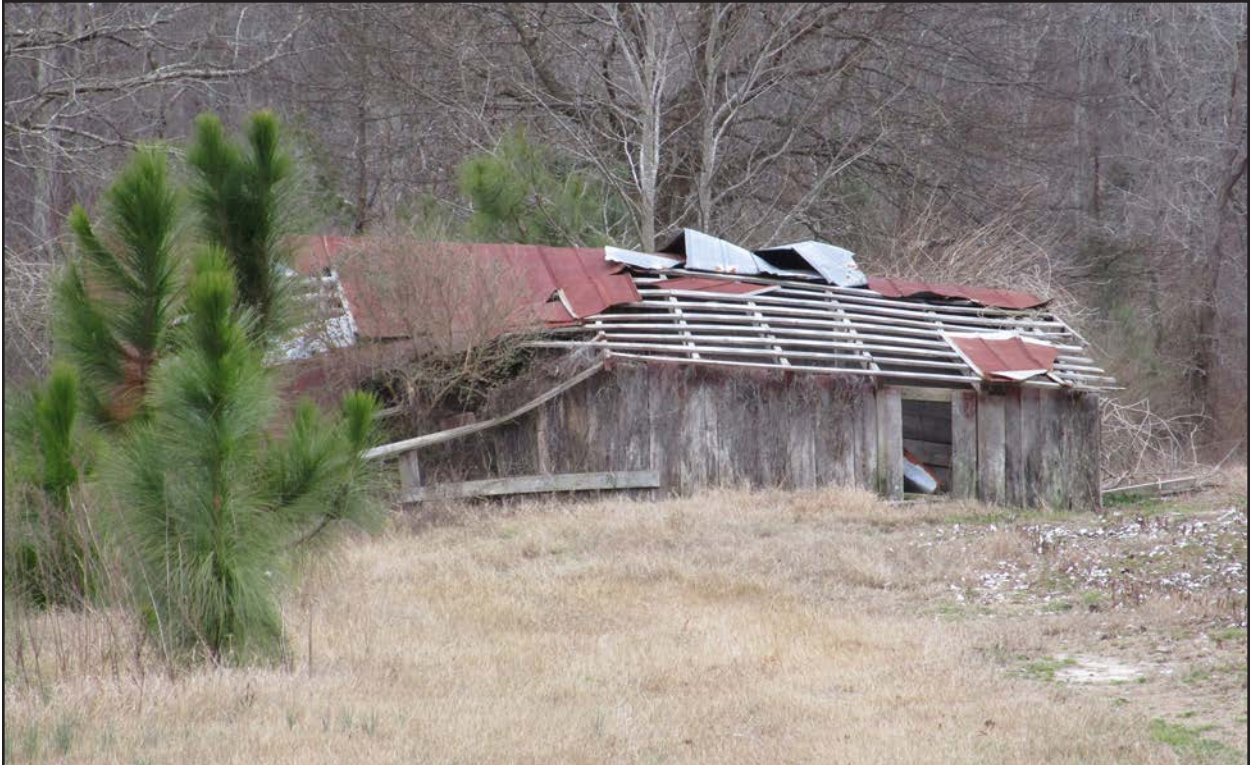
Photo 52. HX1581, storage structure, facing south.
