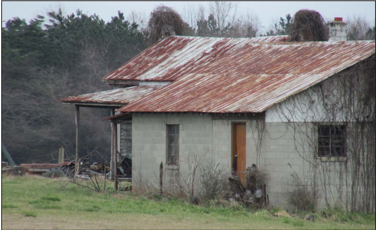
Photo 149. NS1504, facing northeast.
