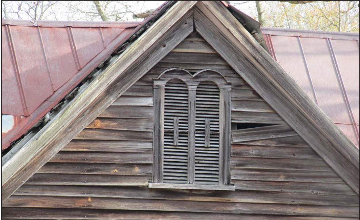
Photo 114. JT1937, vent details, facing east.
