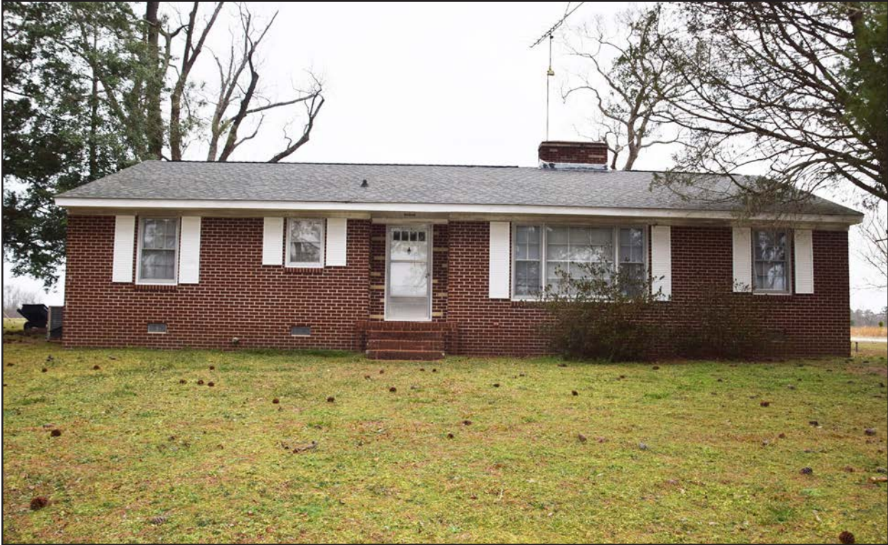
Photo 44. HX1581, facing north-northwest.
