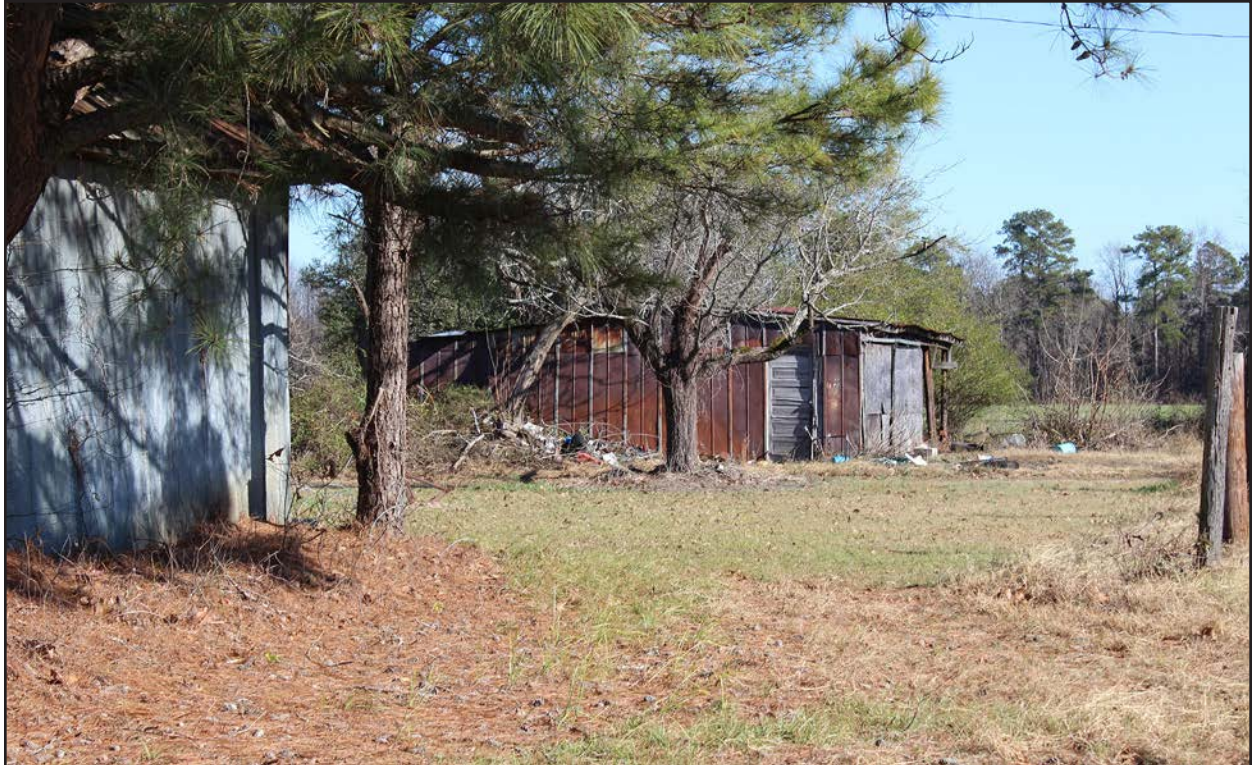
Photo 70. JT0957, gabled accessory structure 3, facing east.
