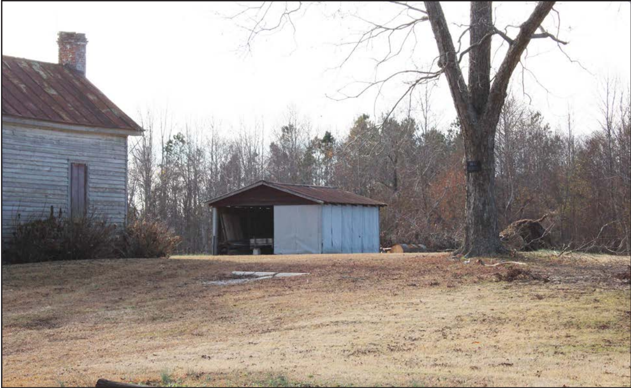
Photo 182. WL2012, outbuilding, facing southwest.
