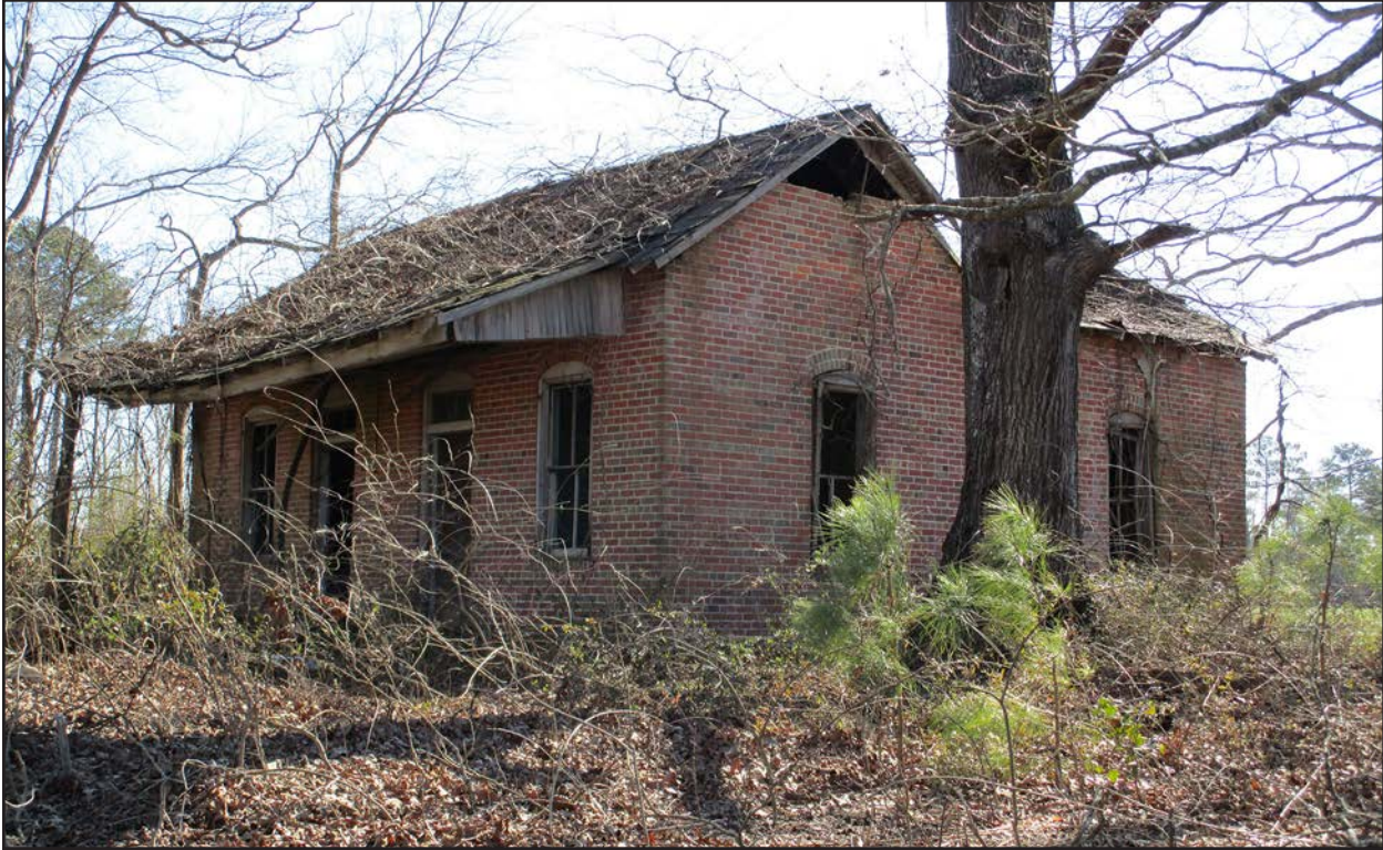
Photo 39. HX0354, facing south.
