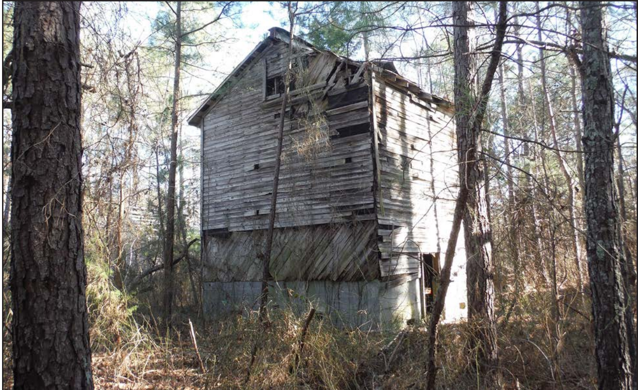
Photo 60. HX1597, tobacco barn 2, facing northeast.
