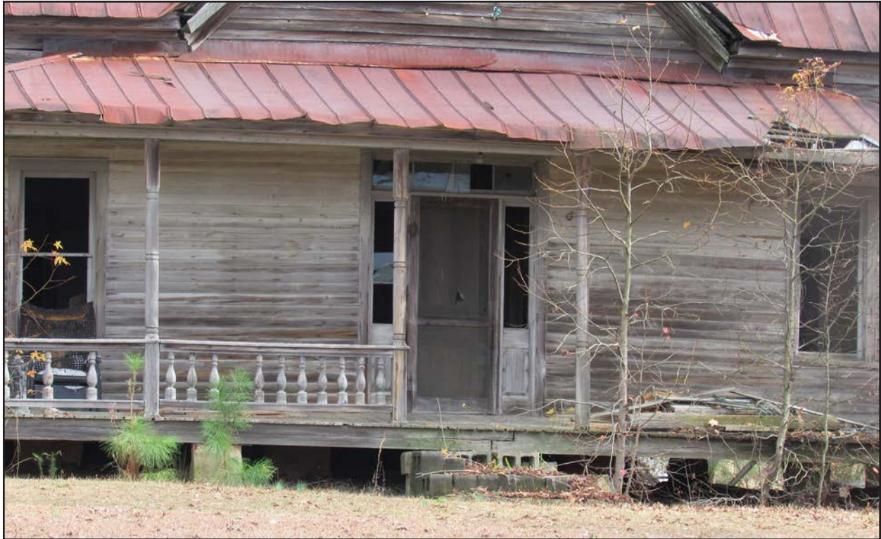
Photo 115. JT1937, main entrance facing east.
