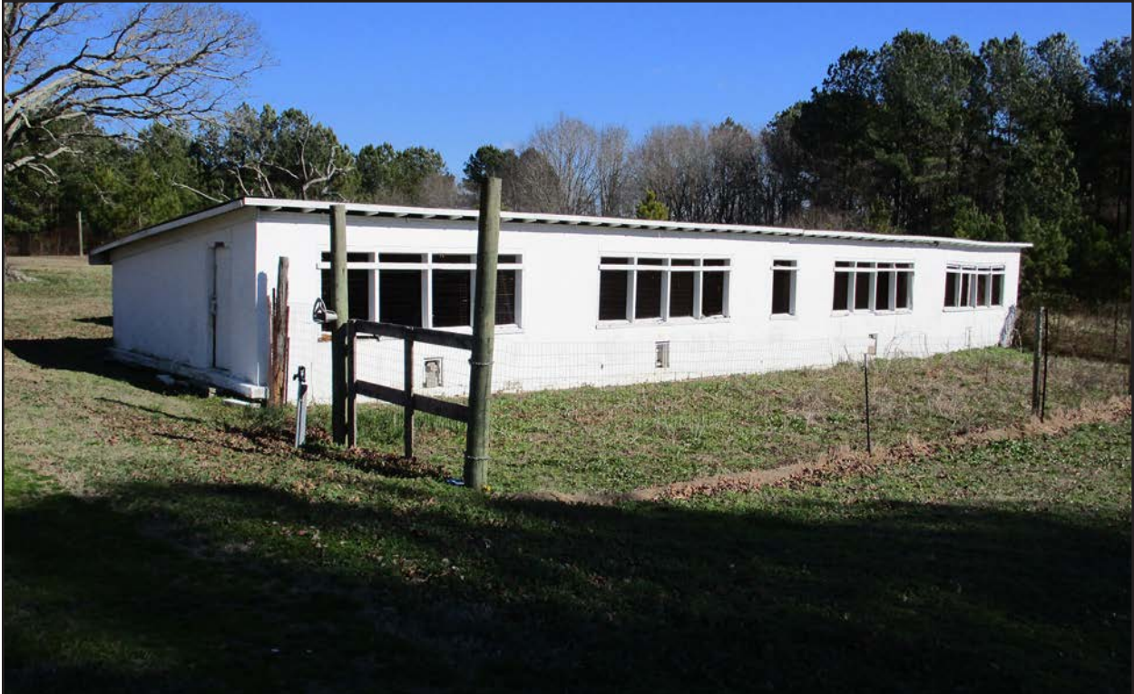
Photo 16. HX0021, chicken house, facing east.
