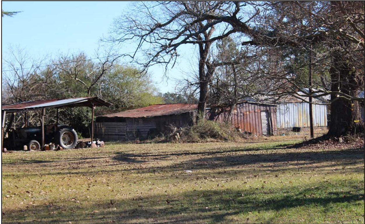
Photo 69. JT0957, gabled accessory structure 3, facing southeast.
