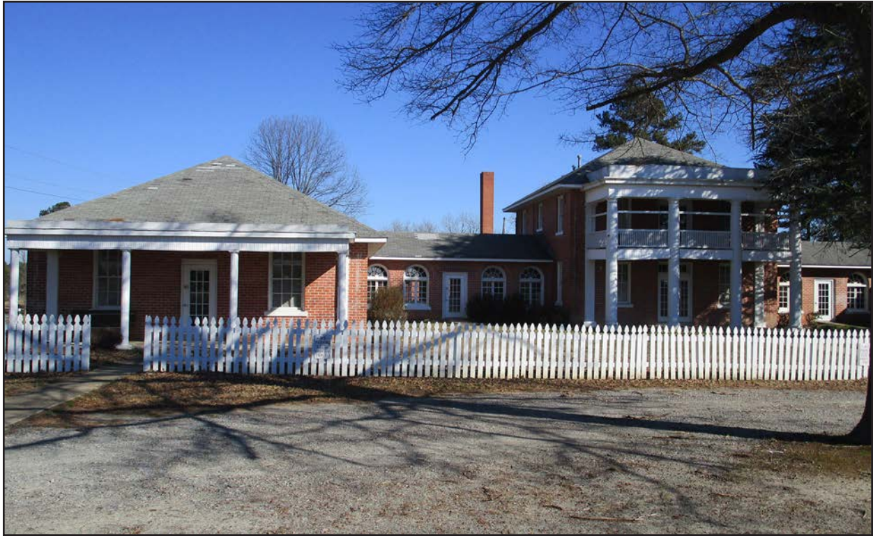
Photo 7. HX0021, facing northeast.
