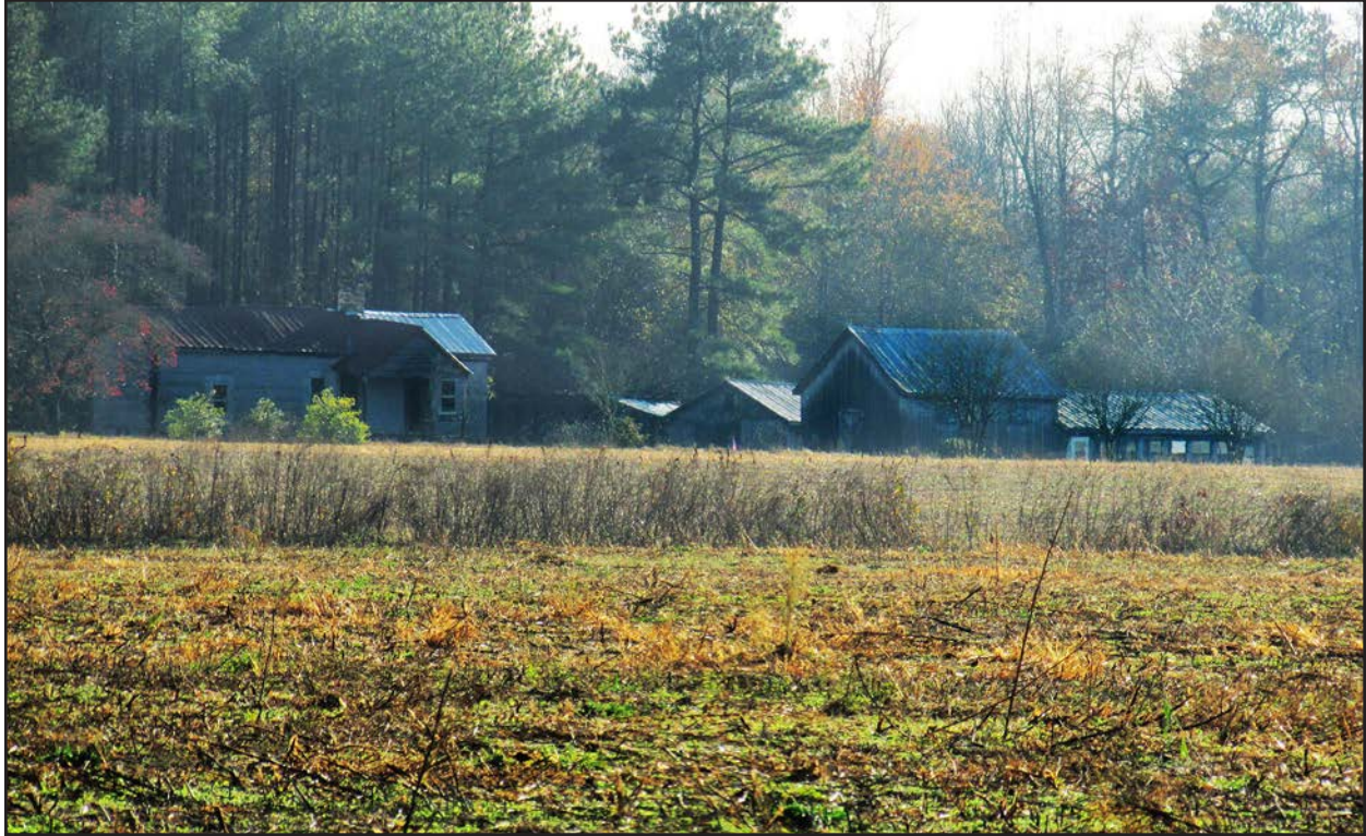
Photo 173. RB0680, agricultural outbuildings, facing south.
