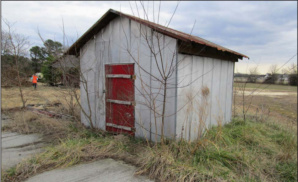
Photo 158. NS1508, ca. 1960 structure, facing southwest.
