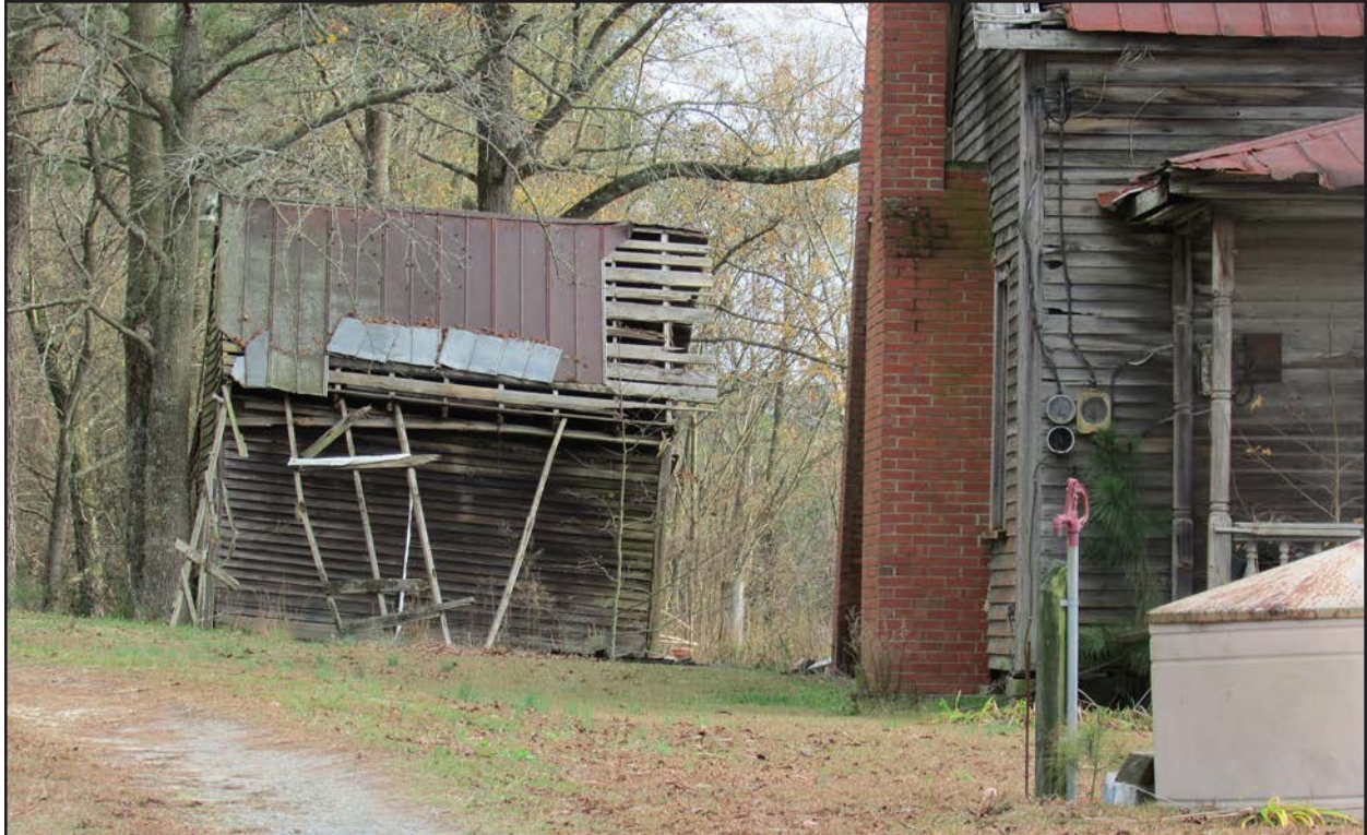
Photo 116. JT1937, accessory structure facing east.
