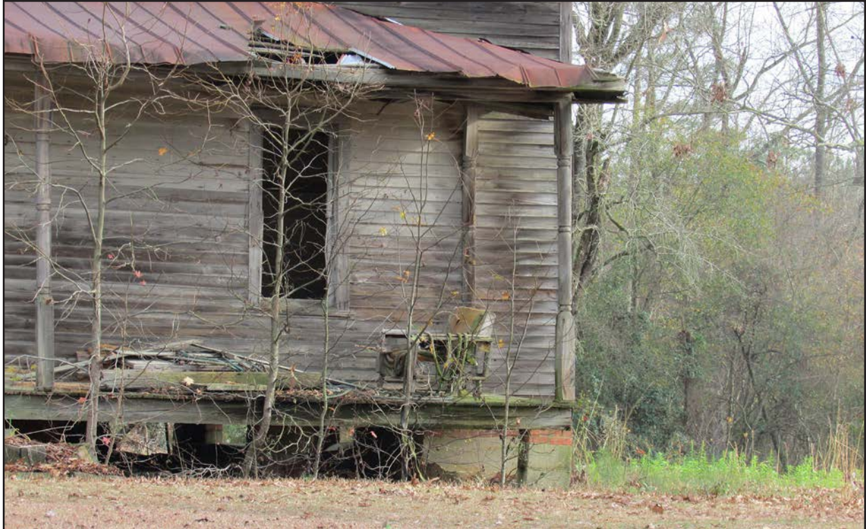
Photo 112. JT1937, foundation, facing southeast.
