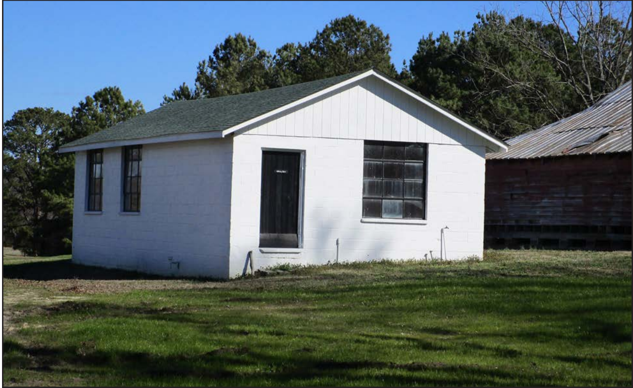
Photo 13. HX0021, milking barn, facing northeast.
