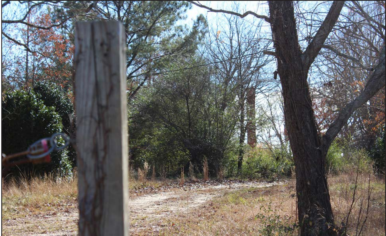
Photo 88. JT1919, free-standing chimney, facing south.
