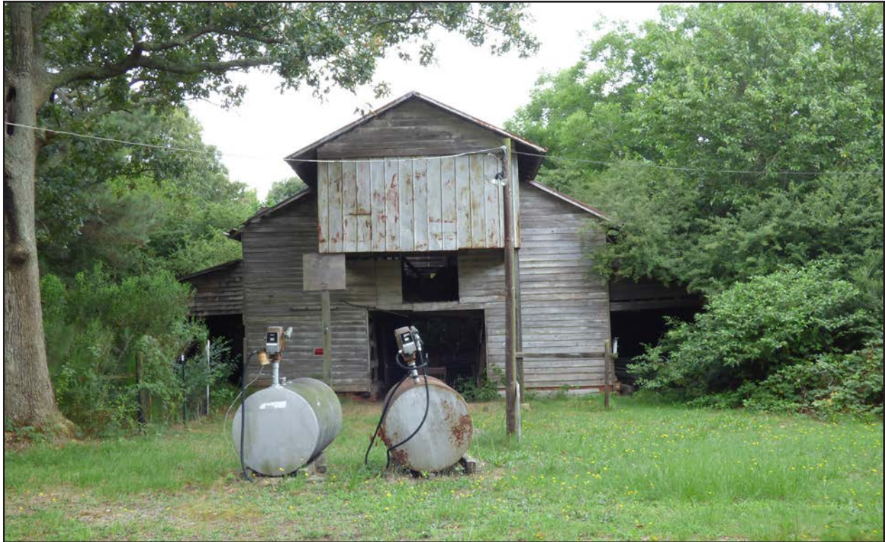
Photo 139. NS1493, hay barn, facing west.
