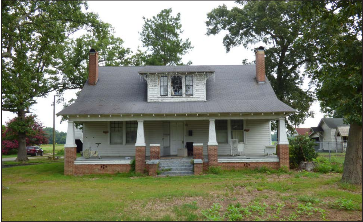
Photo 137. NS1493, dwelling, facing north.
