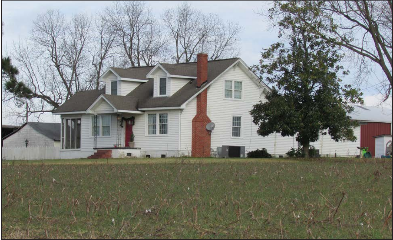
Photo 53. HX1583, facing northeast.
