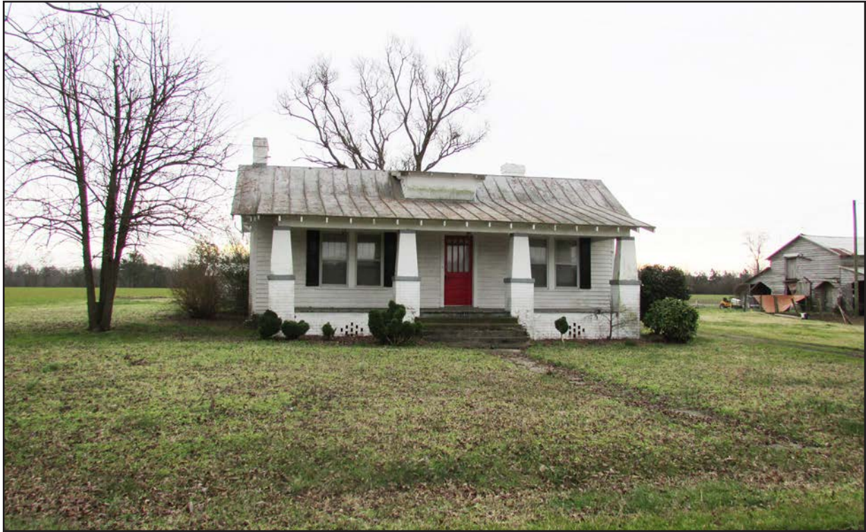
Photo 161. NS1517, dwelling, facing south-southeast.
