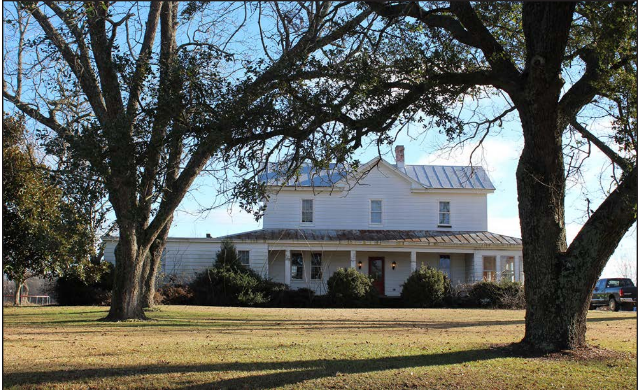
Photo 26. HX0227, main house, facing east.
