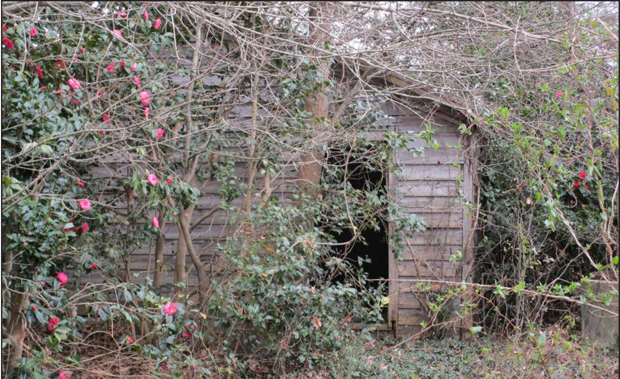
Photo 110. JT1935 accessory structure 2, facing south.
