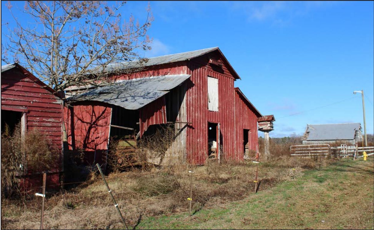
Photo 36. HX0229, facing north-northwest.
