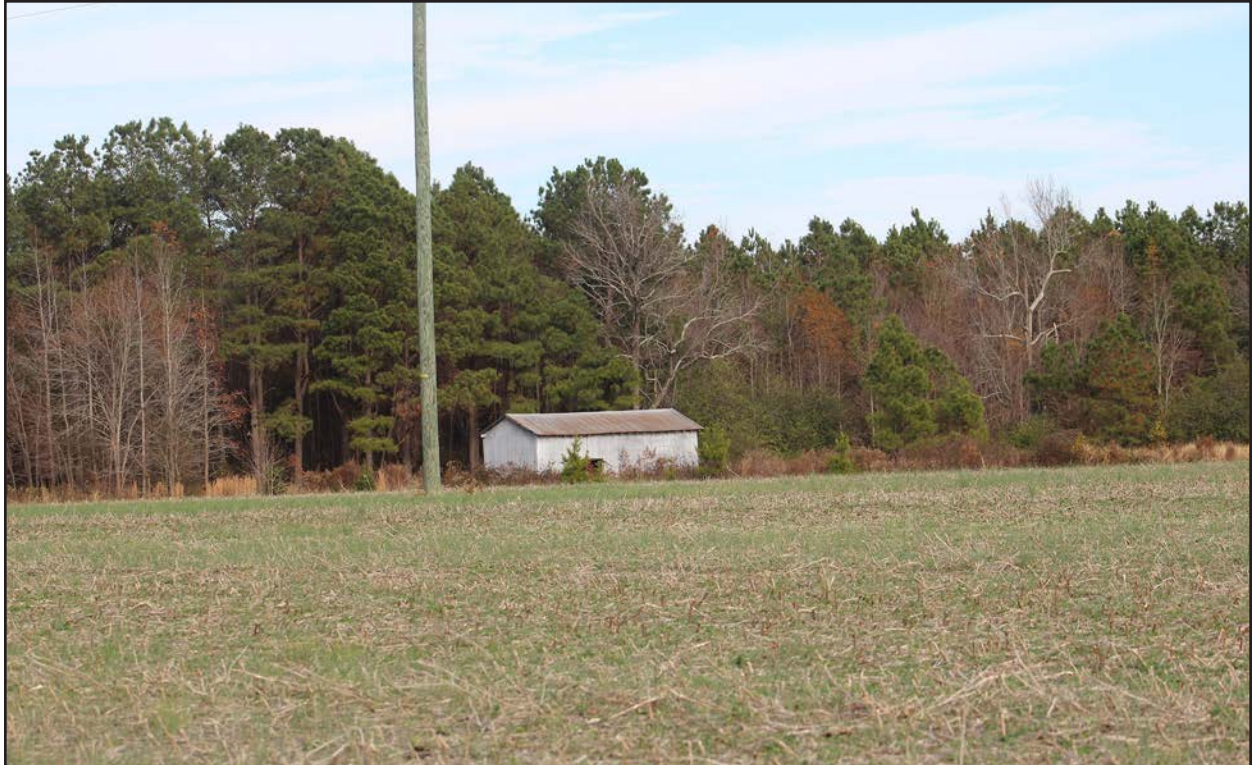
Photo 86. JT1913, storage structure, facing northeast.
