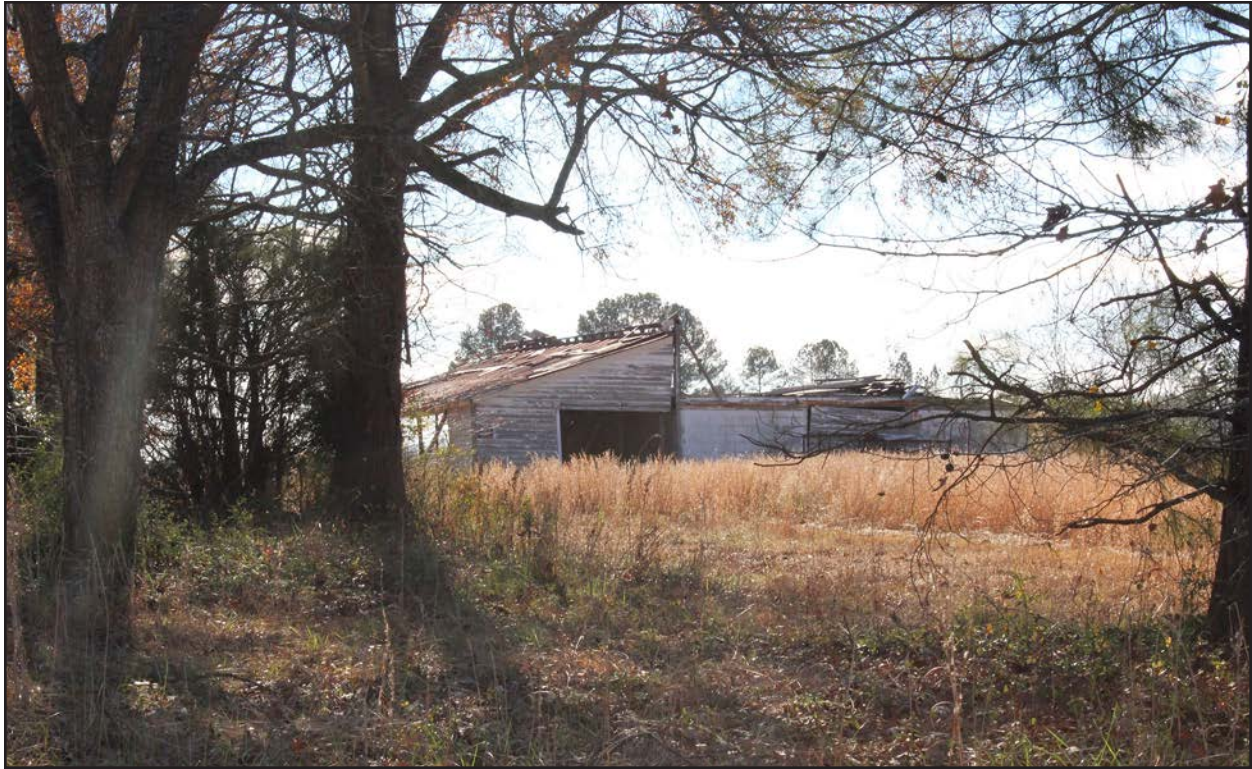
Photo 89. JT1919, accessory structure, facing south-southeast.
