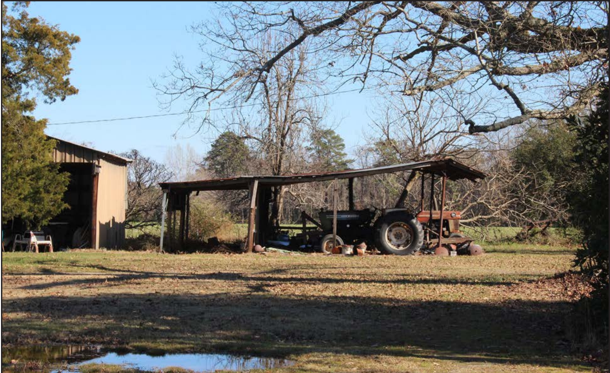
Photo 68. JT0957, pole shelter, facing east.
