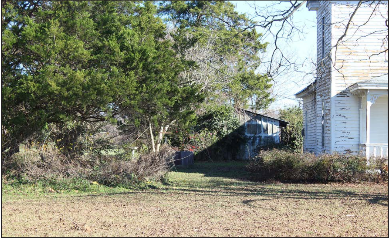
Photo 65. JT0957, gabled accessory structure 1, facing east.
