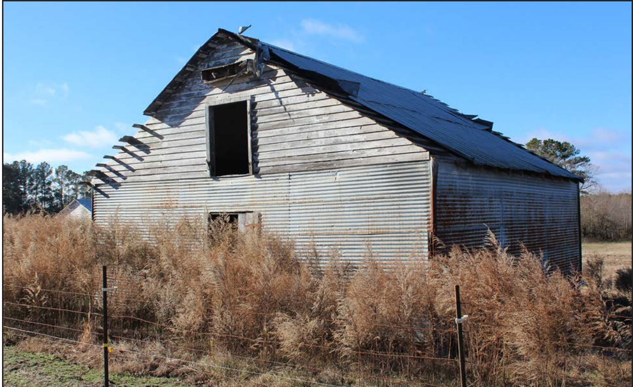
Photo 38. HX0229, facing southwest.
