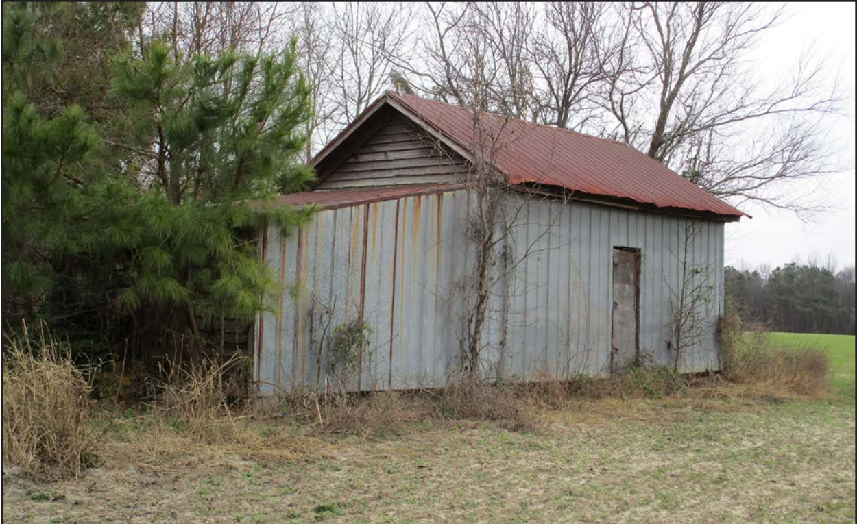
Photo 106. JT1935 accessory structure 1, facing southeast.
