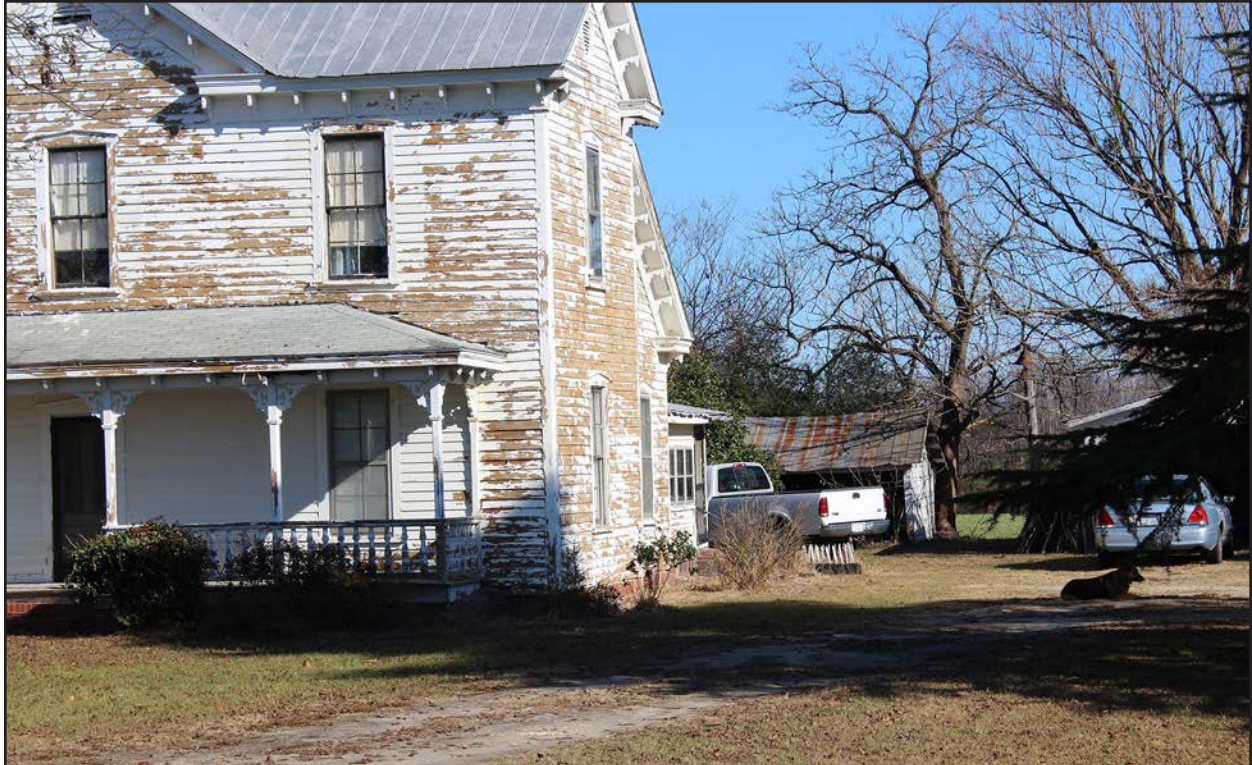
Photo 66. JT0957, gabled accessory structure 2, facing east-northeast.
