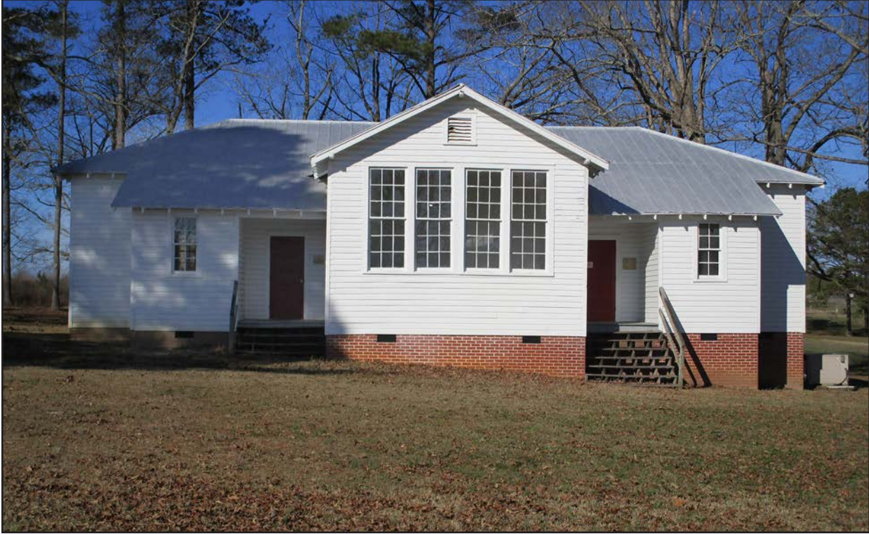
Photo 42. HX1566 (Allen Grove Rosenwald School), facing northwest.
