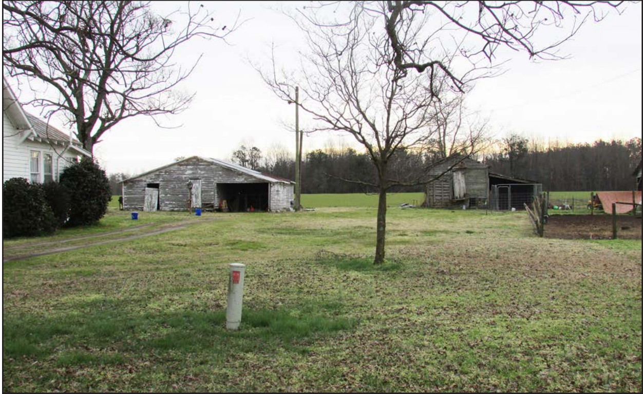
Photo 163. NS1517, outbuildings, facing southeast.
