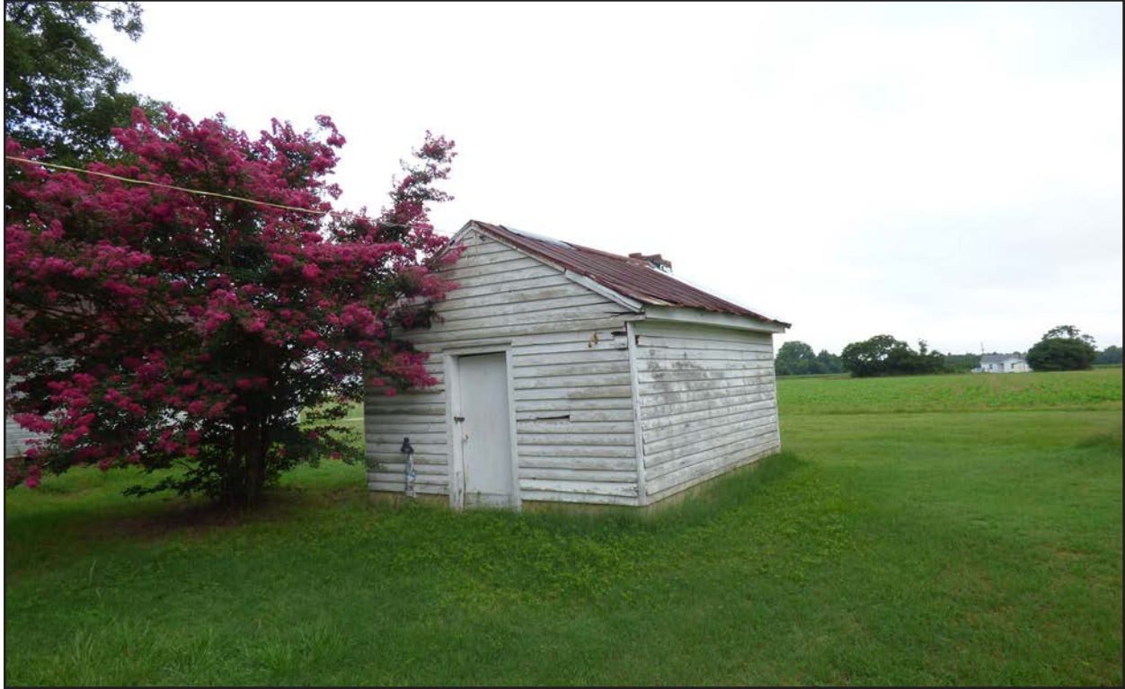
Photo 141. NS1493, agricultural outbuilding, facing northwest.
