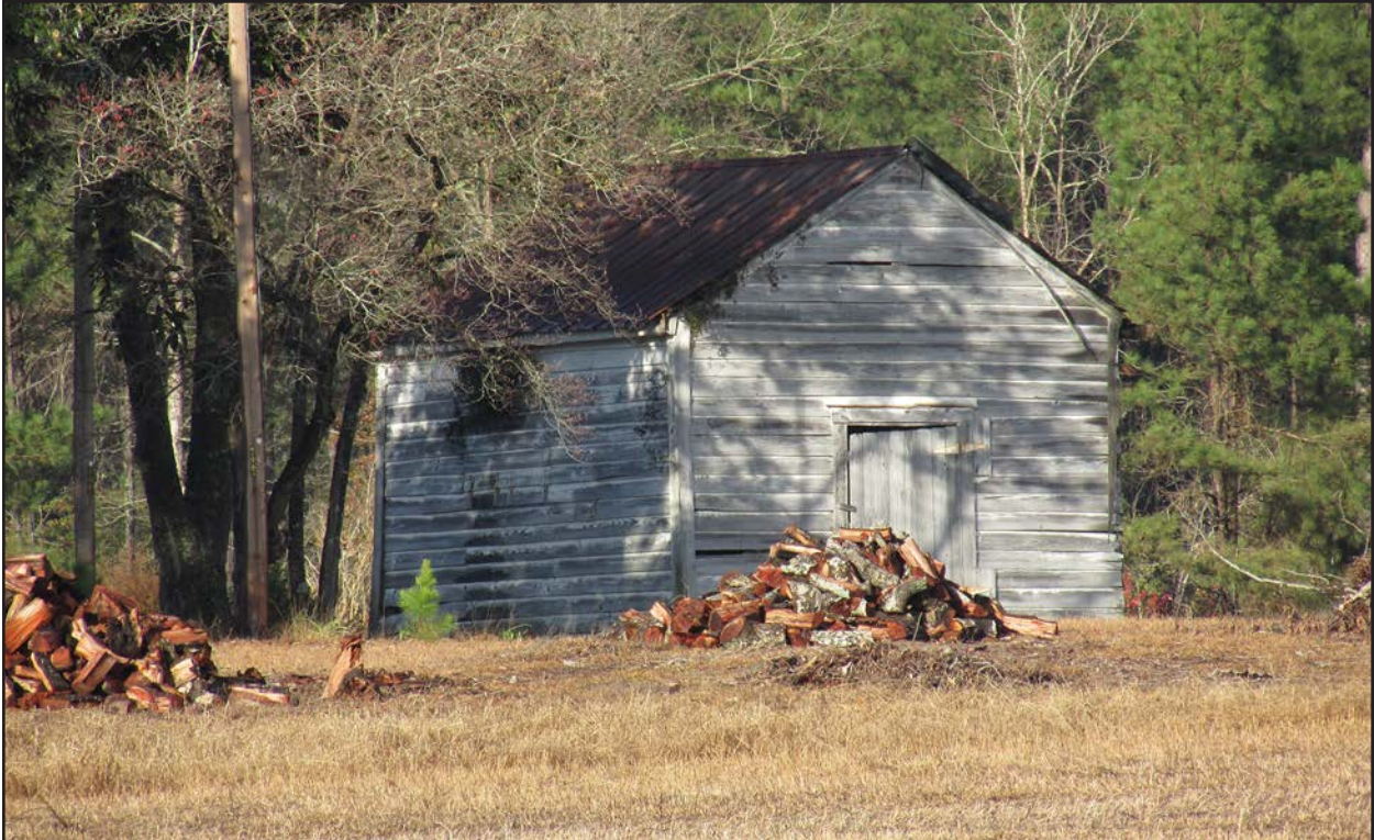
Photo 166. RB0678, shed, facing north.
