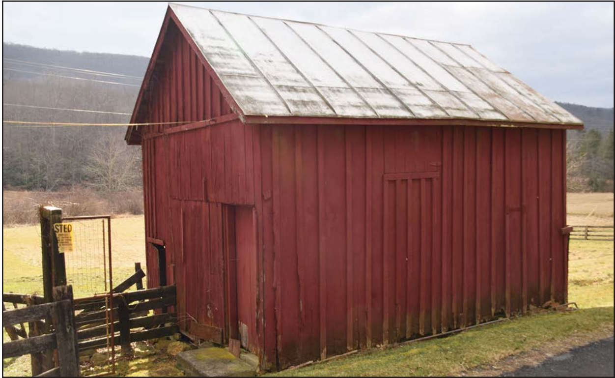
Figure 49. 008-5068, small livestock barn, facing southeast.
