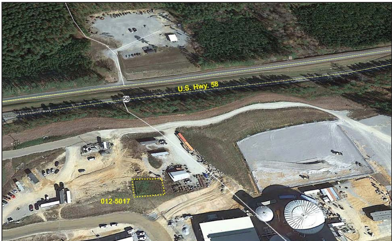
Figure 54. 012-5017, aerial view showing cemetery.
