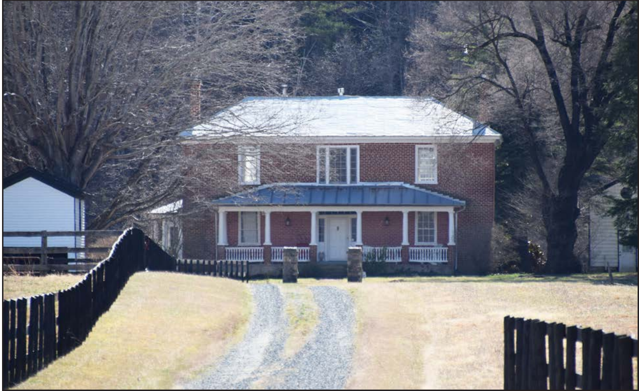
Figure 81. 062-5119-0113, house, facing south.
