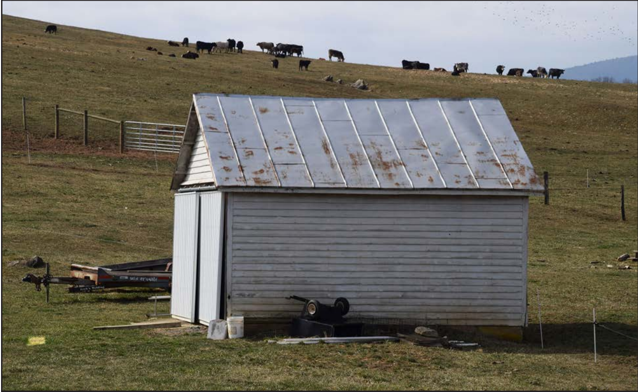
Figure 5. 007-0272, garage, facing northwest.
