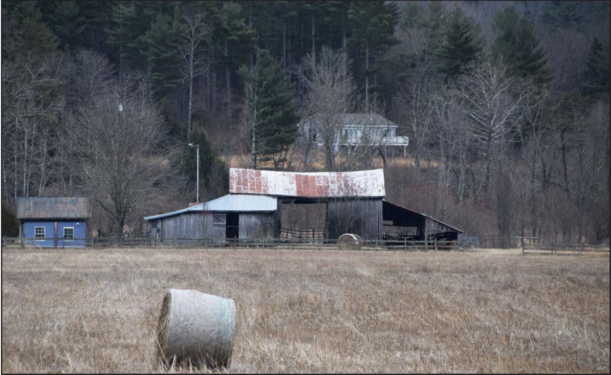
Figure 37. 007-5743, barn and shed, facing south.
