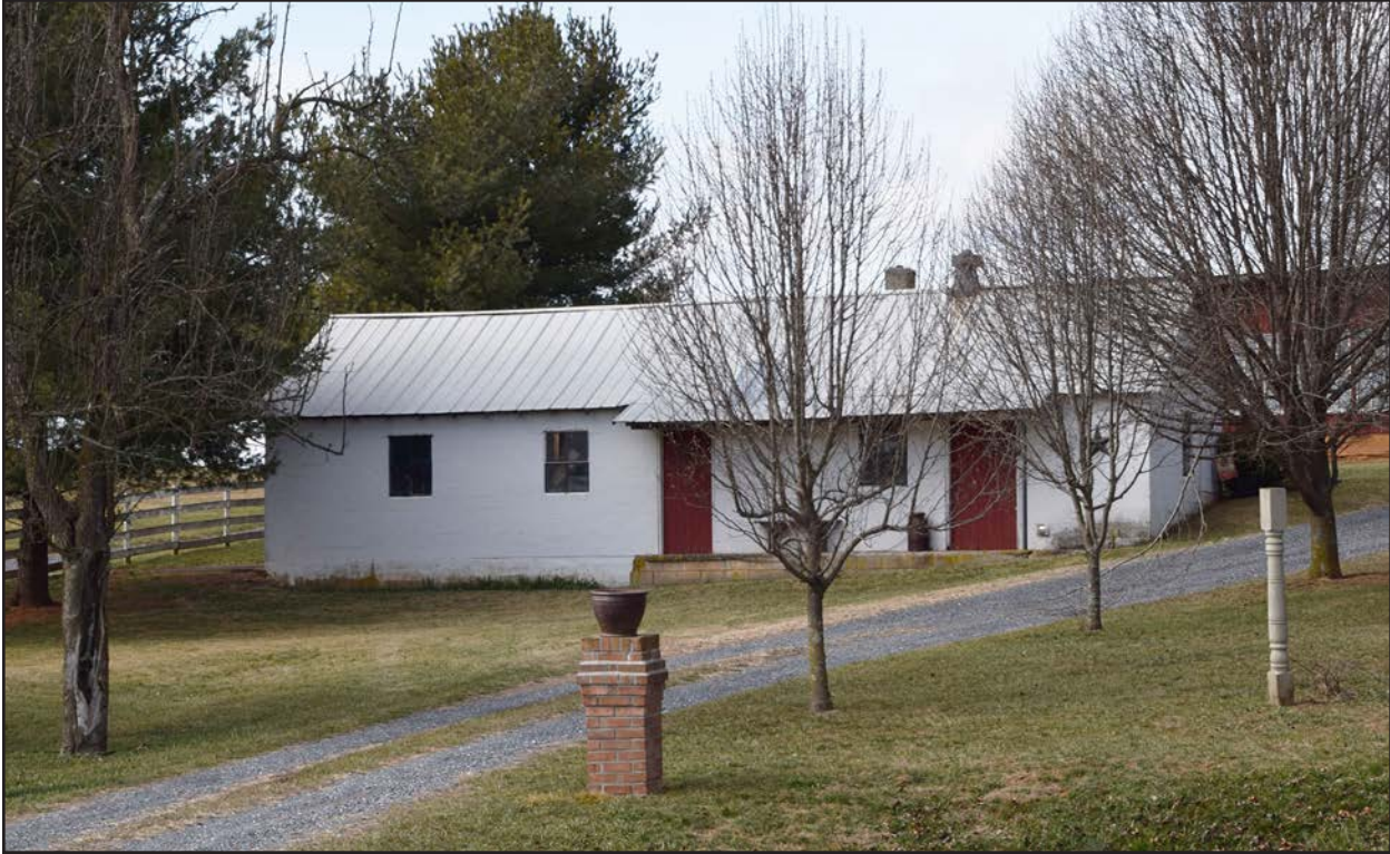
Figure 25. 007-5584, concrete block building detail, facing northwest.
