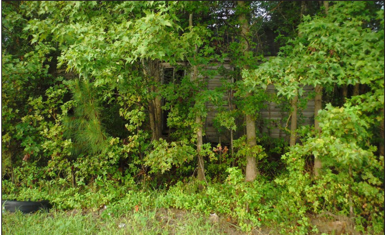
Figure 100. 133-5481, deteriorated structure, facing southwest.
