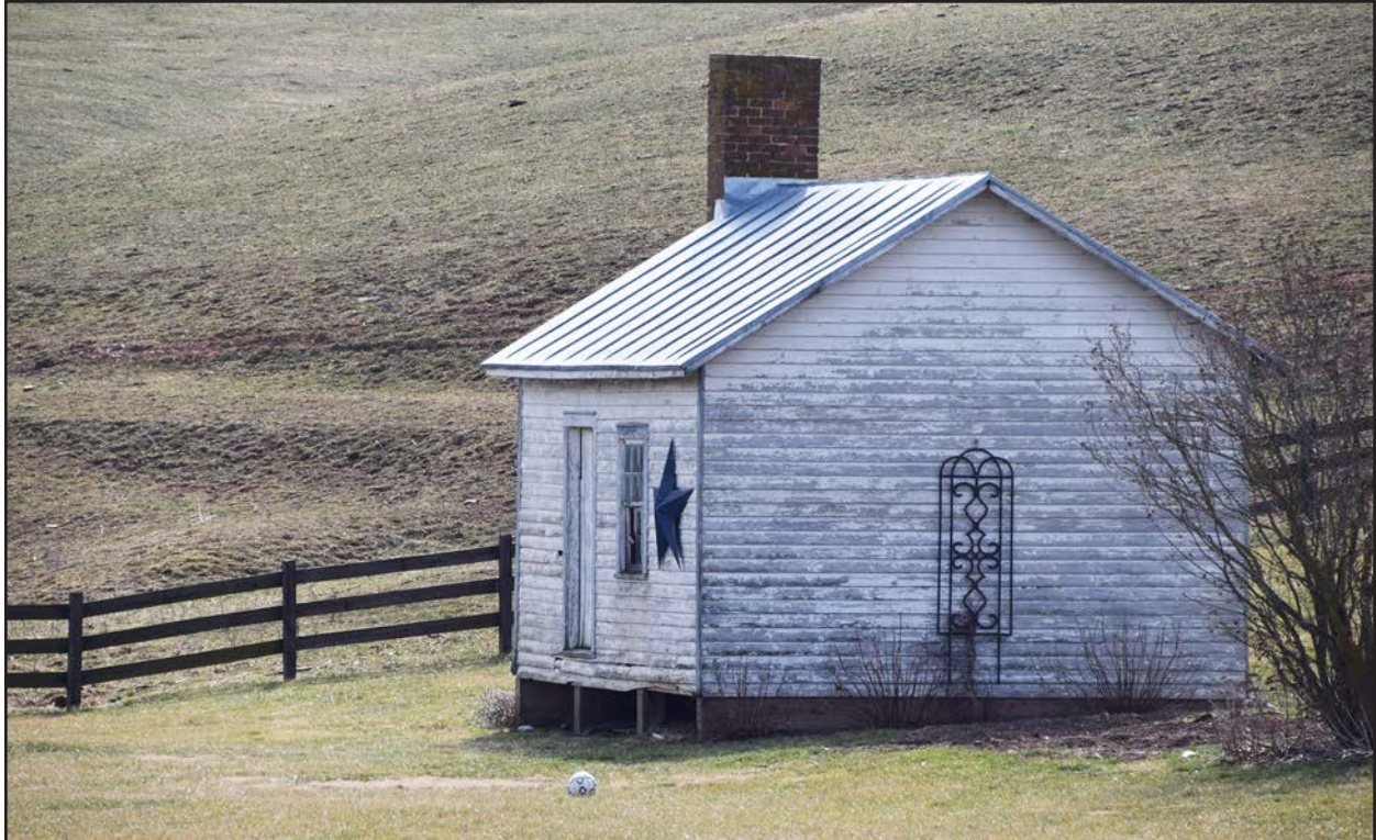
Figure 4. 007-0272, wash house, facing southwest.
