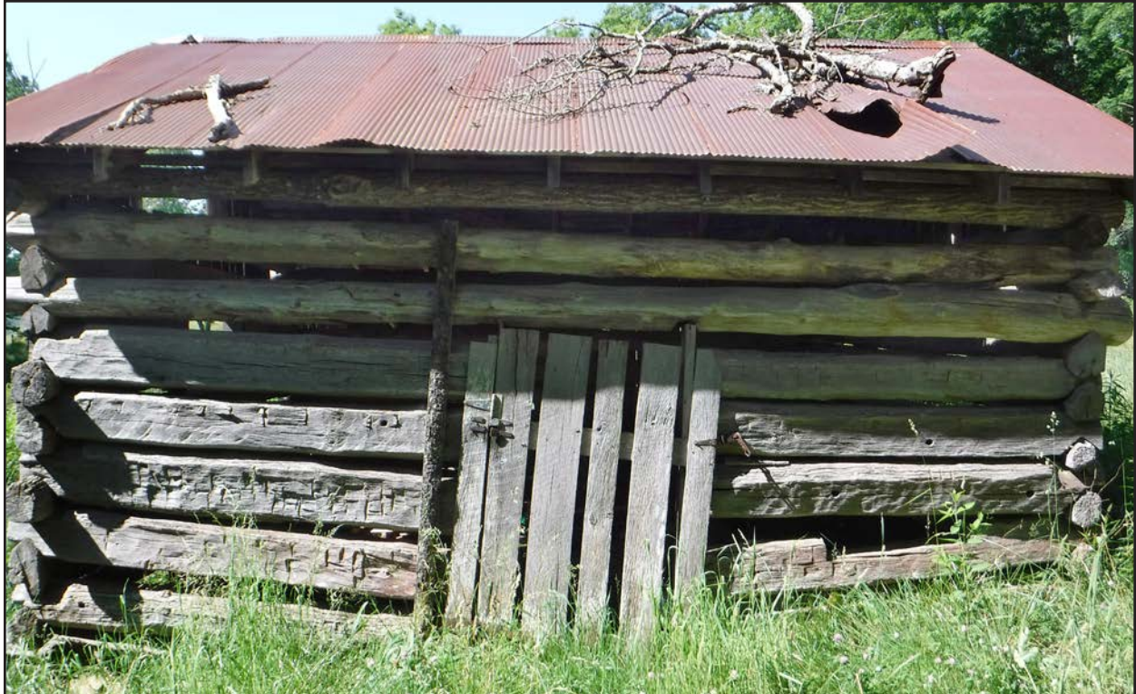
Figure 78. 045-5090, log structure, facing south.
