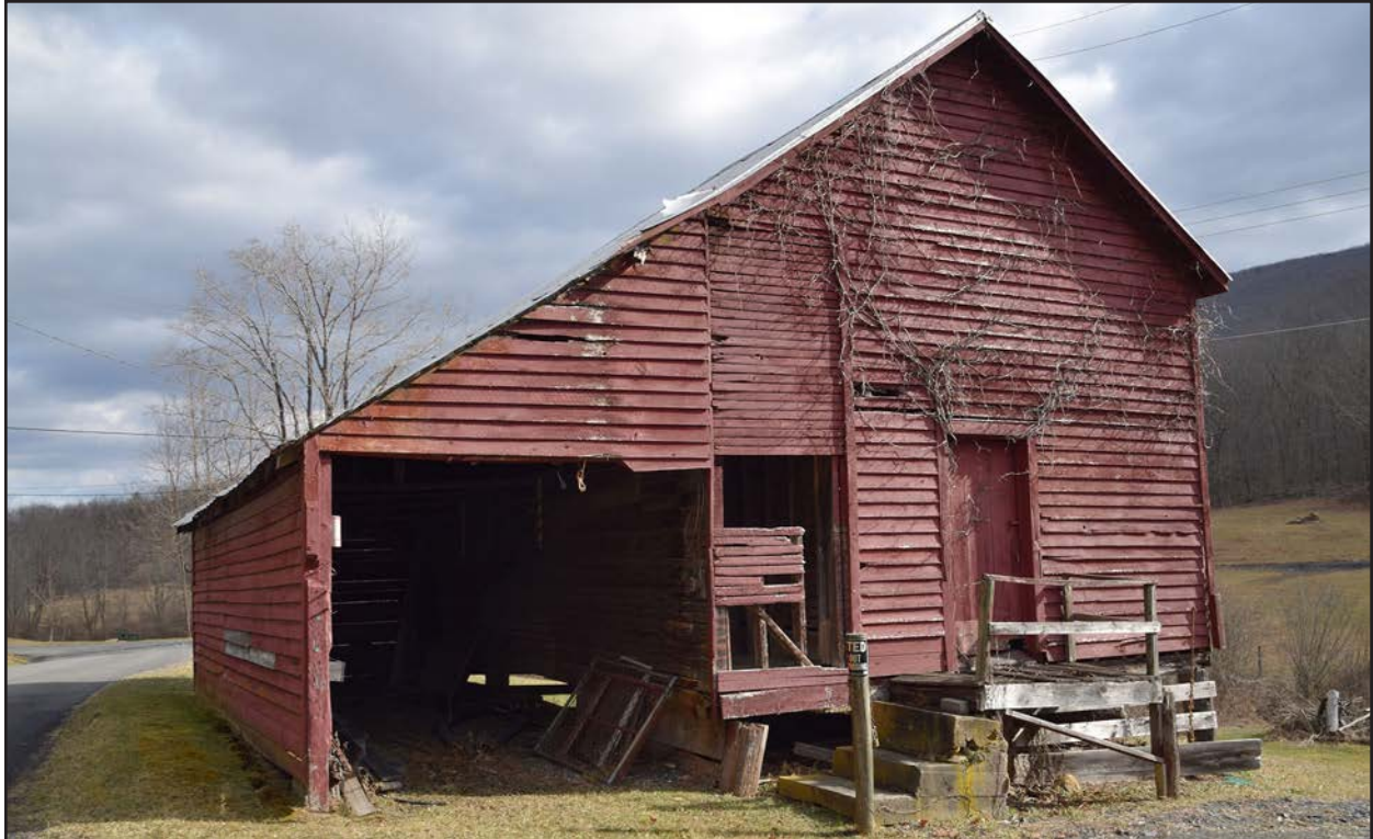
Figure 44. 008-5068, north barn, side detail, facing north.
