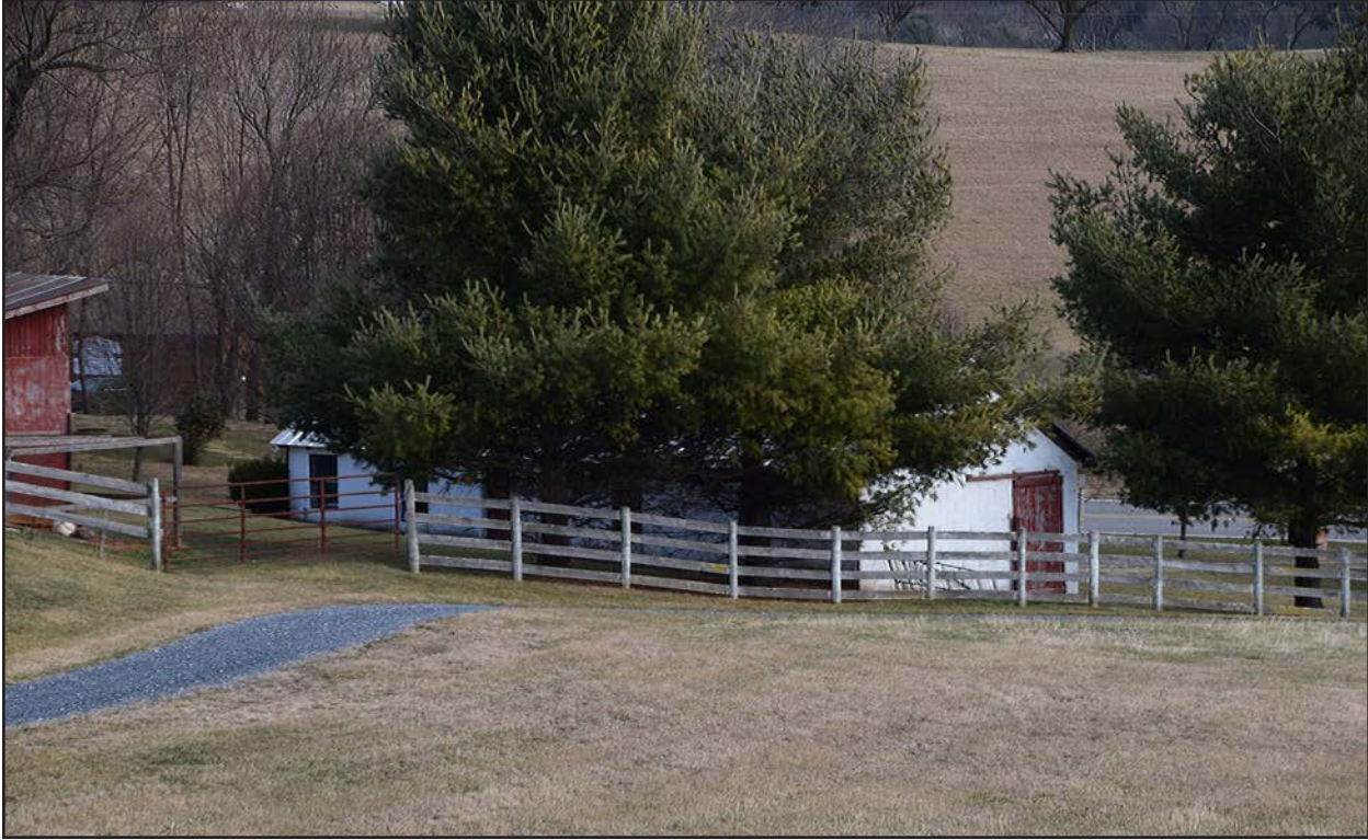
Figure 26. 007-5584, concrete block building, facing northeast.
