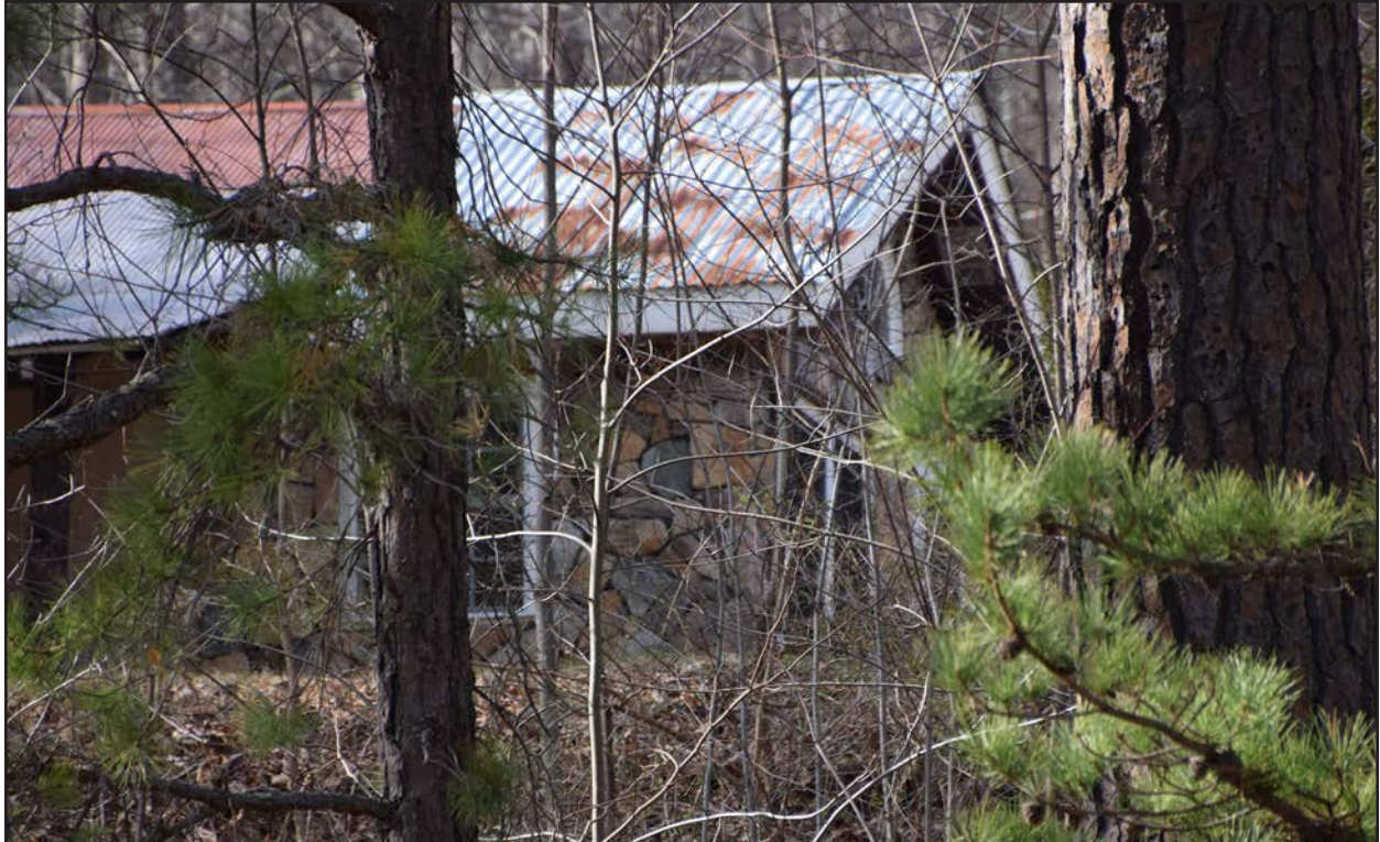
Figure 18. 007-5556, northeast addition, facing west.
