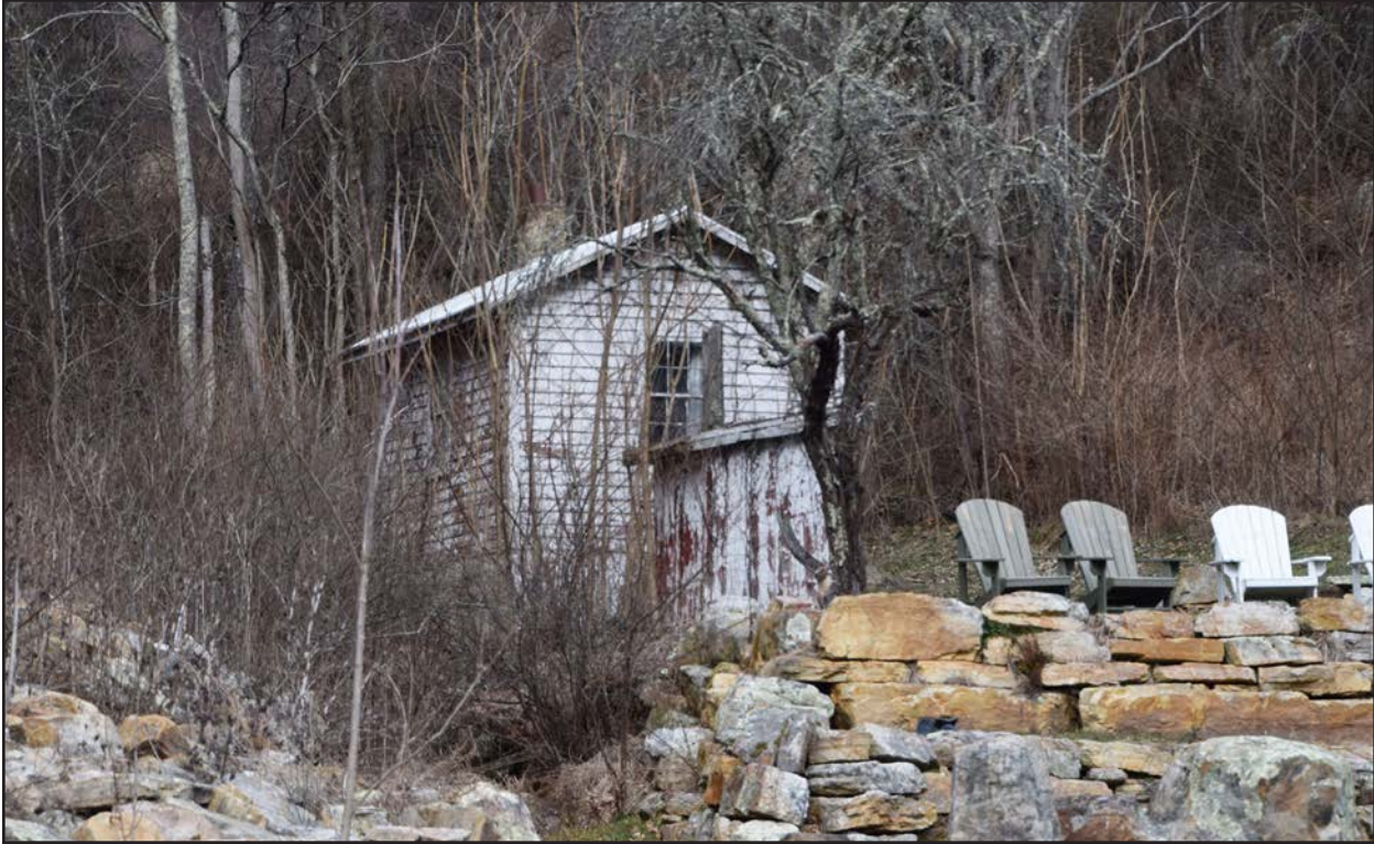
Figure 41. 008-5068, outbuildings, detail, facing northwest.
