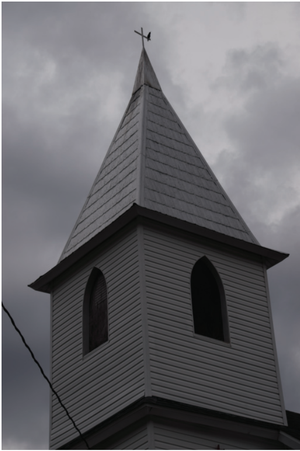
UP-0113, Gothic Revival Church, bell tower, facing northeast.
