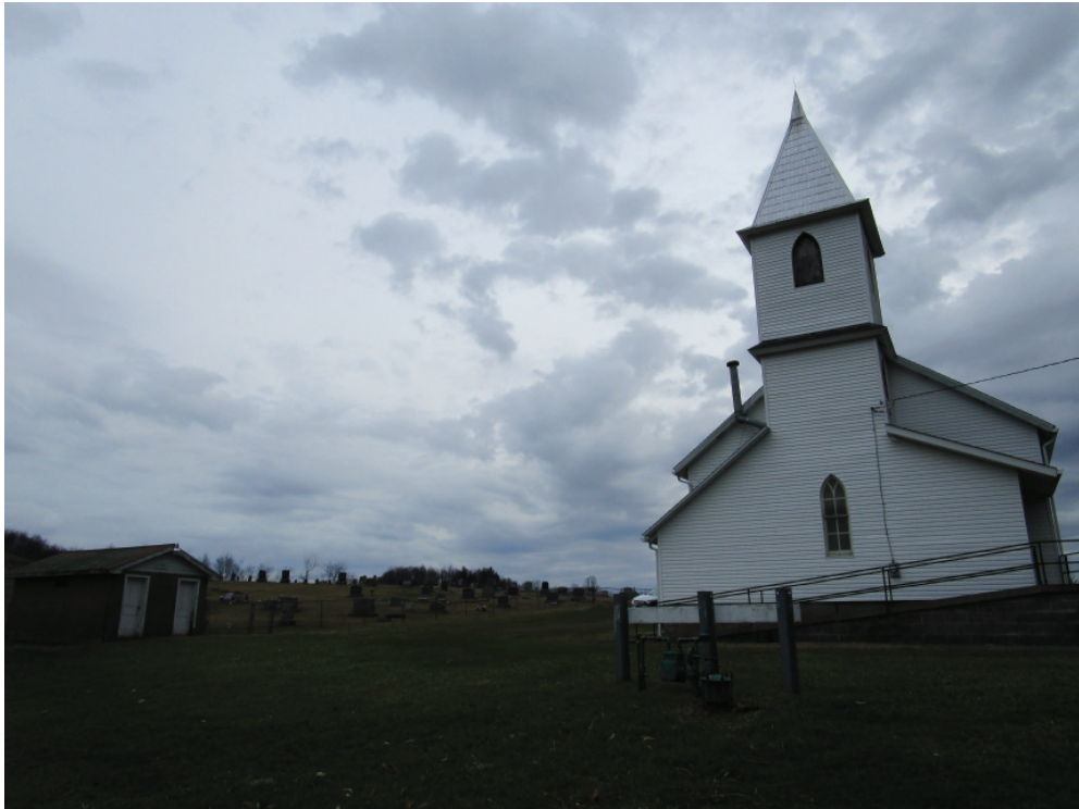
UP-0113 and 46-UP-348, Gothic Revival Church, Shed and Cemetery, facing northeast.
