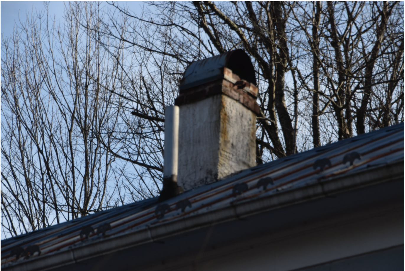
PH-0470, chimney detail, facing southwest.
