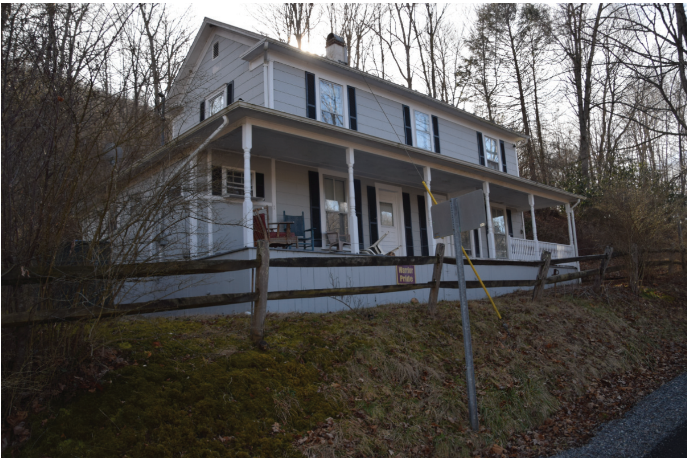
PH-0470, facing southwest.
