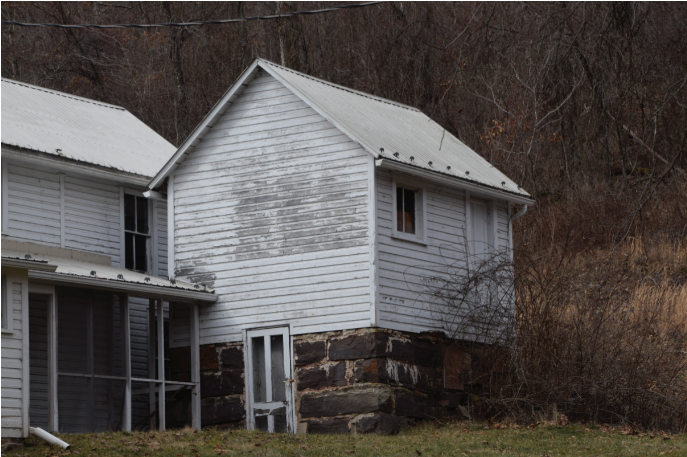
PH-0037-64, smokehouse/root cellar, facing northwest.
