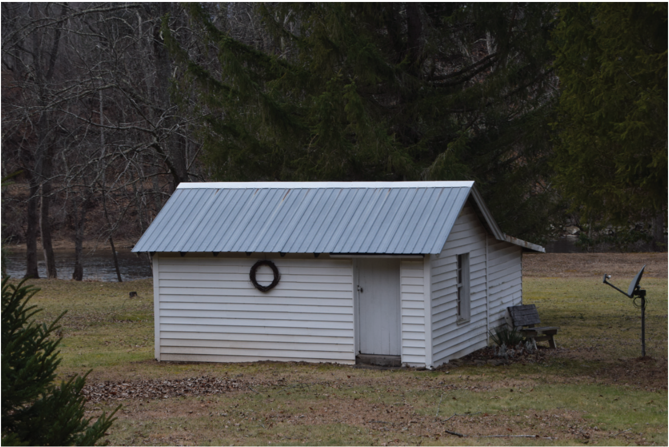
PH-0490, Shed, facing northwest.
