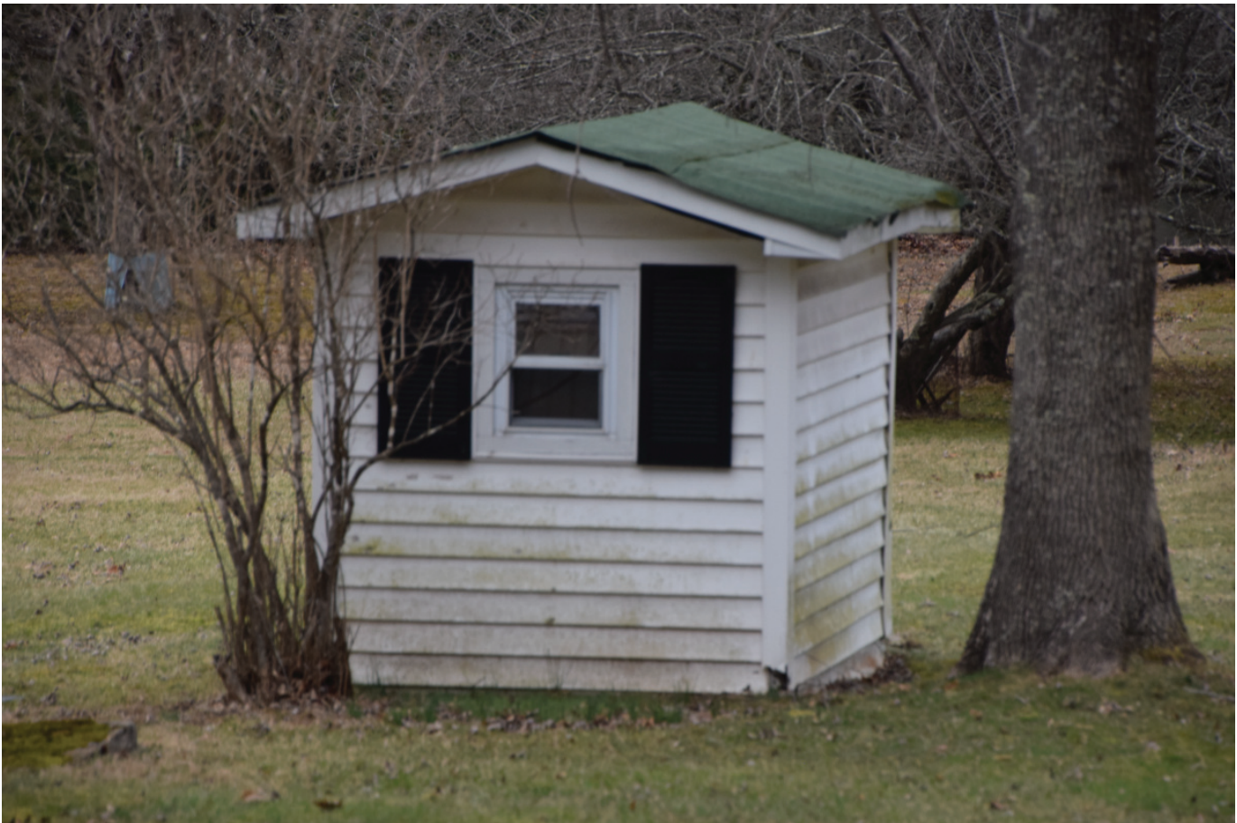
PH-0490, Well House, facing northwest.
