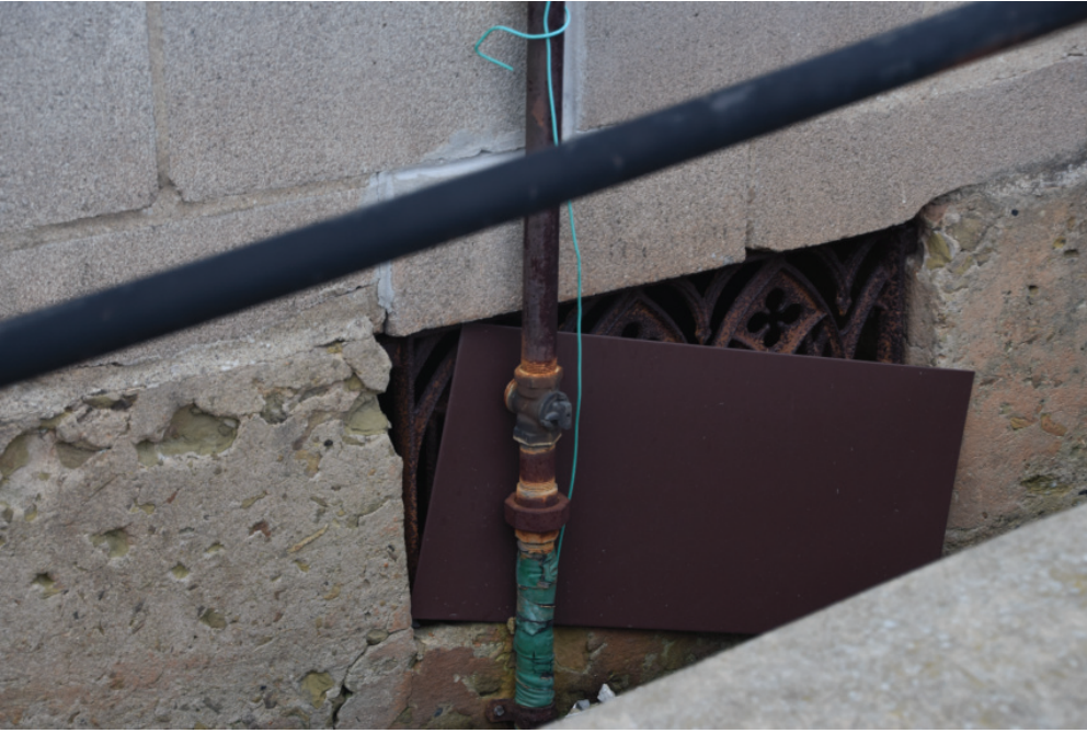
UP-0113, Gothic Revival Church, foundation detail, facing north.
