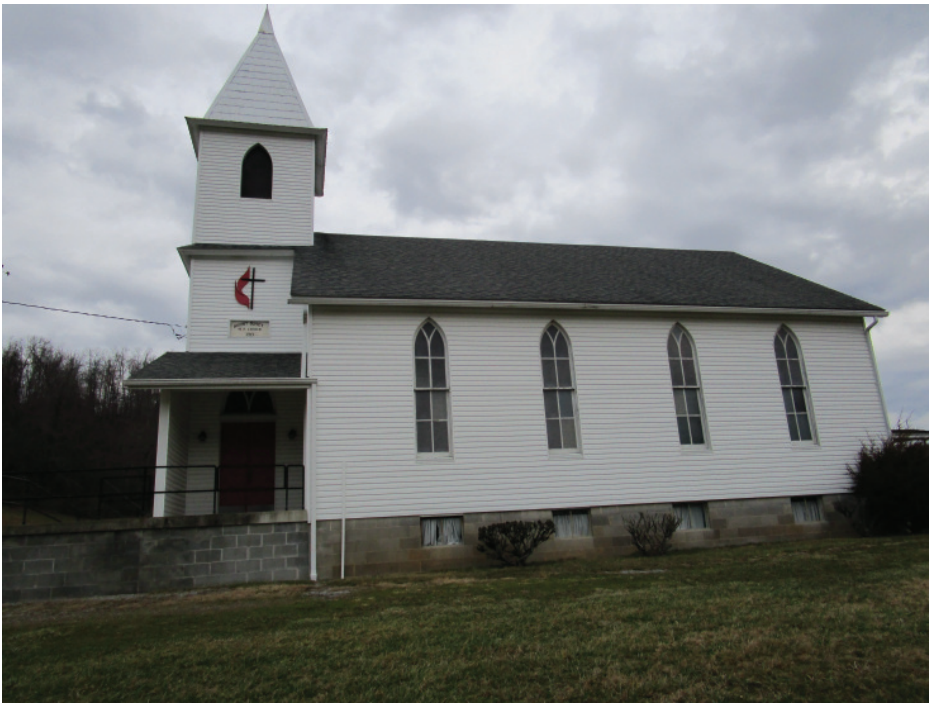
UP-0113, Gothic Revival Church, facing north.
