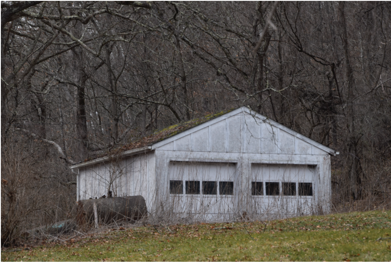
PH-0037-64, garage, facing west.
