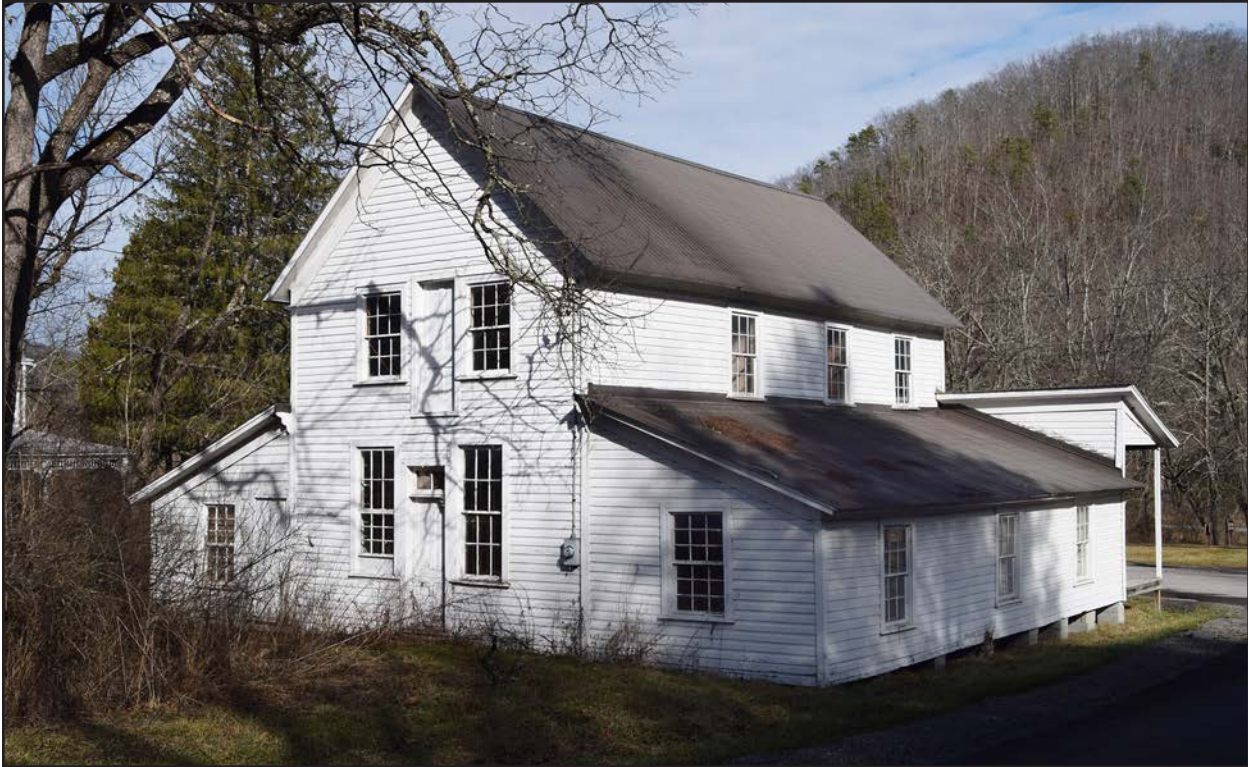
Photo 8. PH-0037-65, store, facing east.
