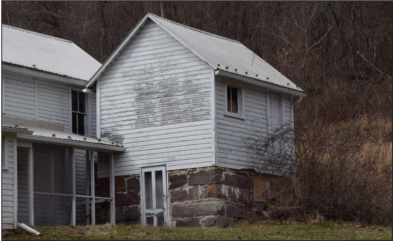
Photo 3. PH-0037-64 smokehouse/root cellar, facing northwest.
