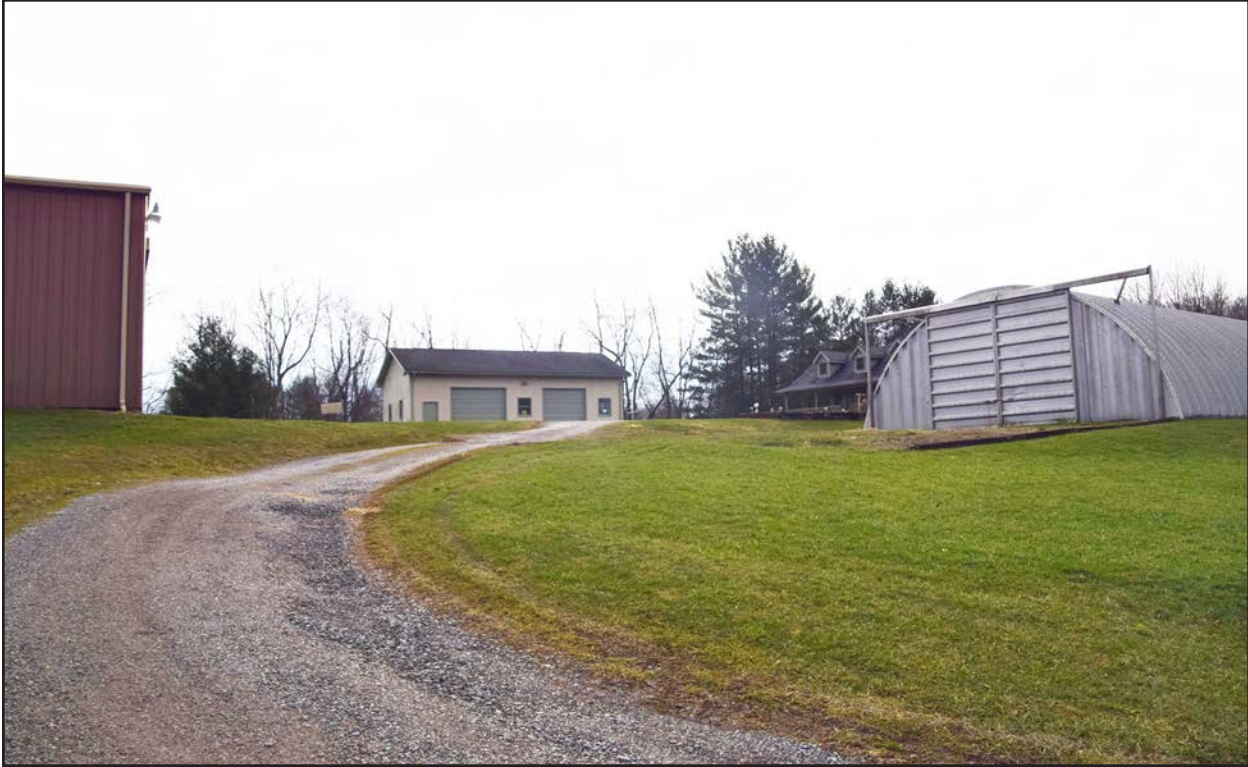
Photo 29. UP-0818, outbuildings, facing southeast.
