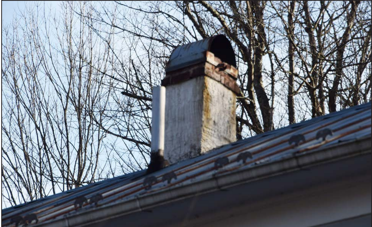
Photo 16. PH-0470, chimney detail, facing southwest.
