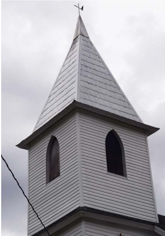
Photo 33. UP-0113, Gothic Revival Church, bell tower, facing northeast.
