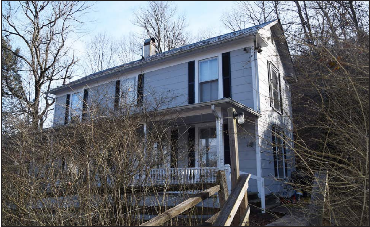
Photo 19. PH-0470, facing southeast.
