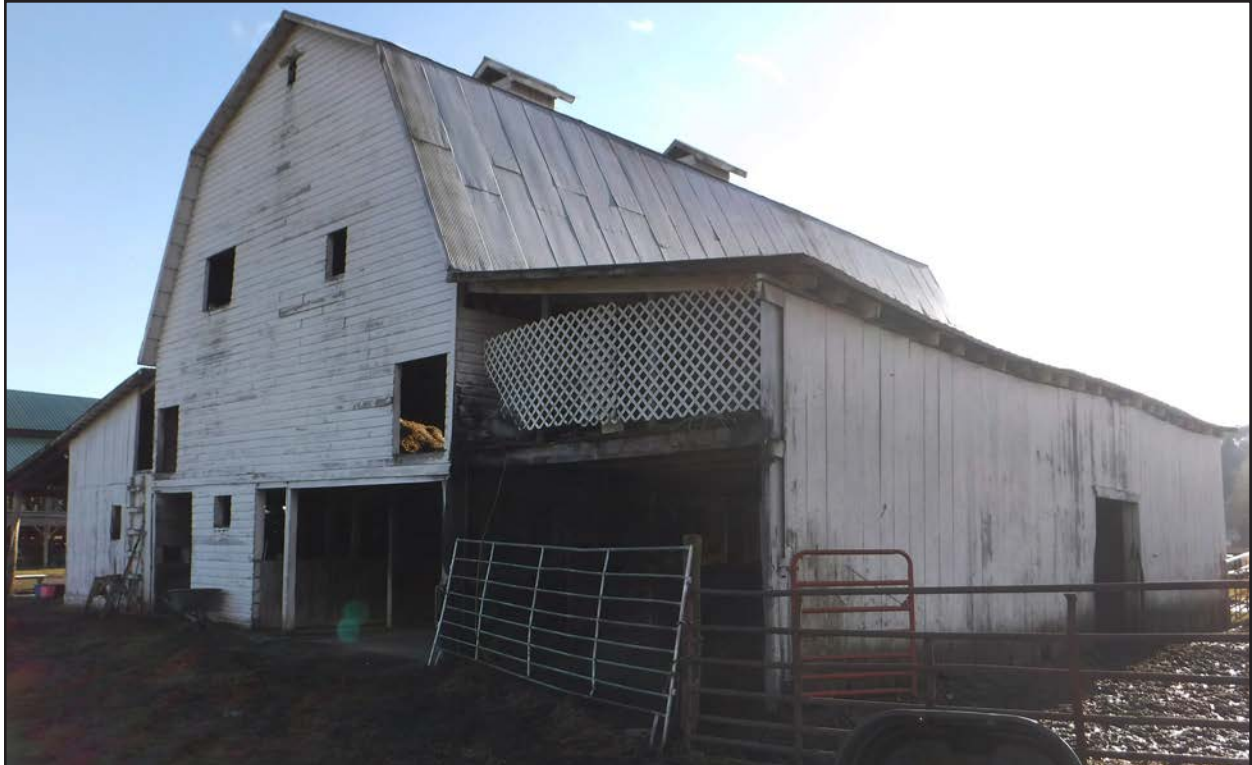
Photo 26. PH-0954, facing south.
