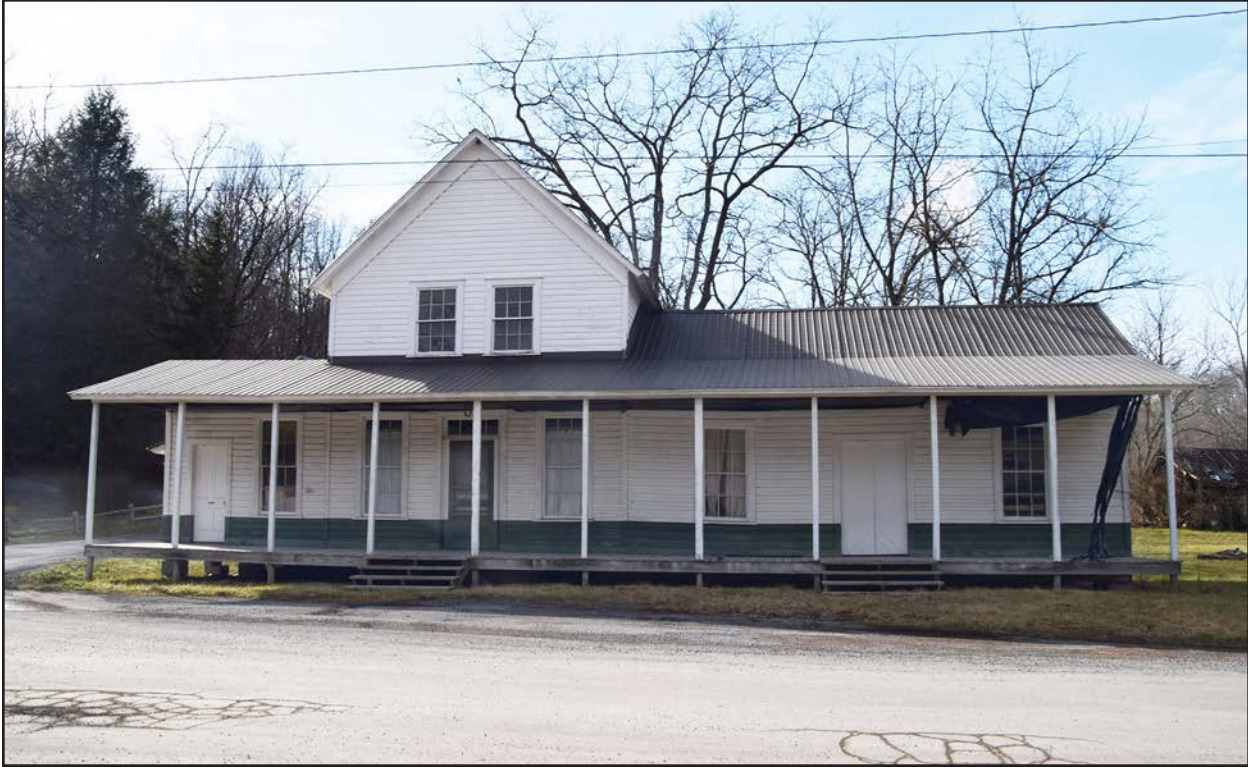
Photo 7. PH-0037-65, store, facing west.
