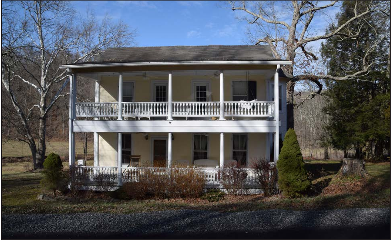
Photo 11. PH-0462, facing north.
