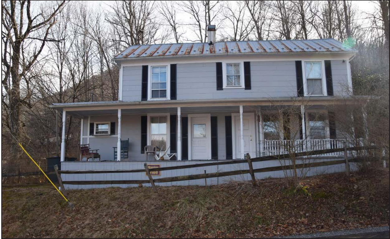
Photo 15. PH-0470, facing south.
