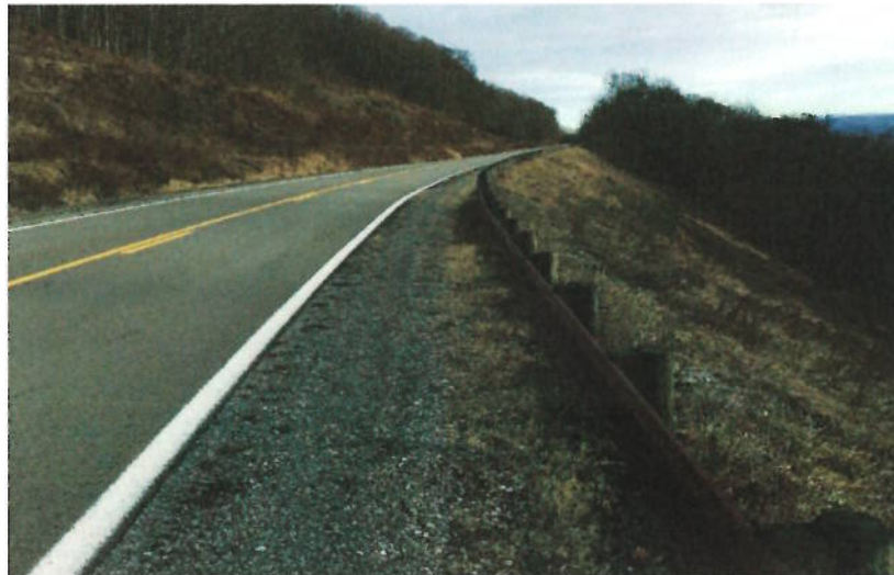
Photo 14 – Landslide Group 4 – SR 150 Red Lick Slip fill slope site –19-Jan-2017– GEO_0804 This is a large road fill site where movement may be ongoing but no landslide was observed.
