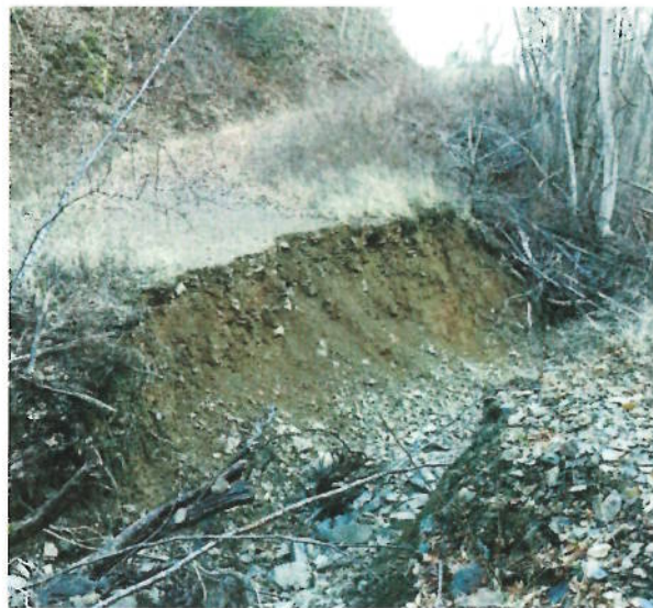
Photo 04 – Landslide Group 1 – FR 719 – Debris Flow Culvert Washout – 18-Jan-2017 GEO_0777 This location was not assigned a Landslide Point, but was observed to be a significant culvert washout.
