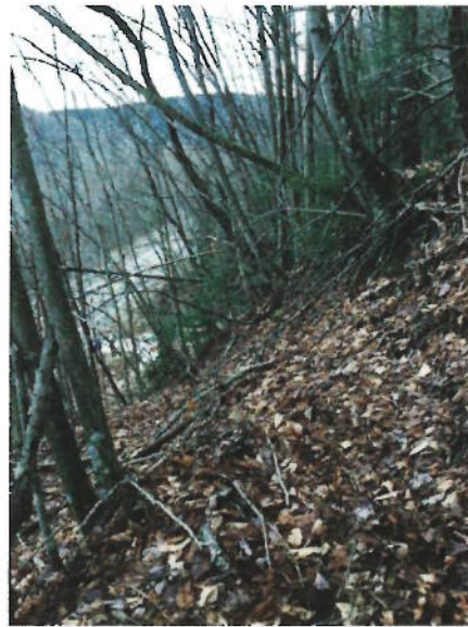
Photo 11 – Landslide Group 4 – SR 150 Highland Scenic Highway Landslide –19-Jan-2017– GEO_0792 Highway construction resulted in significant excavation into the toe of this large landslide which extends over 1,000 feet upslope and there appears to be ongoing cut slope maintenance issues here.
