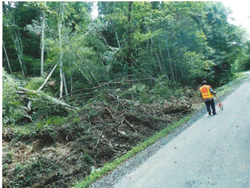
Photo 09 – Landslide Group 3 – FR 86 – MP 14.7 Williams River Road –26-Jul-2016 FS_P7260421 Pre-existing landslide site on the west side of the Williams River that appears to have been recently reactivated by high-intensity precipitation. Geosyntec was unable to visit this site.
