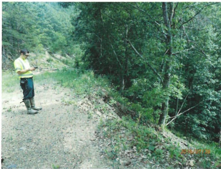
Photo 03 – Landslide Group 1 – FR 719 – Unidentified road fill failure – 28-Jul-2016 FS_P7280791 Evidence that surface runoff ponded on the roadway is visible left of the individual shown. This likely raised pore water pressure in the road fill which failed and subsequently erosion of the fill occurred.
