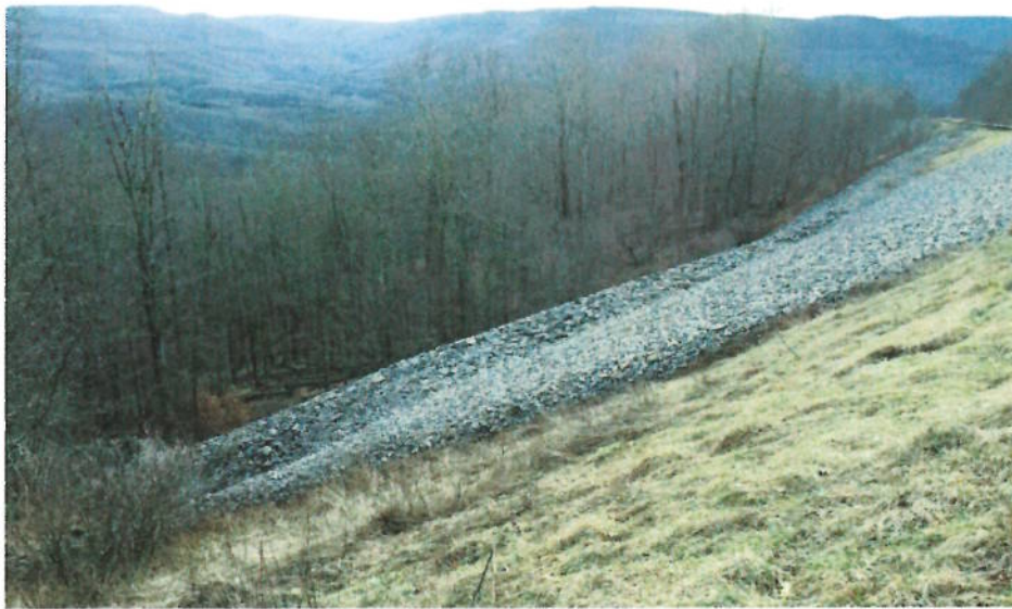
Photo 13 – Landslide Group 4 – SR 150 Honeycomb Rocks Slip fill slope –19-Jan-2017– GEO_0792 Forest Service photos show erosion of a lined culvert discharge channel at the toe of the buttressed large road fill movement site (culvert is in lower left corner of photo).
