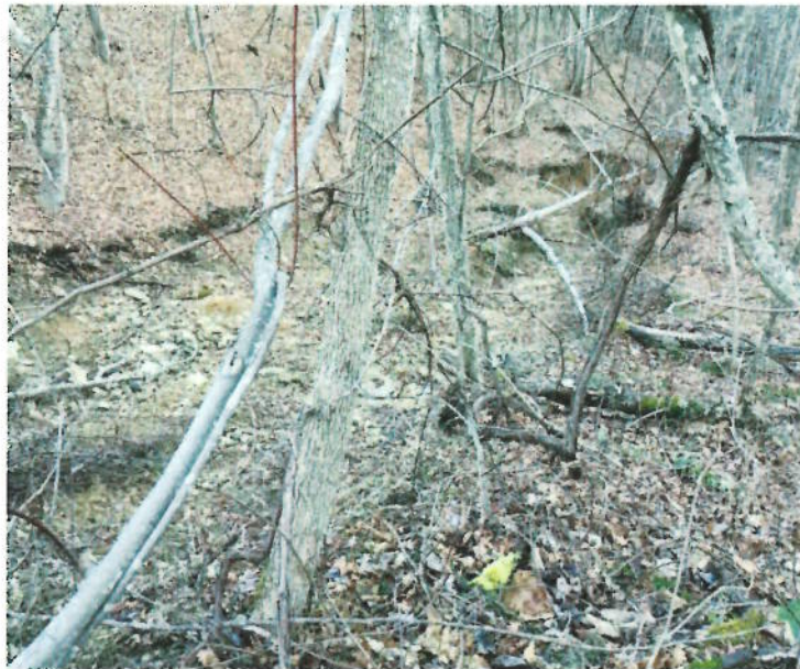
Photo 05 – Landslide Group 1 – FR 719 – Road Fill Erosion Site “C” – 18-Jan-2017 GEO_0779 Runoff across the roadway (located above and left), resulting from a plugged culvert inlet, caused some erosion of the road fill and the cutting of a new erosion channel on the hillside below (right).
