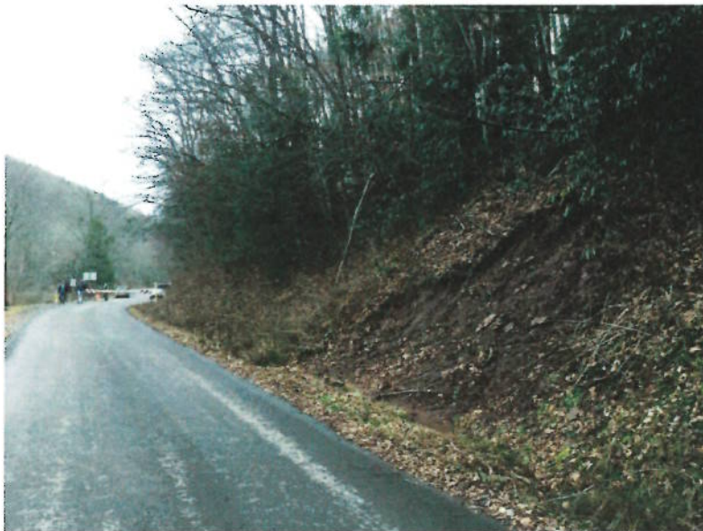
Photo 12 – Landslide Group 4 – FR 86 Cut slope failure -Tea Creek Campsite–19-Jan-2017–GEO_0800 On west side of Williams River a small cut slope failure occurred at the toe of an existing landslide.
