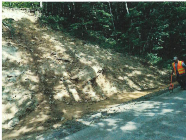
Photo 10 – Landslide Group 3 – FR 86 – MP 15.9 Williams River Road –26-Jun-2016 FS_P7260488 Cut slope failure on east side of the Williams River. Geosyntec was unable to visit this site.
