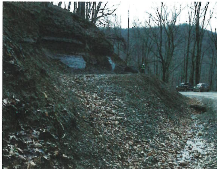
Photo 08 – Landslide Group 2 – FR 101 – Cut Slope Failure Repair –19-Jan-2017 GEO_0784 Fifteen Landslide Points were attributed to this one cut slope failure site (seen here after repair work).
