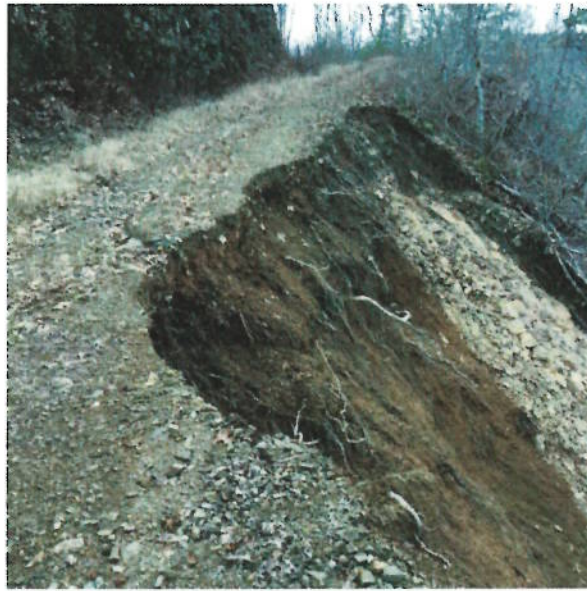
Photo 01 – Landslide Group 1 – FR 719 - Road Fill Failure Site “H/L” – 18-Jan-2017 GEO_0771 A sliver road fill was constructed over shallow steeply dipping bedrock. There is evidence that significant surface runoff flowed down the road and seeped into the road fill causing it to fail.
