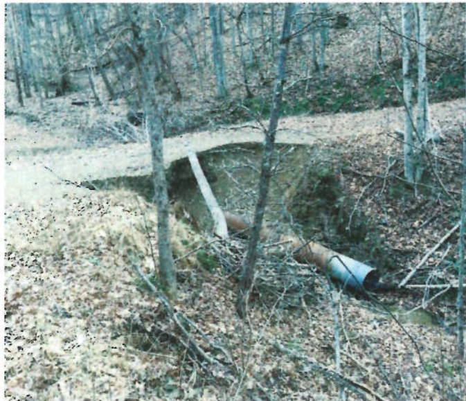
Photo 02 – Landslide Group 1 – FR 719 – Culvert Washout Site “G” - 18-Jan-2017 GEO_0774 An existing culvert inlet appears to have plugged and runoff crossed the roadway eroding the road fill.
