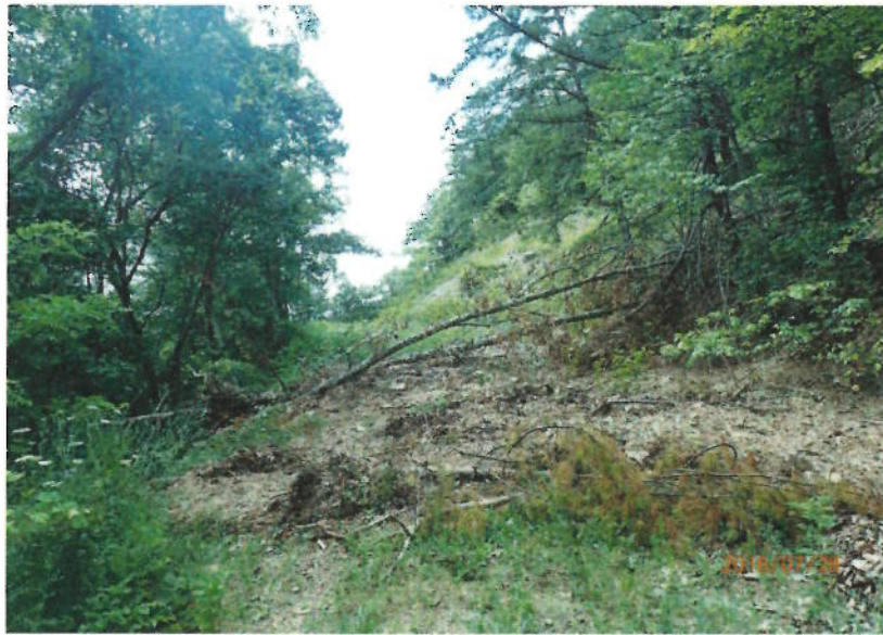
Photo 07 – Landslide Group 1 – FR 719 – Unidentified road cut erosion –28-Jul-2016 FS_P7280807 Significant runoff from hillside above and to the right resulted in erosion of the cut slope and deposition of soil, rock, and other debris on the existing road surface.
