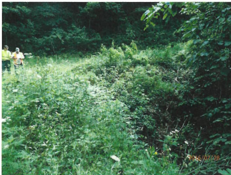
Photo 06 – Landslide Group 1 – FR 719 – Unidentified road fill failure – 28-Jul-2016 FS_P7280818 Fill failure and erosion caused by creek runoff diverted onto road at plugged culvert inlet (top right).
